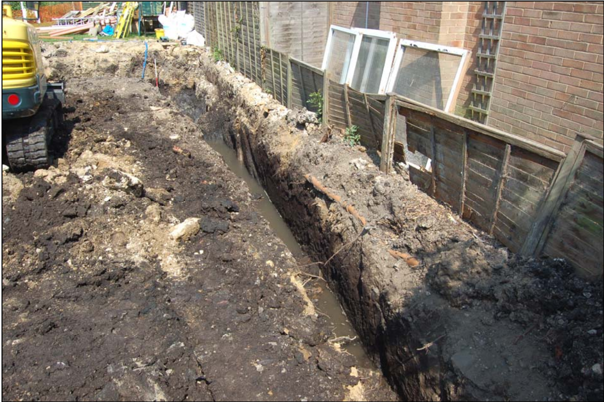
Plate 1 Working shot during excavation through organic deposit 3, viewed to north-west
