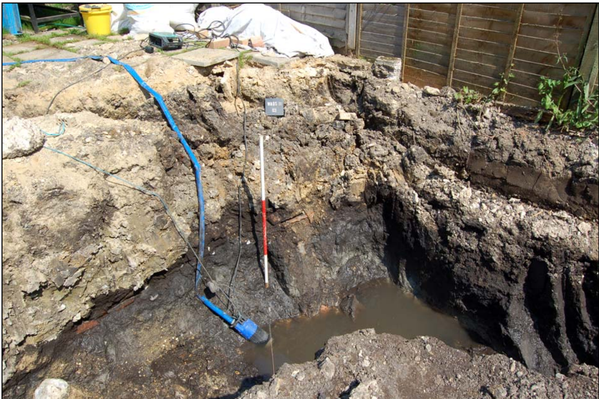
Plate 2 Context 3 in north corner of monitoring trench (1.5m scale)
