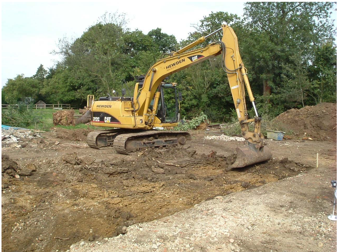
Plate 2 Topsoil stripping of house footprint
