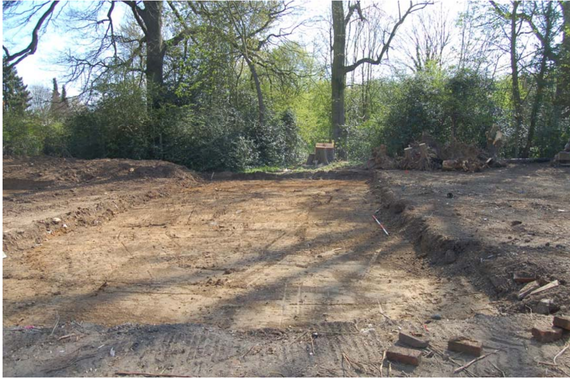
Plate 3 Garage area following topsoil stripping
