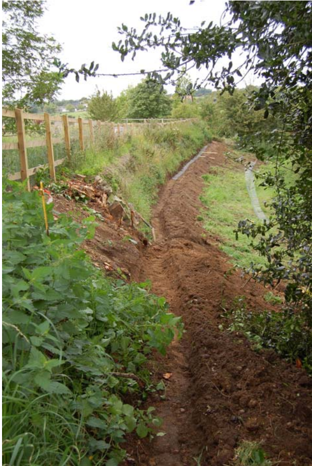
Plate 5 Trench along the churchyard wall
