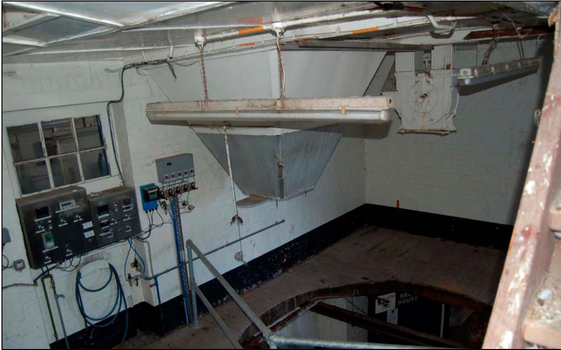
Plate 48 Mashing room viewed to north-west
