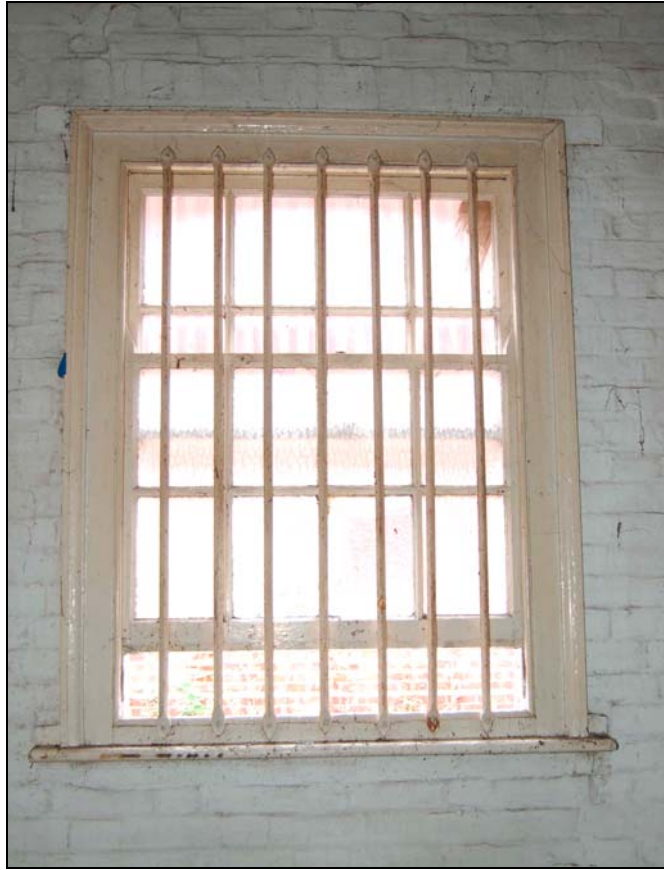
Plate 17 Typical barred sash window
