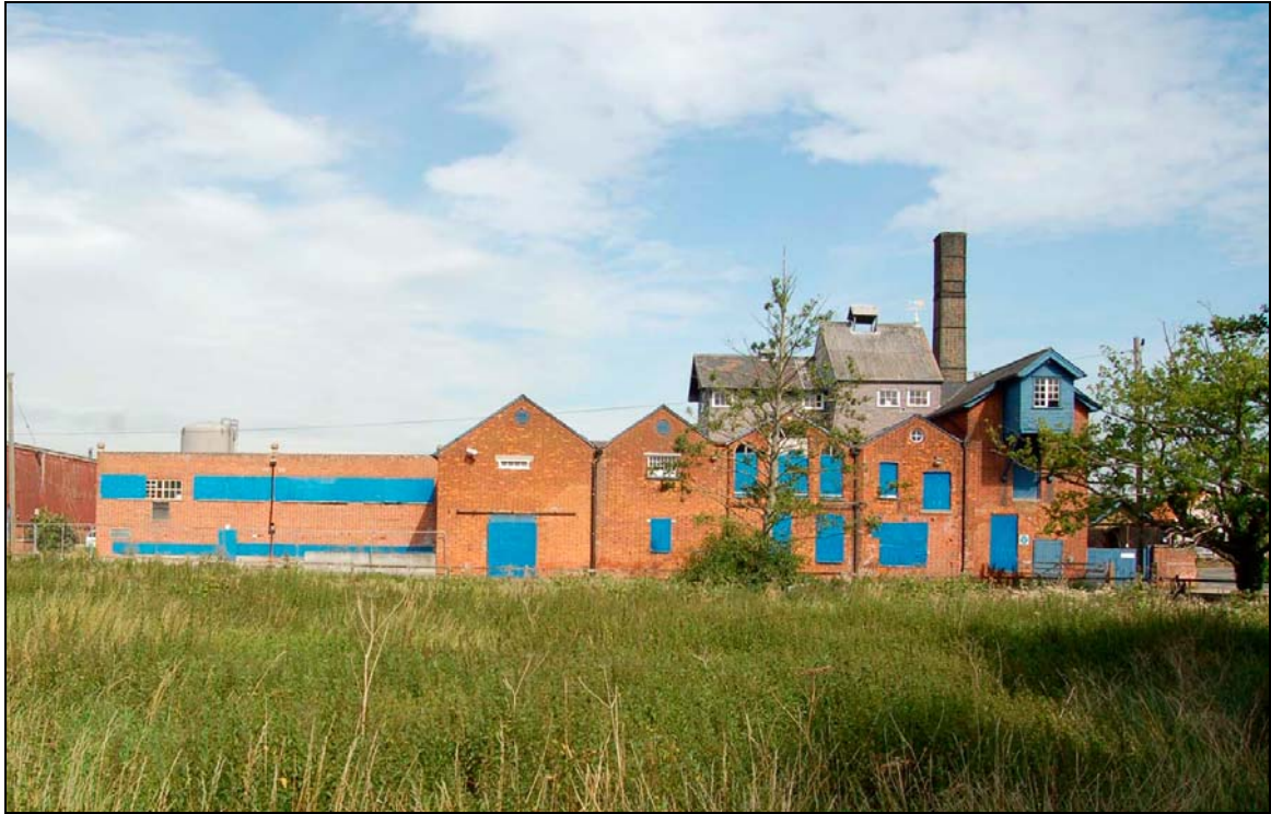
Plate 1 Main elevation viewed to north-west
