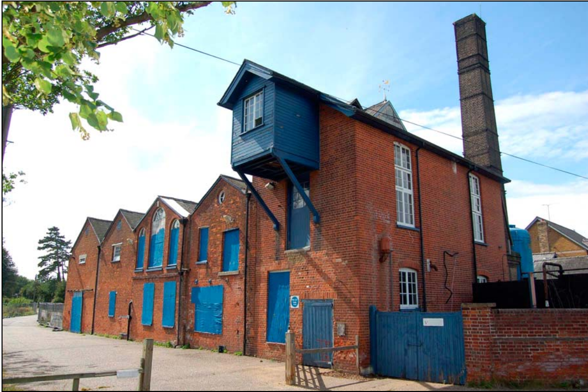
Plate 5 Brewhouse viewed to north-west
