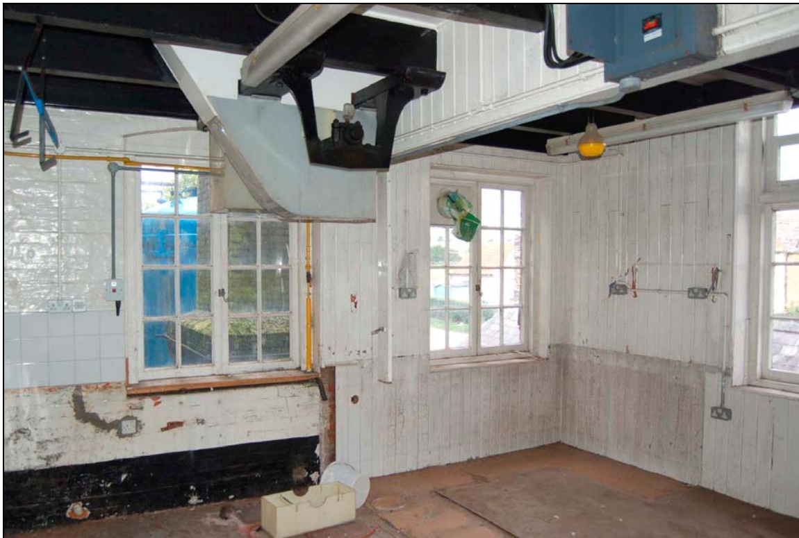
Plate 47 Enclosed drive wheels in laboratory for chain hoist above
