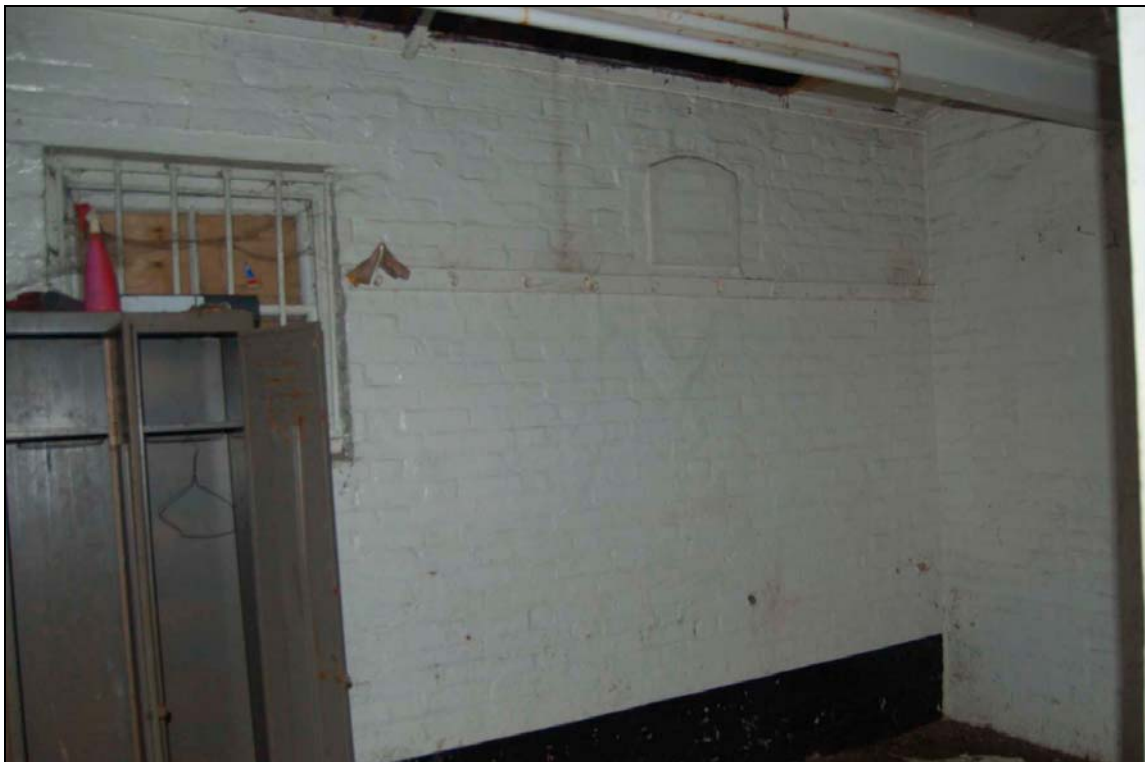
Plate 16 Bearing box and blocked ?band aperture in staff room 5
