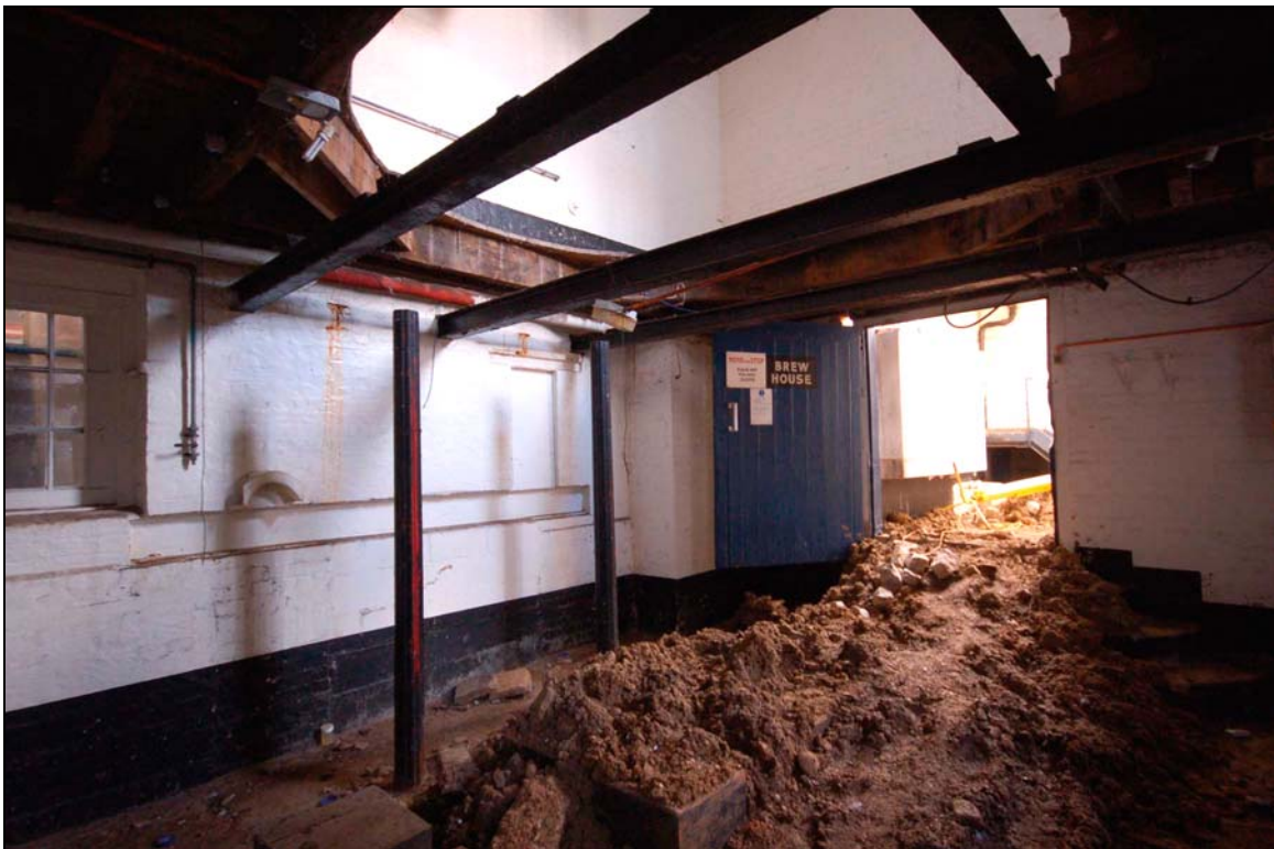
Plate 30 Engine room viewed to north-west
