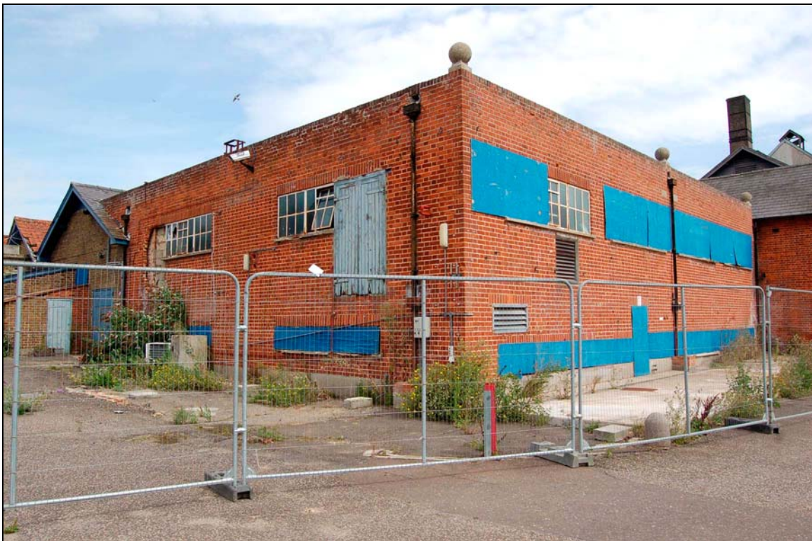
Plate 6 Conditioning plant viewed to north-east
