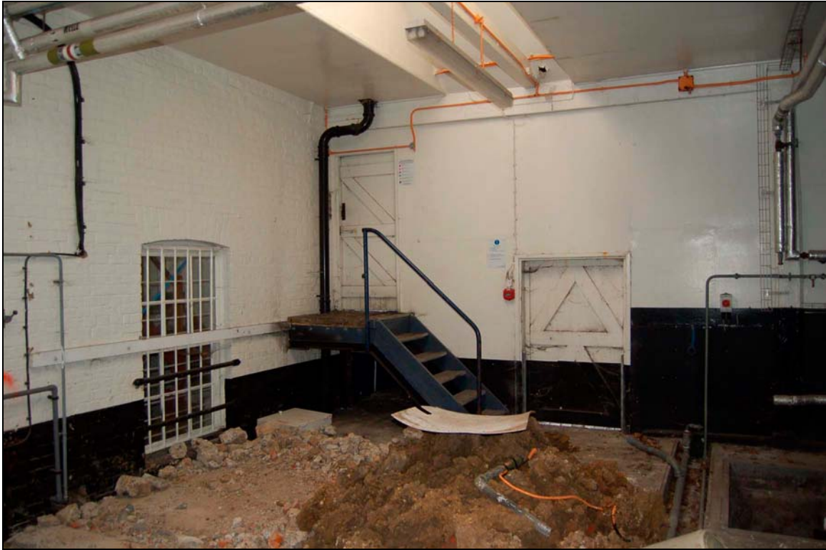
Plate 31 Cask repair area viewed to north-west
