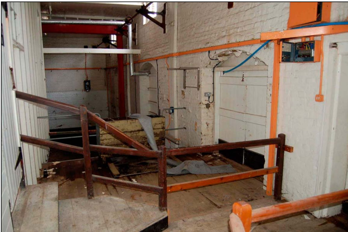
Plate 36 Platform 4 viewed to north-west showing overhead line-shafting
