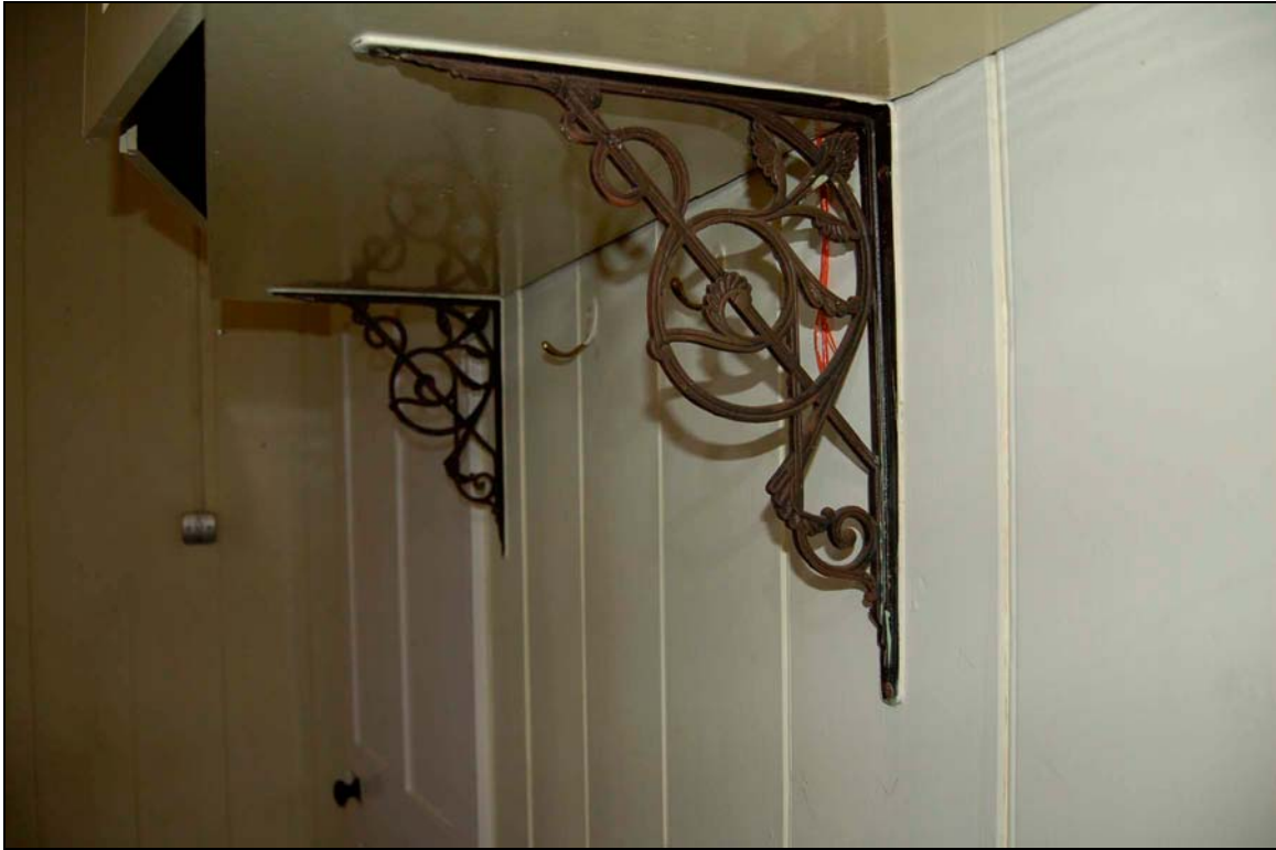
Plate 52 Brackets for fitted cupboards
