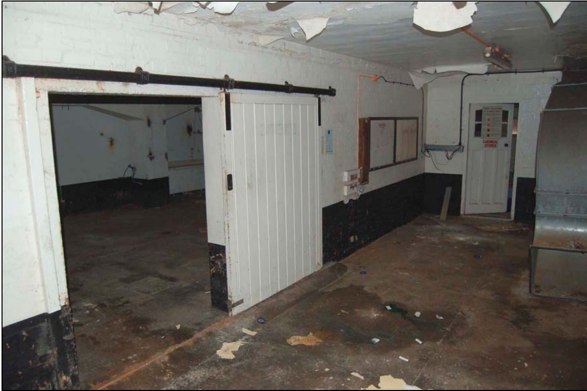
Plate 19 Compressor room viewed to east
