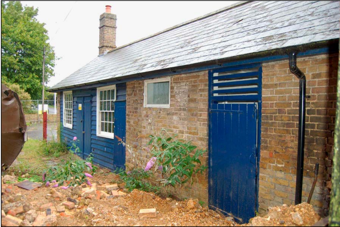
Plate 62 Cooper's shop viewed to north
