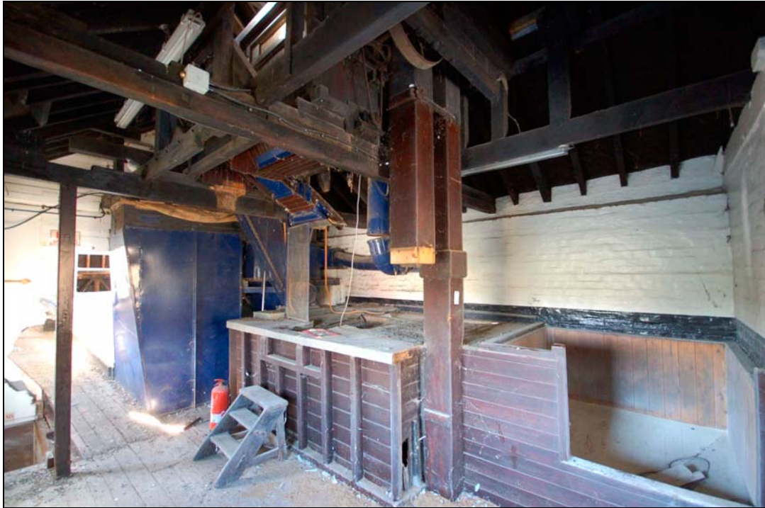
Plate 56 Mill room viewed to south-east
