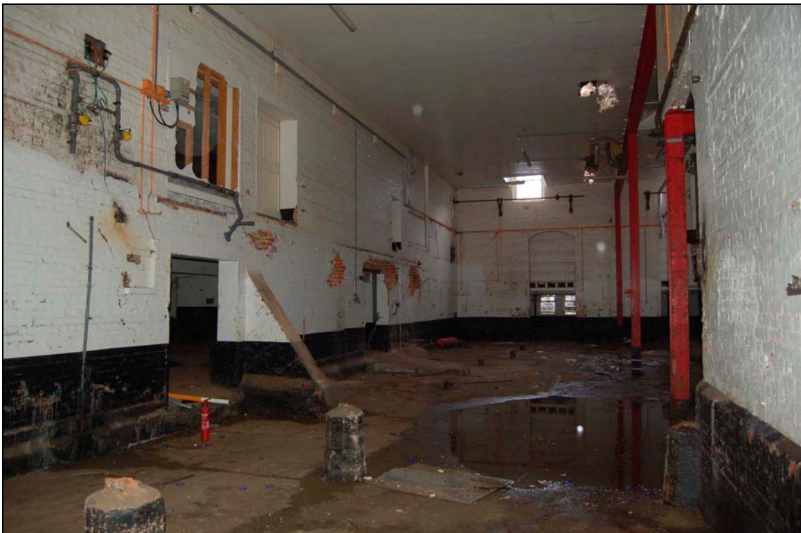
Plate 24 Brewing hall viewed to north-west
