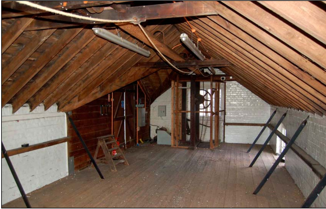
Plate 54 Malt and hop store viewed to north-west
