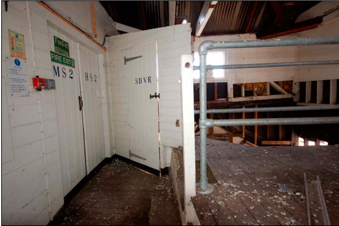
Plate 60 Typical Victorian door form (into malt/hop store and sugar dissolving room)
