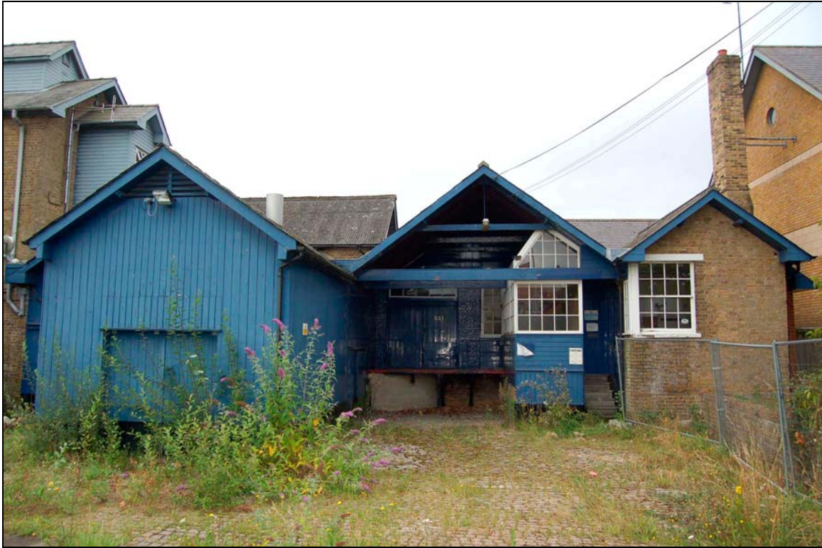
Plate 9 Dispatch/offices area viewed to north-west
