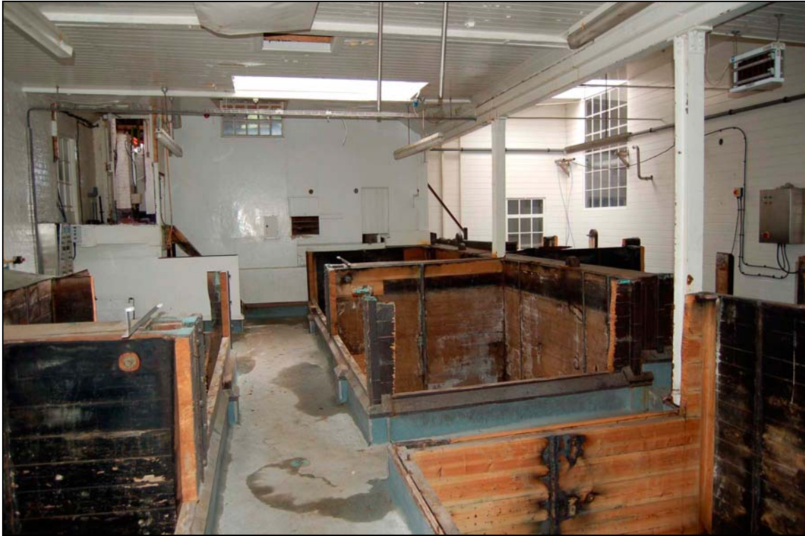
Plate 40 Fermentation room viewed to south-east (hopback)
