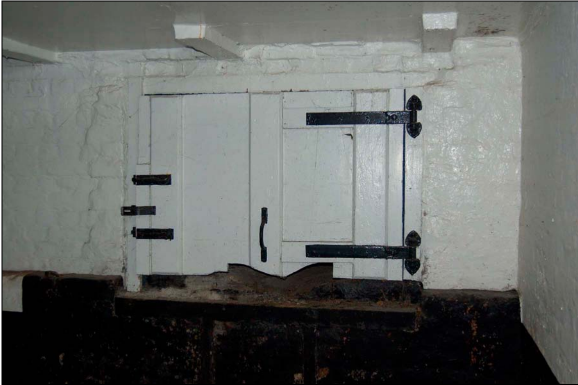
Plate 27 Door from cask repair area into cask fill room
