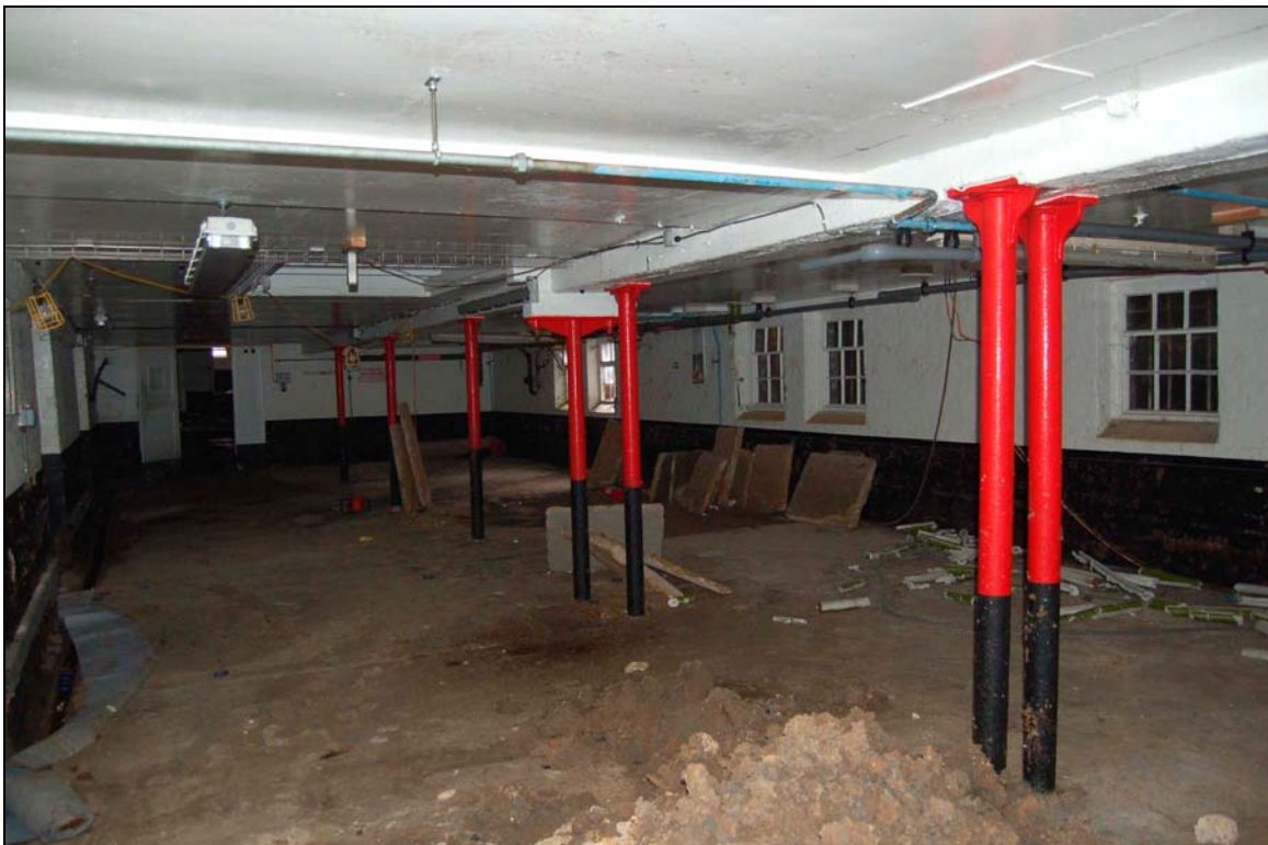
Plate 26 Cask fill area viewed to south-west
