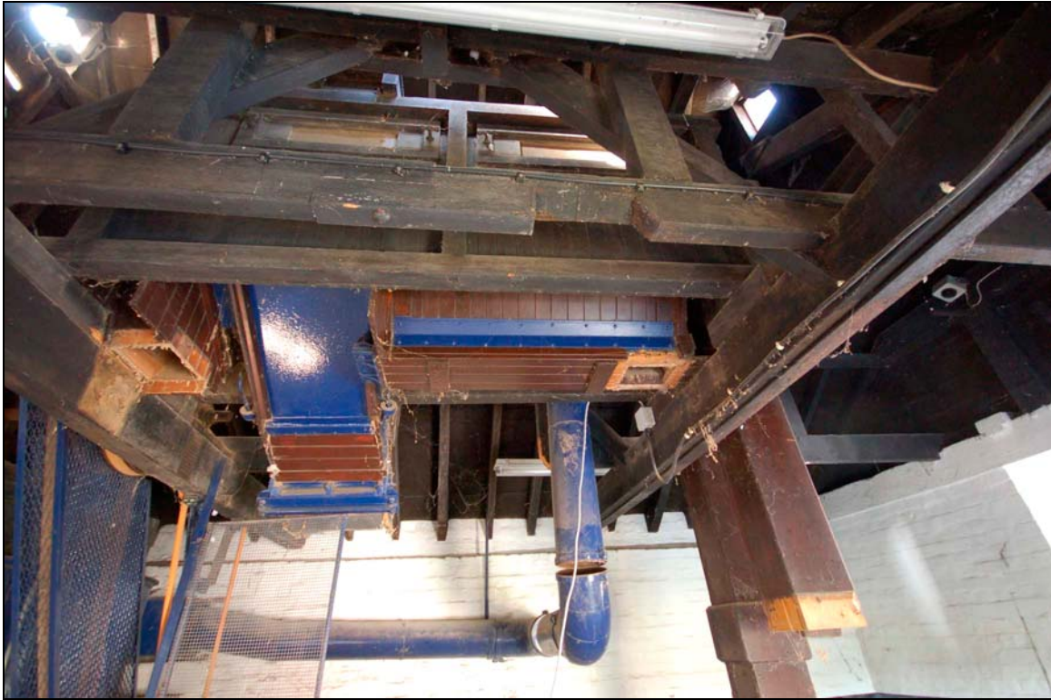
Plate 58 Malt mill and chutes viewed to south-west
