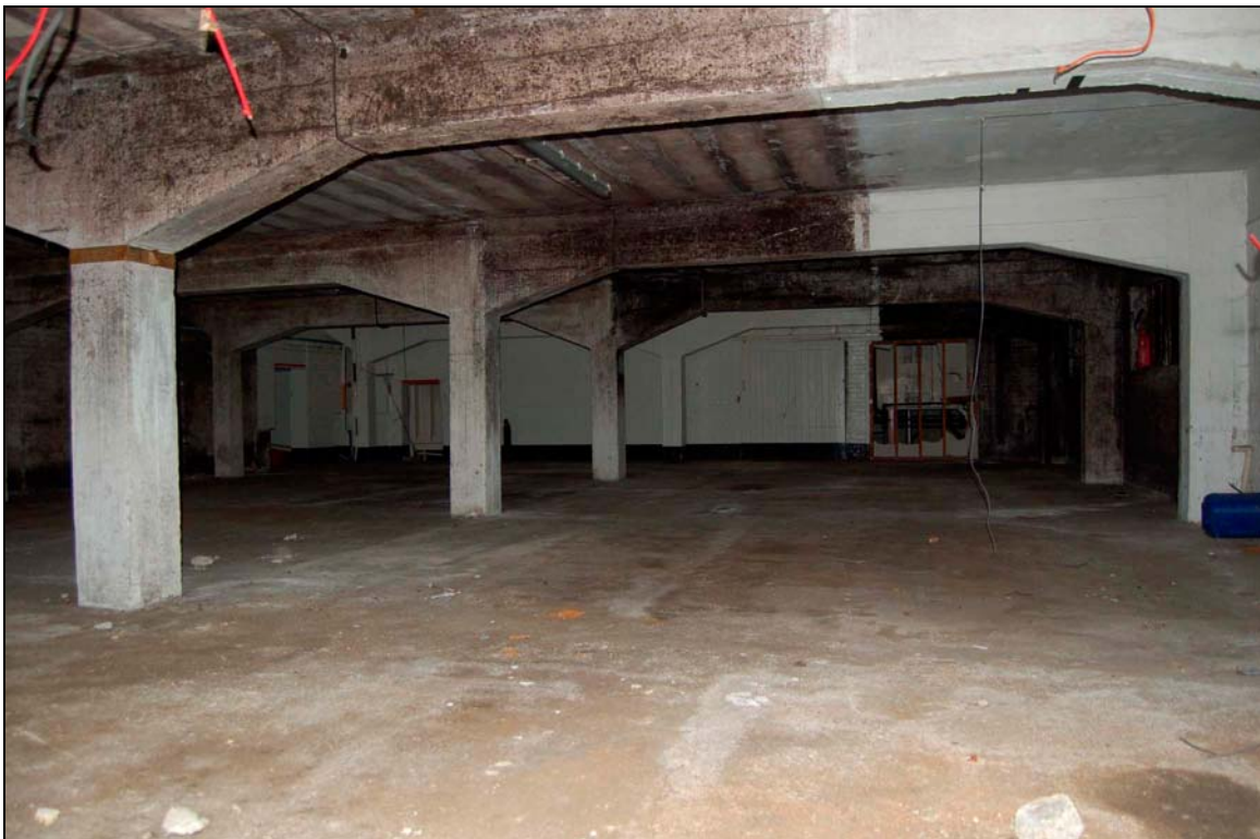
Plate 32 First floor of conditioning room stores viewed to north-east (brewing hall)
