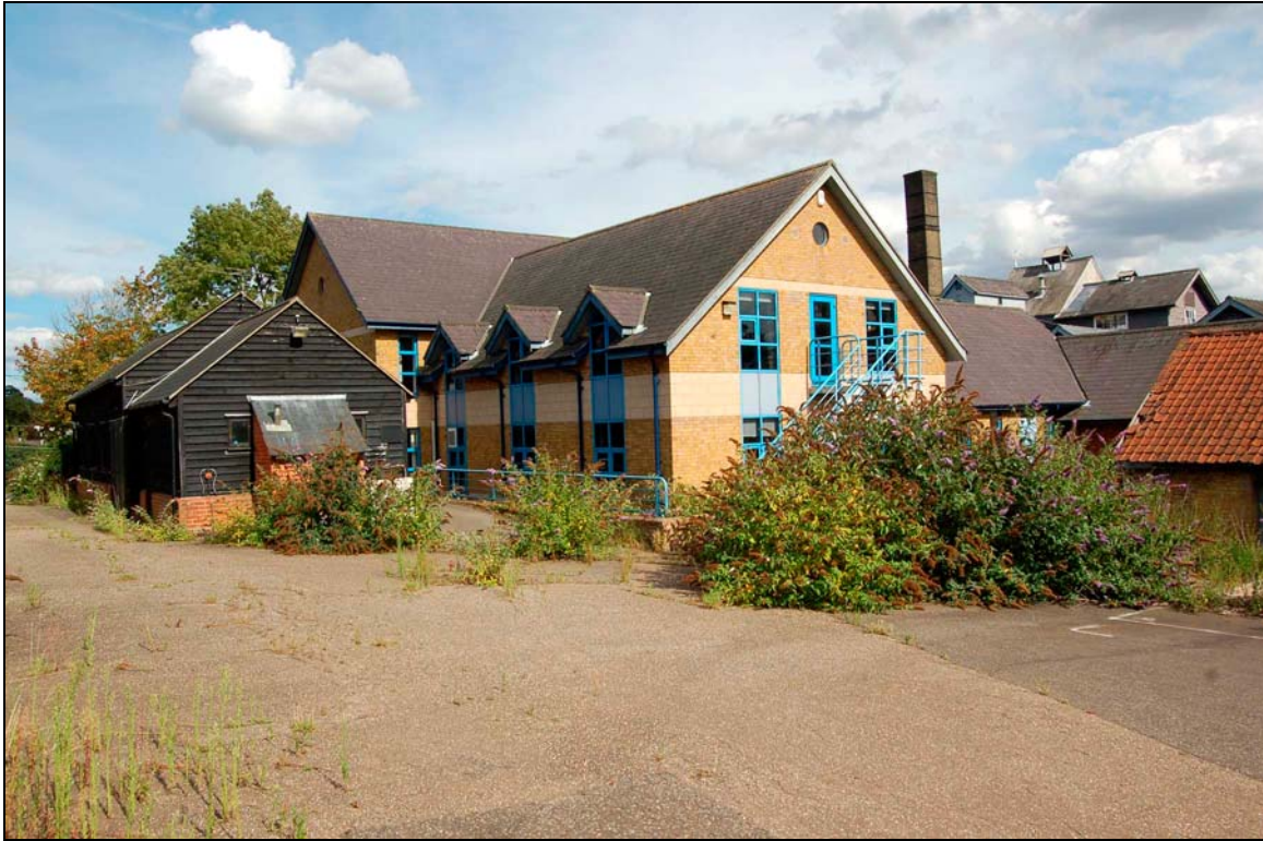
Plate 11 Modern offices attached to north-west end of brewhouse
