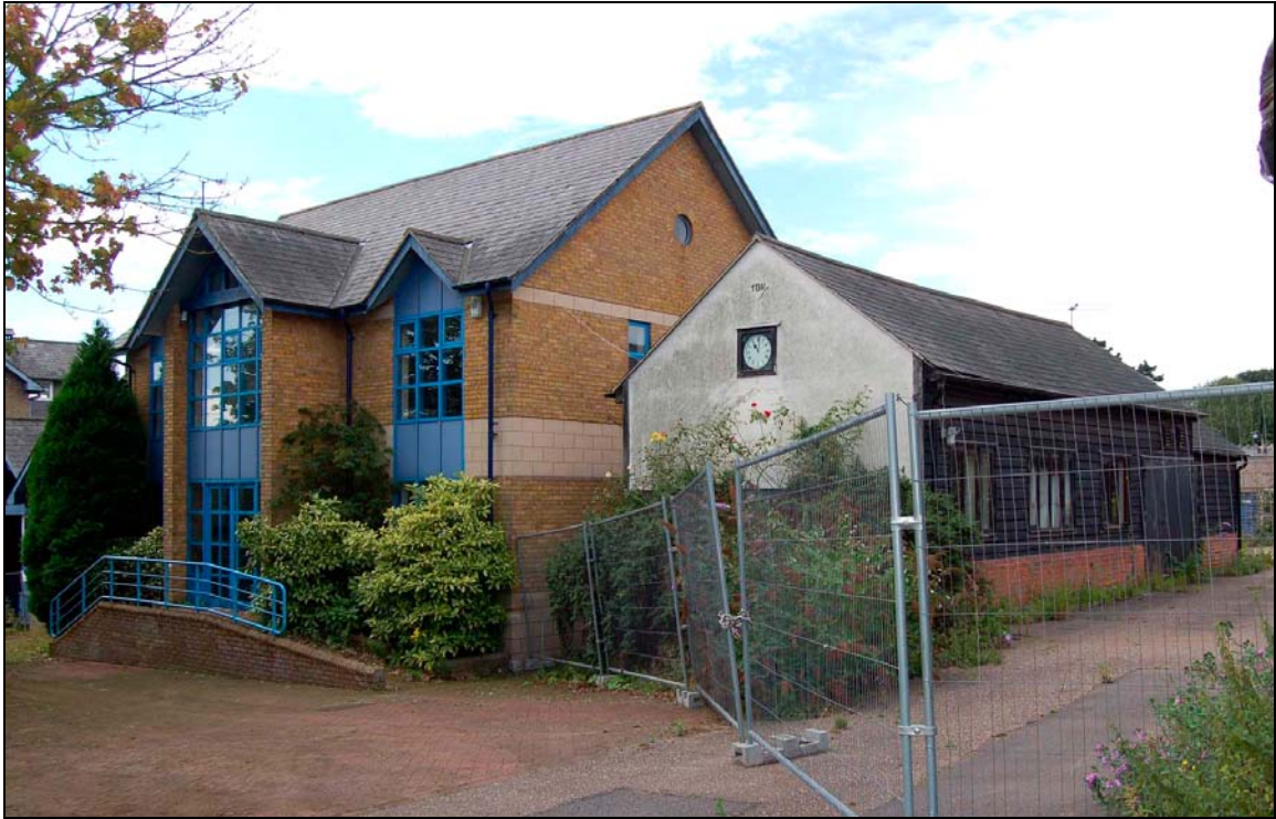
Plate 68 Modern offices and clockhouse viewed to south
