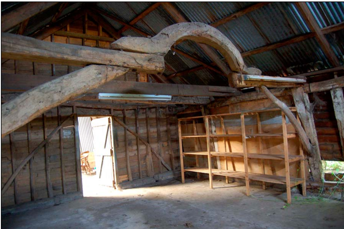
Plate 65 Raised tie beam in cart bay viewed to west
