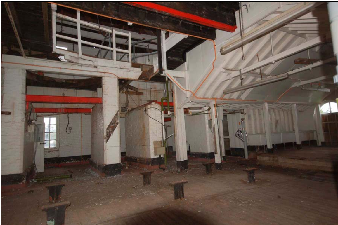
Plate 43 Hopback base and piers for coppers
