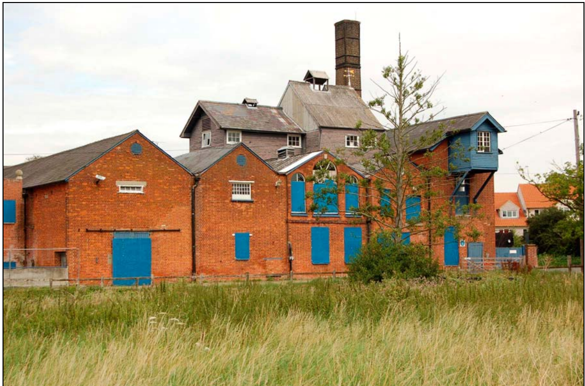
Plate 2 Brewhouse viewed to north
