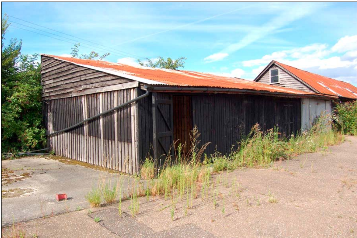
Plate 67 Modern barrel store viewed to north-east
