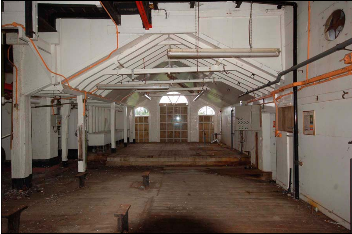
Plate 42 First floor of brewhouse and main gable viewed to south-east
