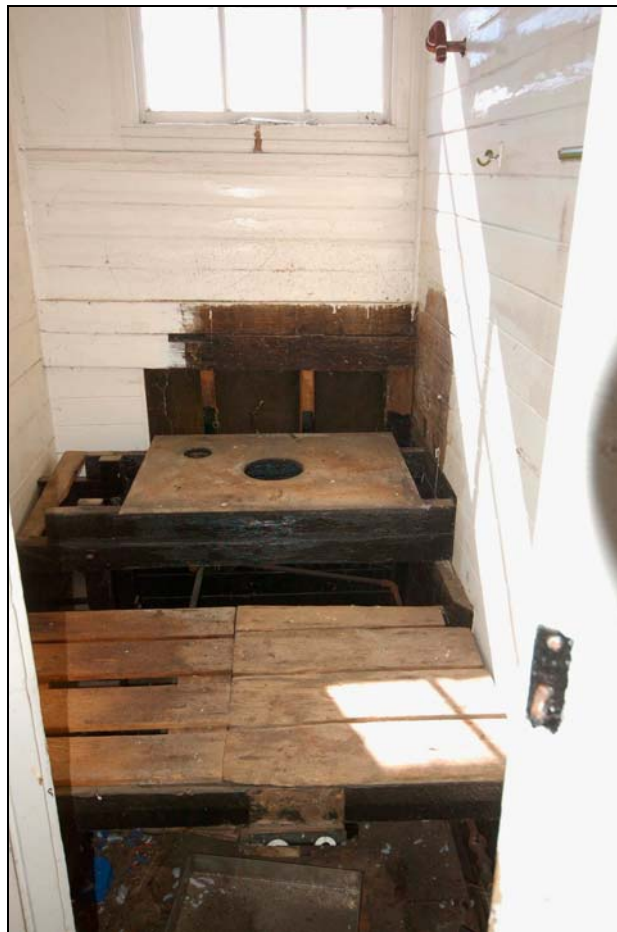
Plate 61 Interior of sugar dissolving room
