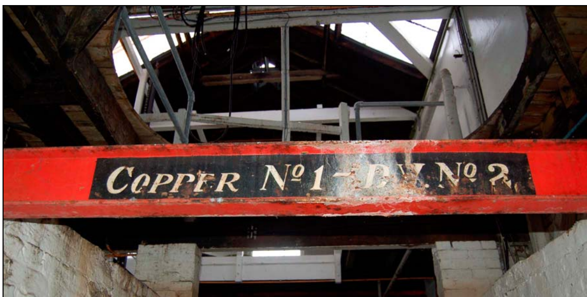
Plate 45 Vacant supporting joists for copper no. 1
