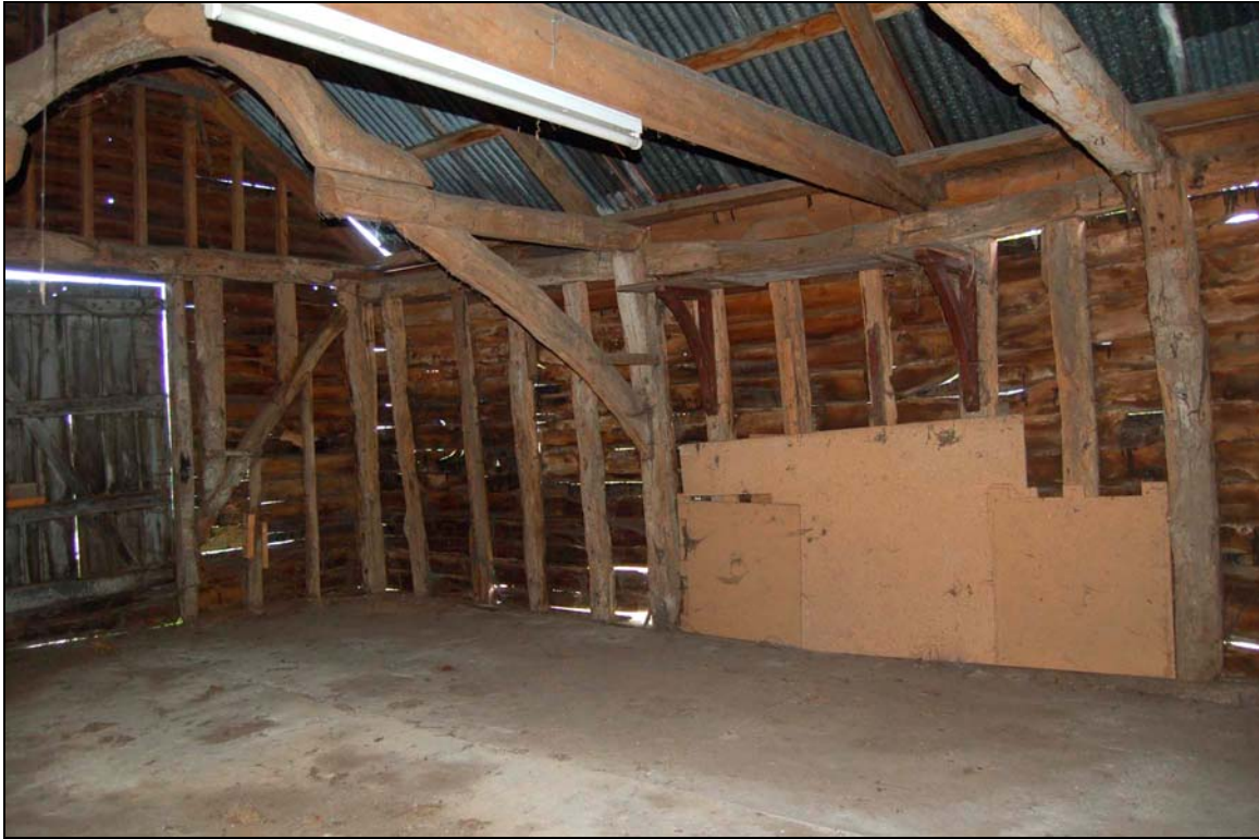
Plate 66 Typical c.16th century framing viewed to cartdoors (east)
