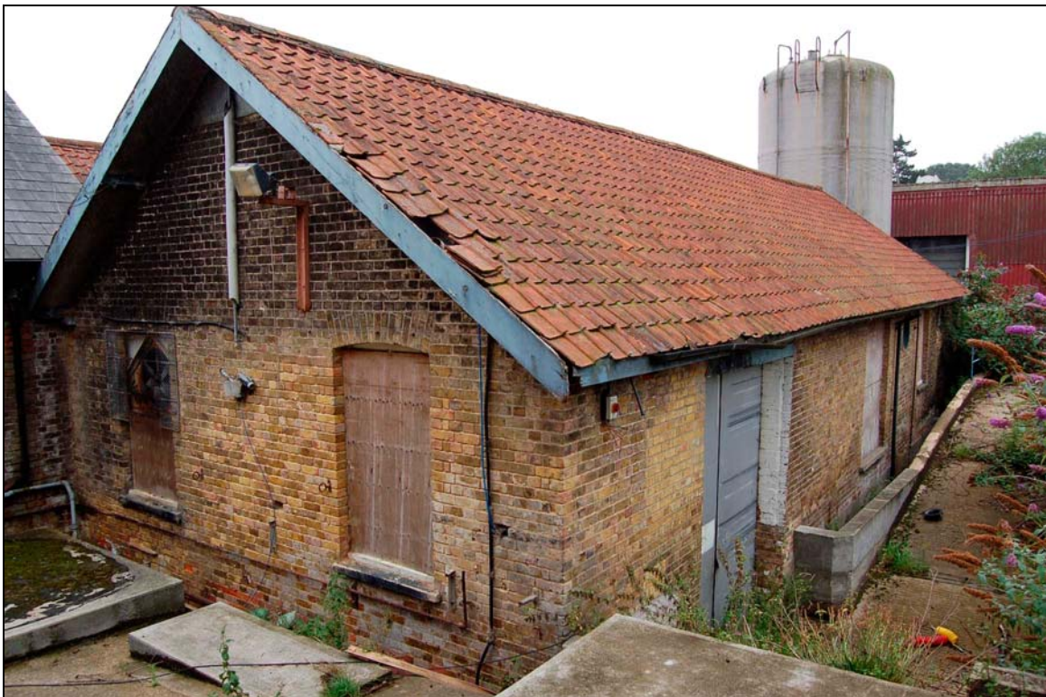
Plate 12 Bottling plant viewed to south-east
