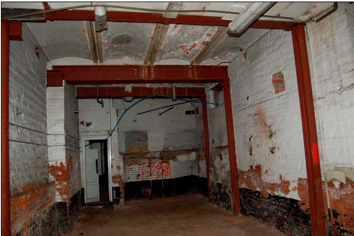
Plate 28 Jack arch ceiling in boiler room viewed to north-west
