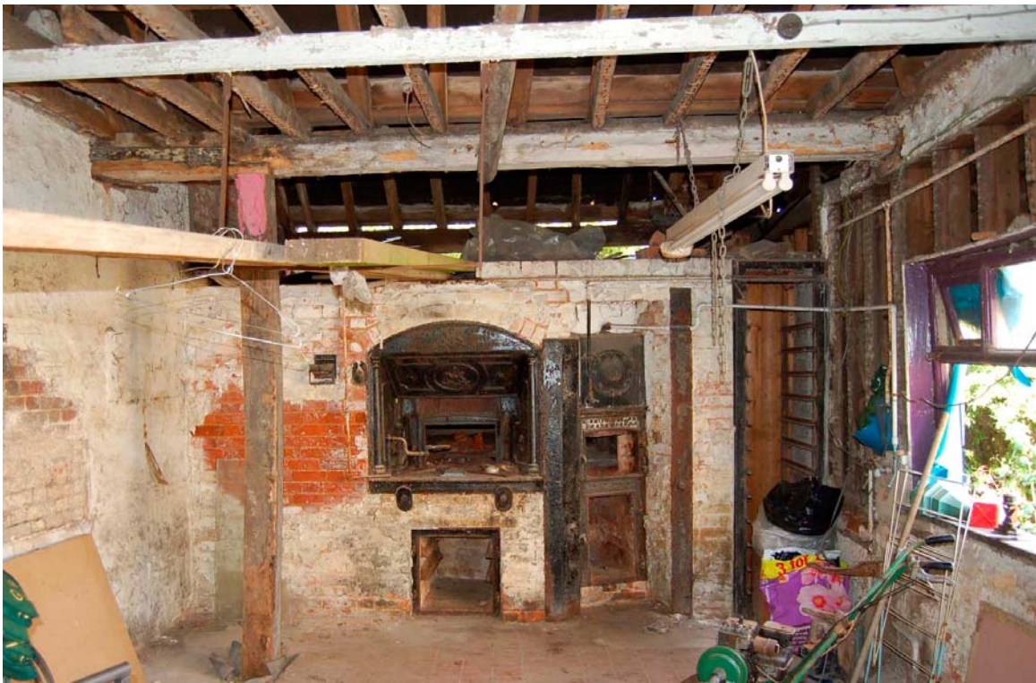
Plate 6 Interior viewed to west
