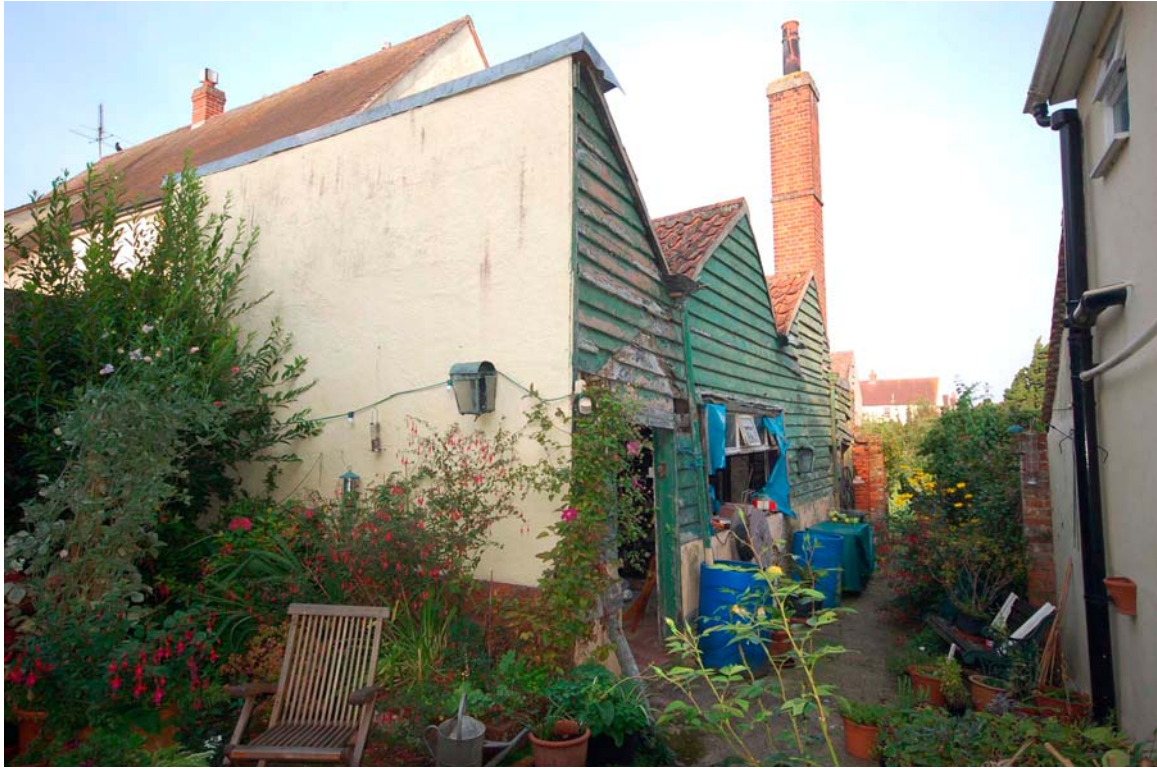
Plate 1 Bakehouse viewed from house (west)
