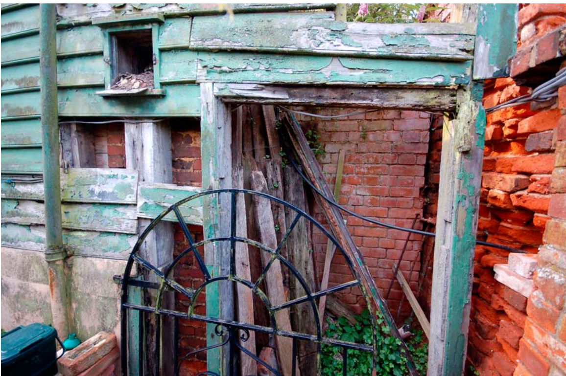
Plate 4 Chimney base and oven wall
