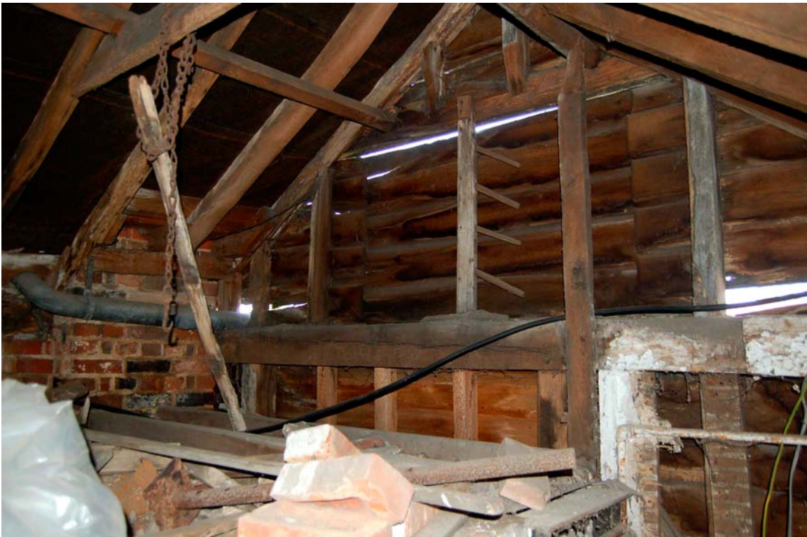
Plate 8 Oven roof and remains of wooden gable vent
