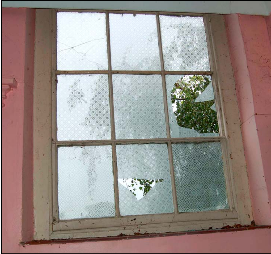
Plate 16 Detail of stencilled glass at north-east end
