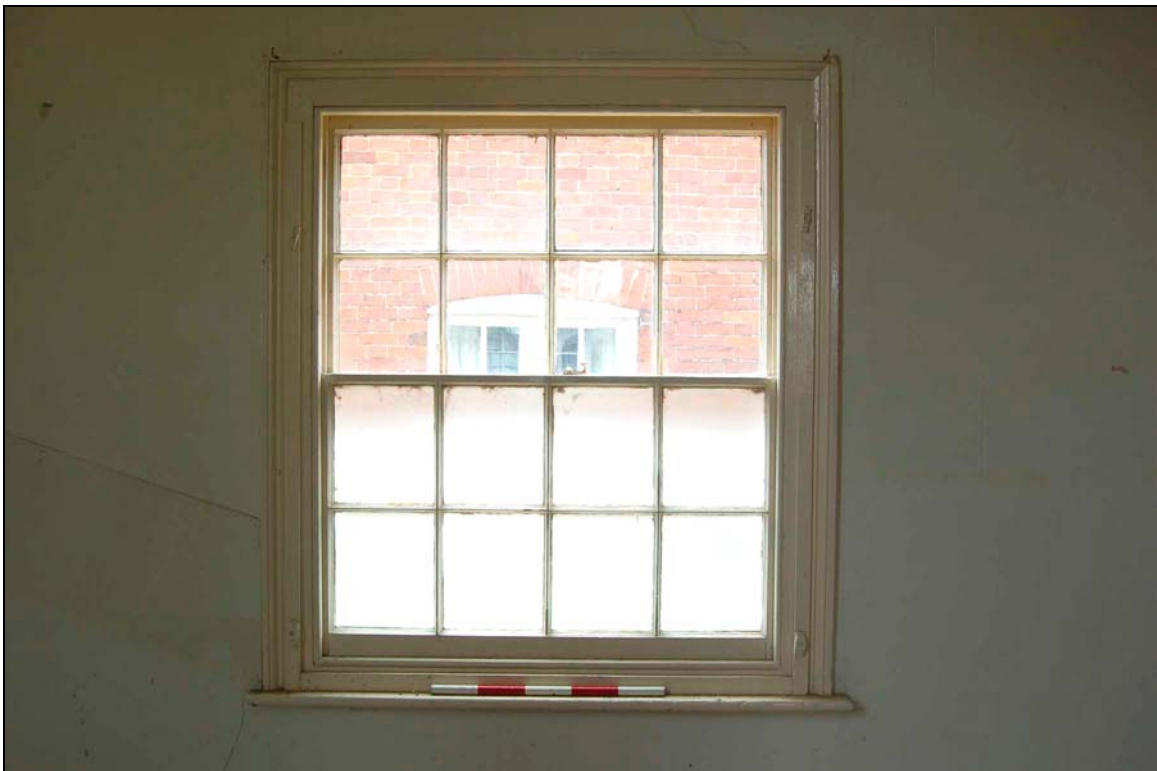
Plate 13 Window on south-west side of schoolroom (0.5m scale)
