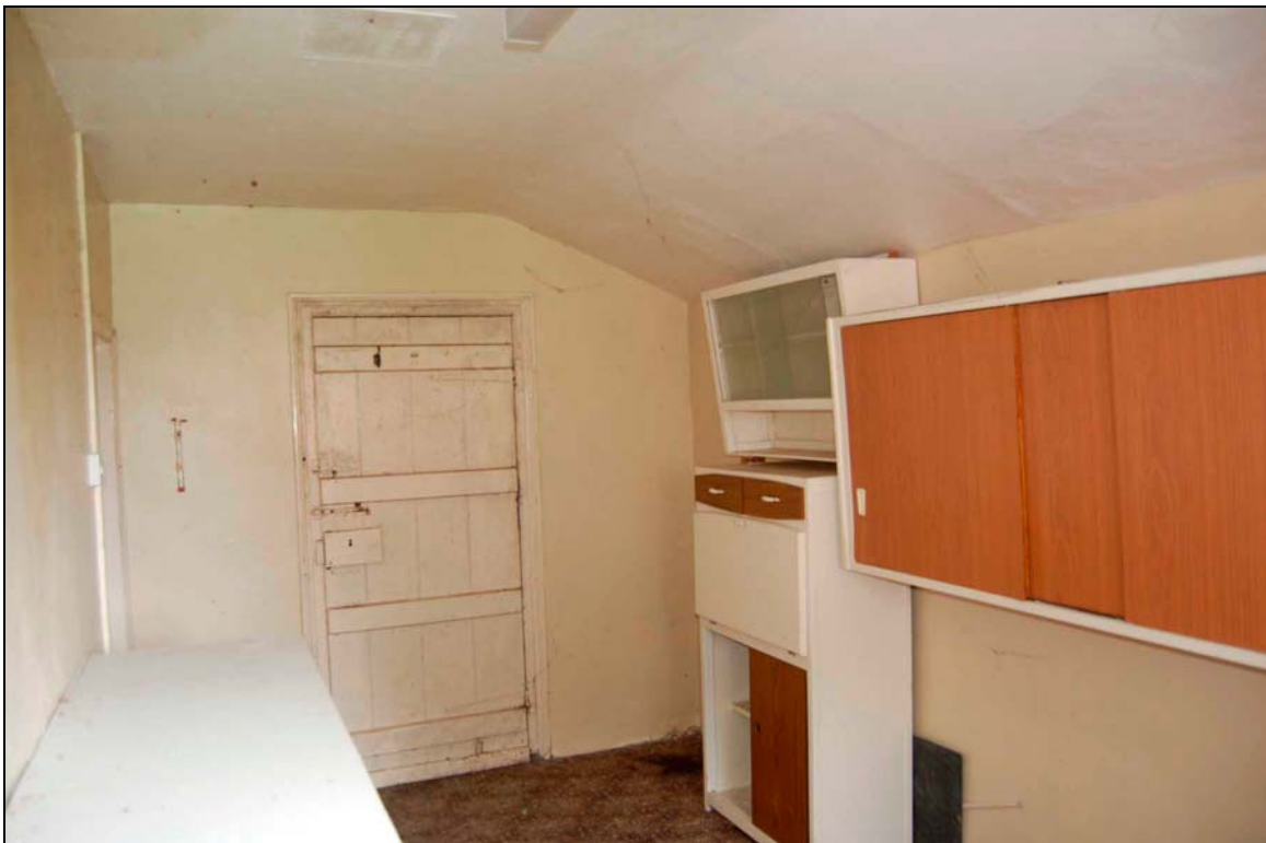
Plate 25 Kitchen interior, viewed to north-west
