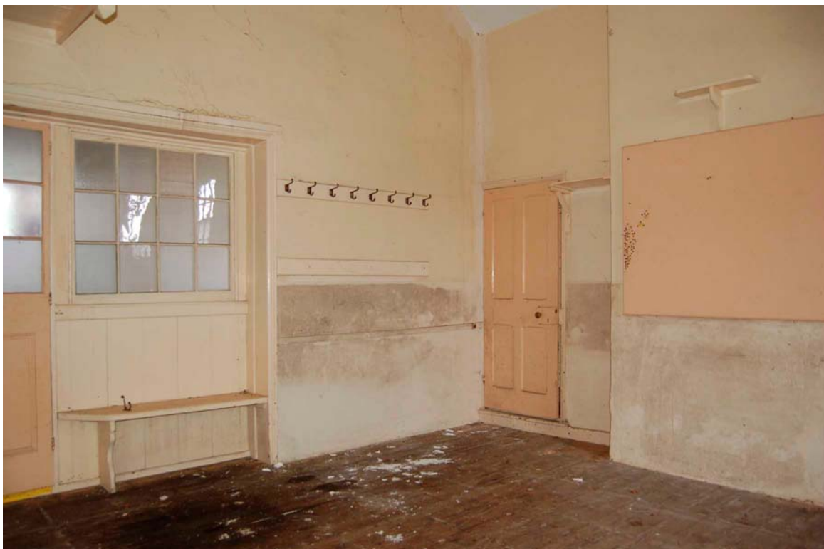
Plate 11 Historic fixtures around entrance to kitchen
