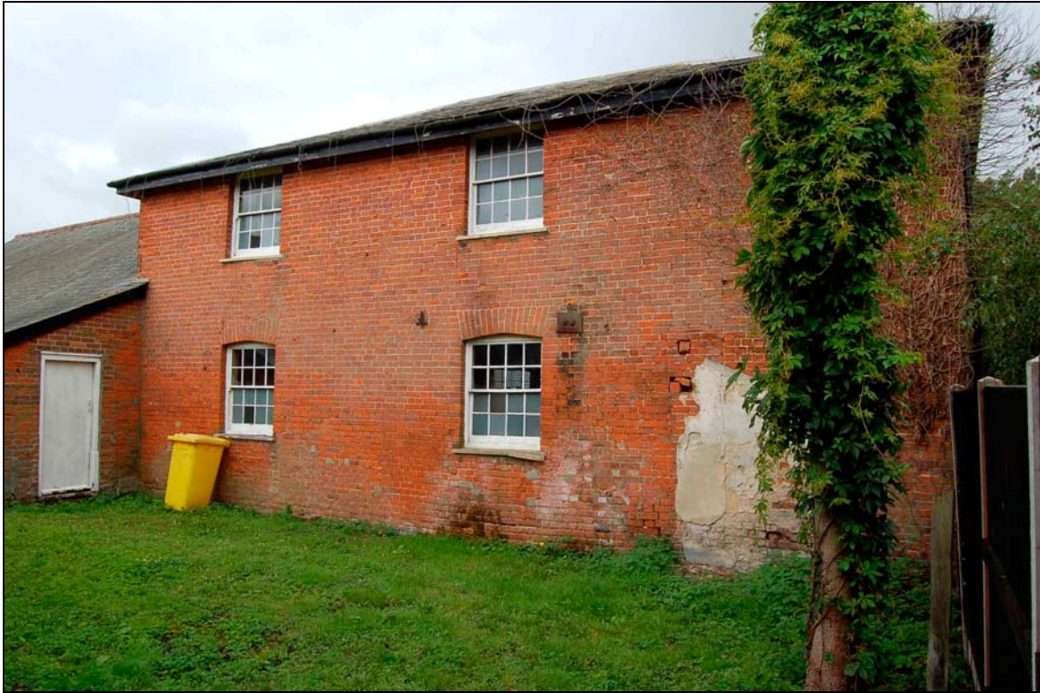
Plate 8 North-east elevation (chapel)
