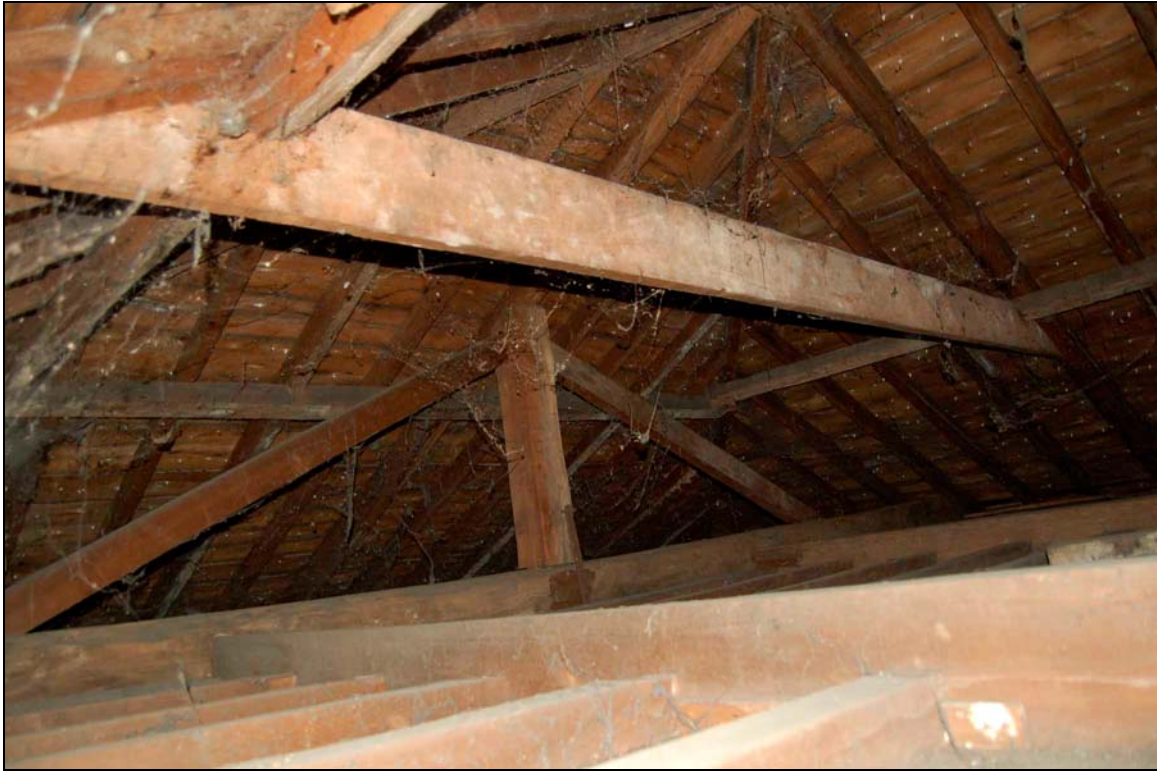
Plate 24 Chapel roof timbers
