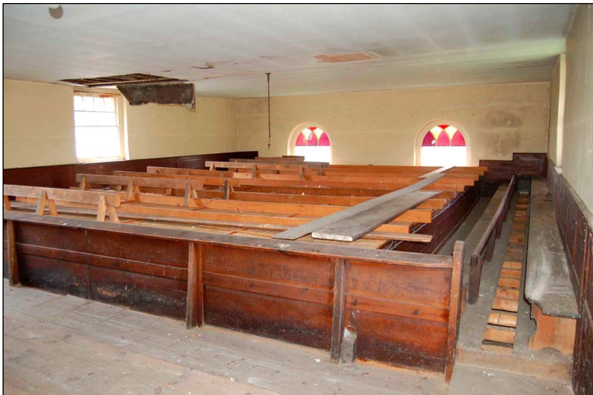
Plate 21 First floor viewed to north-west
