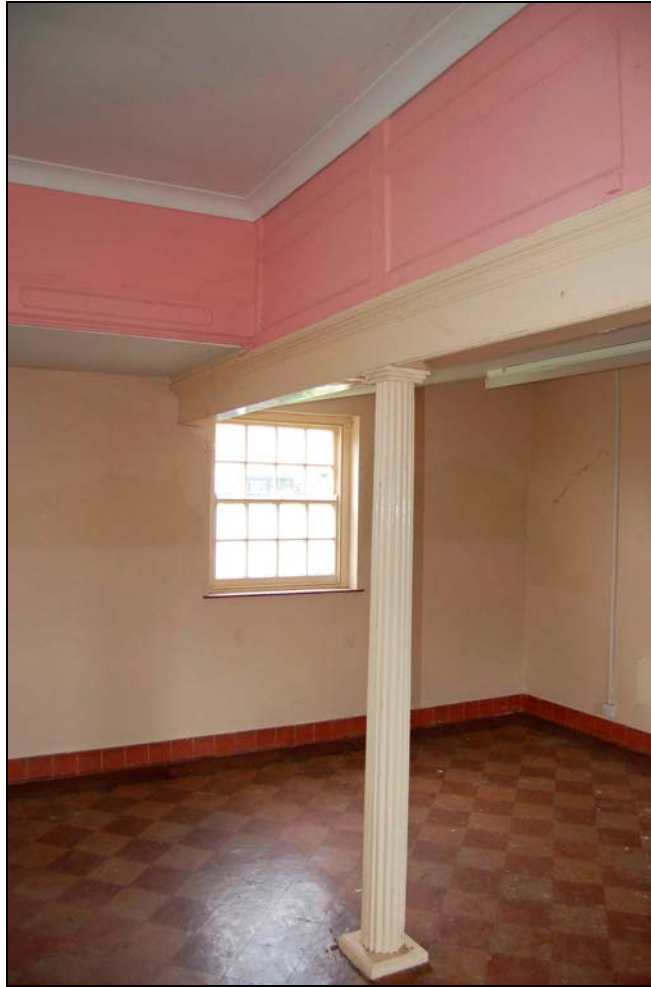
Plate 18 Detail of column and gallery panelling
