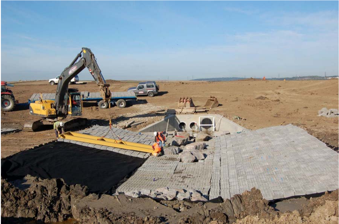
Plate 5 Scour mats being placed in the channel (from the temporary bund)
