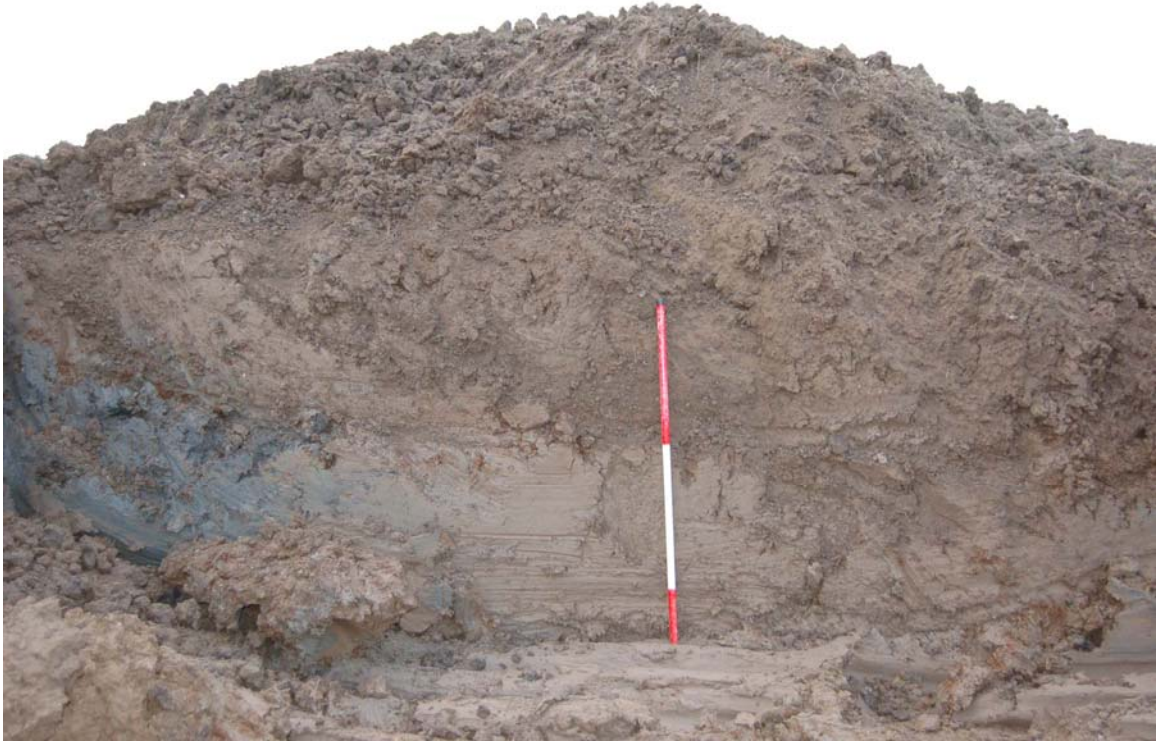
Plate 3 Section through seawall (1.5m scale)
