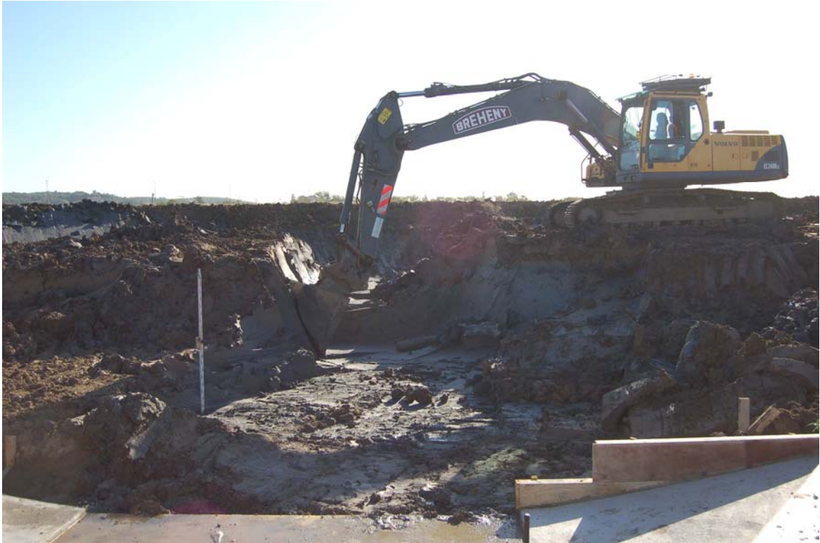
Plate 4 Excavation of the channel between the spillway and temporary bund
