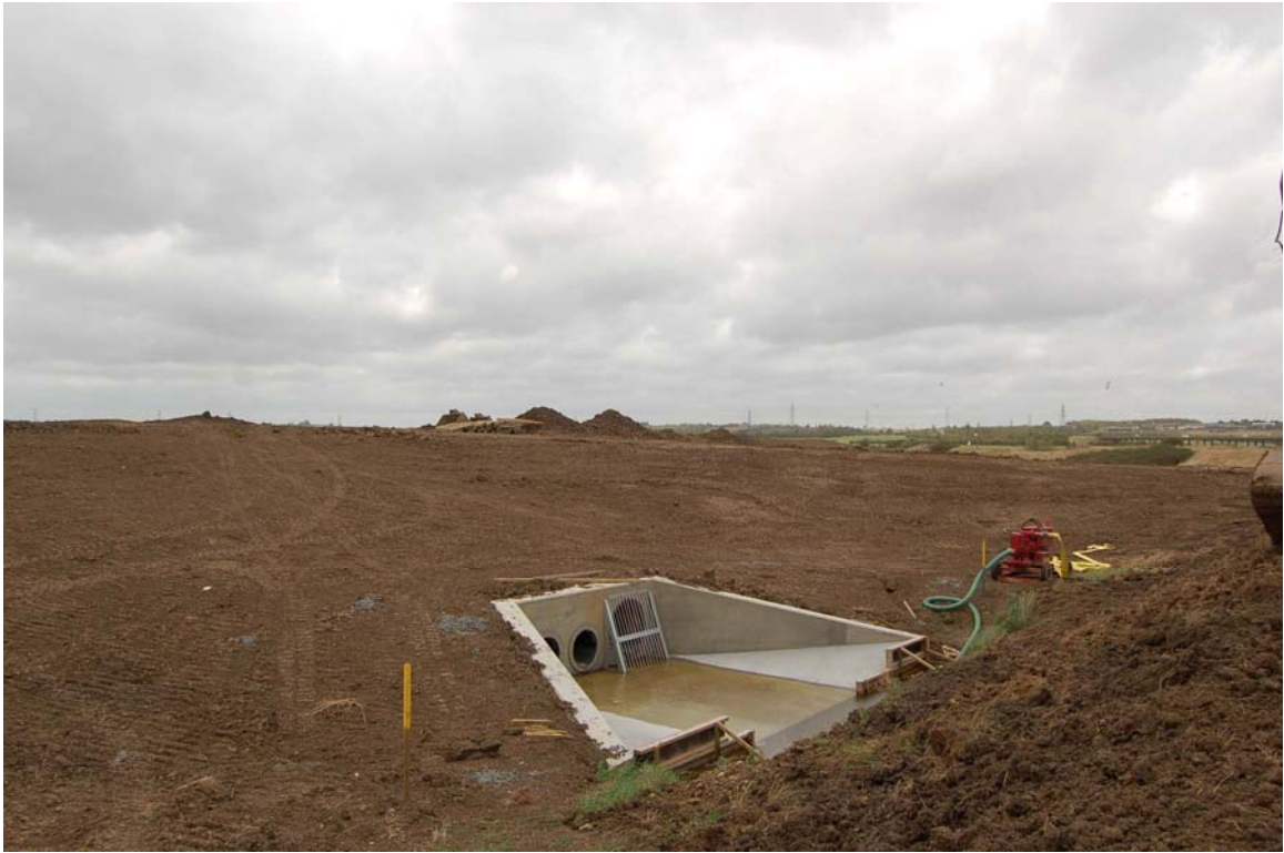
Plate 1 Saline lagoon embankment and concrete spillway (from seawall)
