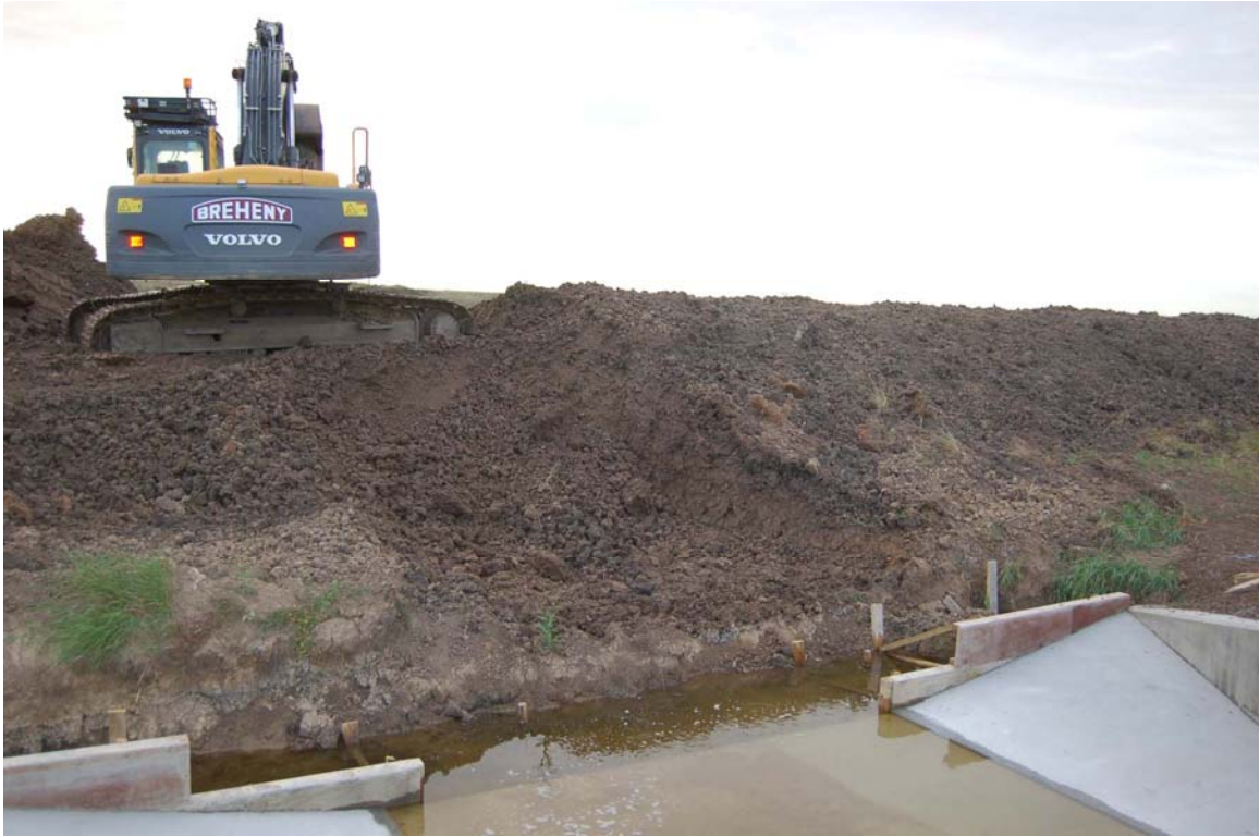
Plate 2 Seawall being removed
