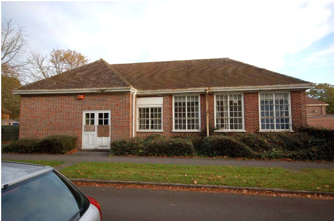
Plate 4 South elevation from road
