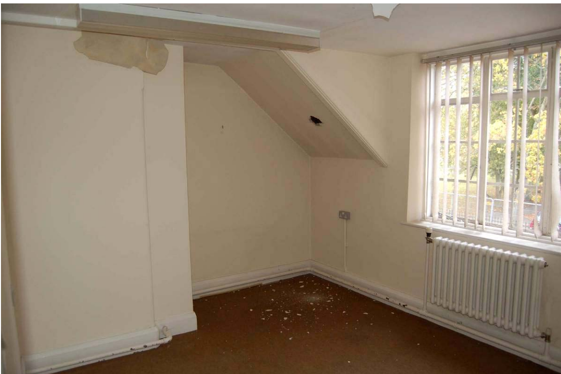
Plate 22 Staff room viewed to north-west
