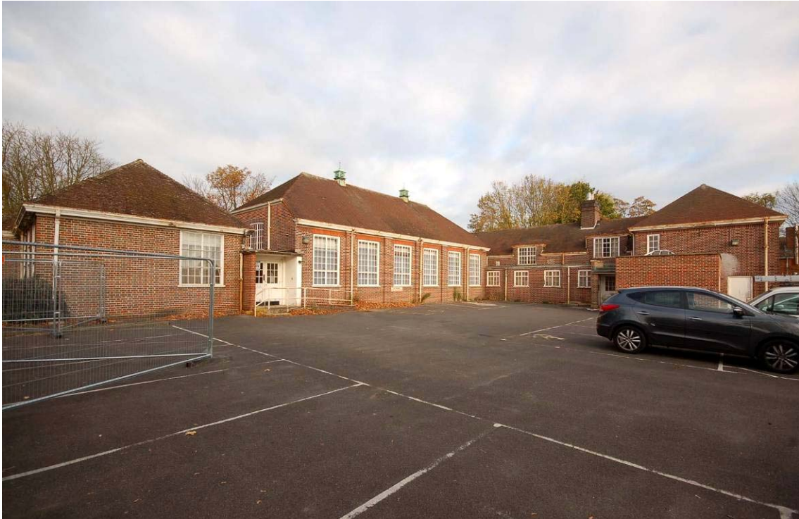
Plate 9 Rear of school viewed to north
