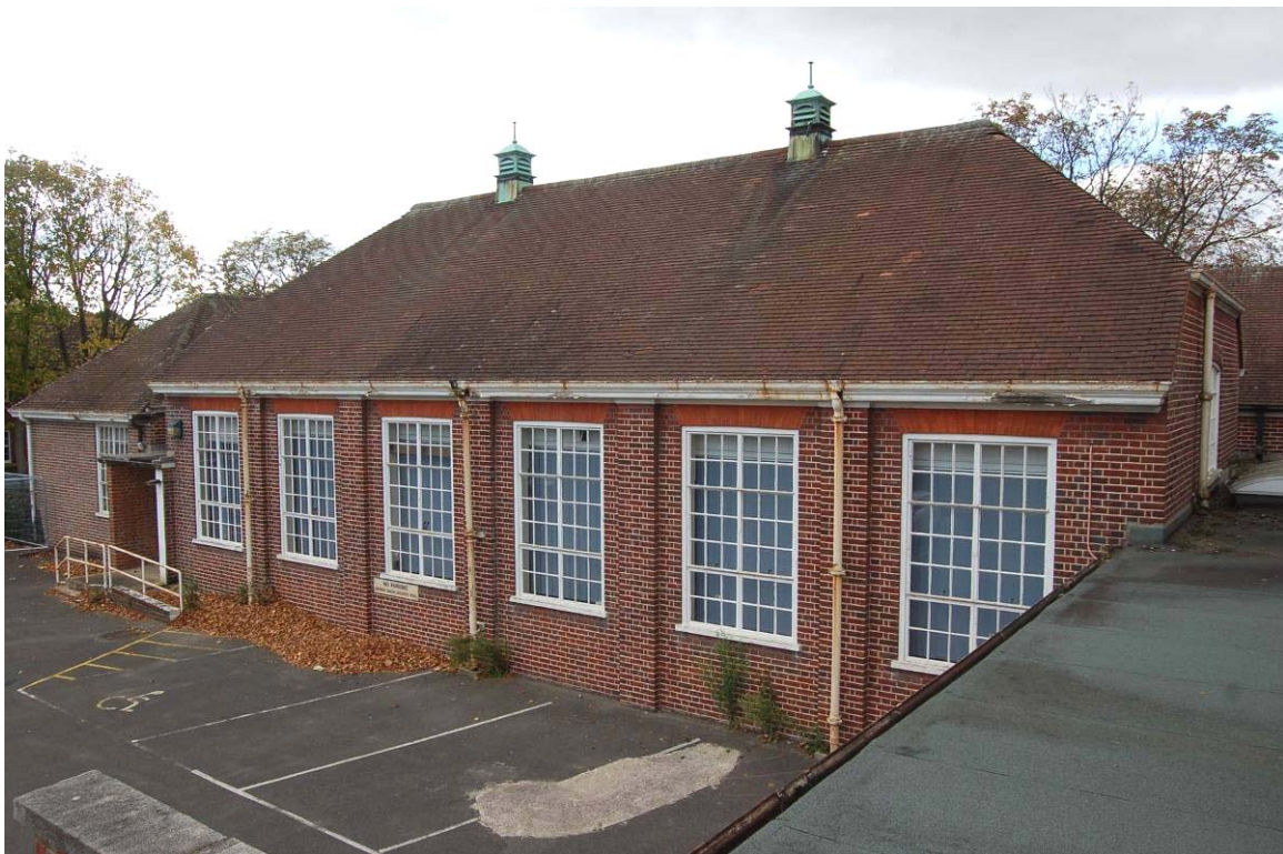
Plate 10 Assembly hall viewed to south-west from north corridor roof
