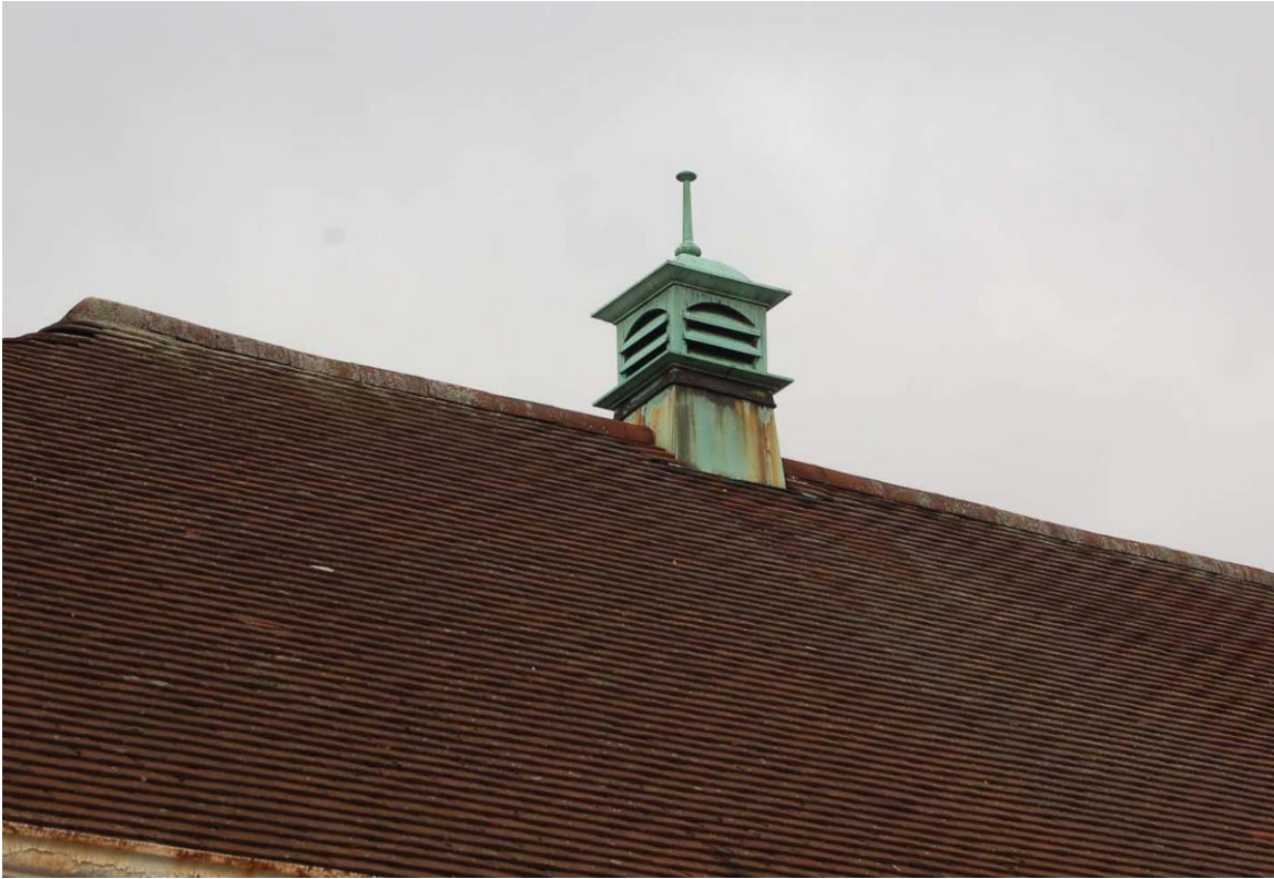
Plate 11 Ridge vent on assembly hall
