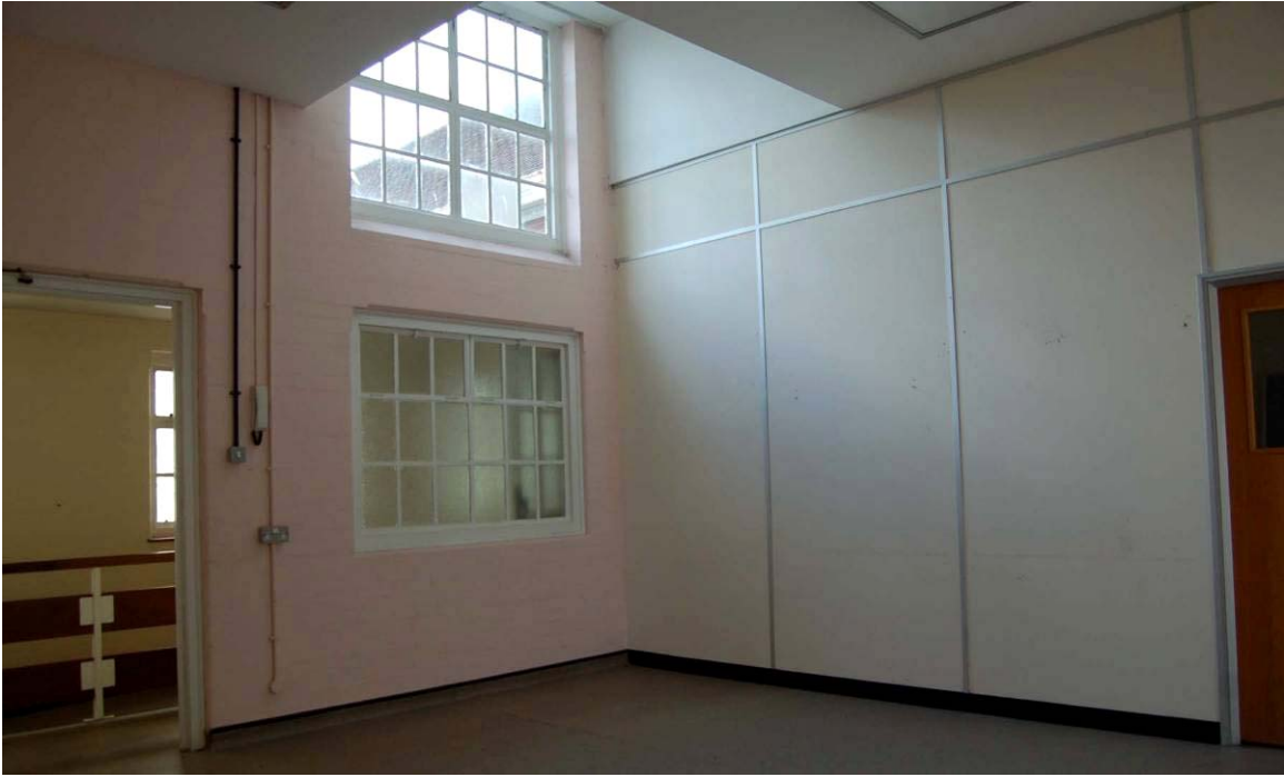
Plate 15 Classroom 1 viewed to south
