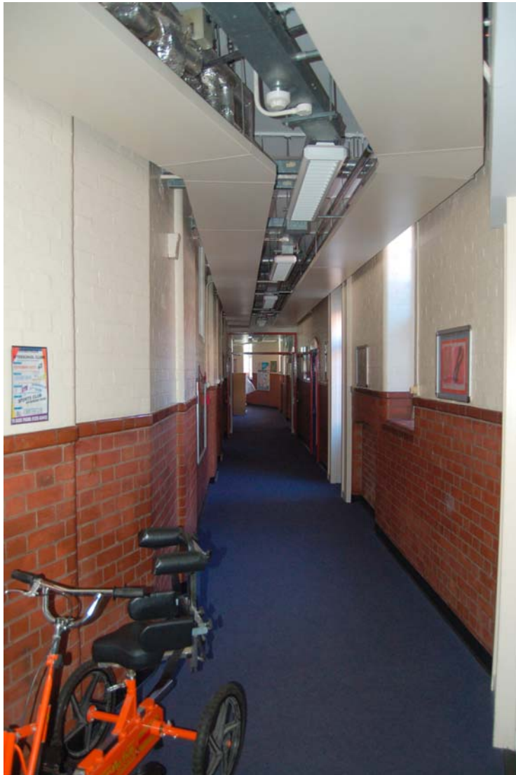
Plate 41 Corridor 30/43 viewed to south
