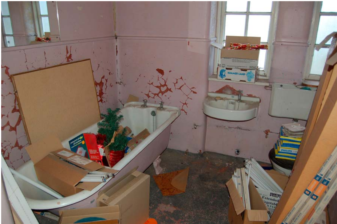
Plate 55 Bathroom 36 in staff living area
