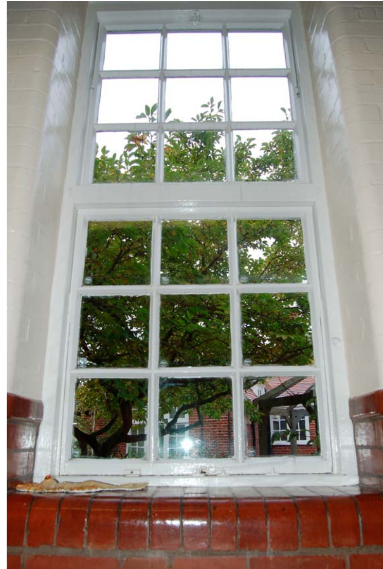
Plate 42 Typical corridor window
