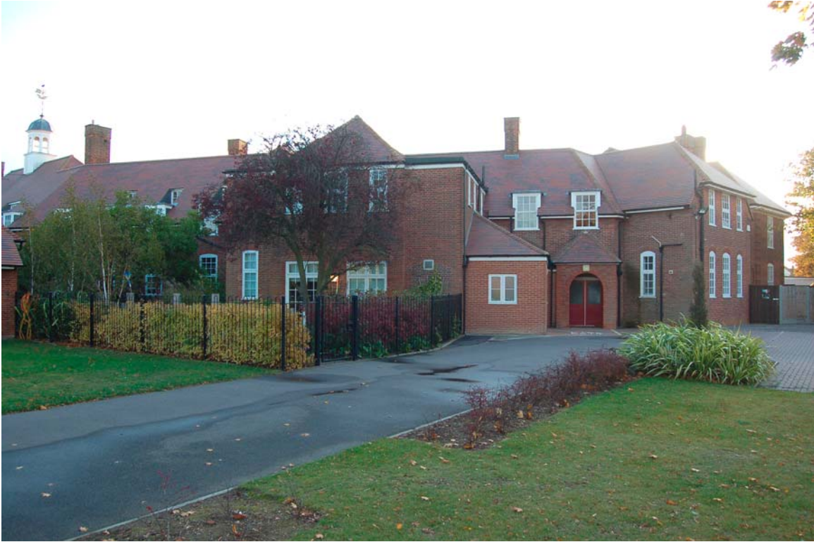
Plate 13 North-west (rear) elevation of school, with sanitary block (south wing)
