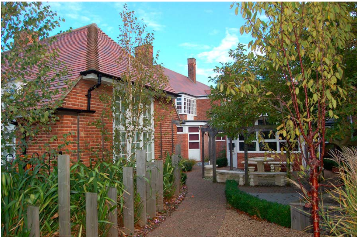
Plate 8 Isolation wing viewed to north
