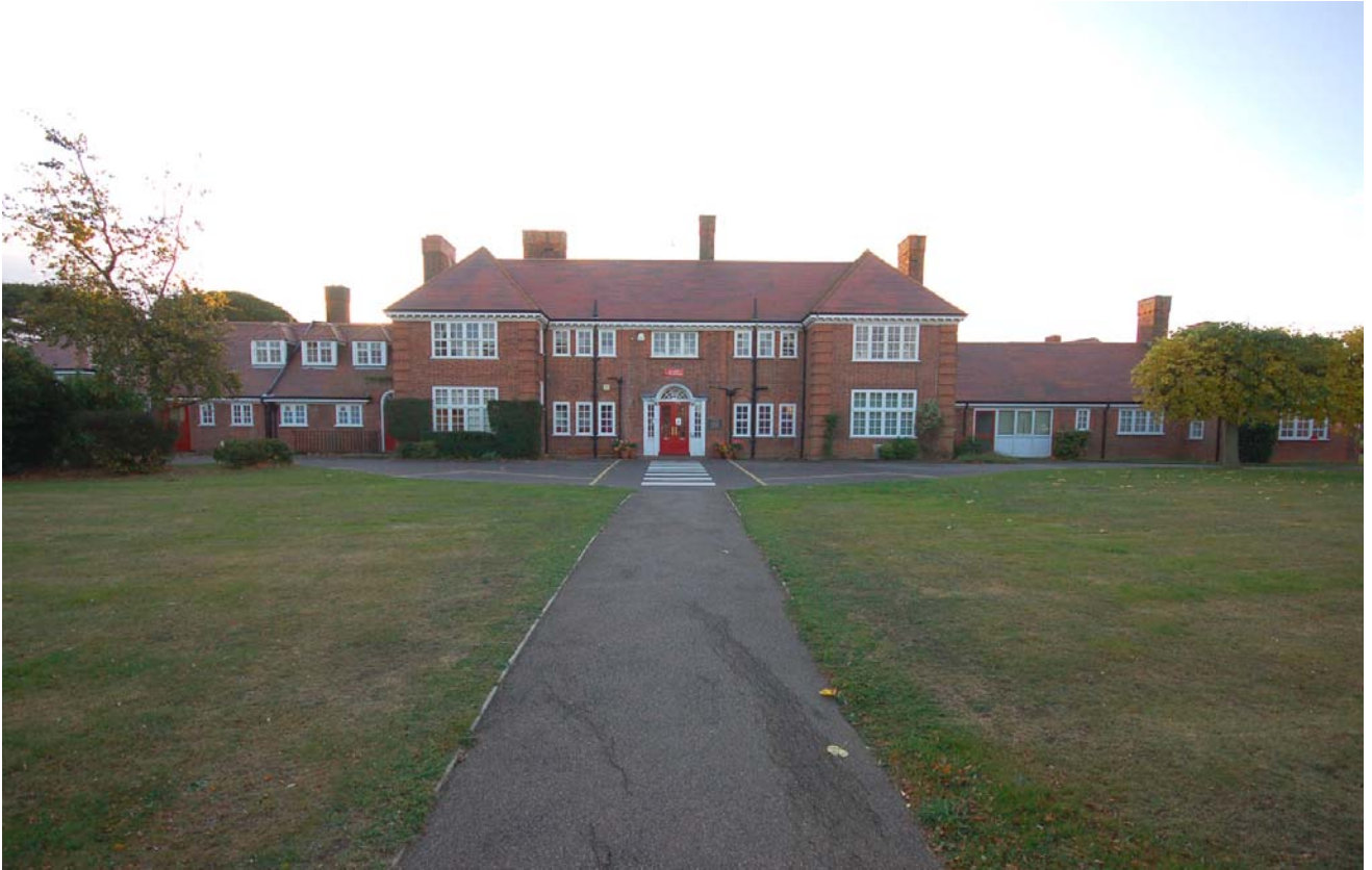
Plate 1 North-west elevation of admin building
