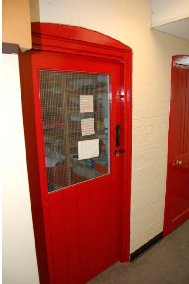
Plate 33 Storeroom door in corridor 22 (store 25)
