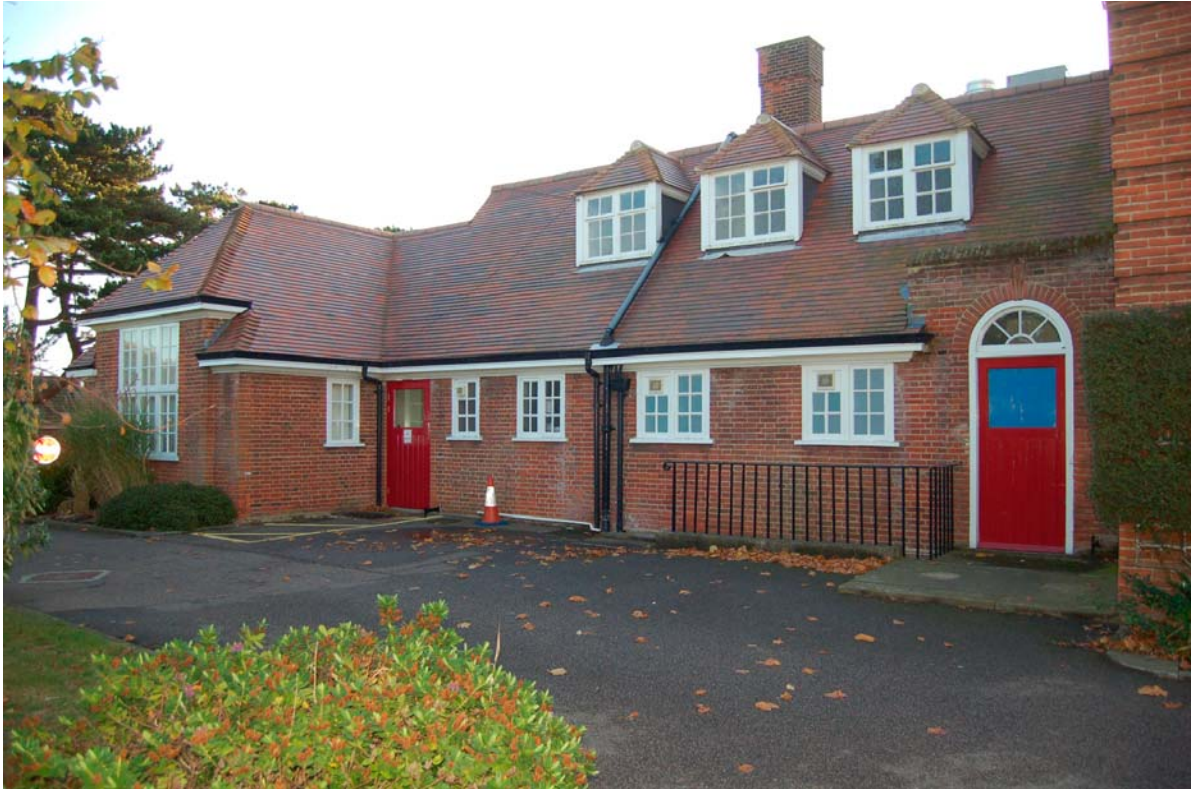
Plate 5 Kitchen wing viewed to east
