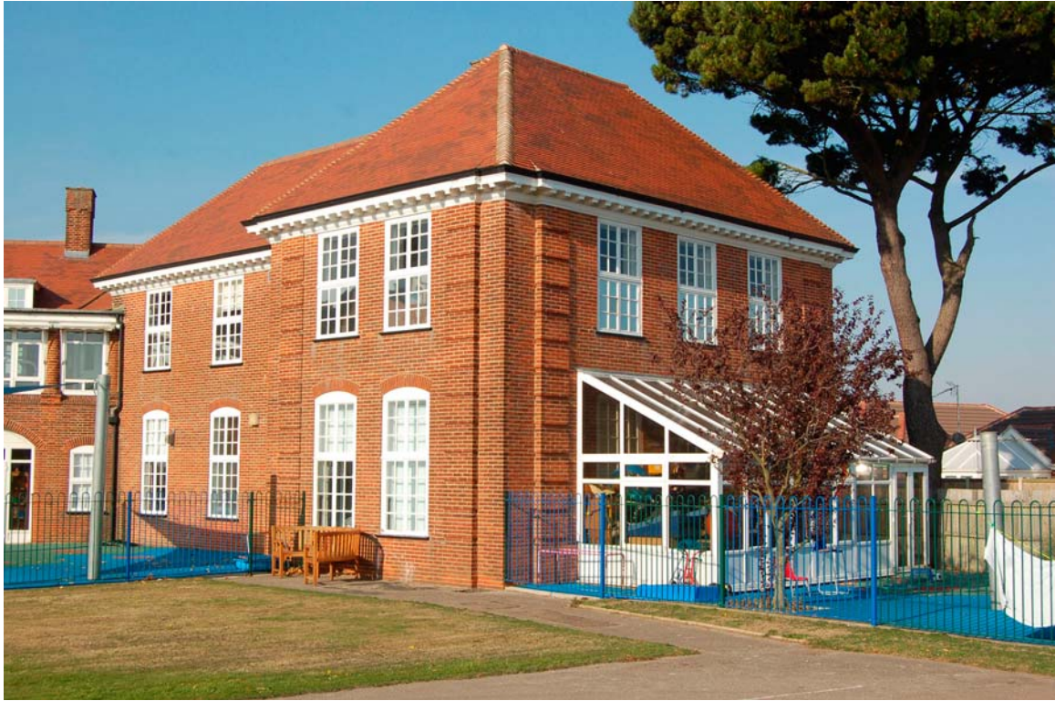
Plate 17 North wing extension viewed to north
