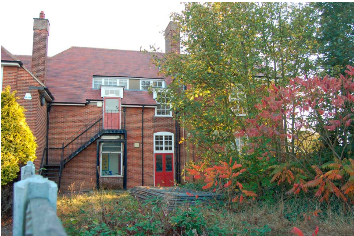
Plate 18 Rear of south wing extension viewed to north-east
