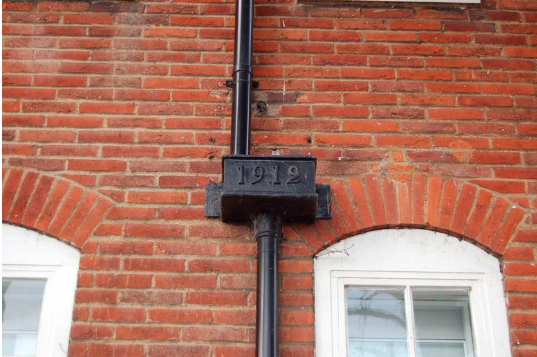
Plate 19 Reused 1912 rainwater hopper on rear of north wing
