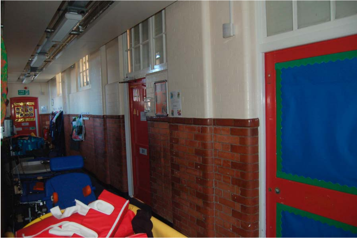
Plate 51 Corridor 37 in north wing extension
