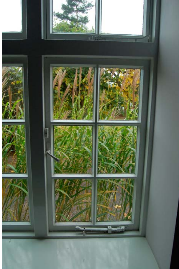
Plate 35 Window detail in room 27
