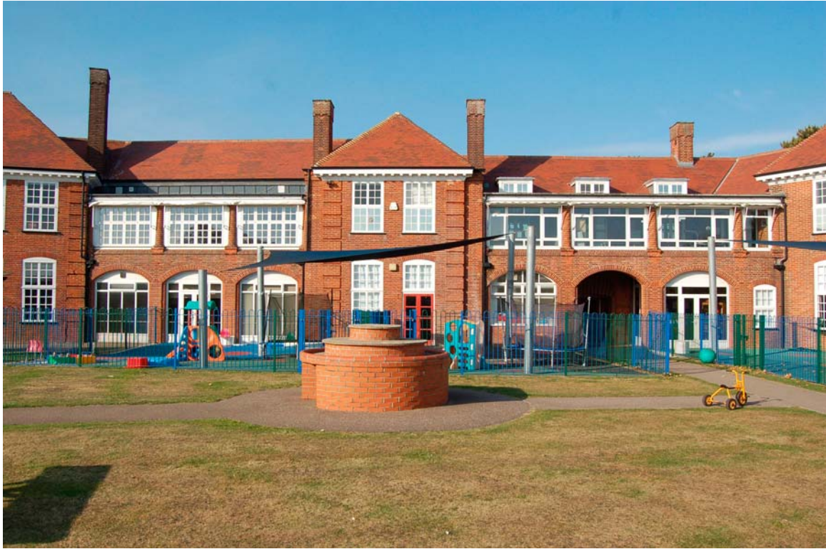
Plate 11 Dormitory block between verandah ranges (north wing)
