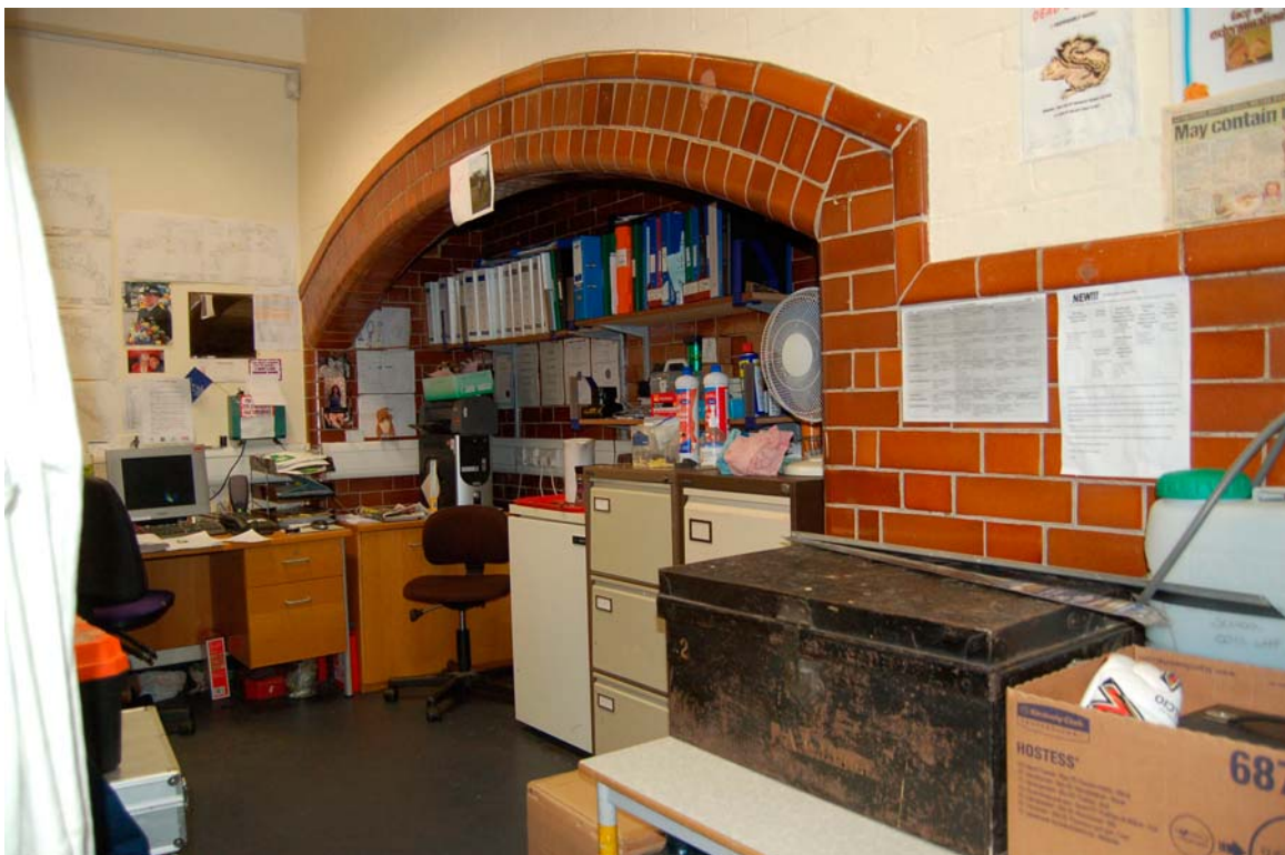
Plate 32 Brick hearth for former cooking range
