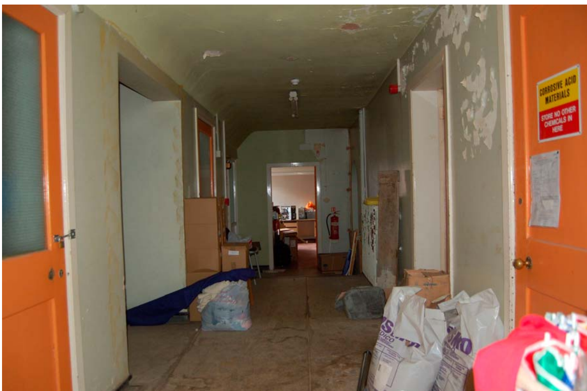
Plate 56 Corridor 35 viewed to north-west (matron's flat)
