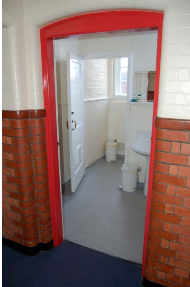
Plate 53 Original toilet in south wing extension (wc 49)
