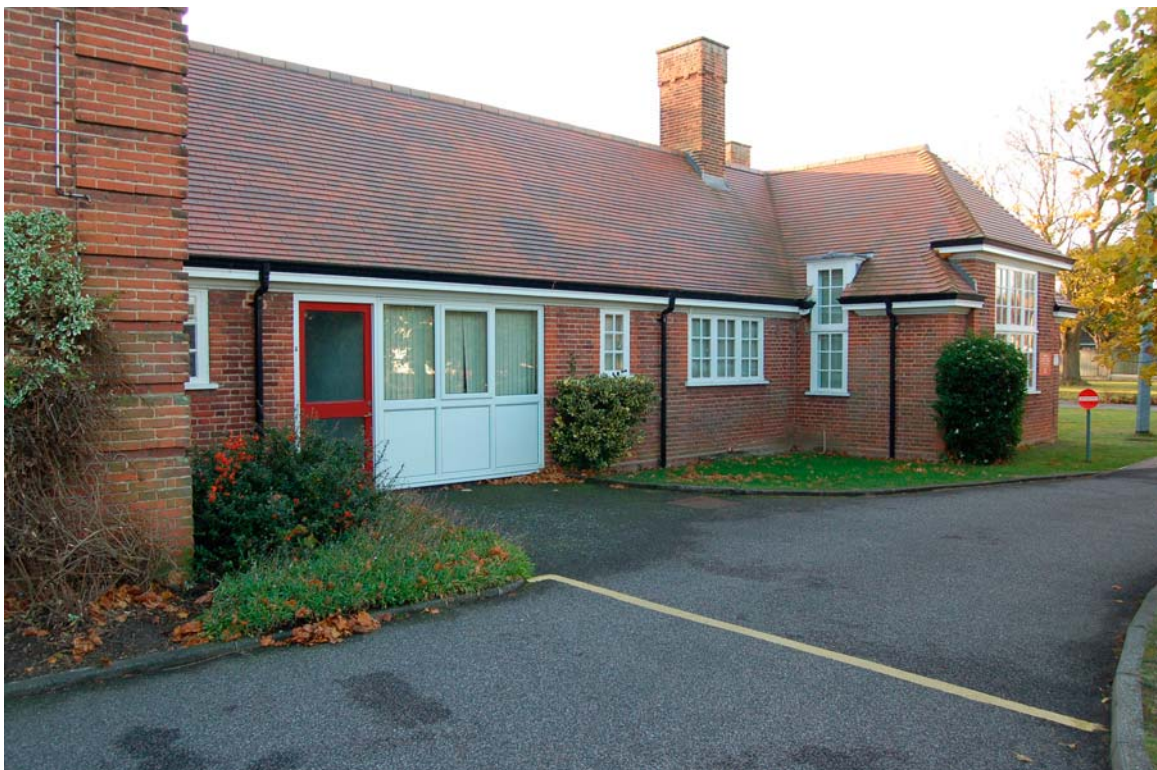
Plate 4 Isolation wing viewed to south
