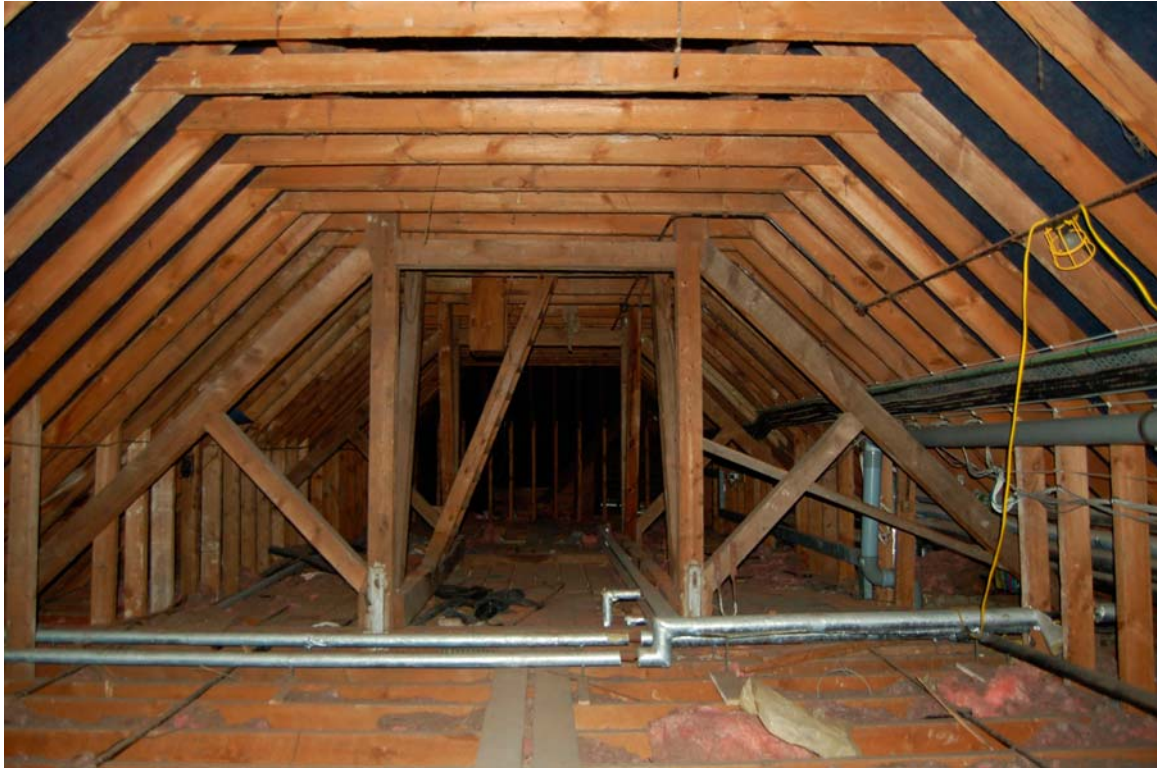
Plate 73 Roof and bell tower frame over central block
