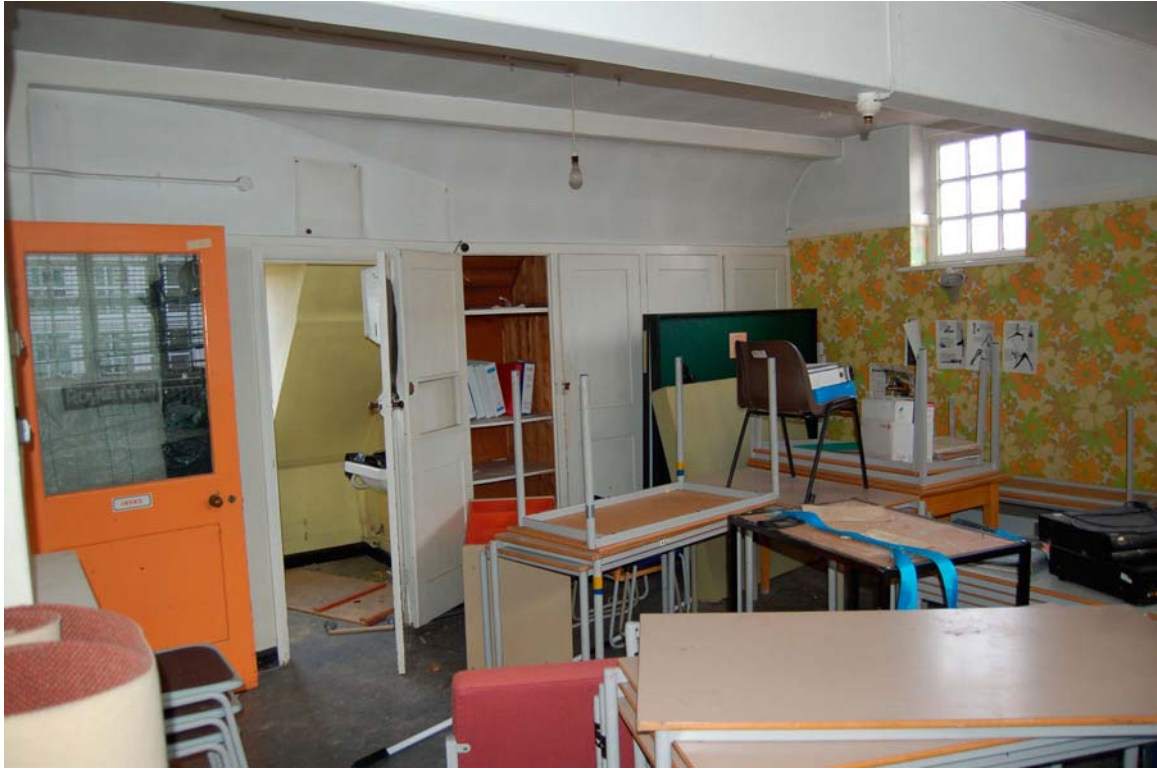
Plate 61 Bedroom 39 viewed to north-west (front)
