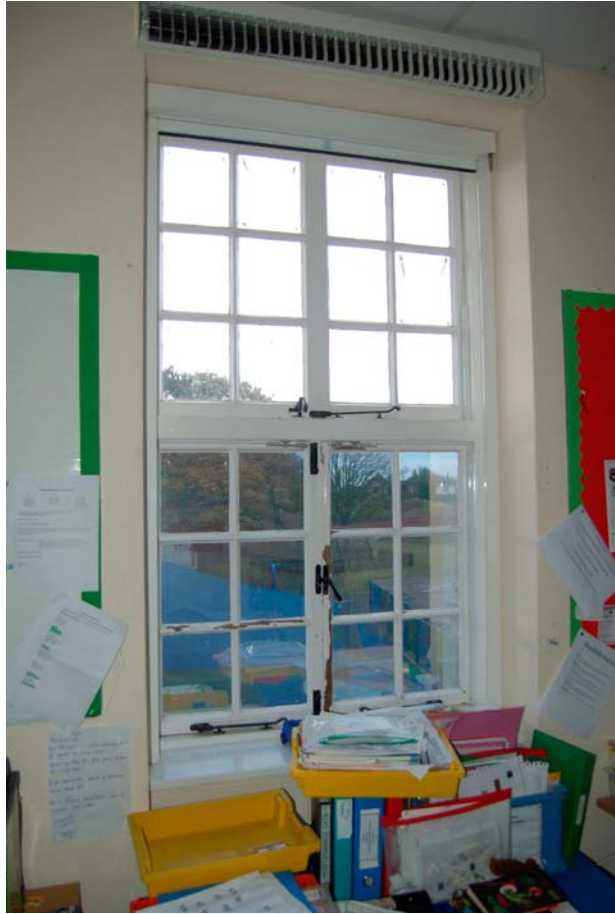
Plate 75 Typical casement/tilting windows (room 34)
