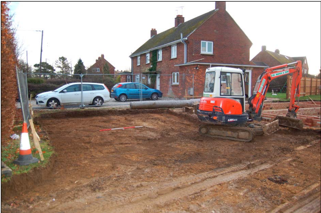
Plate 2 New driveway post-excitation, viewed to south-east
