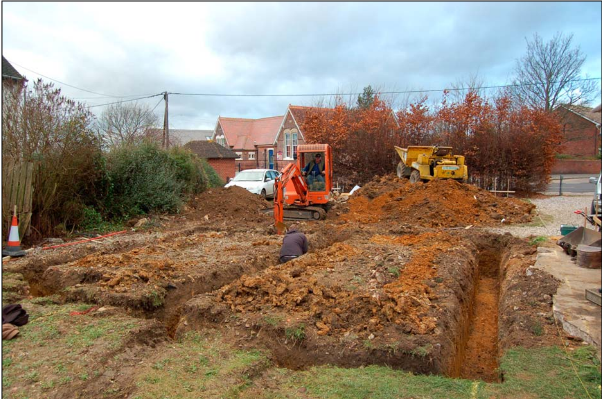
Plate 1 Excavation of house footings, viewed to north
