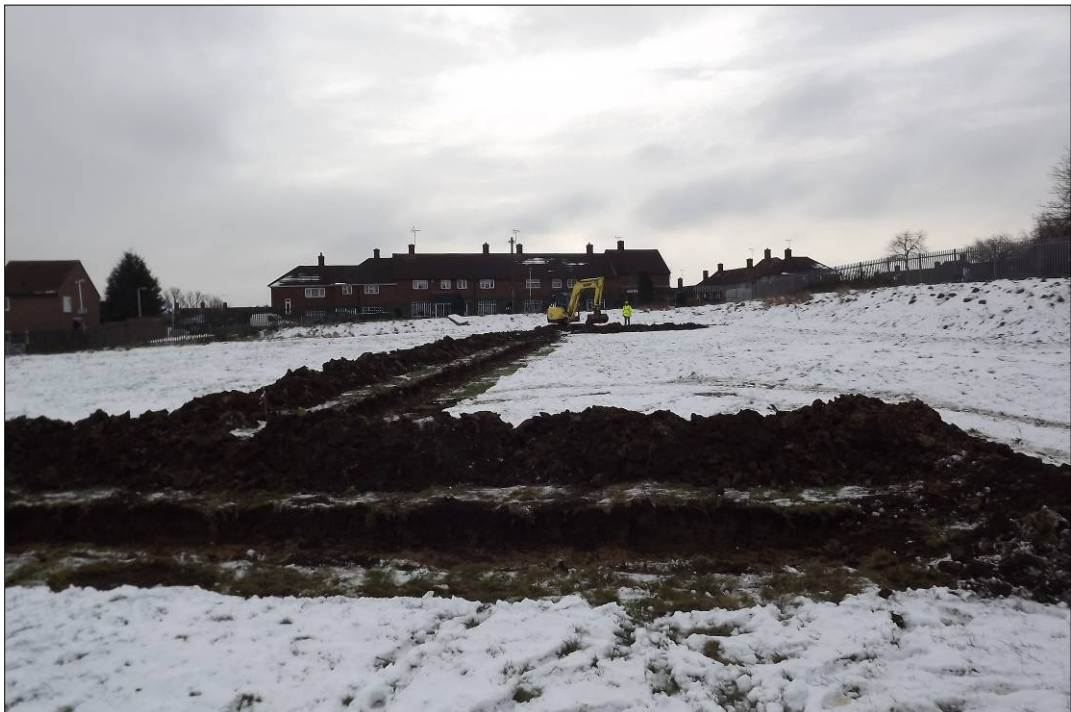
Plate 6. General site view
