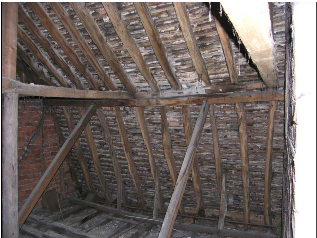
Plate 6: Mansard roof structure
