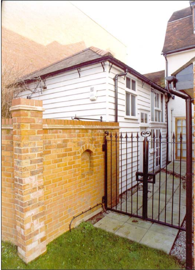
Plate 7: Slaughterhouse viewed from south-west
