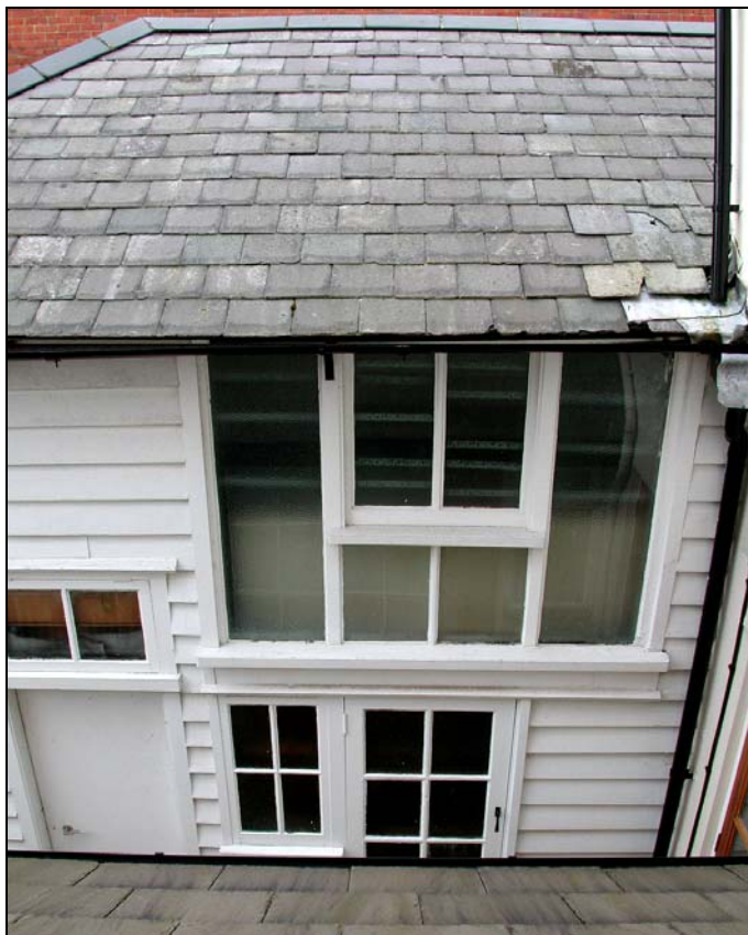
Plate 8: Slaughterhouse south elevation
