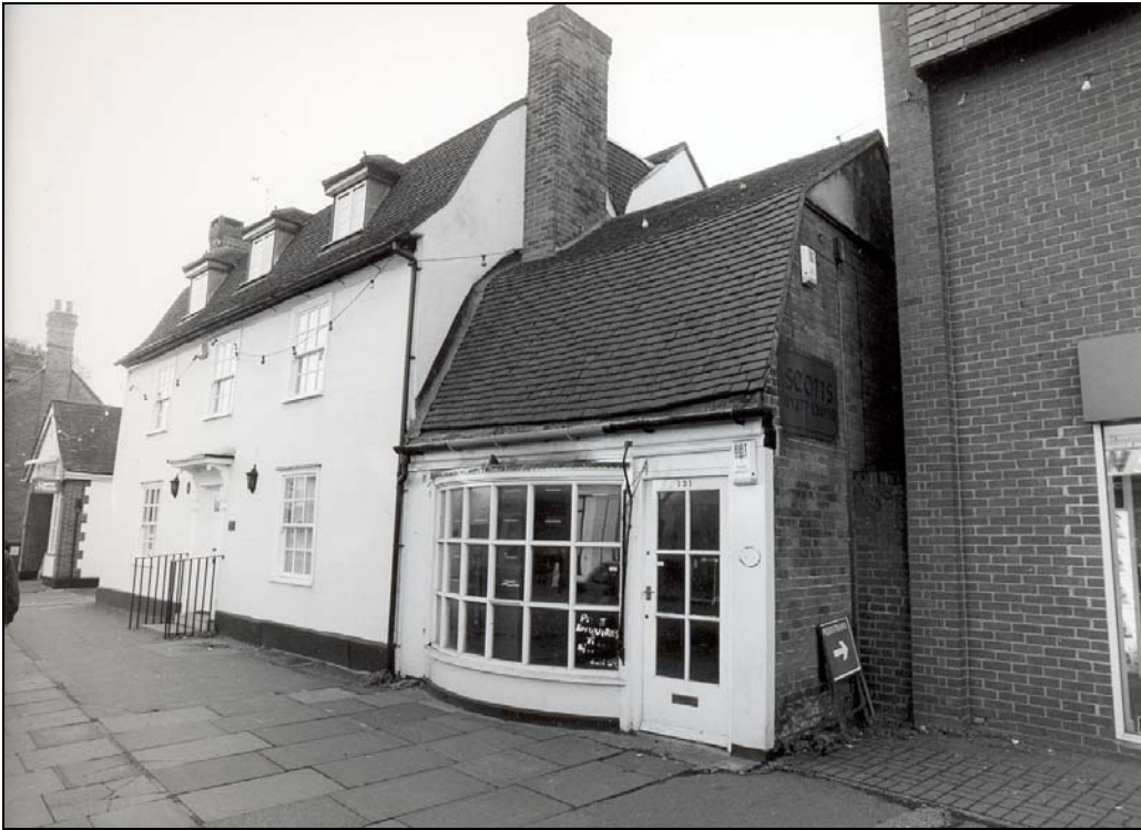
Plate 1: 133 and 131 High Street viewed from north-east
