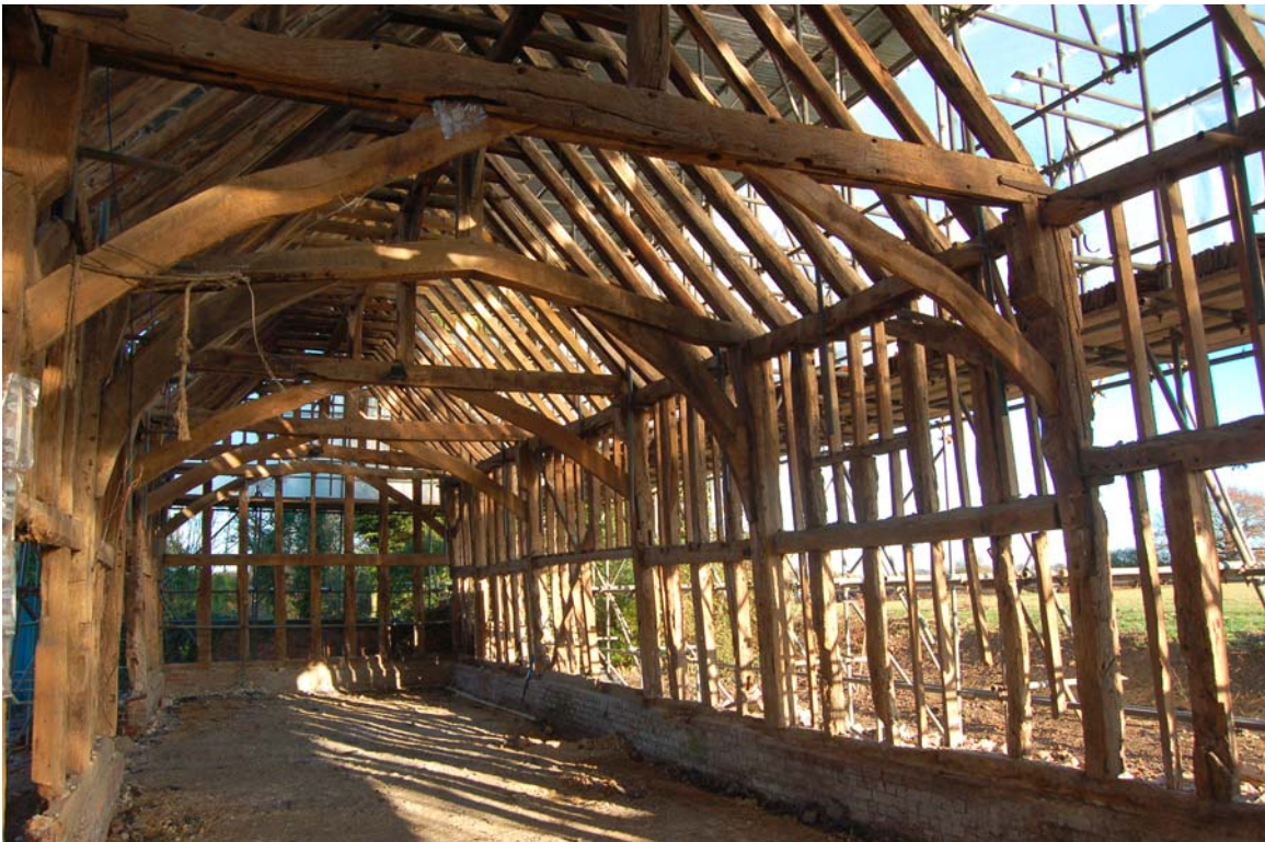
Plate 8 Timber-frame viewed internally to north-east during conversion works
