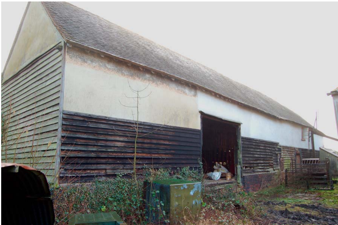
Plate 2 Barn viewed to south-east
