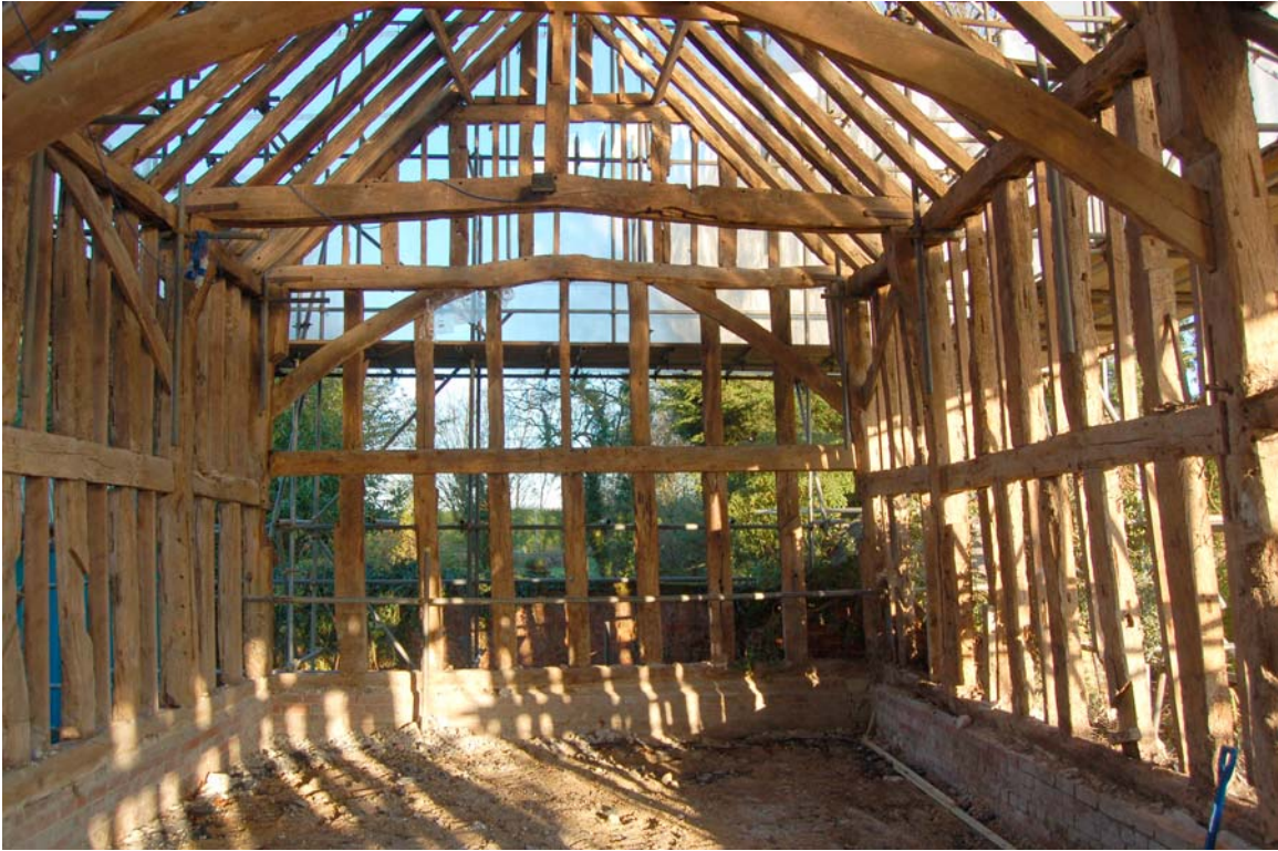
Plate 9 North end of barn viewed internally during conversion works
