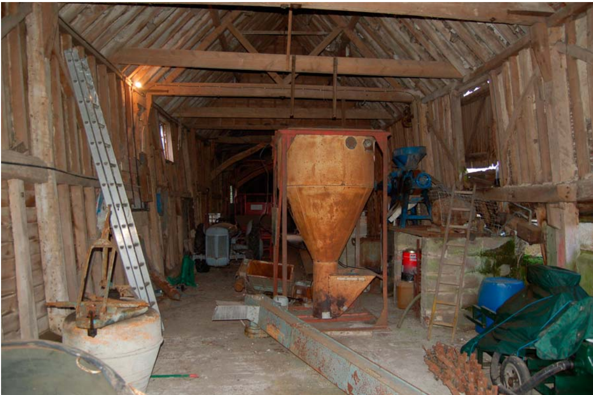
Plate 16 Barn 3 viewed to north
