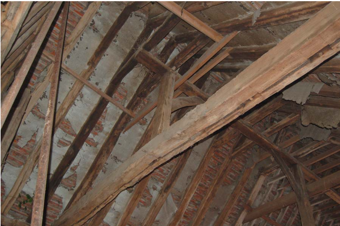
Plate 14 End of crown post roof (T2)
