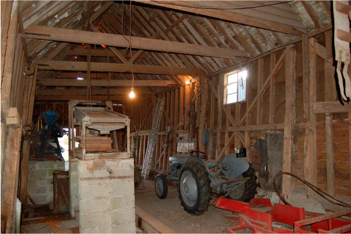
Plate 15 Barn 3 and end of extension 2 viewed to south west
