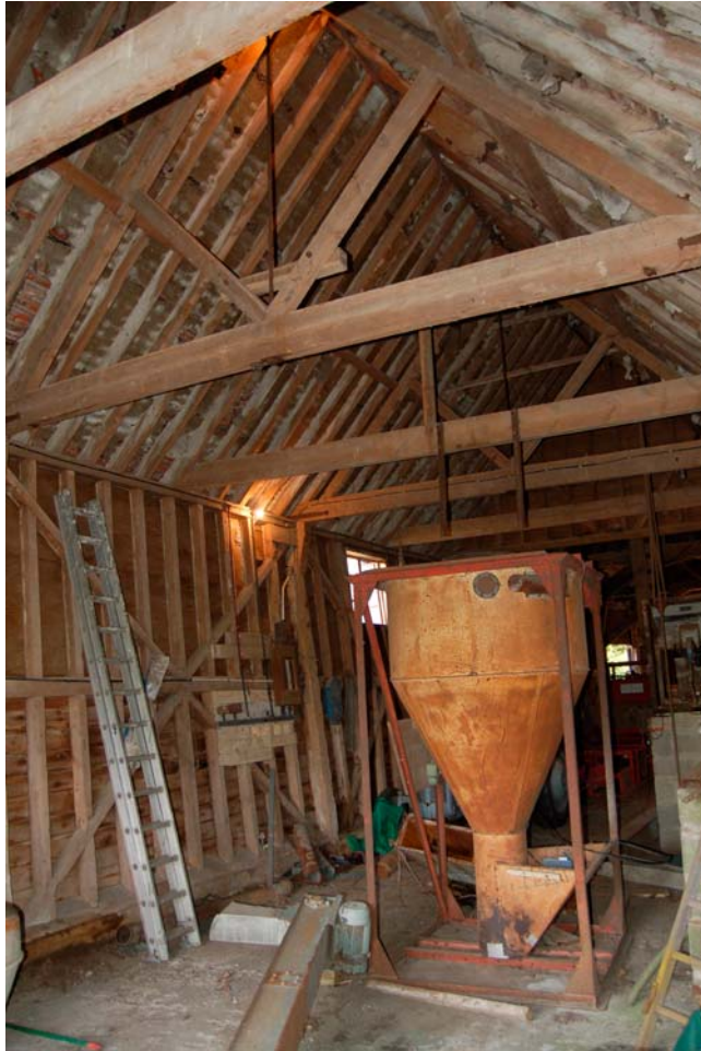
Plate 17 Barn 3 viewed to north-west showing roof structure
