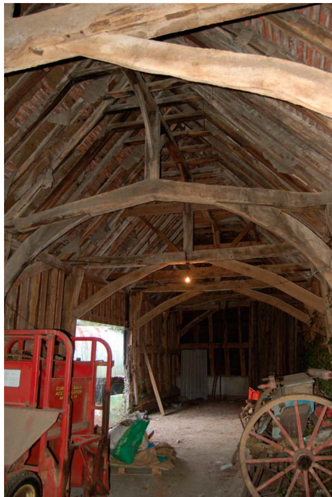
Plate 6 Medieval truss T5 and crown-post roof viewed to north
