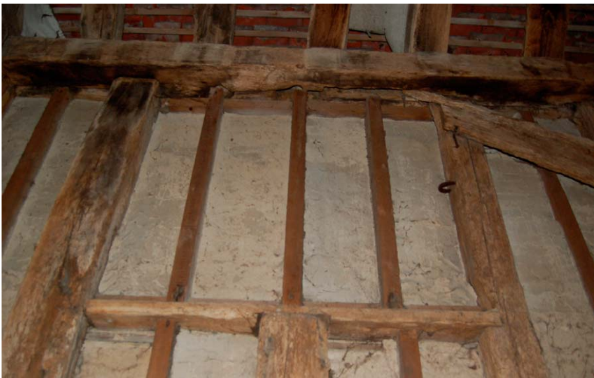
Plate 10 Former mullioned window within later blocked window in bay 5 east
