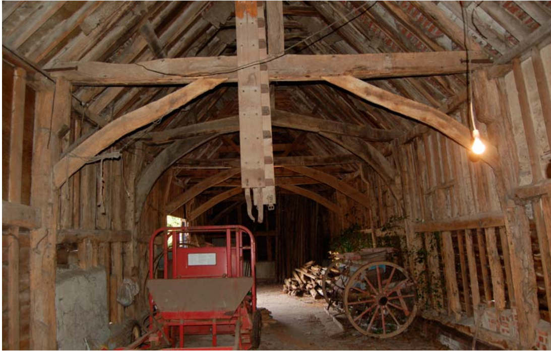
Plate 5 Interior viewed to north from T6
