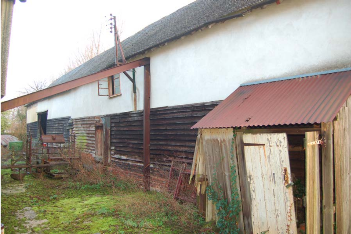
Plate 3 Barn viewed to north-east
