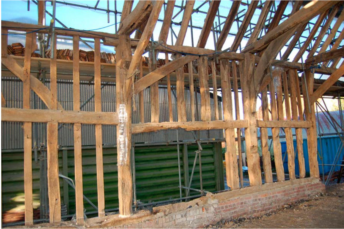
Plate 11 Join between barn 1 and extension 2 and former window, viewed to north-east
