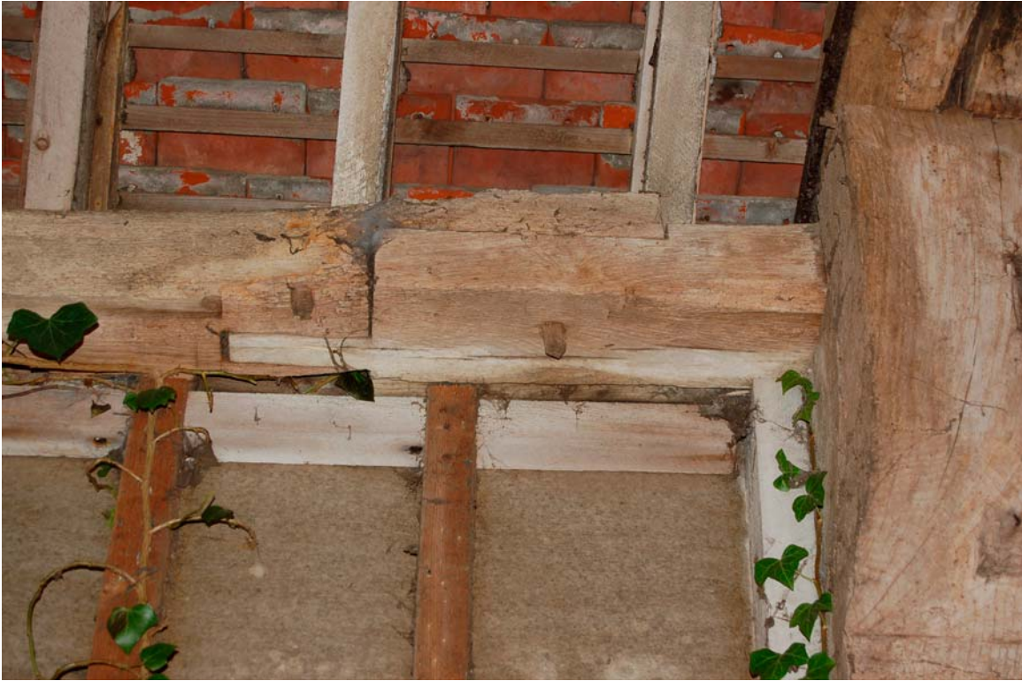
Plate 7 Bridge-scarf joint in bay 3 east (midstrey)
