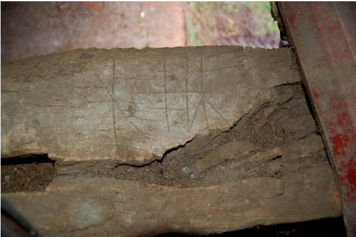
Plate 12 Tagged carpenter's mark (13) on west side of T3 tie-beam
