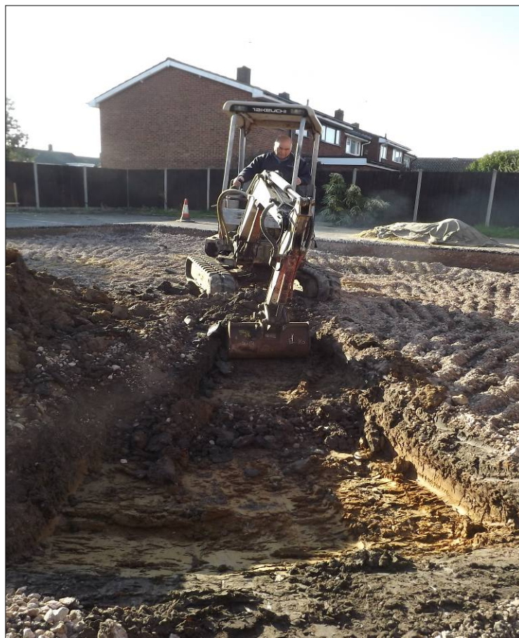
Plate 2. The trench under excavation
