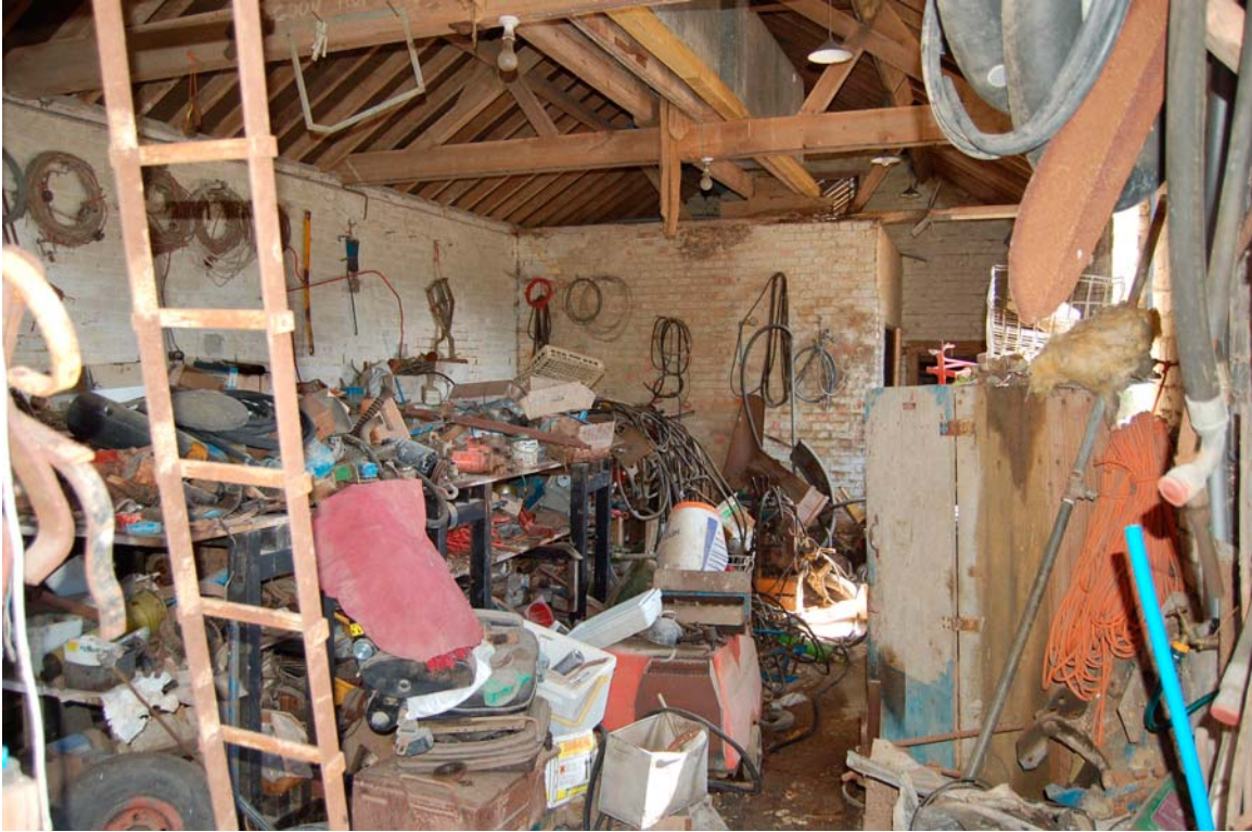
Plate 13 Interior of cow house 2 viewed to south-east
