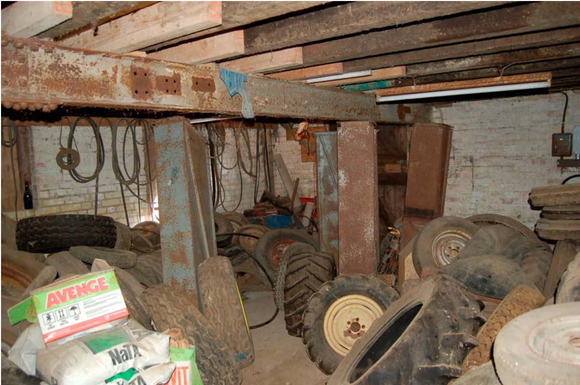
Plate 14 Mill room 3 interior viewed to south-east
