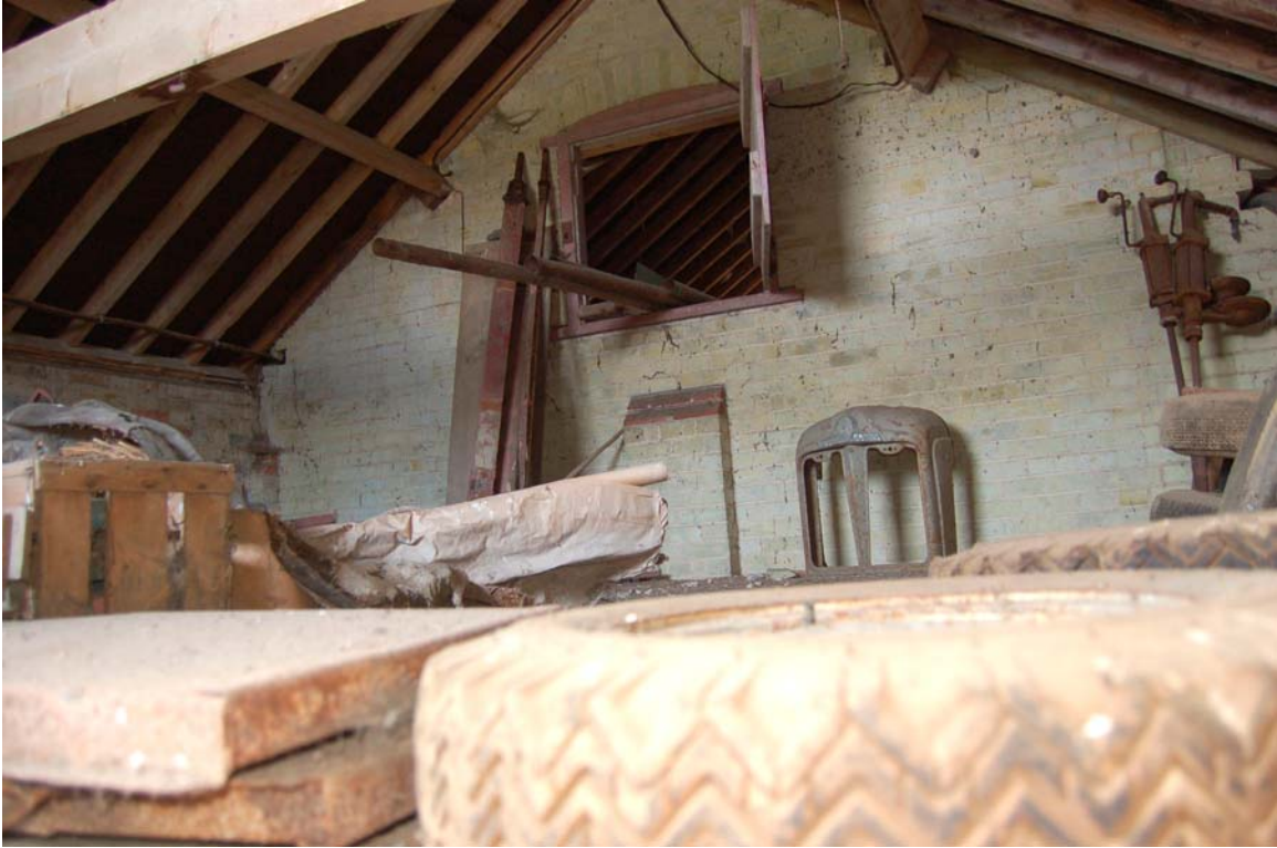
Plate 15 First floor of mill room viewed to north-west
