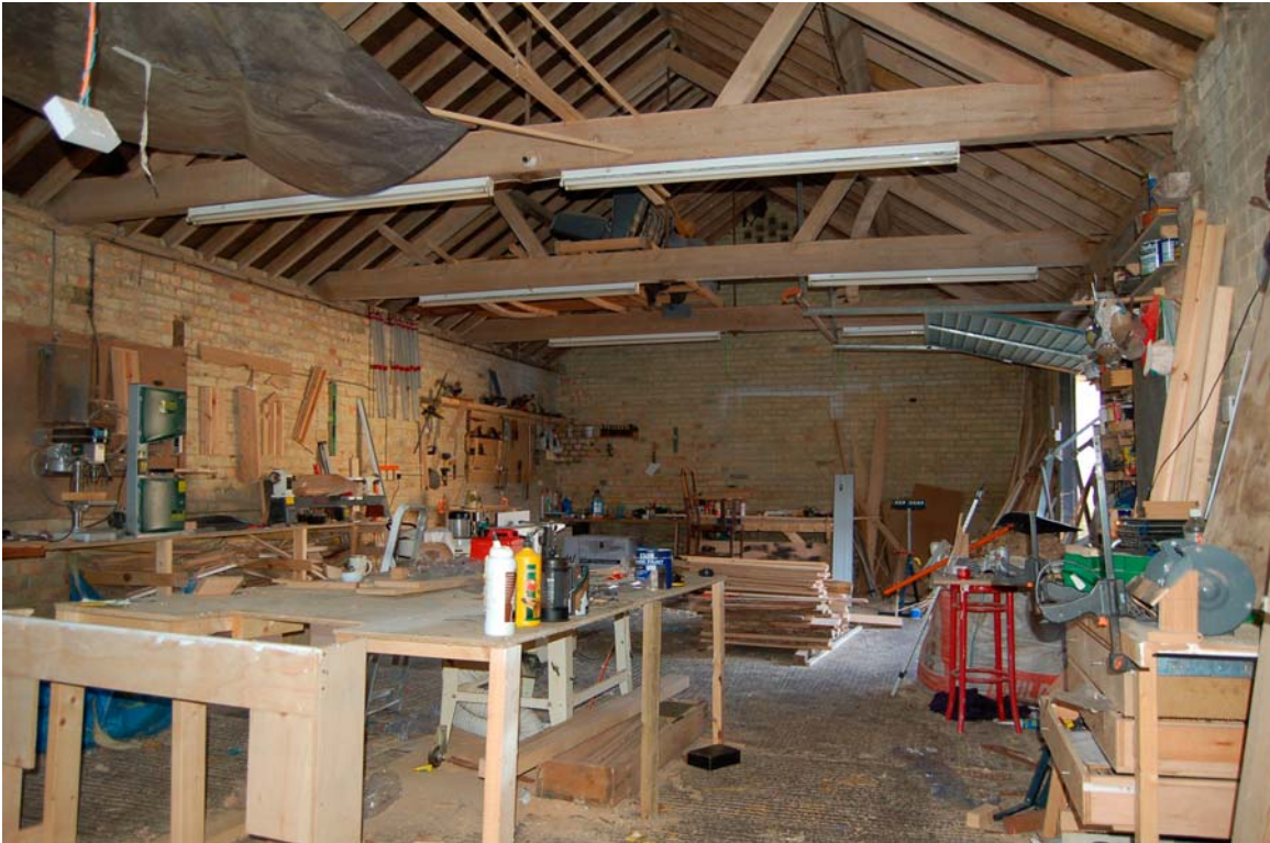
Plate 16 Pig shed 5 viewed to south-west
