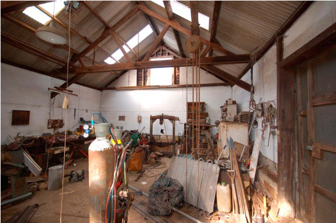
Plate 20 Interior of meal shed viewed to north-west
