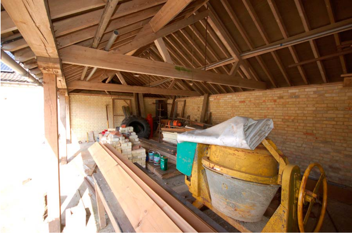
Plate 17 Shelter shed 6 viewed to north-west
