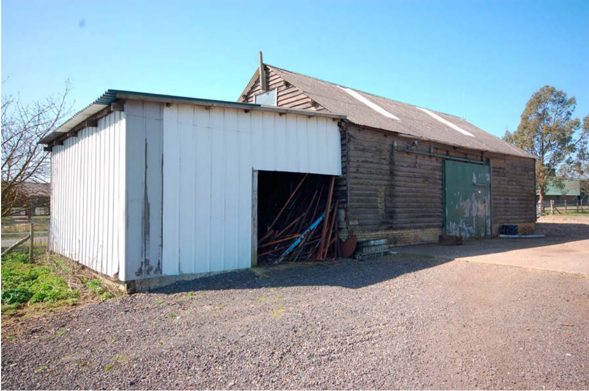
Plate 19 Meal shed 10 viewed to south-west
