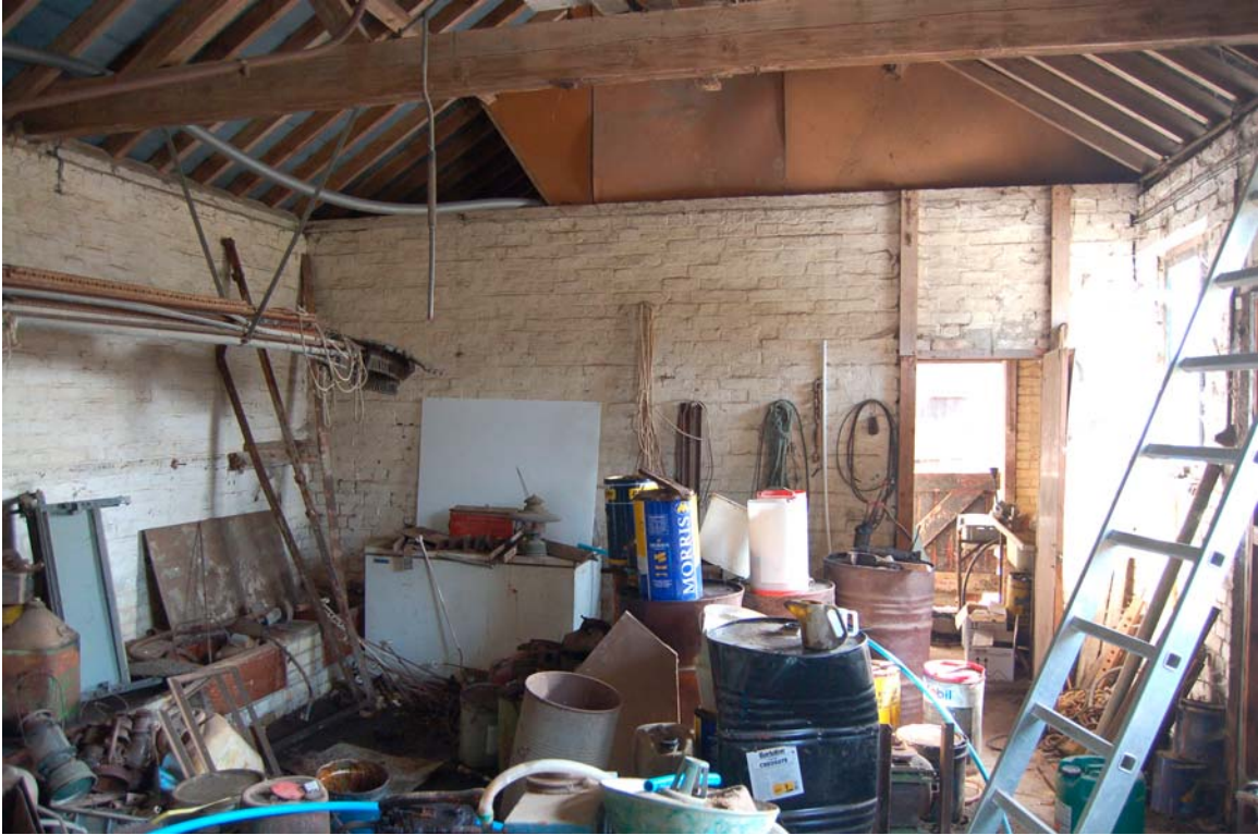
Plate 11 Interior of cow house 1 viewed to south-east
