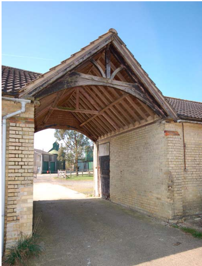
Plate 8 Covered entrance viewed from yard
