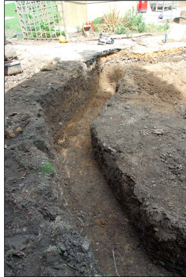
Plate 4. South Trench, looking northeast
