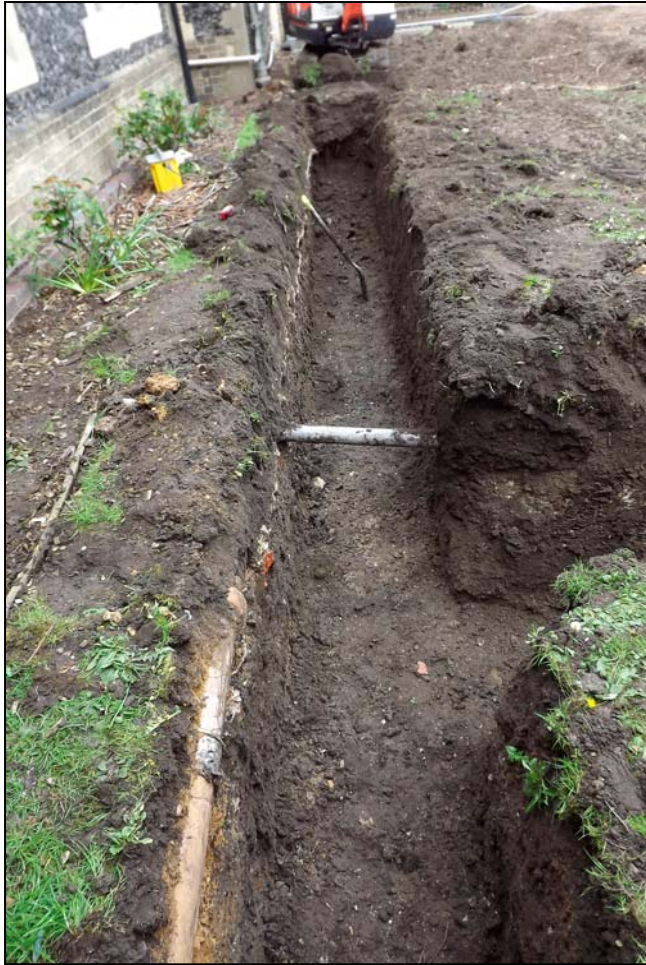
Plate 3. West foundation trench, looking north
