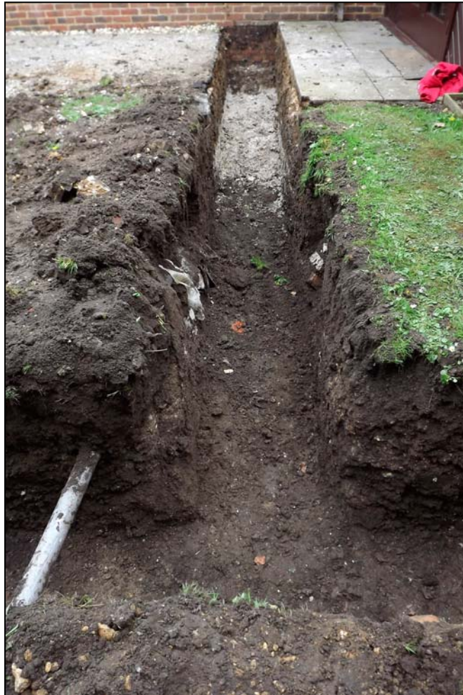
Plate 2. South foundation trench, looking east
