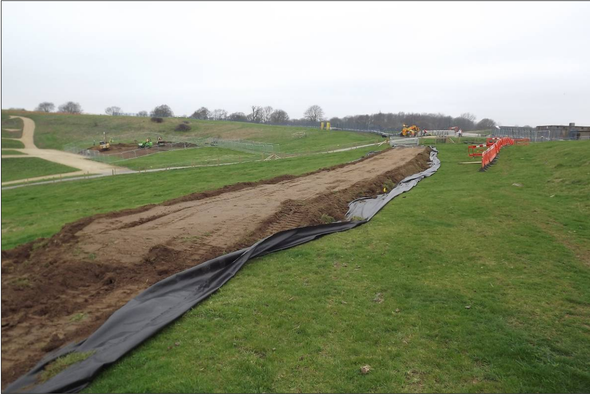
Plate 5. Temporary trackway on Adder's Hill and general site view, looking northwest
