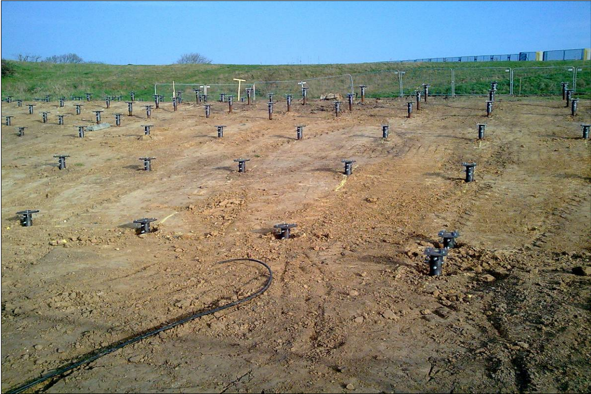
Plate 3. Screw-piles in the Accredited Stand area, looking northwest
