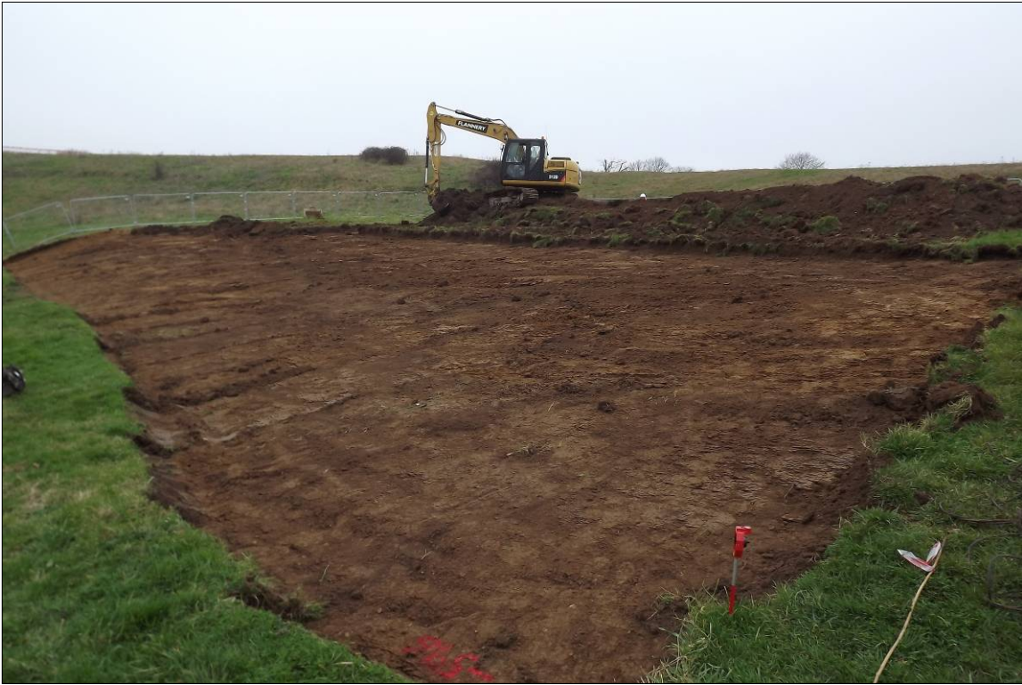
Plate 1. Topsoil stripping in the Accredited Stand area, looking northwest
