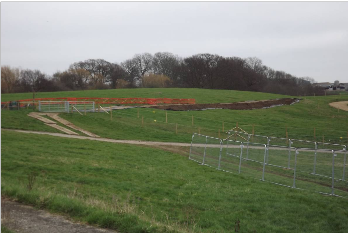
Plate 4. Temporary trackway on Adder's Hill, looking east
