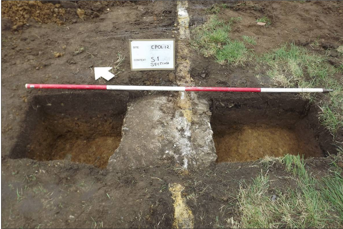
Plate 7. Section through the building foundations
