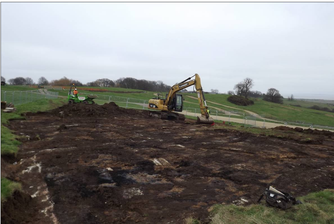
Plate 6. WW II building in the Accredited Stand area, looking east
