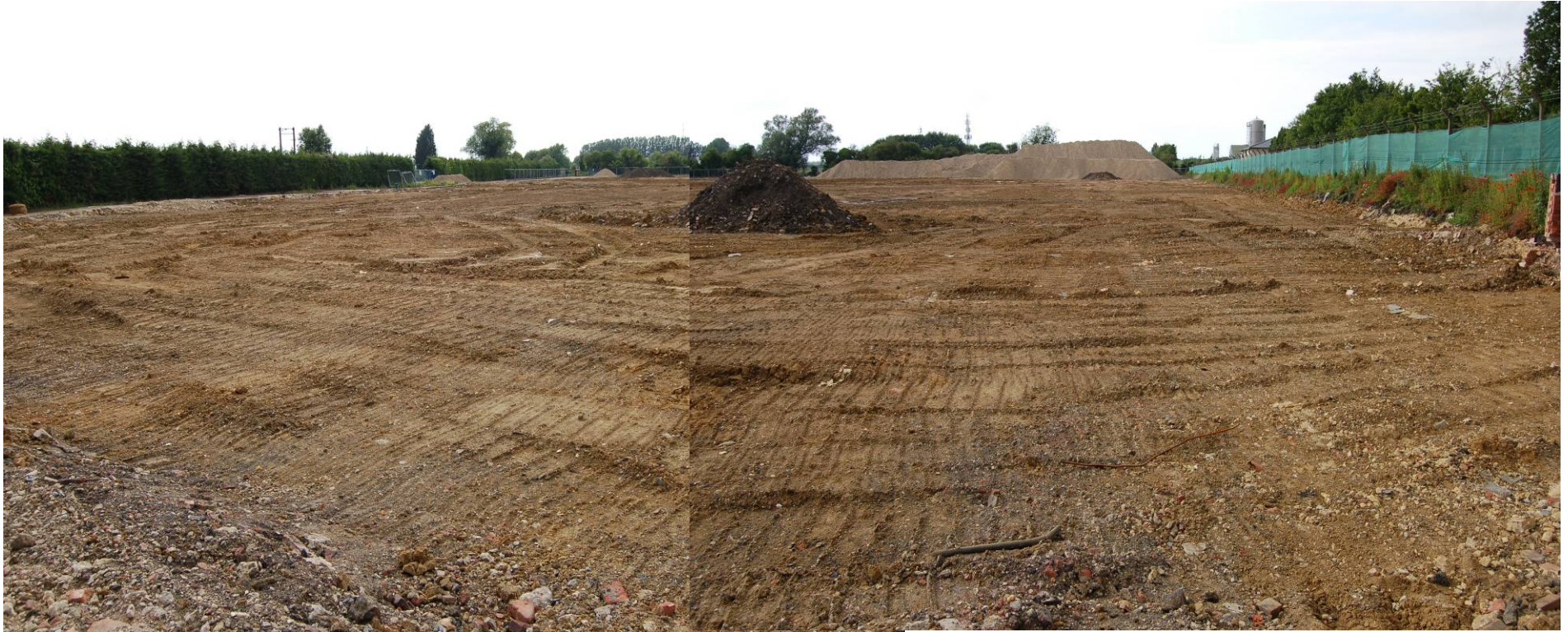
Plate 1. General view of site (composite), looking northwest
