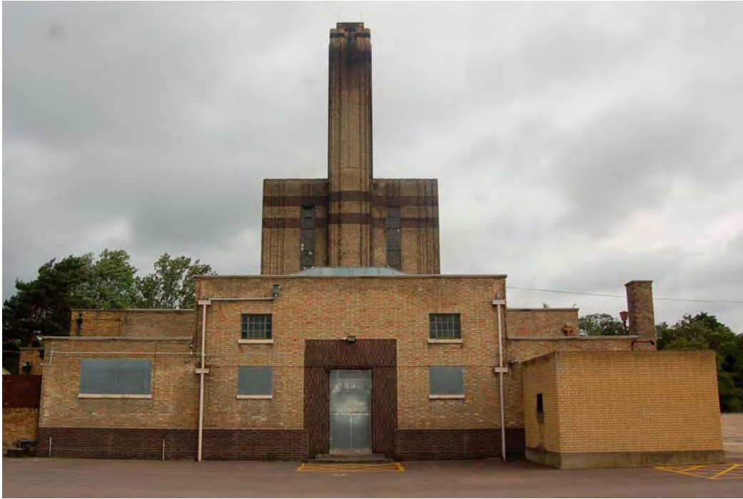
Plate 135 South elevation of Boiler house
