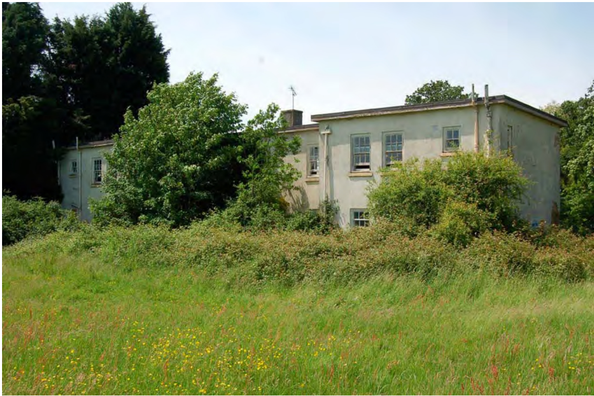
Plate 109 Oakfield viewed to south-west
