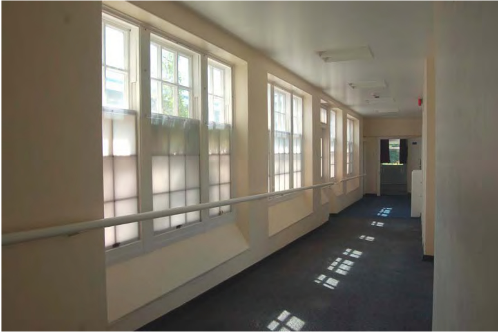
Plate 61 Courtyard corridor R21
