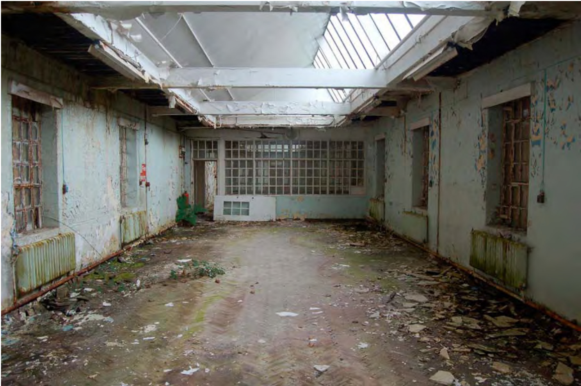
Plate 148 Room R3 & supervisor's office
