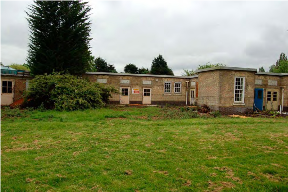
Plate 41 Isolation rooms and former verandah (Ambleside)
