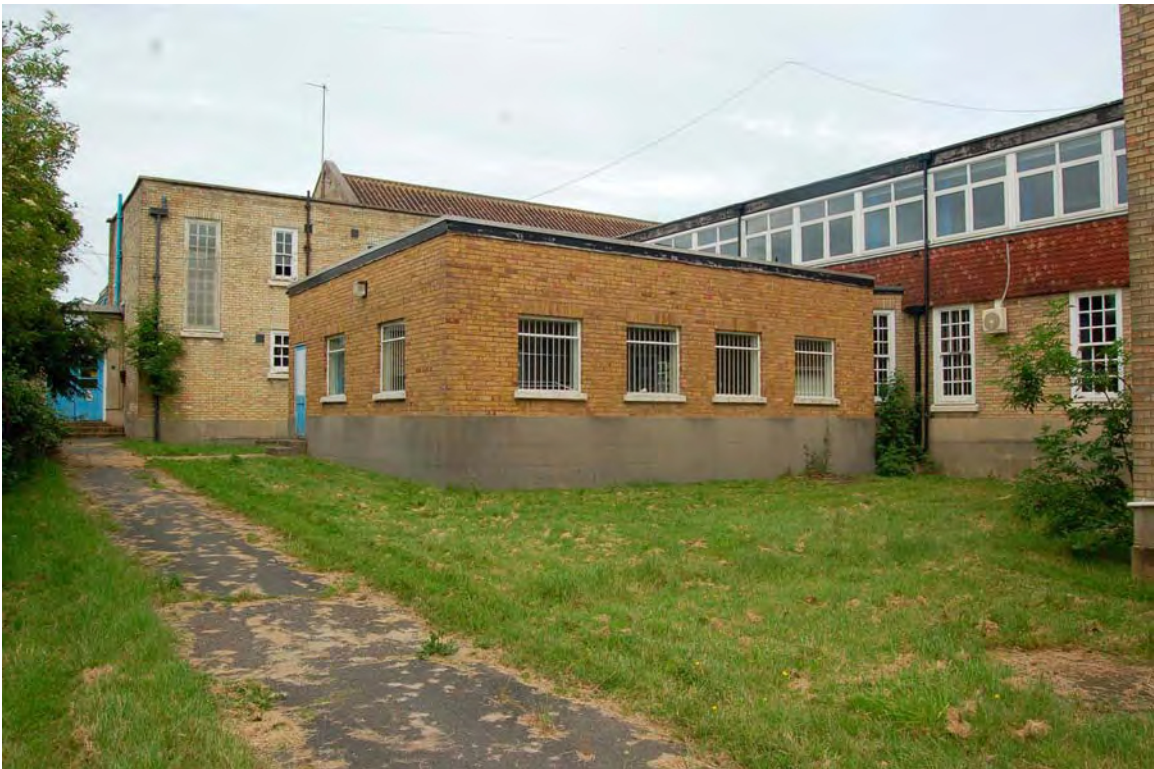
Plate 4 West elevation of administration building
