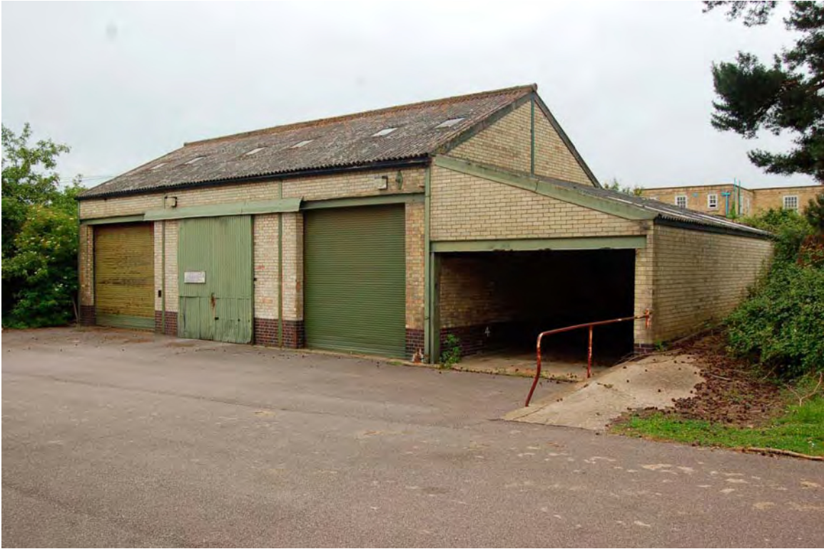
Plate 163 Porter's Garage viewed to south-east
