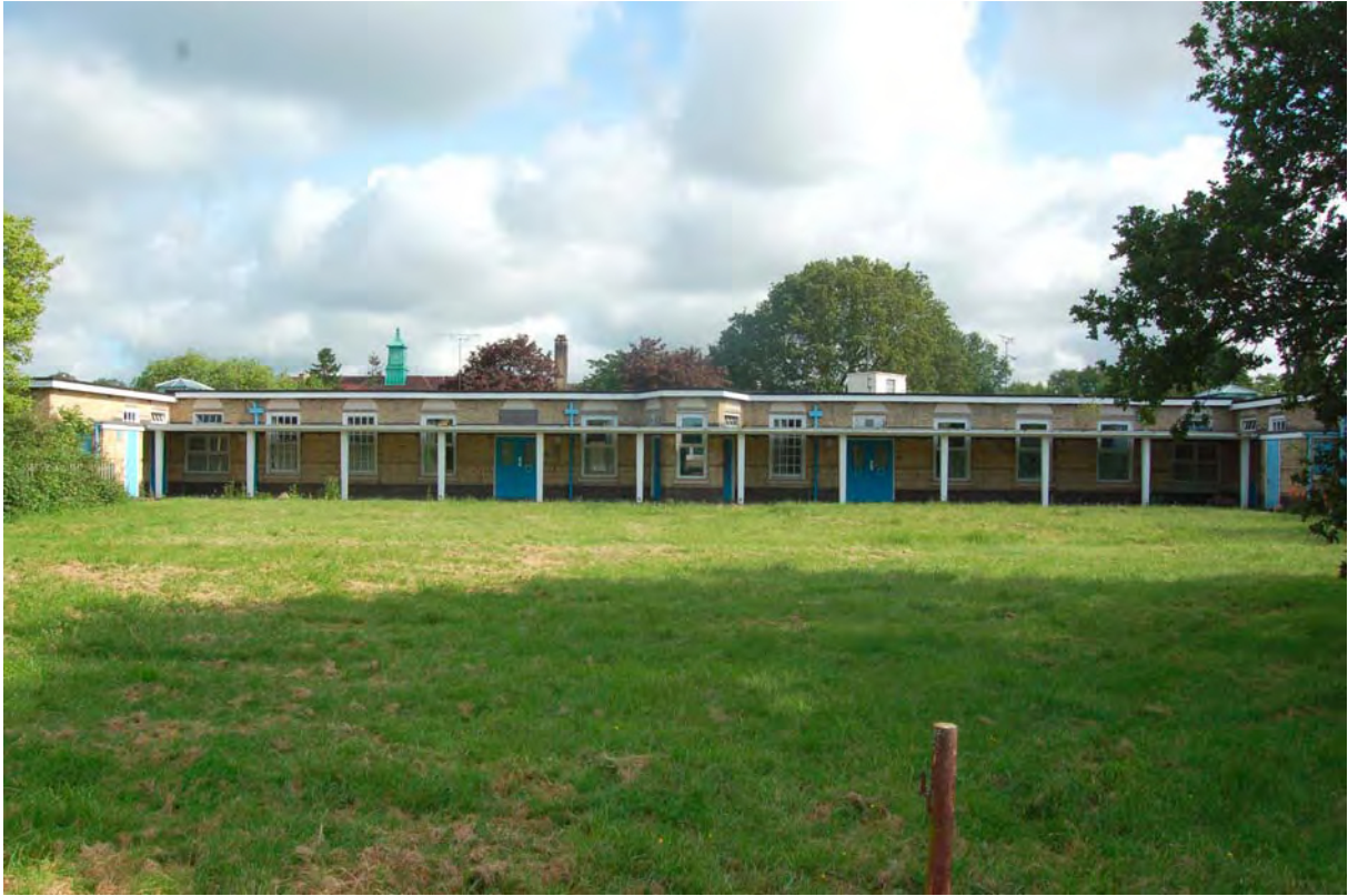
Plate 53 Sick hospital verandah (Dove)
