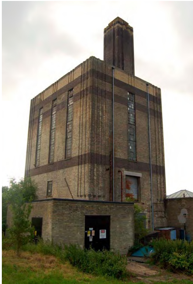
Plate 136 Tower viewed to south-east
