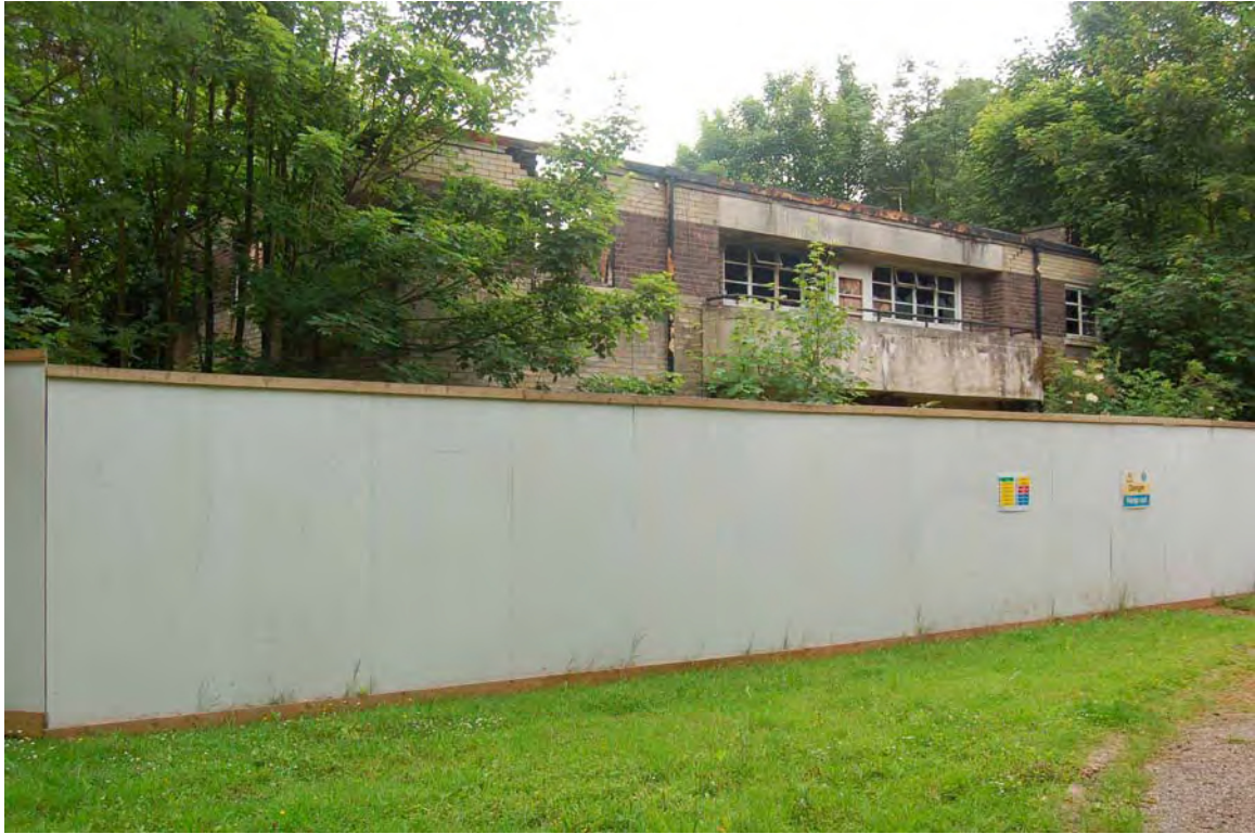
Plate 153 West elevation of Charters
