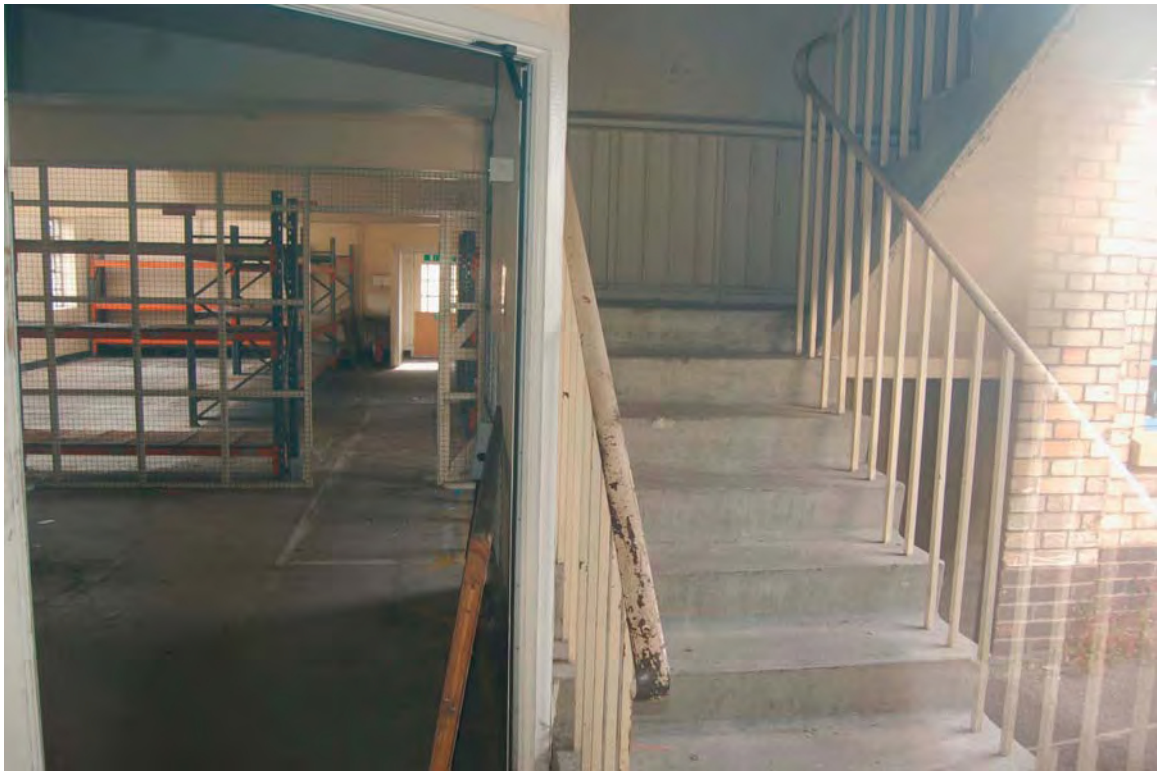
Plate 143 Storage area and stair
