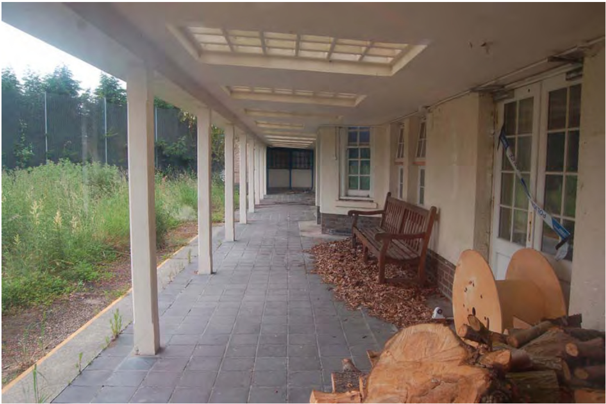
Plate 55 TB hospital verandah (Oakview)
