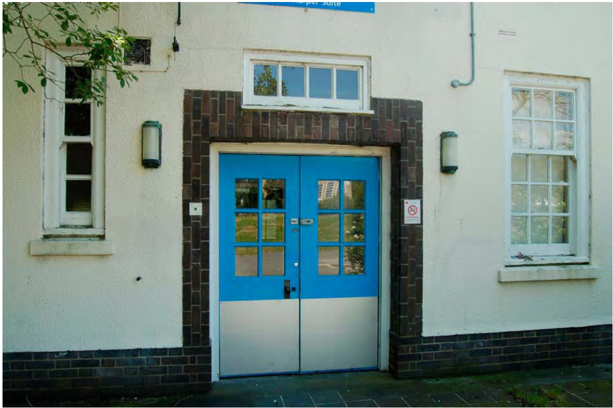
Plate 51 Typical Harper Unit doorway
