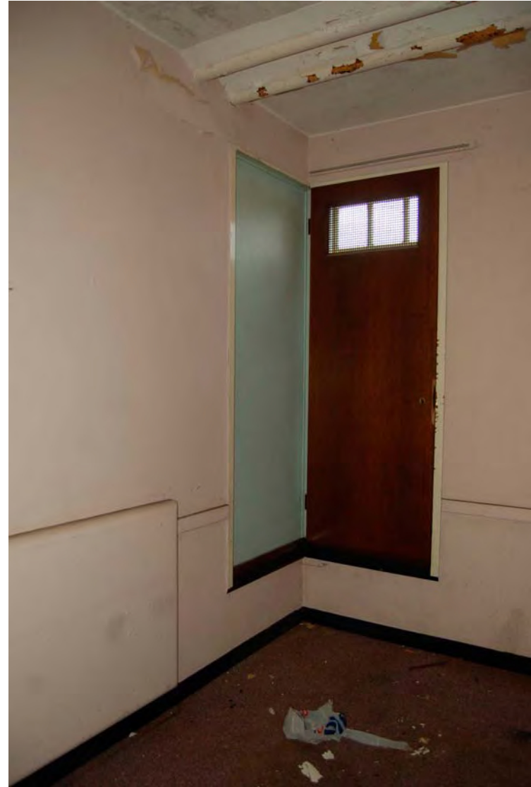
Plate 48 Typical isolation room interior
