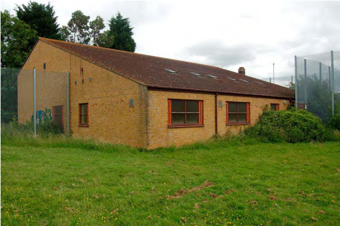
Plate 174 Sports Hall viewed to north-east
