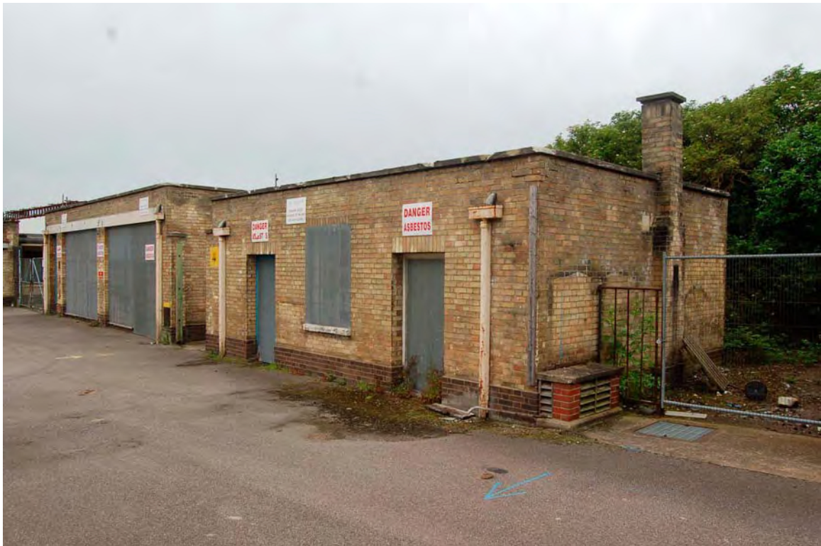
Plate 134 Workshops R13/14 & R38 viewed to south-west
