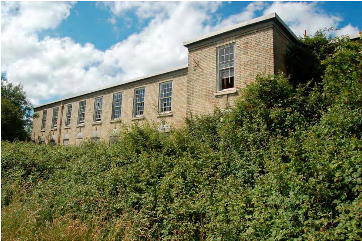
Plate 119 Windsor & Sandringham viewed to north-west
