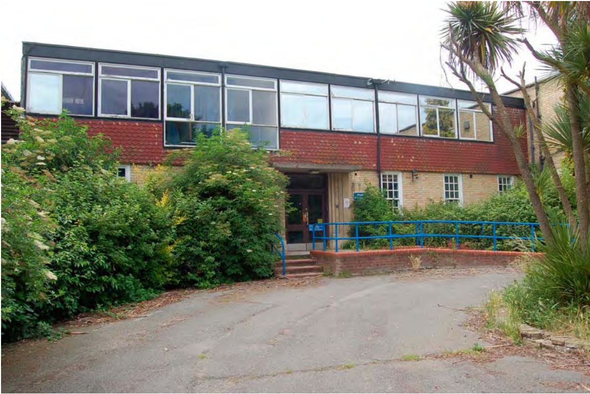
Plate 5 Reception area of east side of administration building
