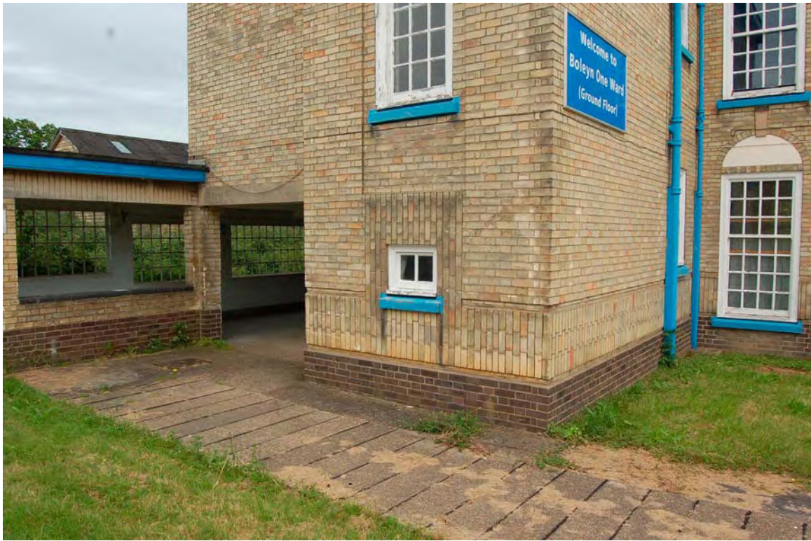
Plate 79 Detailing below stair window
