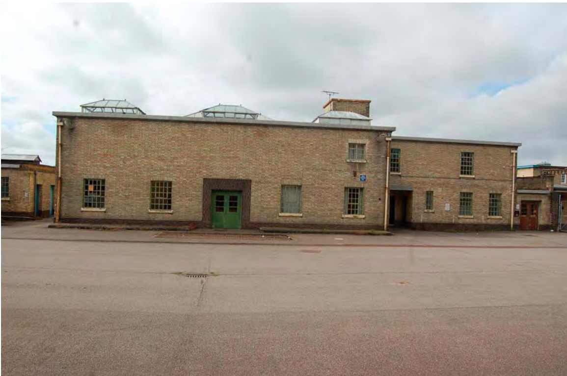
Plate 142 North elevation of kitchen stores
