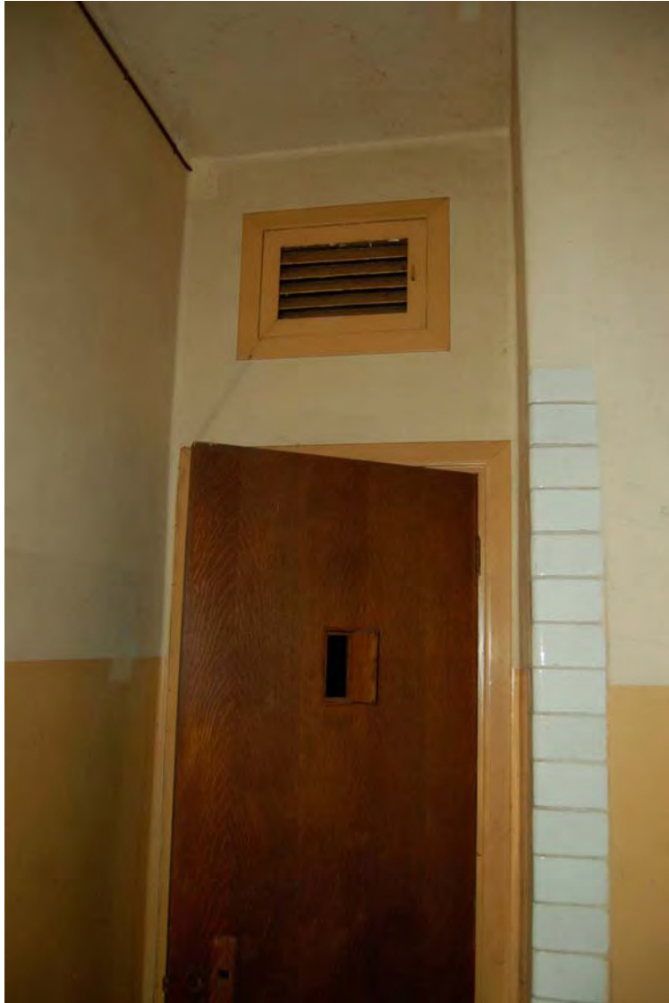
Plate 47 Extant spy-hole and ventilation grill over isolation door
