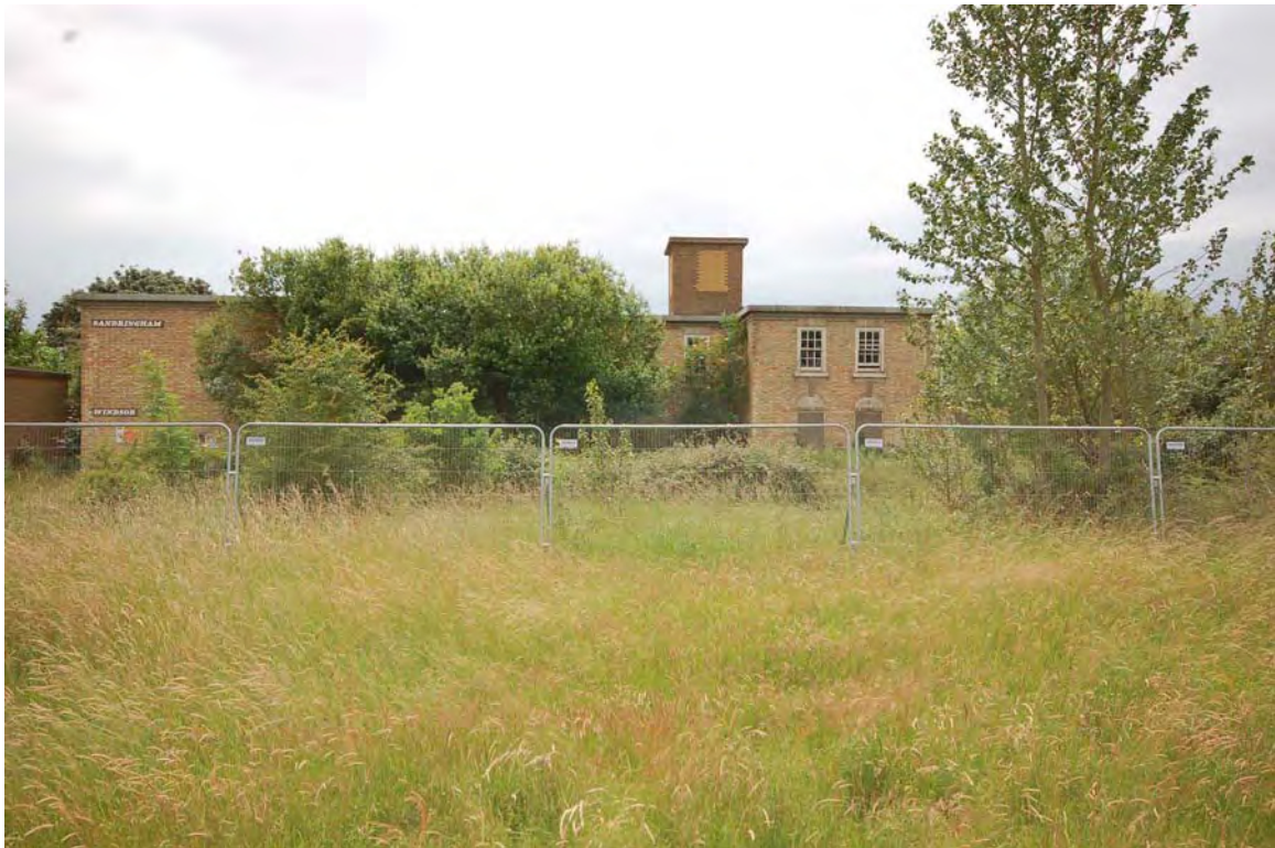
Plate 116 Boundary House (Windsor & Sandringham) viewed to south
