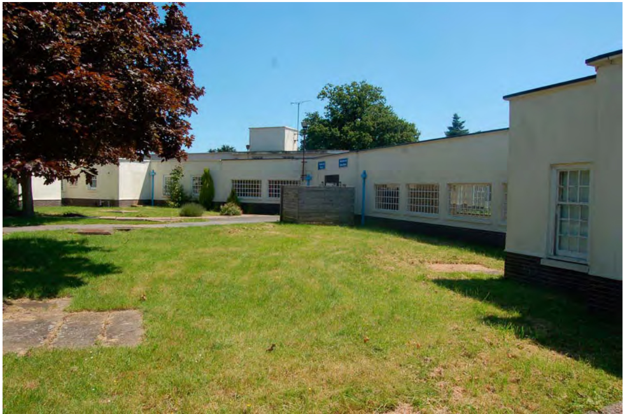
Plate 52 Harper Unit viewed to south-east (Dove & Oakview)
