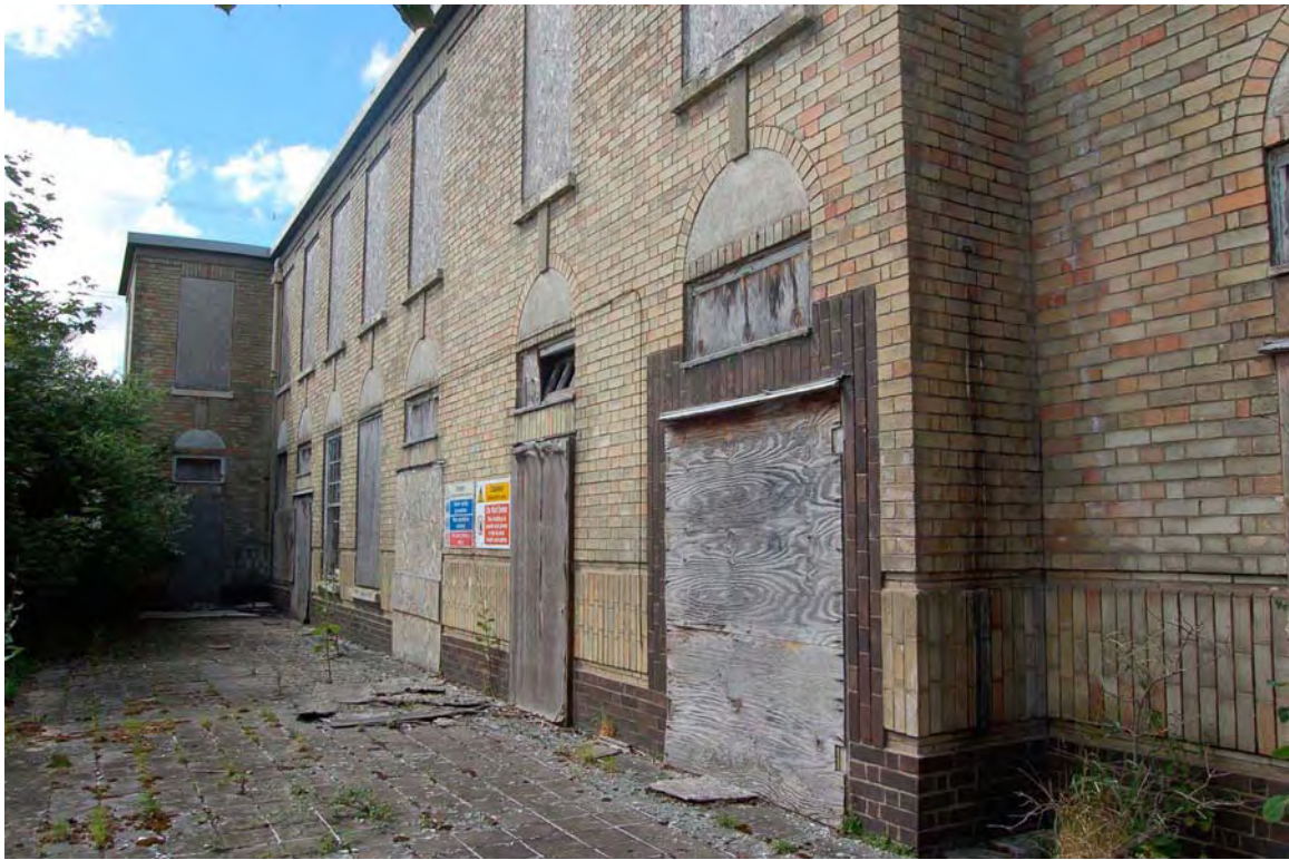
Plate 117 Boundary House terrace (Nightingale)
