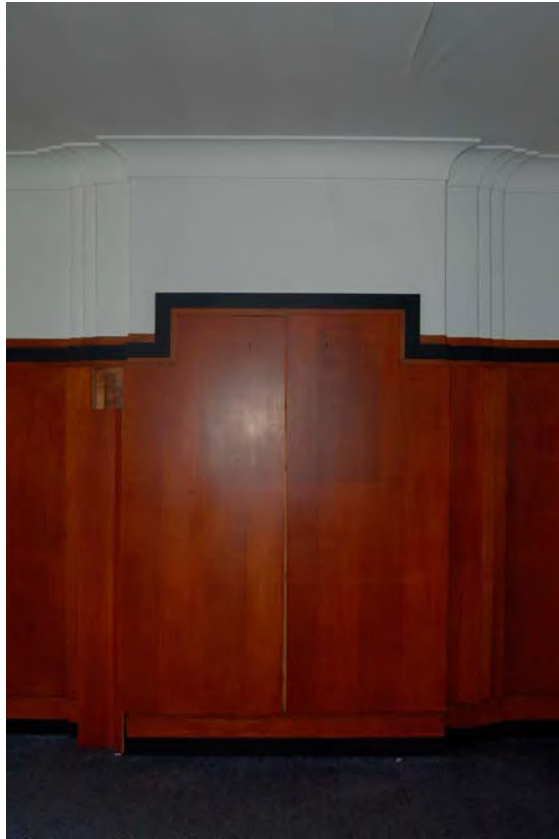
Plate 15 Detailing around stack in meeting room
