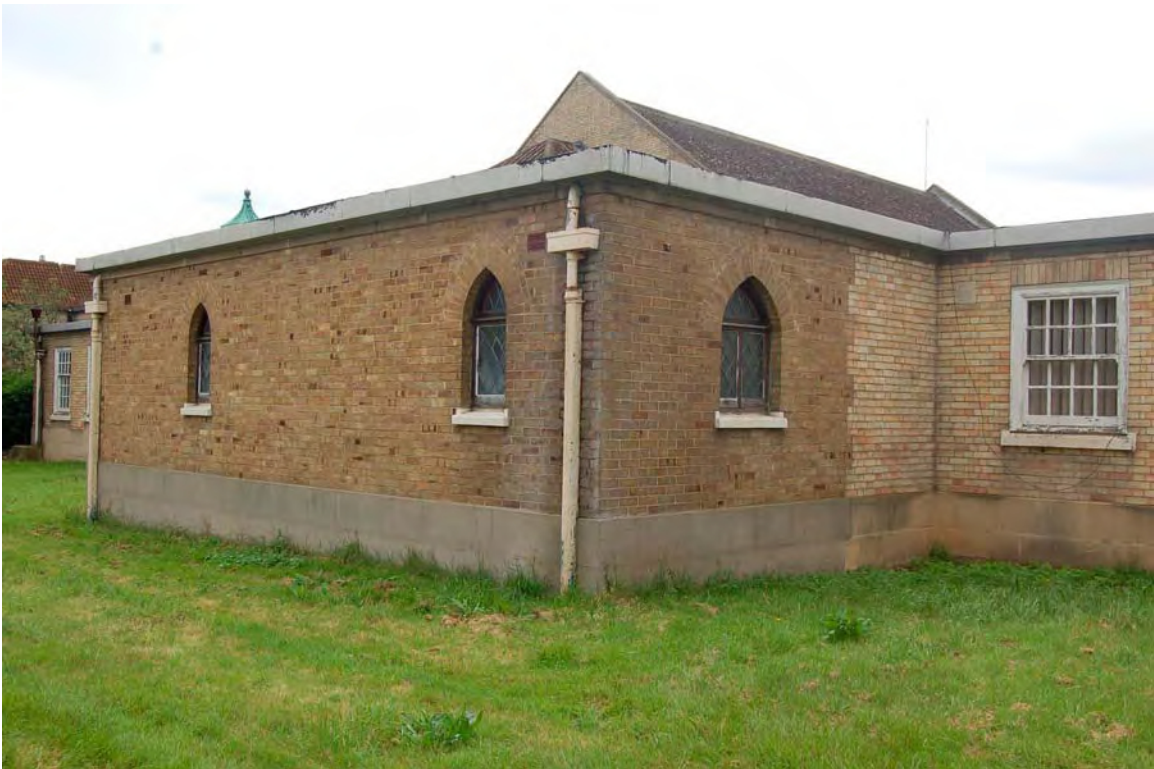
Plate 8 RC chapel viewed to south-west
