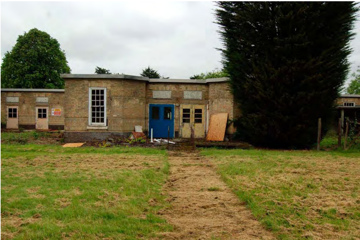
Plate 42 South end of Ambleside ward
