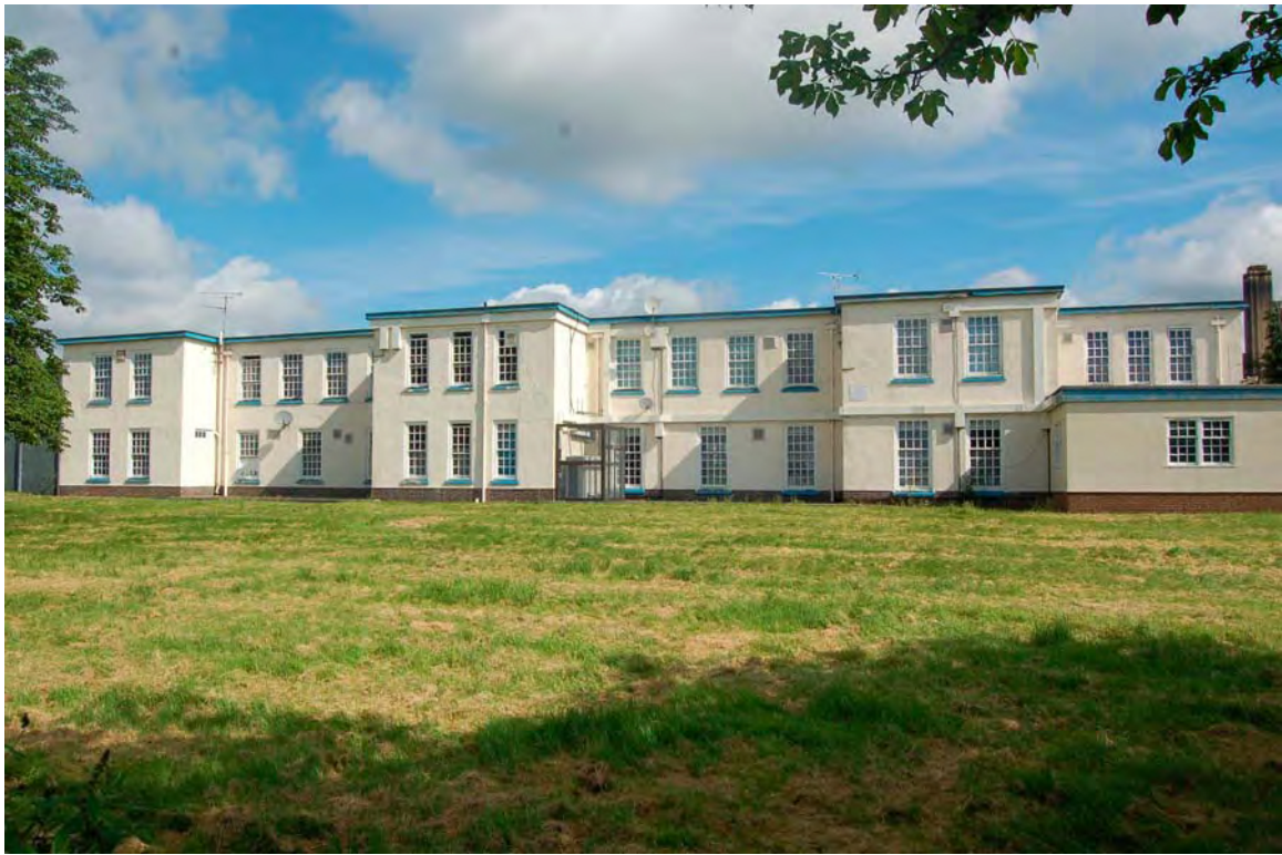
Plate 91 South elevation of Hullbridge
