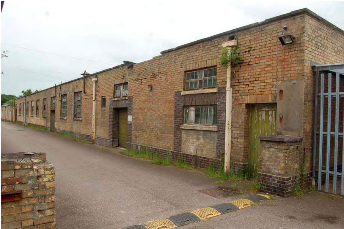
Plate 145 Laundry viewed to south-east
