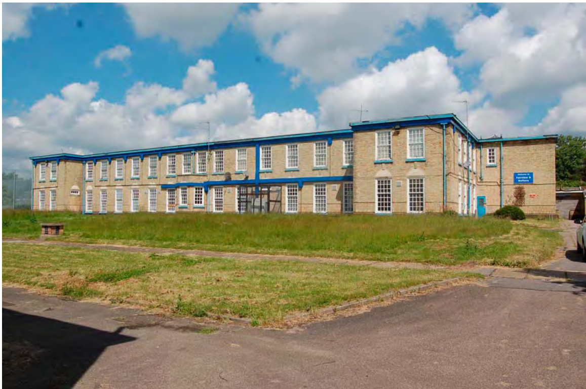
Plate 72 South elevation of Belfairs
