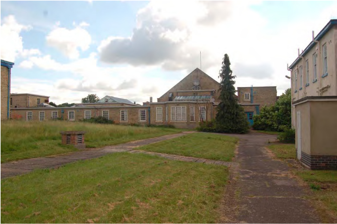
Plate 9 West elevation of administrative building
