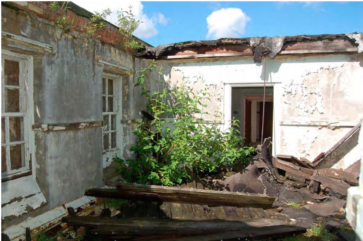
Plate 112 General roof construction (Hillview)
