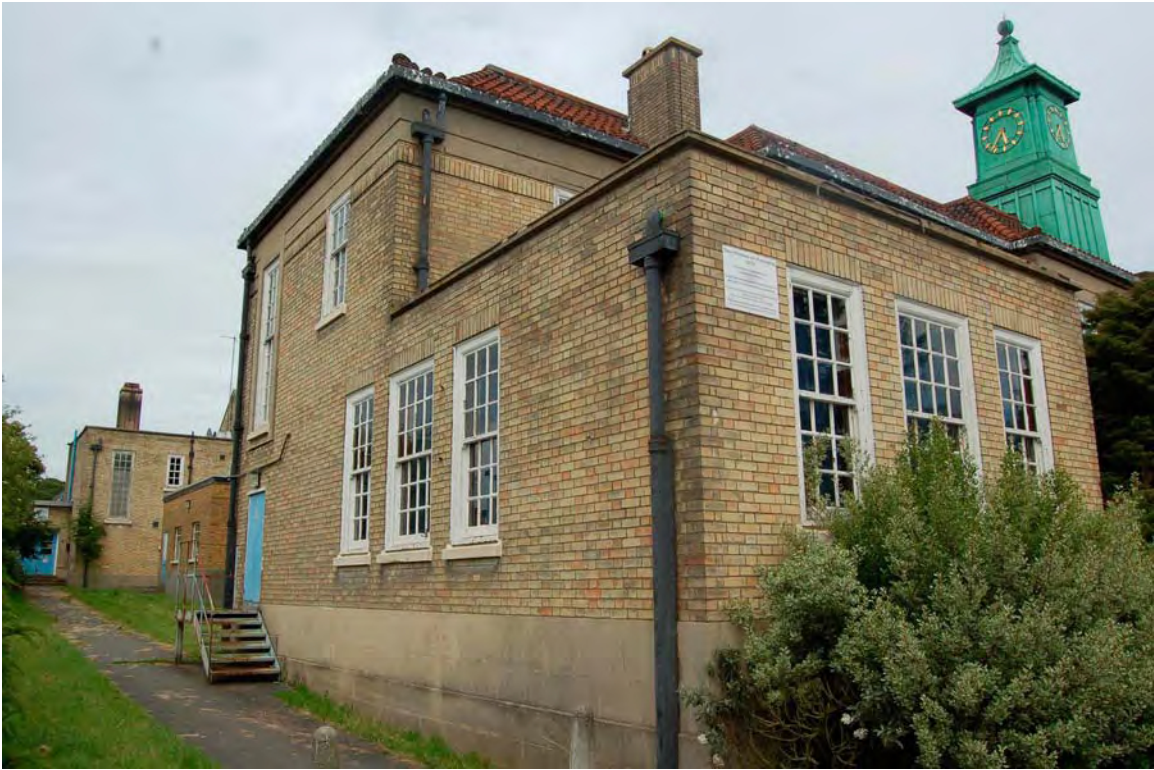
Plate 3 West wing of admin block
