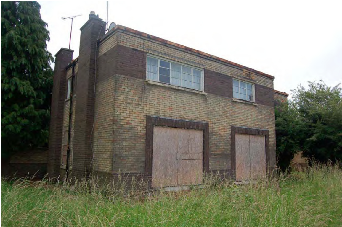
Plate 156 Newick viewed to south-east
