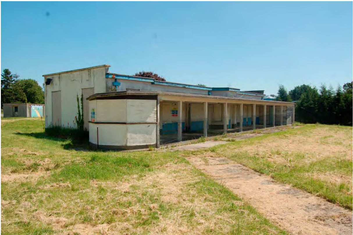
Plate 56 TB hospital verandah (Medical Secretaries)
