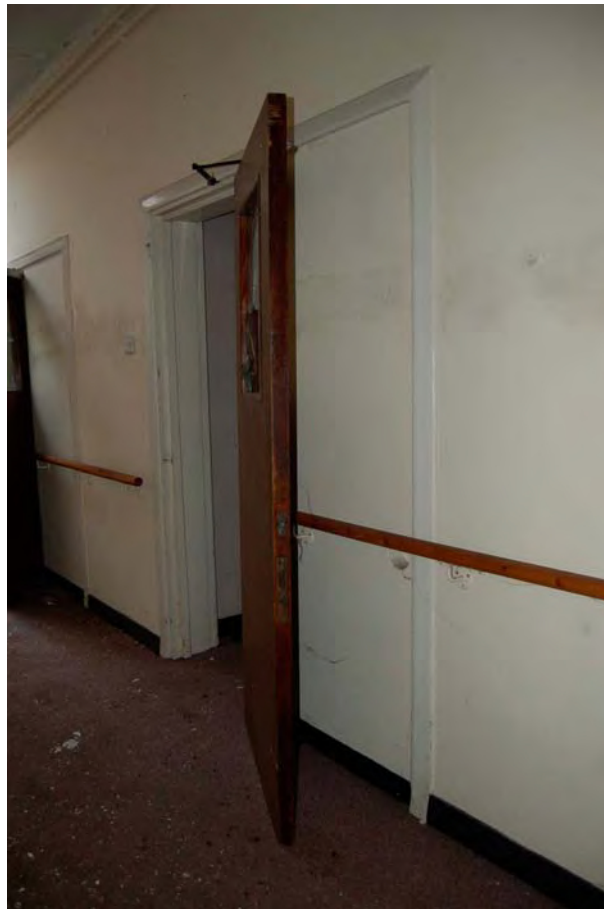
Plate 46 Isolation room viewed from corridor
