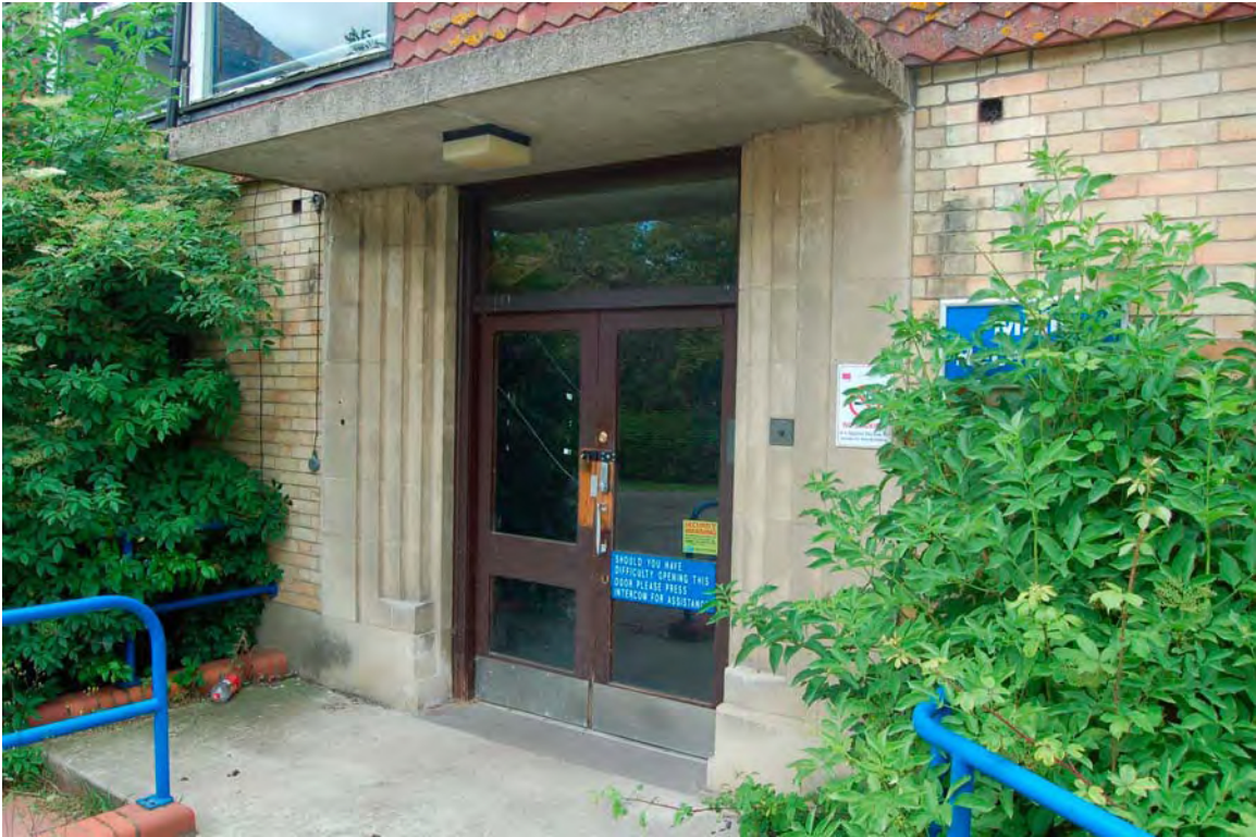
Plate 6 Detail of reception area doorway
