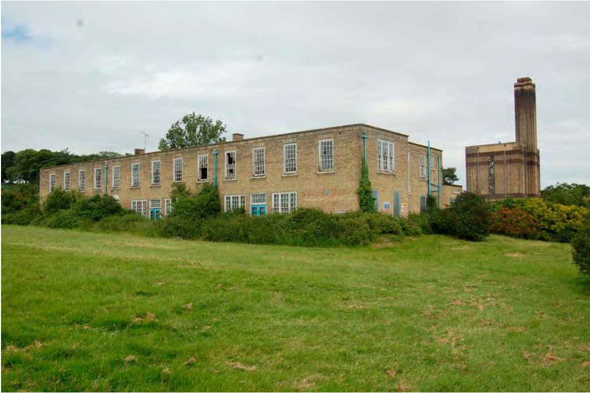
Plate 63 Woodside viewed to north-east
