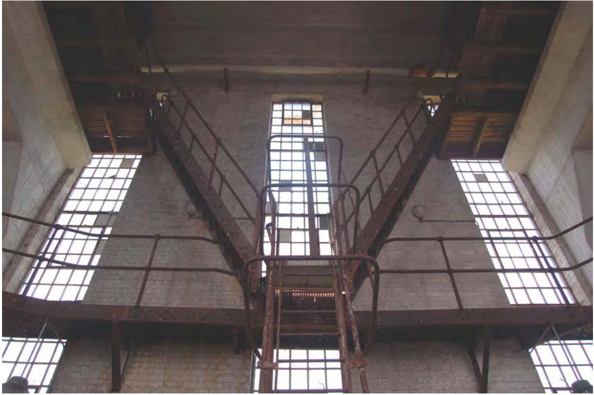
Plate 139 Upper tank room
