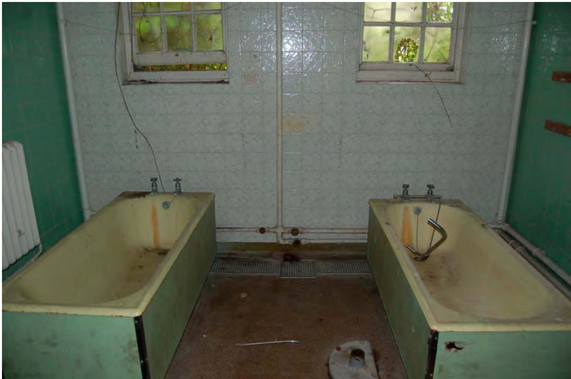
Plate 122 Typical Boundary House bathroom
