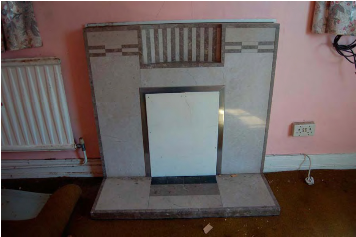
Plate 161 Fireplace in room R12
