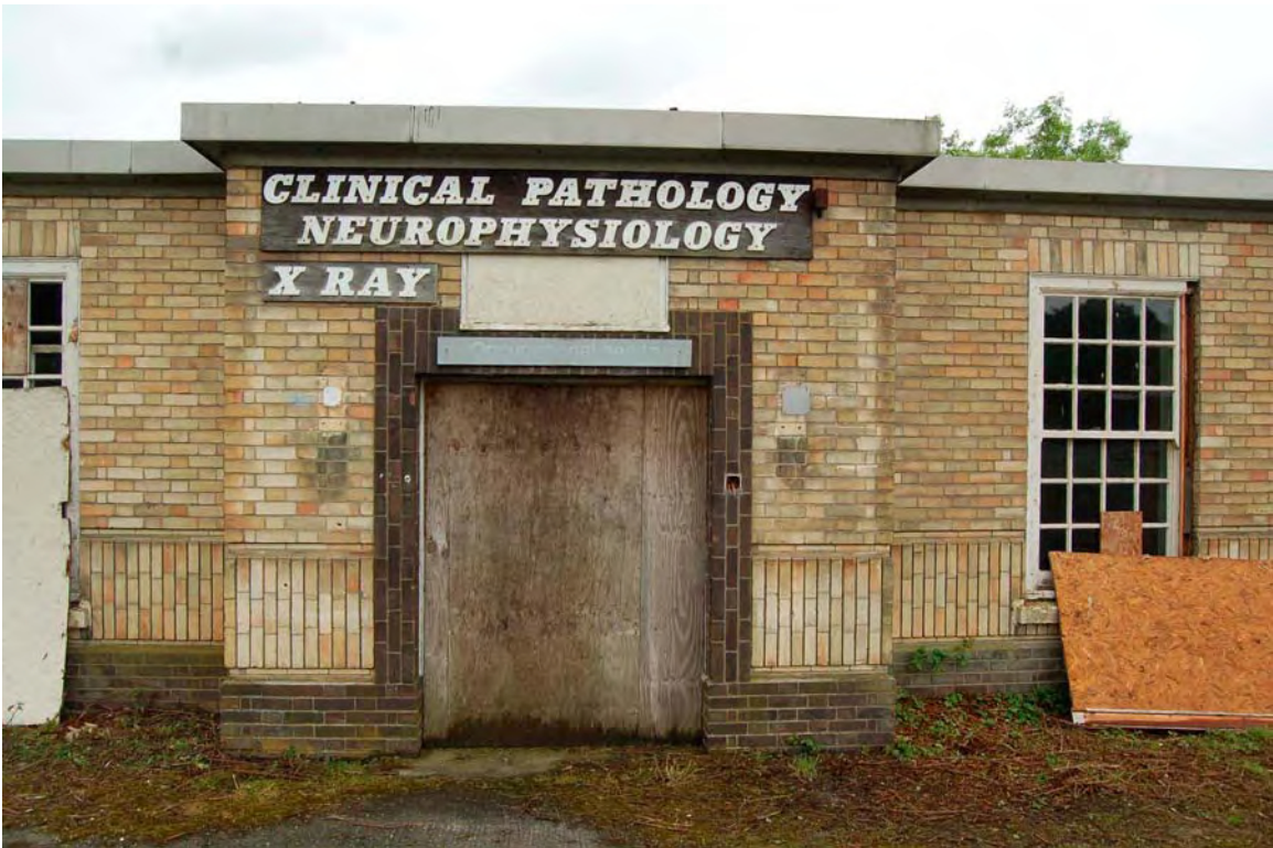
Plate 38 Main entrance into X-ray
