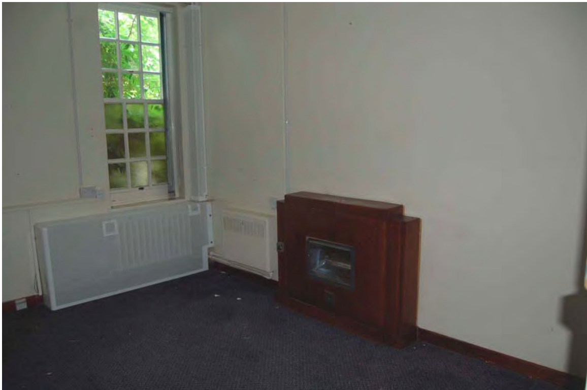
Plate 16 Electric fire in office R21
