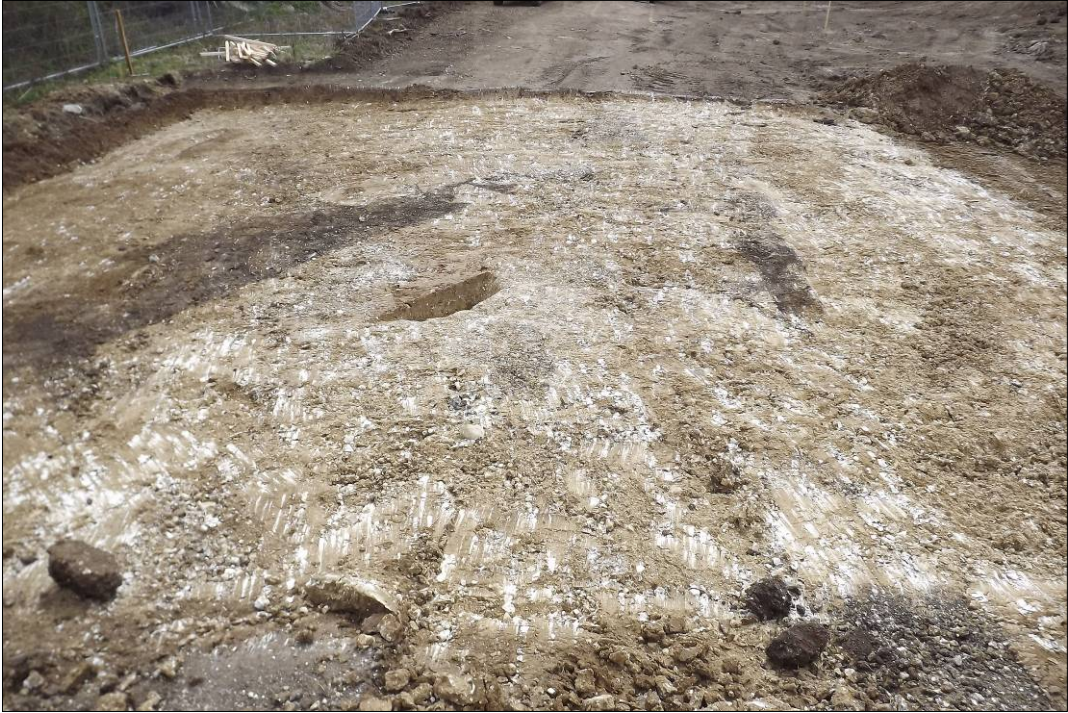
Plate 1. Area 2, looking south-east
