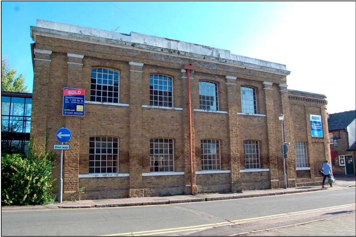
Plate 3. South elevation of silk mill/radio factory
