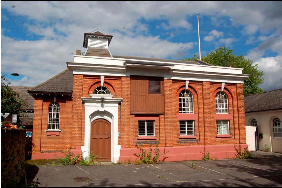
Plate 19. South elevation of pump house
