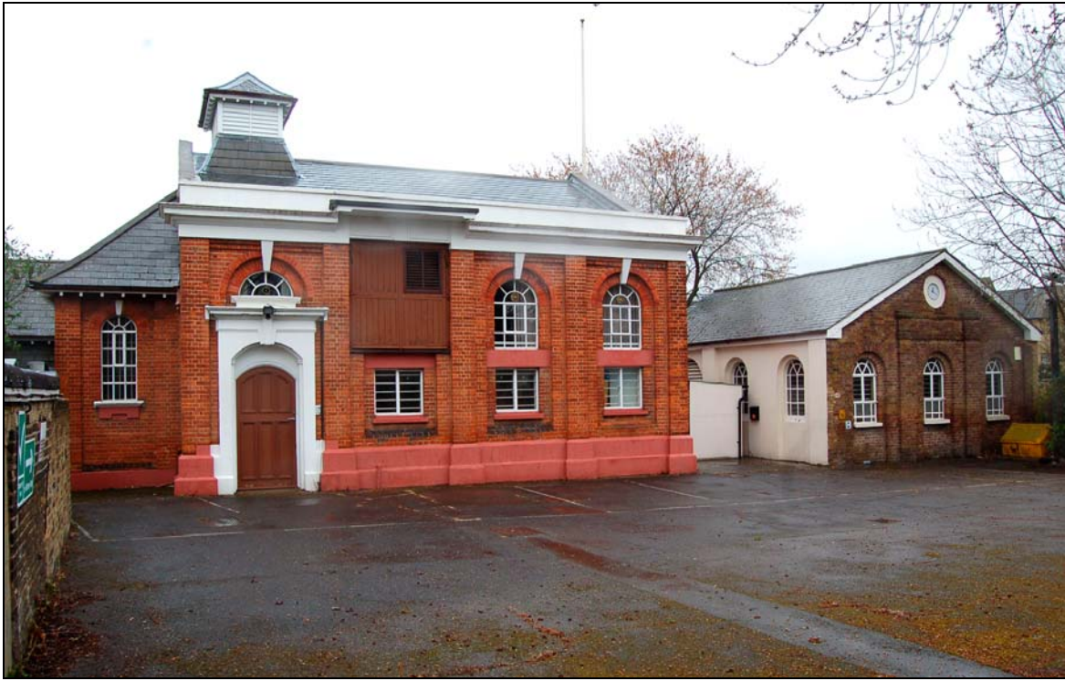
Plate 15. Generator building and pump house, viewed from yard
