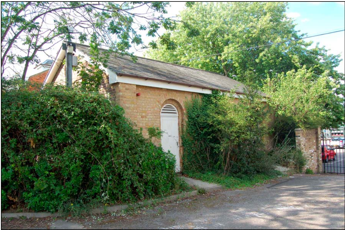
Plate 16. Generator building, viewed to north-west
