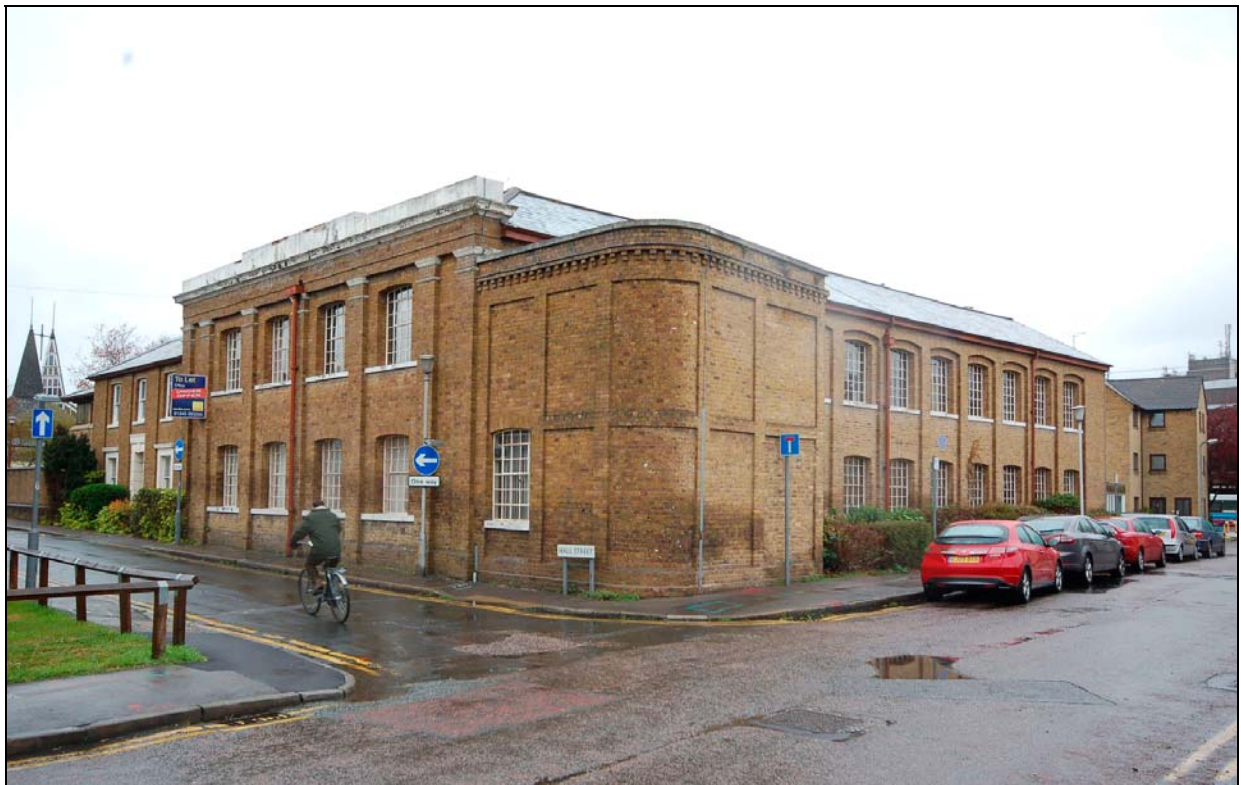
Plate 2 Silk mill/radio factory, viewed to north-west
