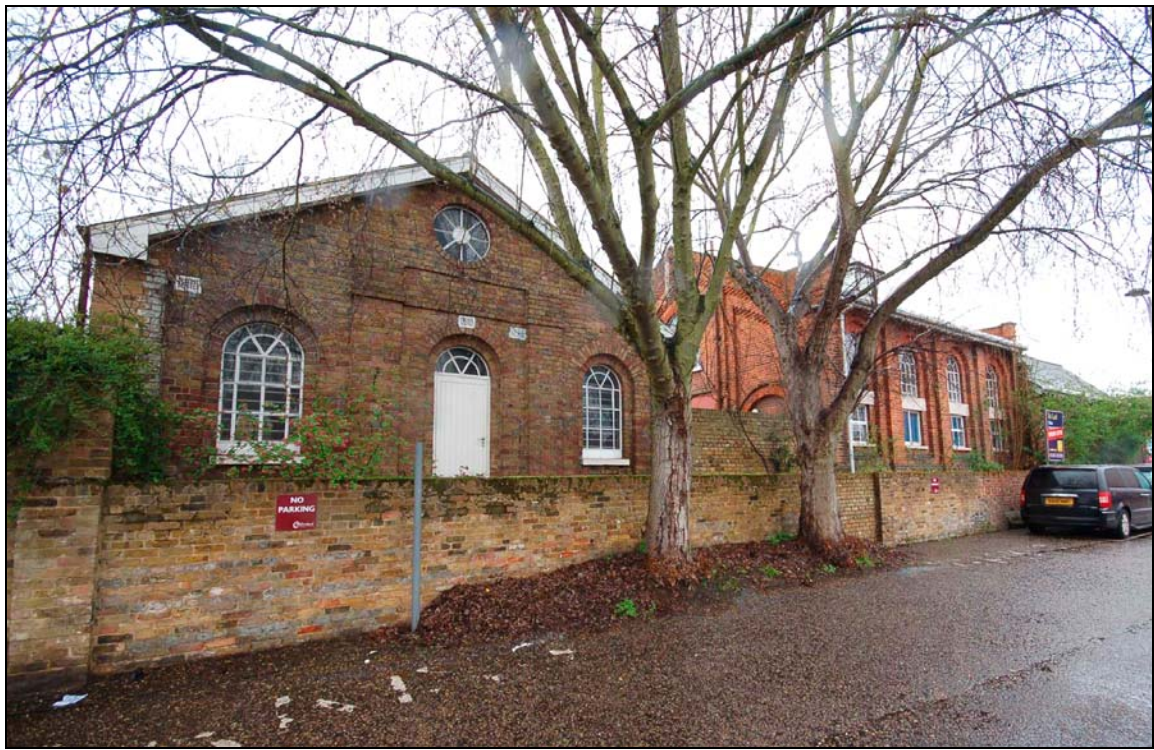
Plate 14. Generator building (left) and pump house, viewed to south-west from car park
