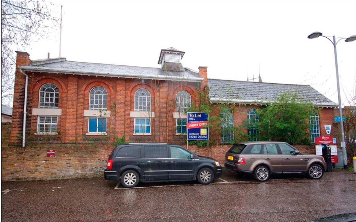
Plate 22. Pump house, viewed to south from car park
