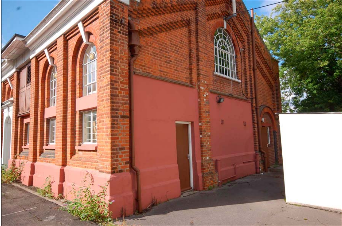
Plate 20. Pump house, viewed to north-west
