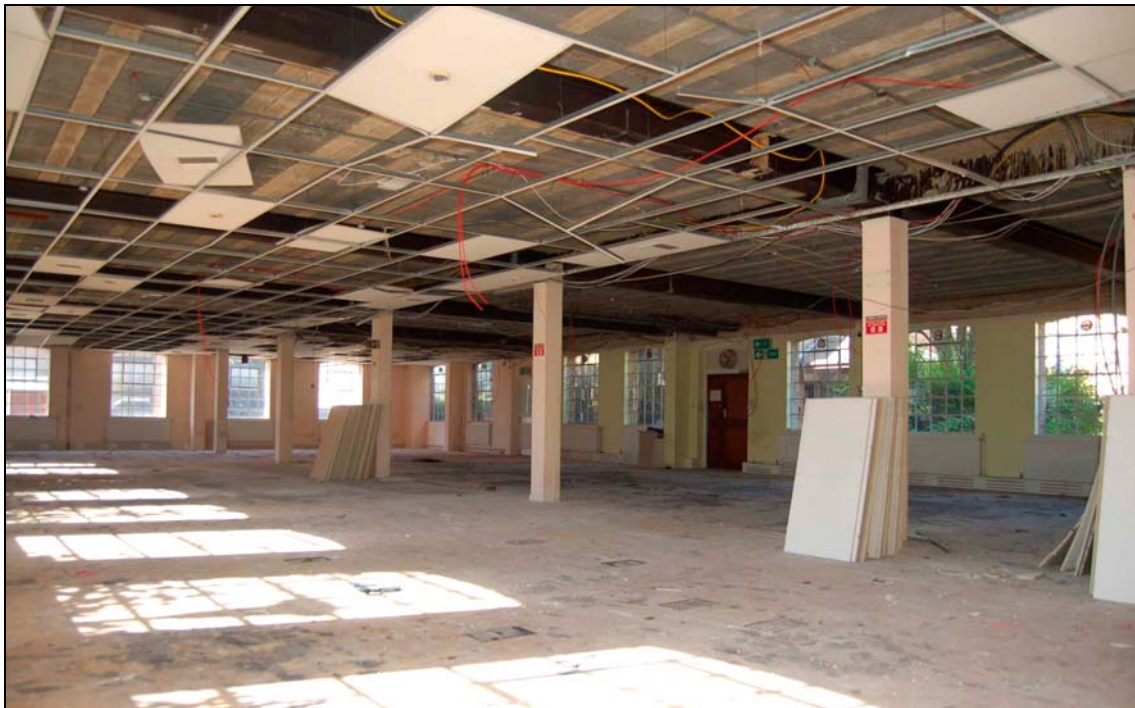
Plate 6. First floor, viewed to south-west after strip
