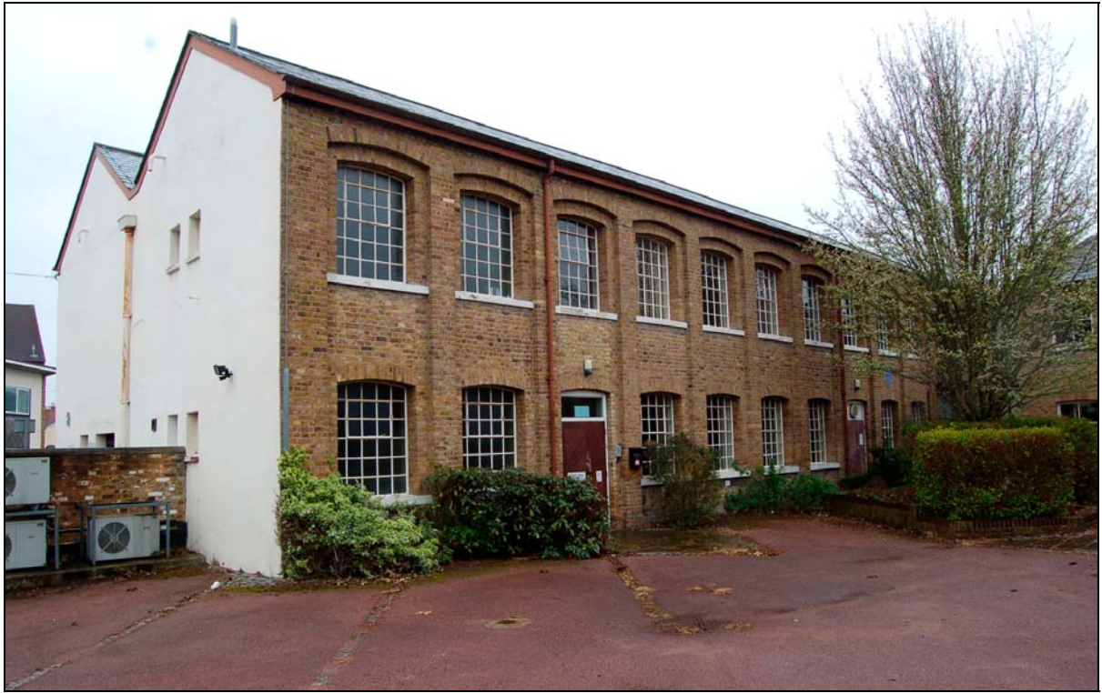
Plate 1. Silk mill/radio factory, viewed to south
