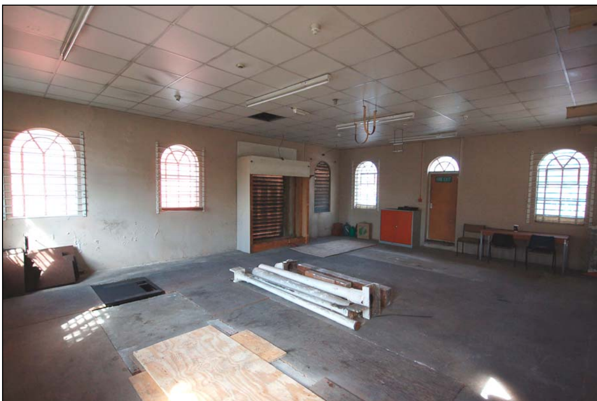
Plate 17. Interior of generator building, viewed to north-west
