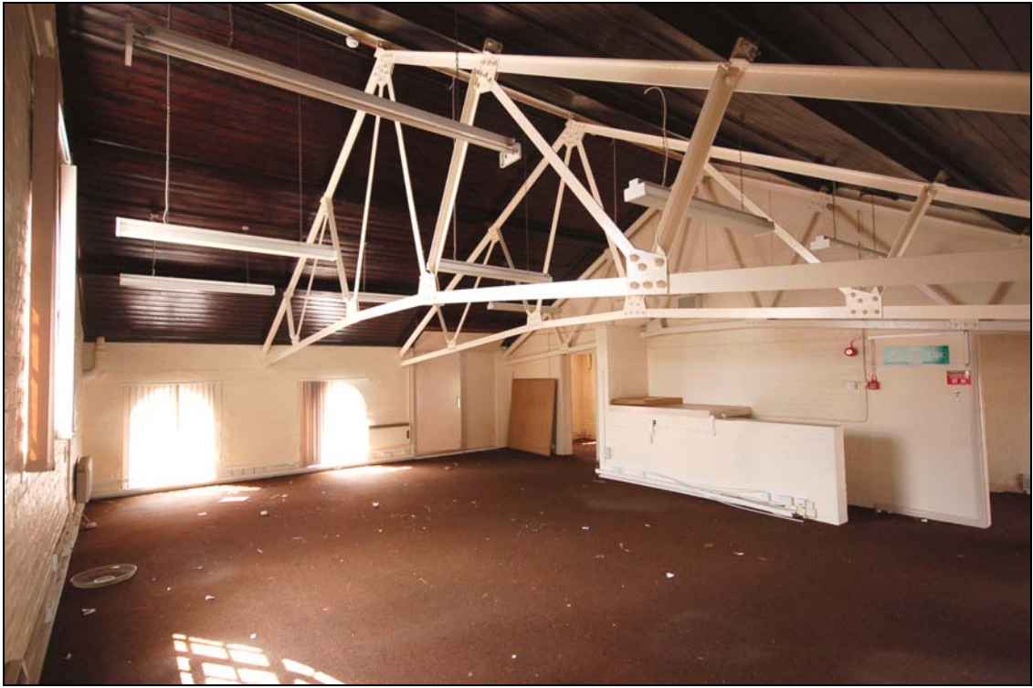
Plate 27. First floor of pump room, viewed to south
