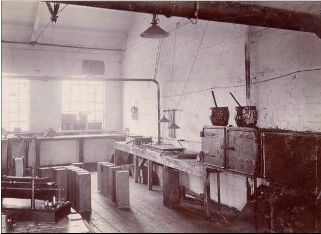
Plate 31. Coil drying workshop (c.1898), radio factory upper floor
