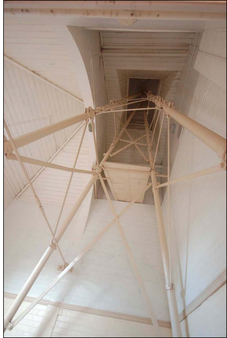
Plate 24. Cast iron frame and maintenance platform
