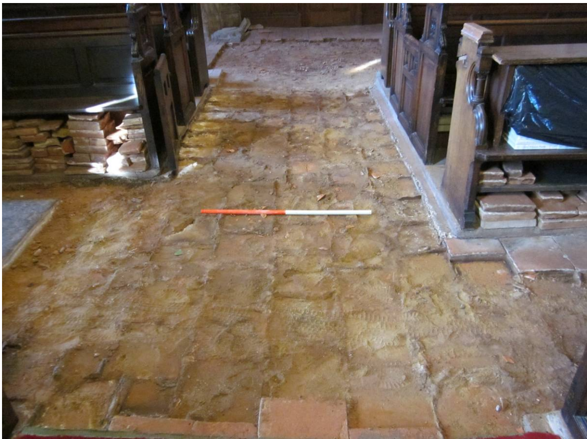
Plate 2: Nave Aisle floor bedding material, looking west (1m scale)
