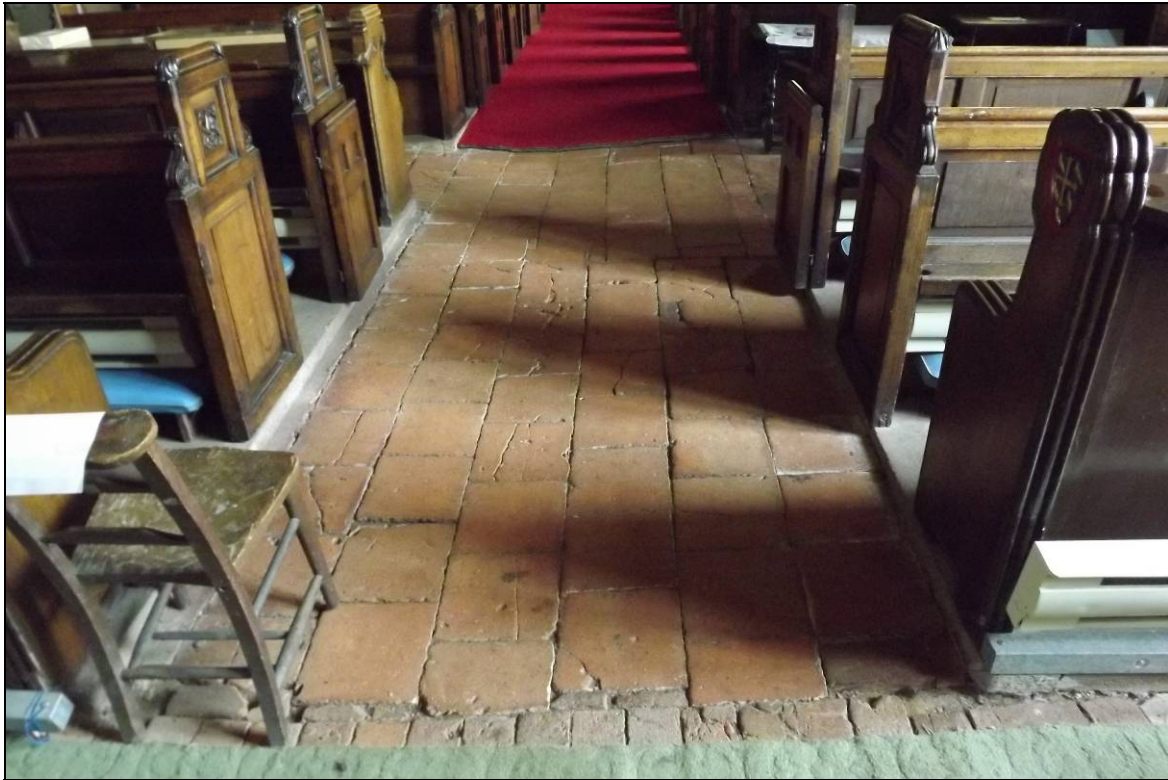
Plate 1: Nave Aisle floor prior to lifting, looking east
