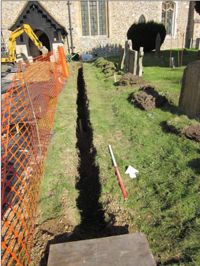
Plate 3. Sewer trench, looking north (1m scale)
