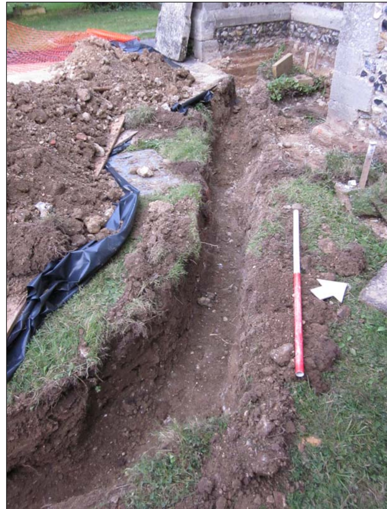
Plate 4. Sewer trench, at base of Tower, looking NW (1m scale)
