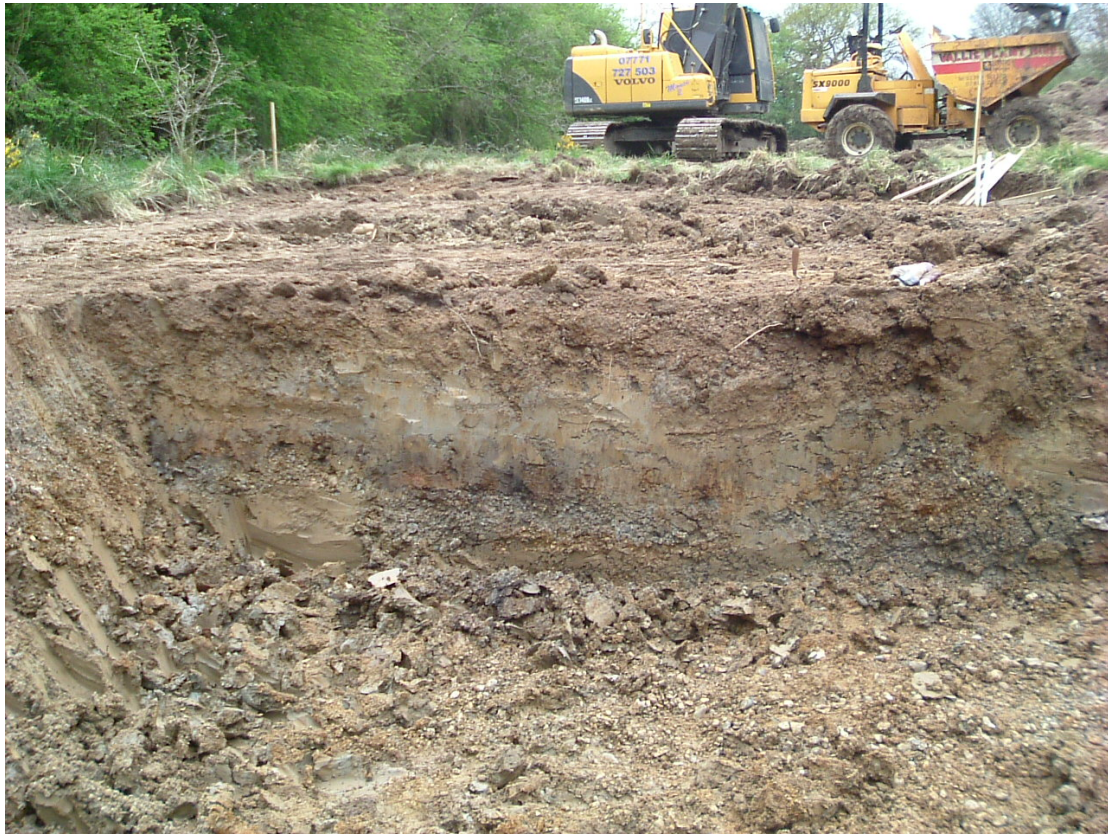
Plate 1: Tree throw revealed in exploratory trench – flood compensation area
