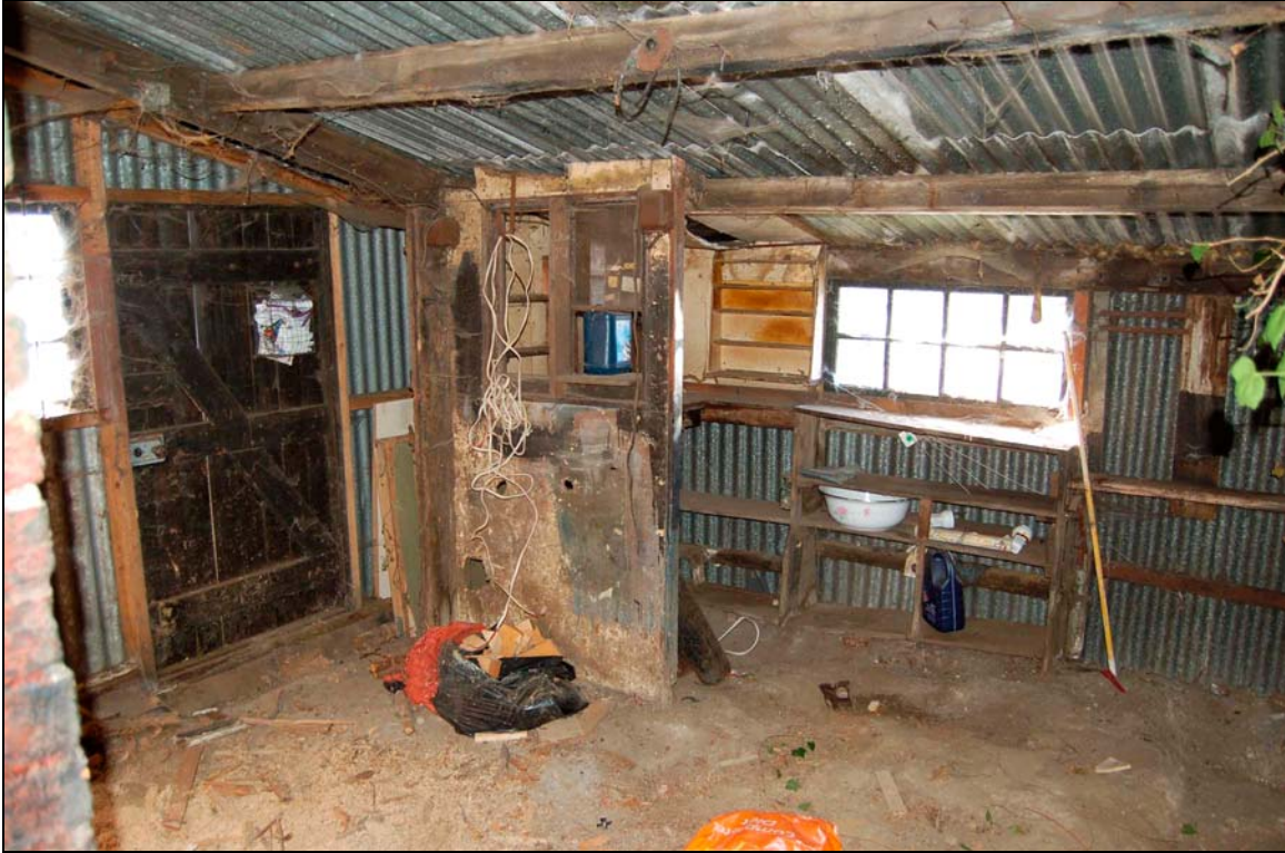
Plate 15 Office/storeroom interior viewed to east
