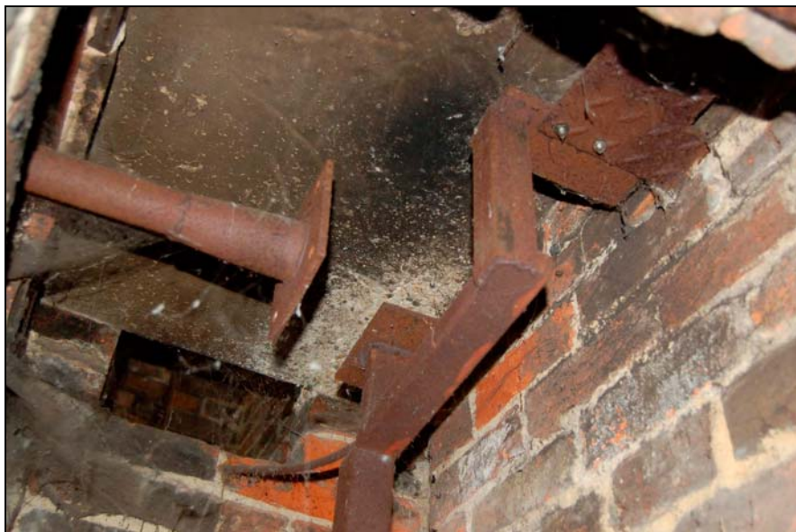
Plate 12 Cast iron tuyere and mountings
