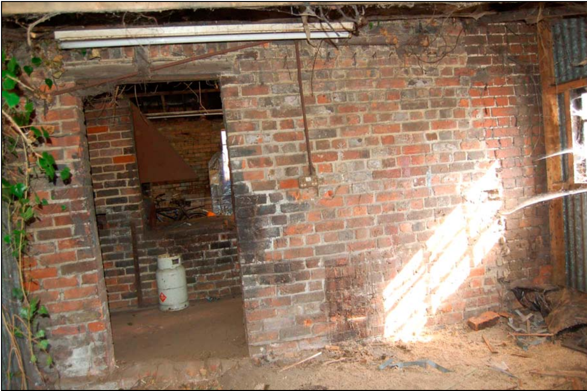
Plate 13 Blocked walling around doorway from office into forge
