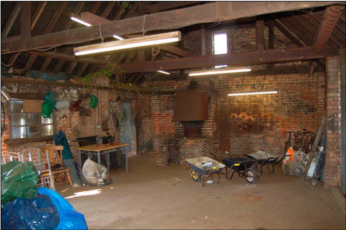
Plate 8 Interior of forge viewed to south-west
