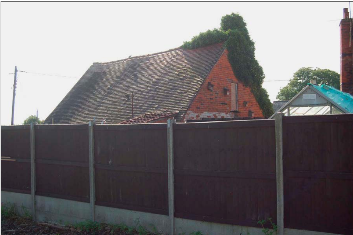
Plate 6 Forge viewed to east from behind neighbouring property
