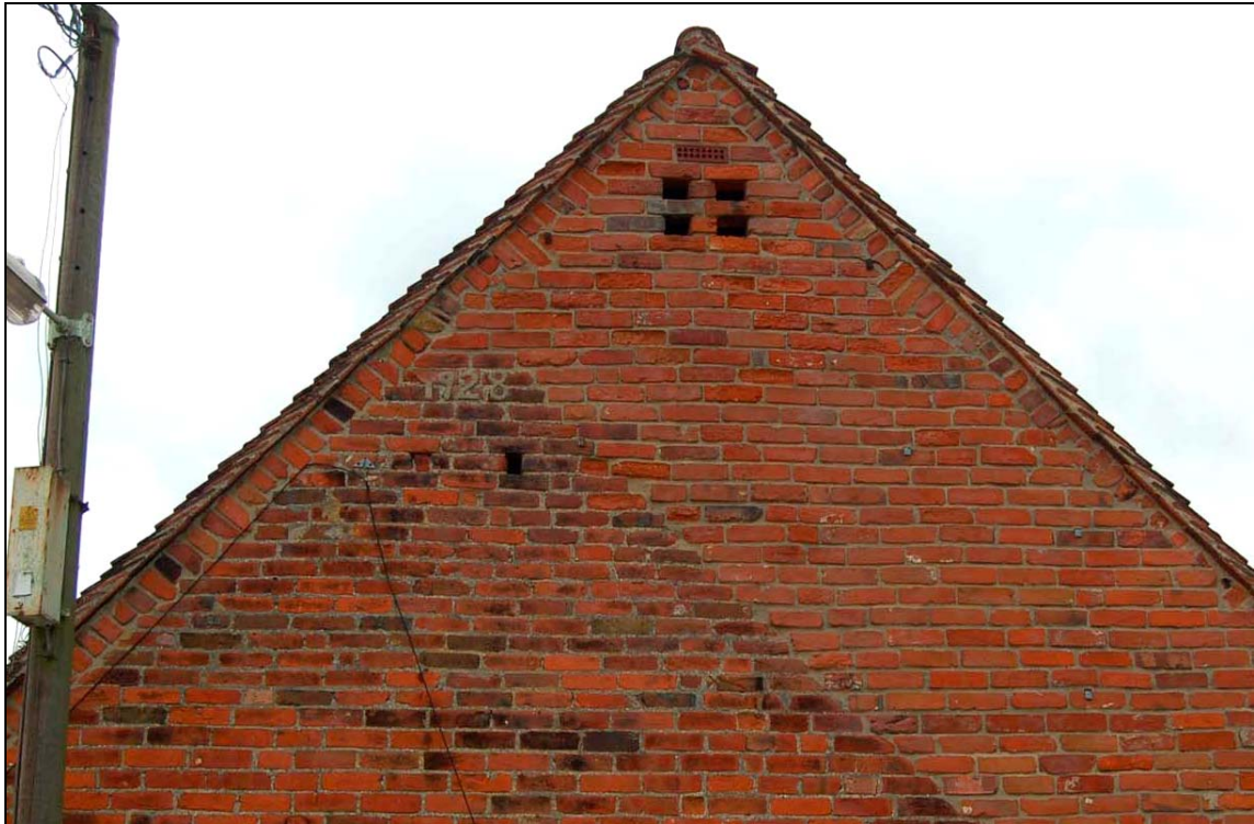
Plate 4 Outline of earlier roofline on north-east elevation
