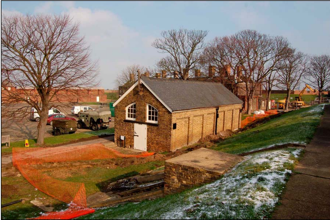
Plate 1 Pipe trench viewed from south-west end
