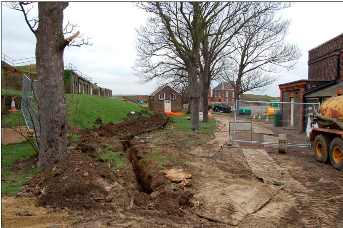
Plate 2 Pipe trench viewed from north-east end
