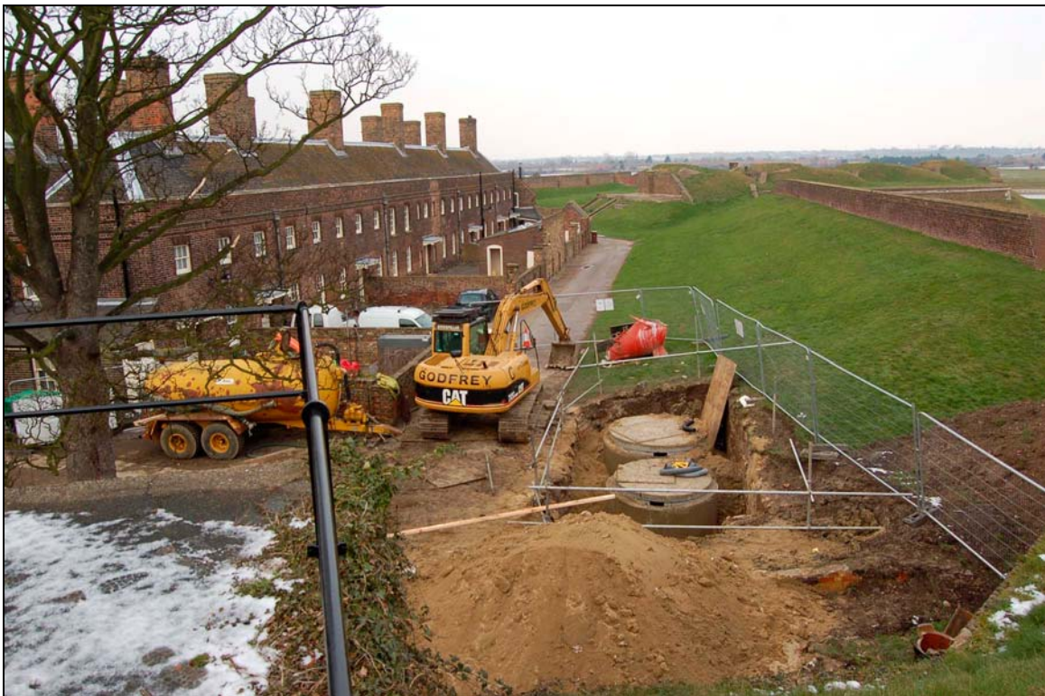
Plate 6 Excavated area for new tank viewed to north
