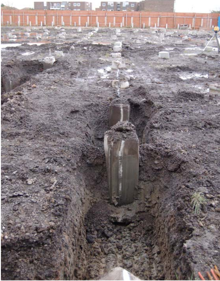
Plate 3 General shot, looking north
