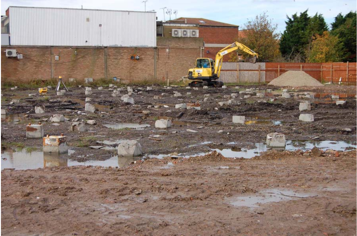
Plate 1 Development site, looking west, following the insertion of the piles
