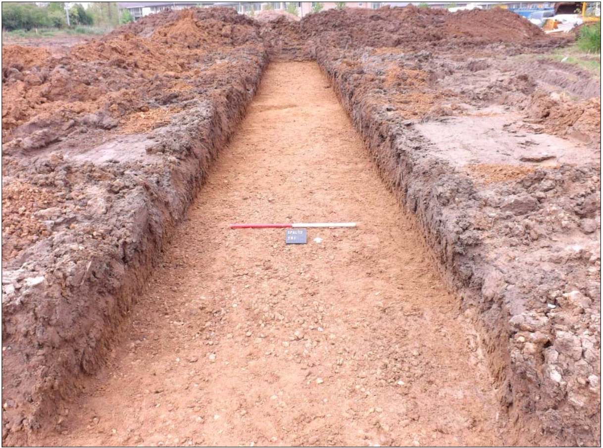
Plate 1. Trial trench 1, looking north (1m scale)
