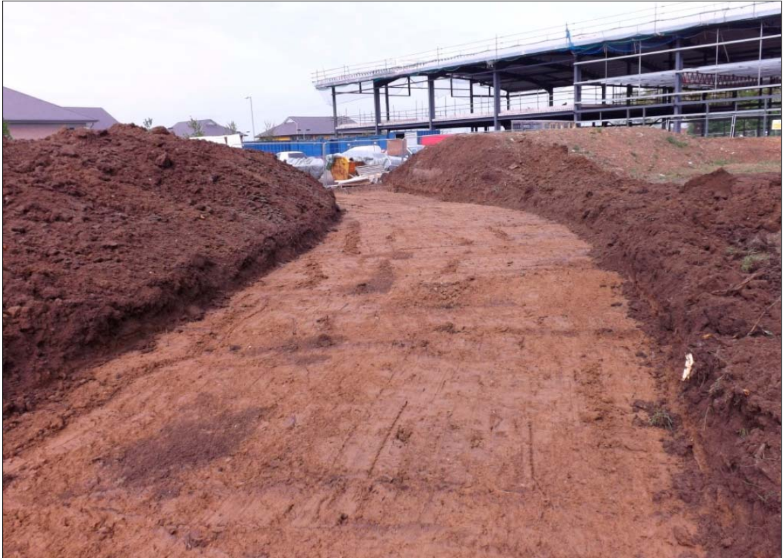
Plate 3. Access road strip, looking NE toward Plot K
