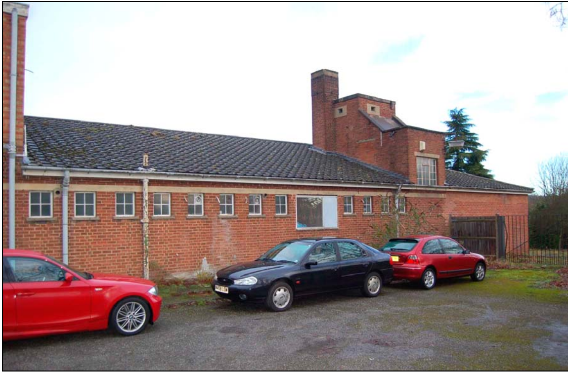
Plate 3 South elevation with pillbox
