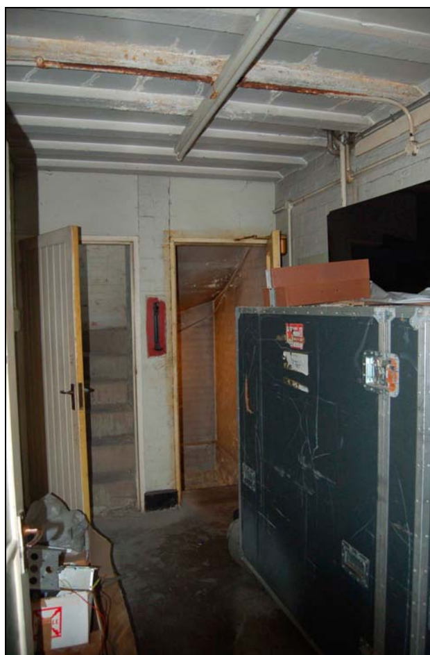
Plate 10 Ground floor viewed to south
