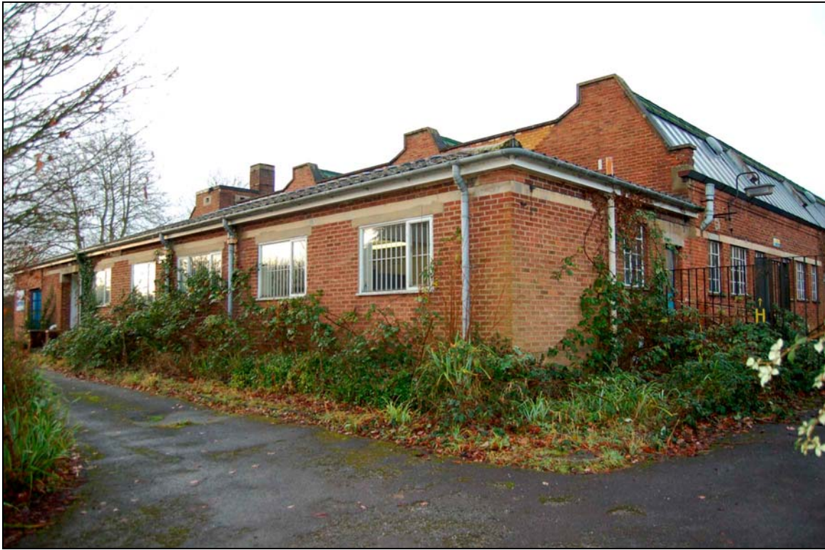
Plate 5 East and north elevations
