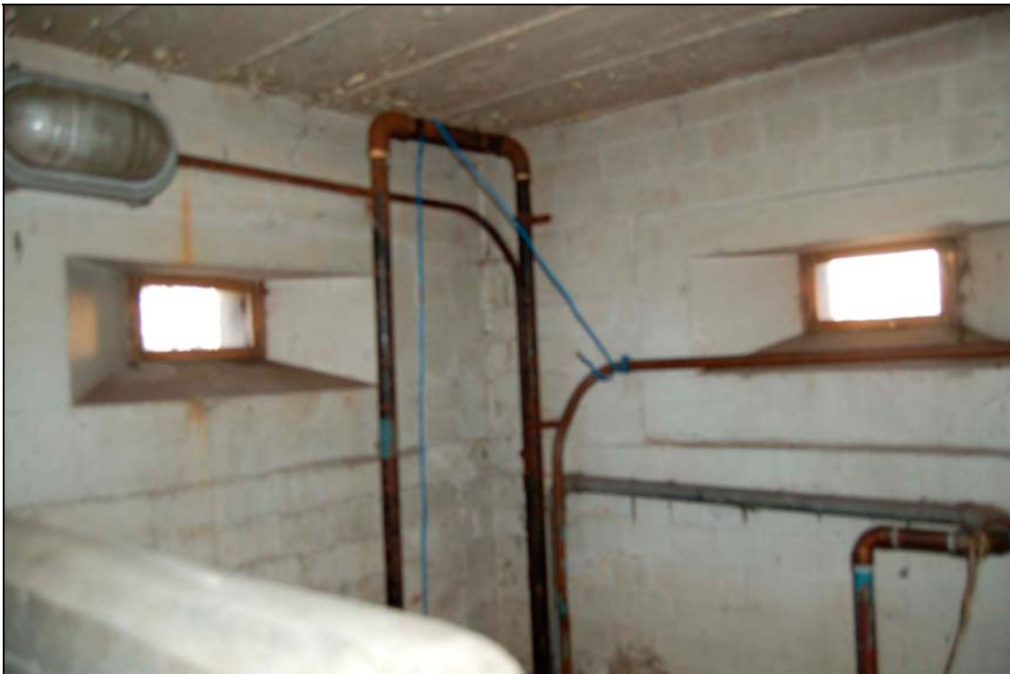
Plate 14 Second floor viewed to south-west
