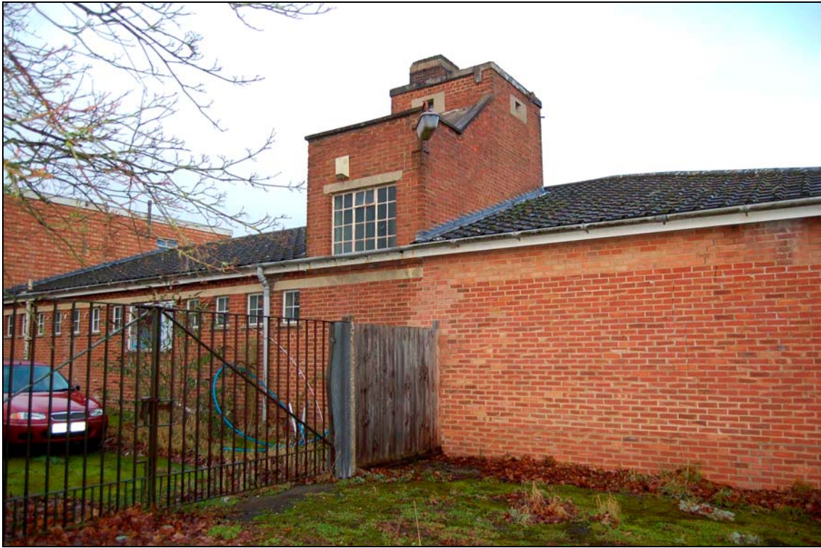
Plate 7 Detail of pillbox and south-east corner of factory
