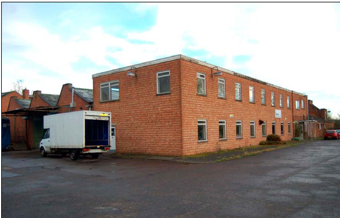
Plate 6 West and south elevations
