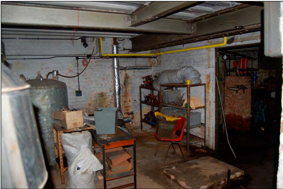
Plate 16 Basement viewed to north-east
