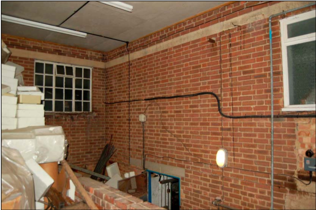
Plate 11 Original window and factory corner enclosed by boiler house extension
