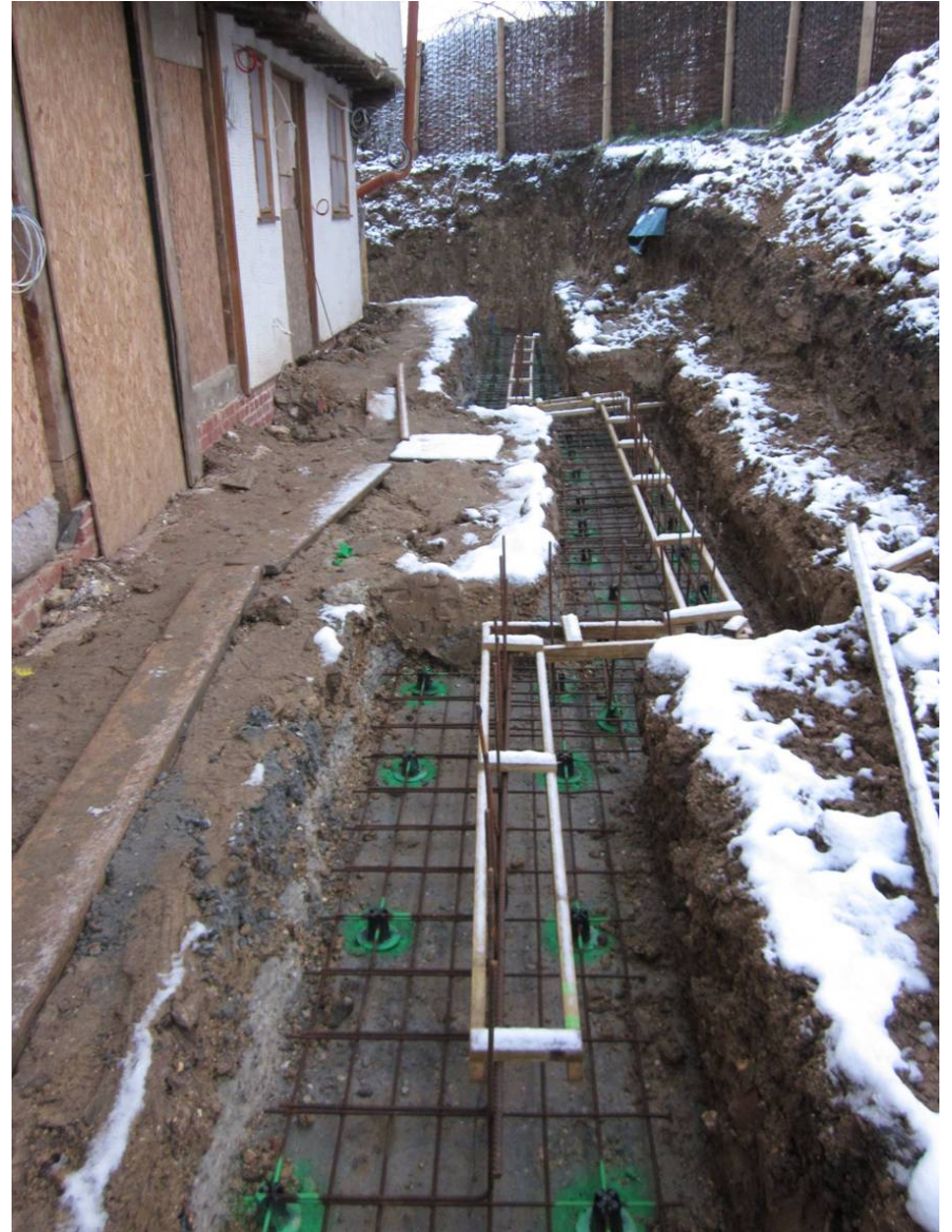
Plate 16. Foundations for new extension/walkway
