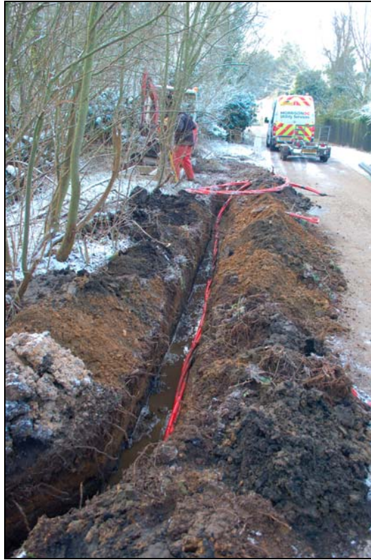
Plate 1: Cable trench 0 to 30m (S1), looking south
