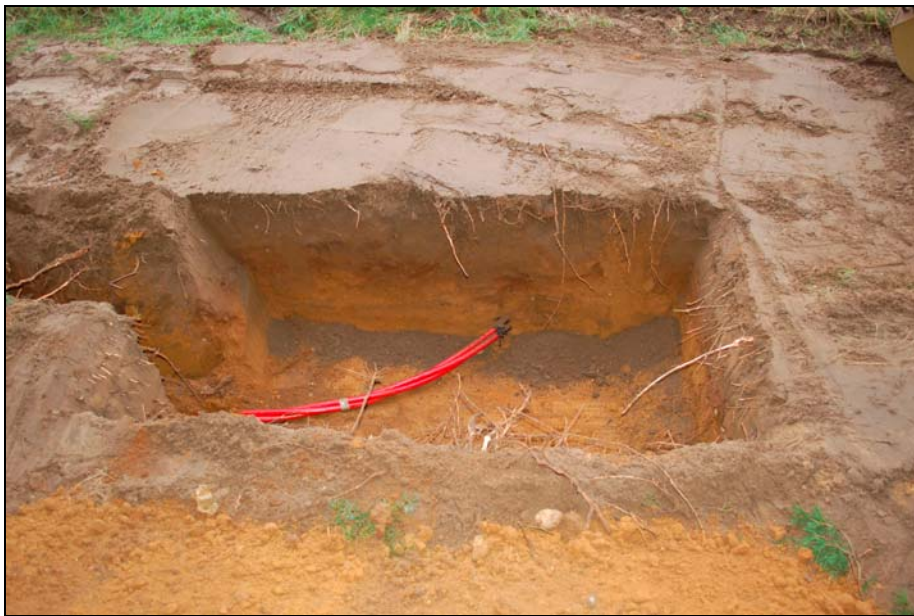
Plate 6: Cable connecting pit 7, looking north
