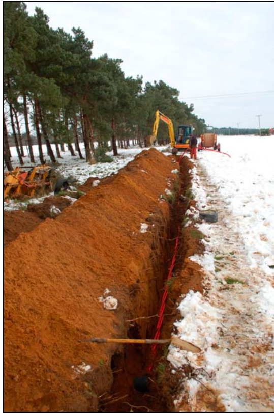
Plate 3: Cable trench 630 to 715m (S6), looking east
