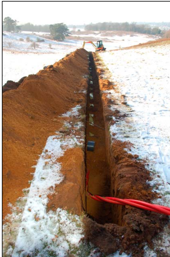
Plate 2: Cable trench 450 to 500m (S4), looking west
