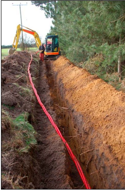
Plate 5: Cable trench 1350 to 1205m (S11), looking west
