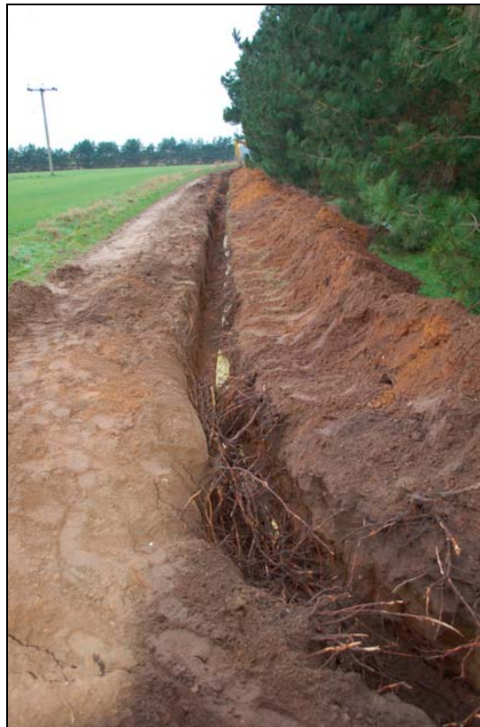
Plate 4: Cable trench 1350 to 1205m (S11), looking west
