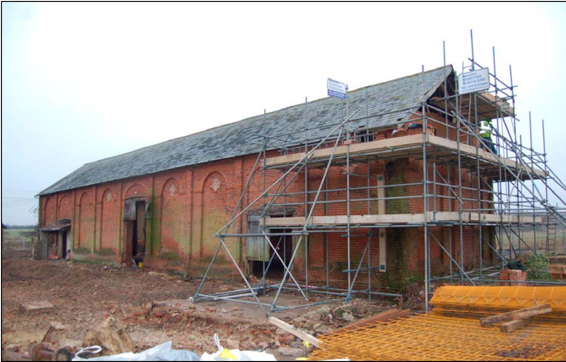
Plate 5 Barn viewed to north-east
