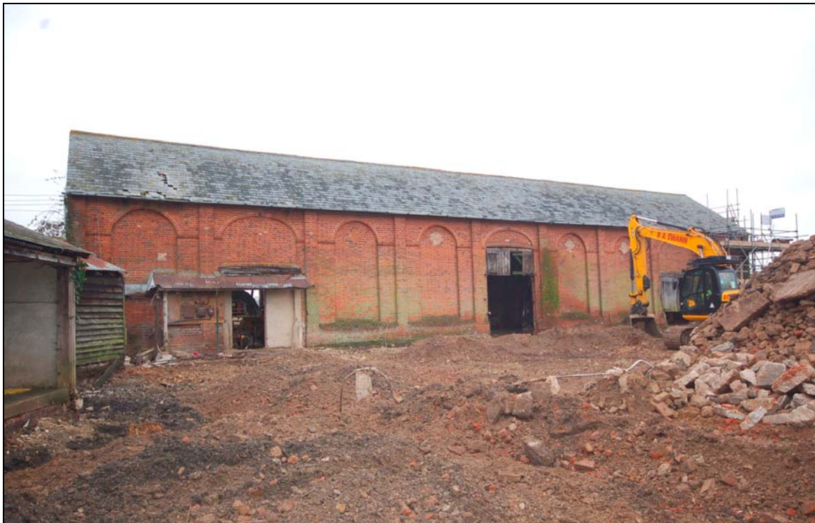
Plate 6 South elevation of barn
