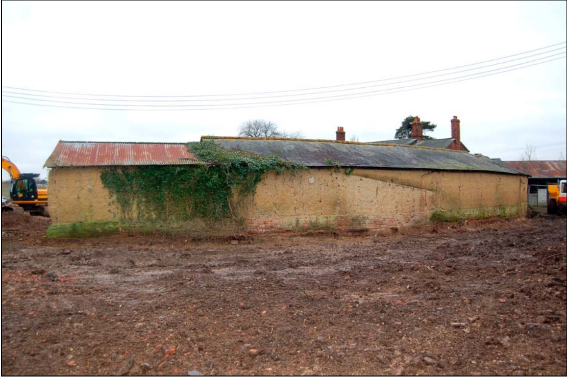
Plate 15 Rear of west range viewed to east
