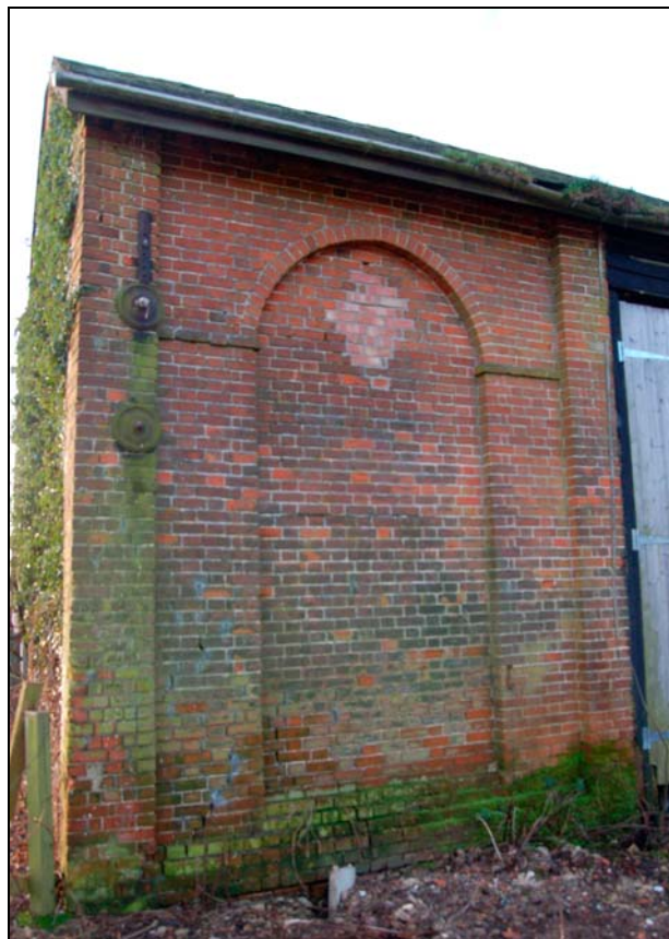
Plate 2 Pier and panel detail at east end of elevation
