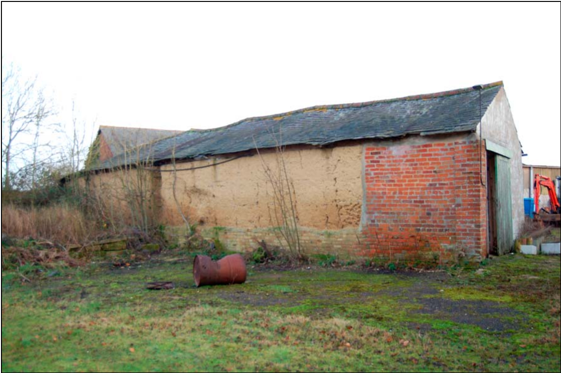
Plate 16 Rear of west range viewed to north-east
