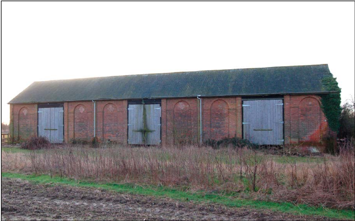
Plate 1 North elevation of barn
