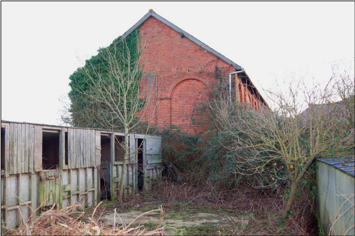
Plate 4 West elevation of barn (with modern stables)
