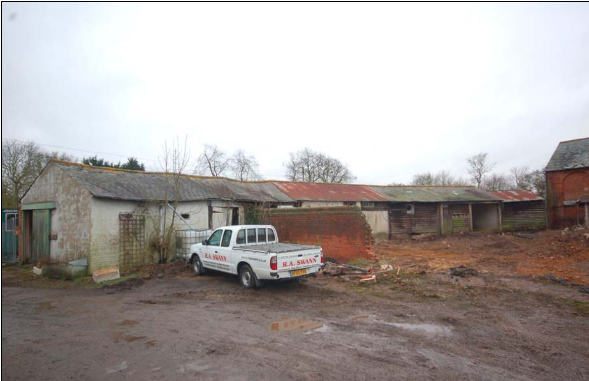
Plate 14 West range viewed to north-west from yard
