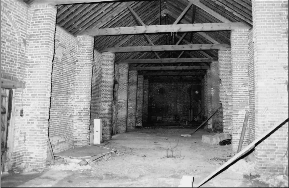
Plate 9 Barn interior viewed to west
