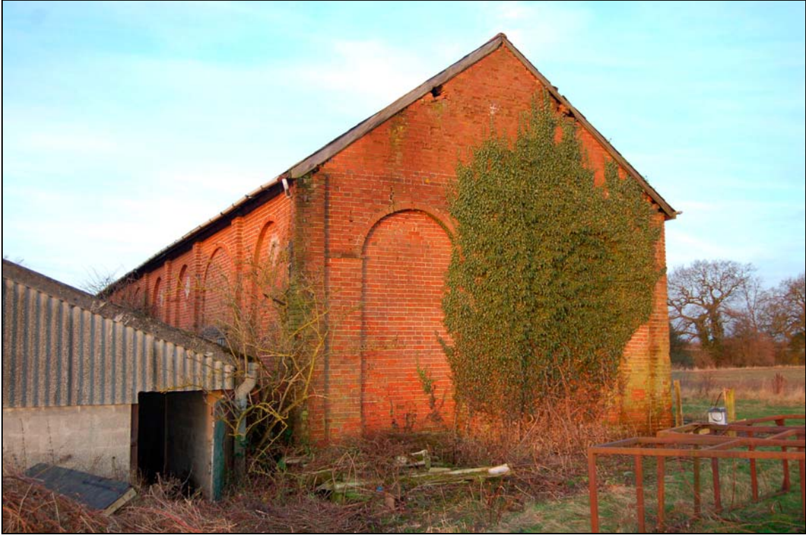
Plate 3 East elevation of barn (with modern cow shed)
