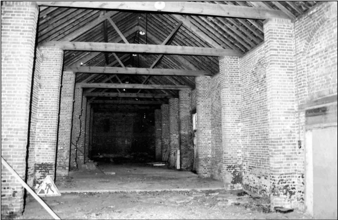
Plate 10 Barn interior viewed to east
