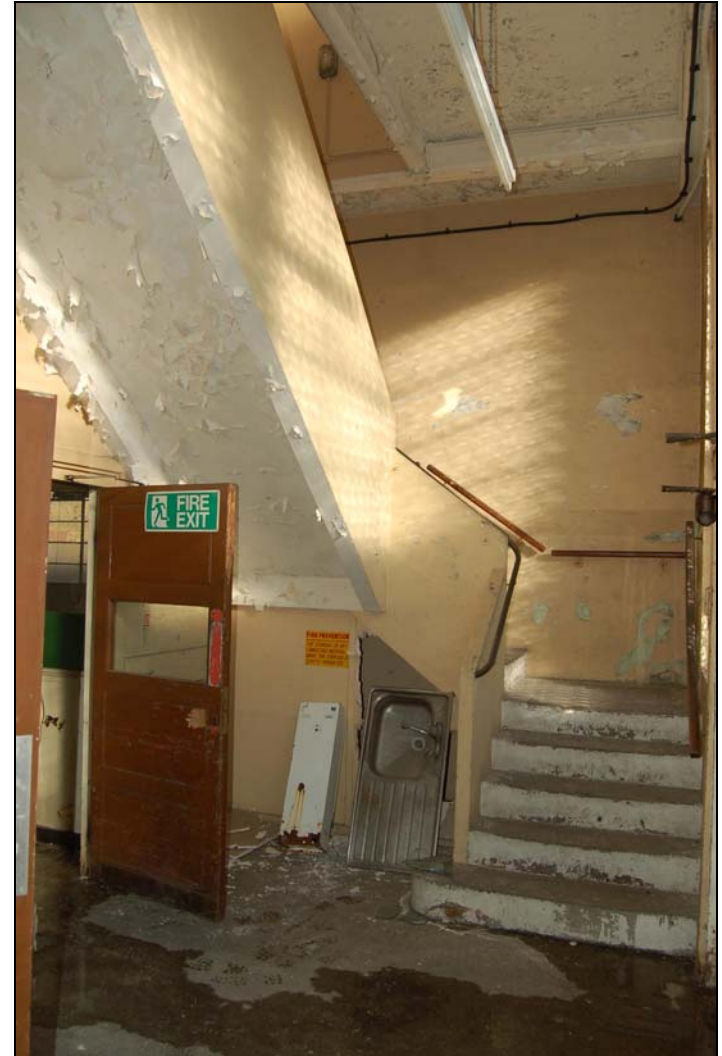
Plate 70 West tower stair
