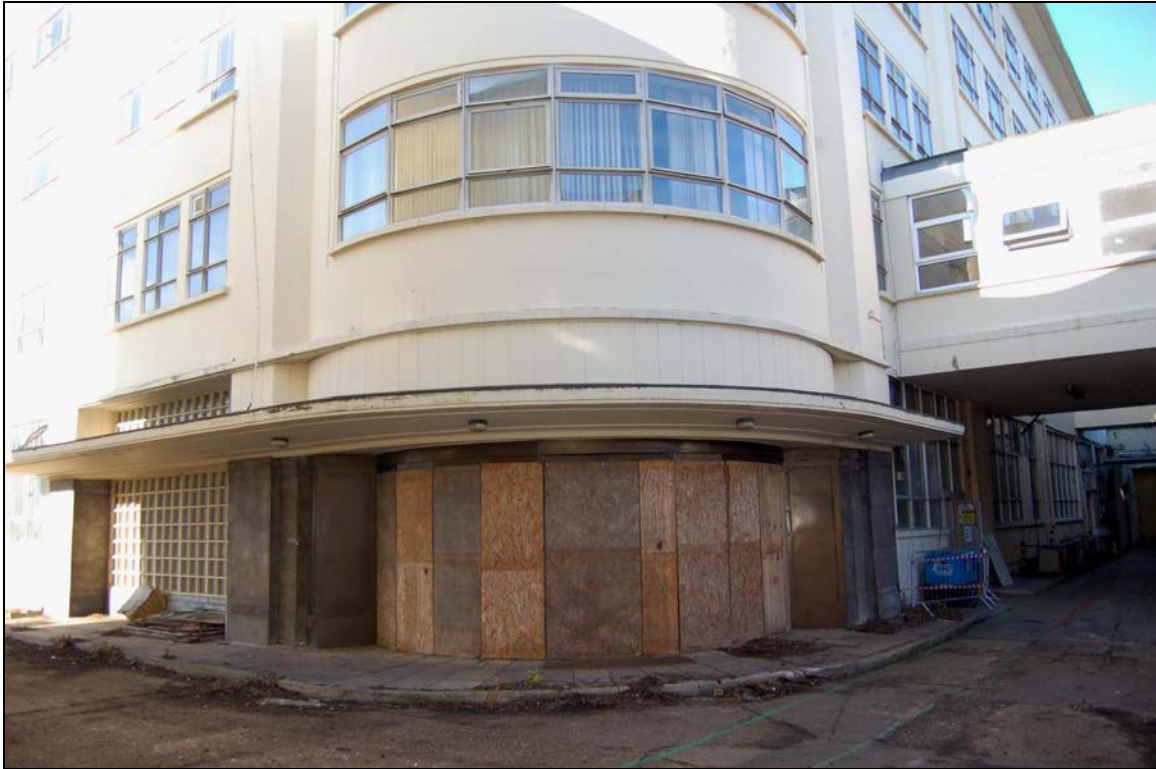
Plate 81 Rotunda base, with boarded entrance lobby
