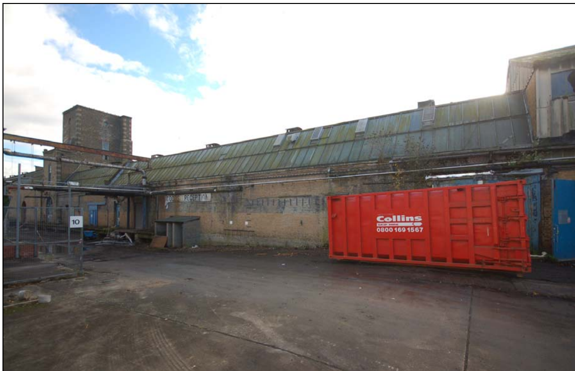
Plate 42 North elevation of 1912 factory (west end)
