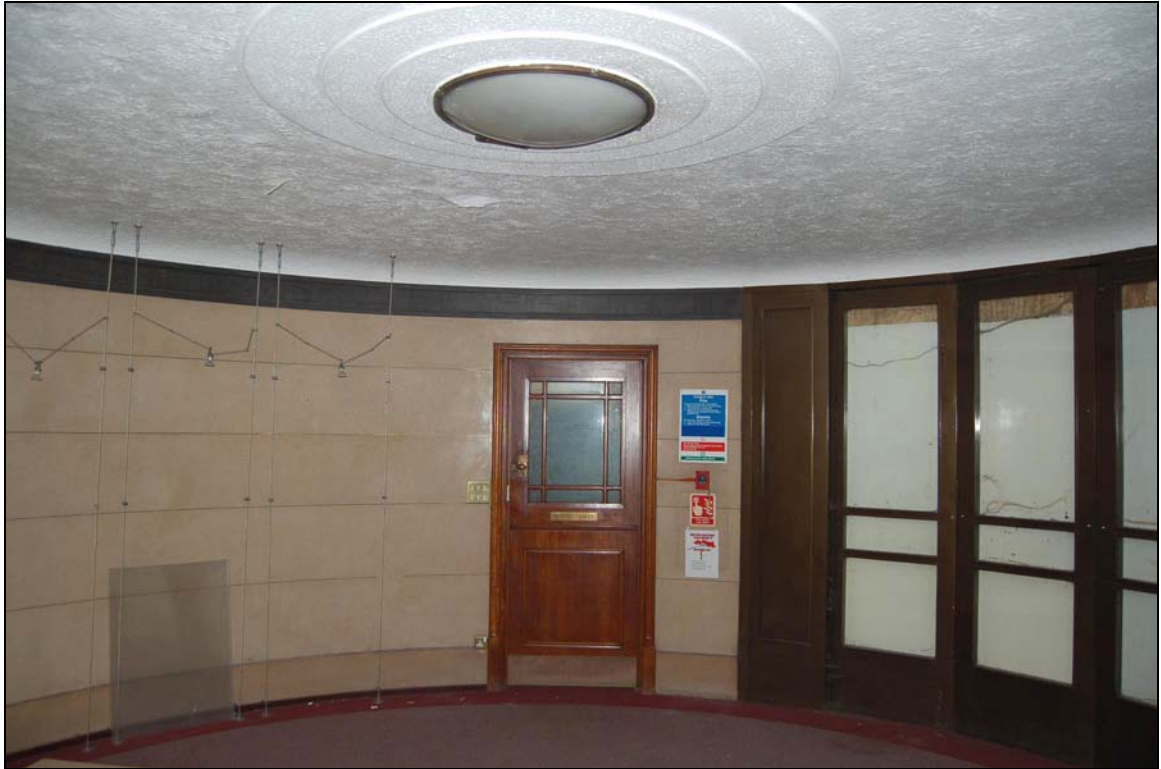
Plate 85 Entrance lobby 1 viewed to north-east
