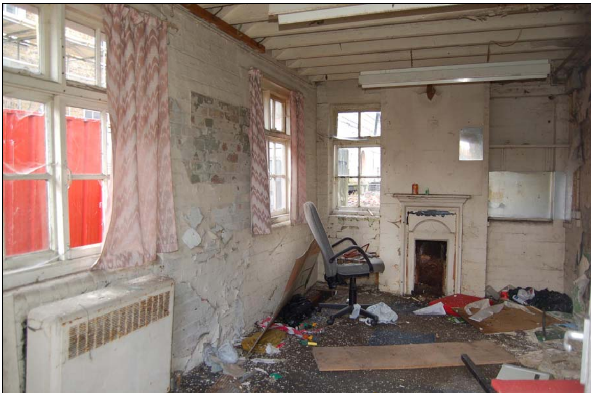
Plate 144 Interior of weigh house
