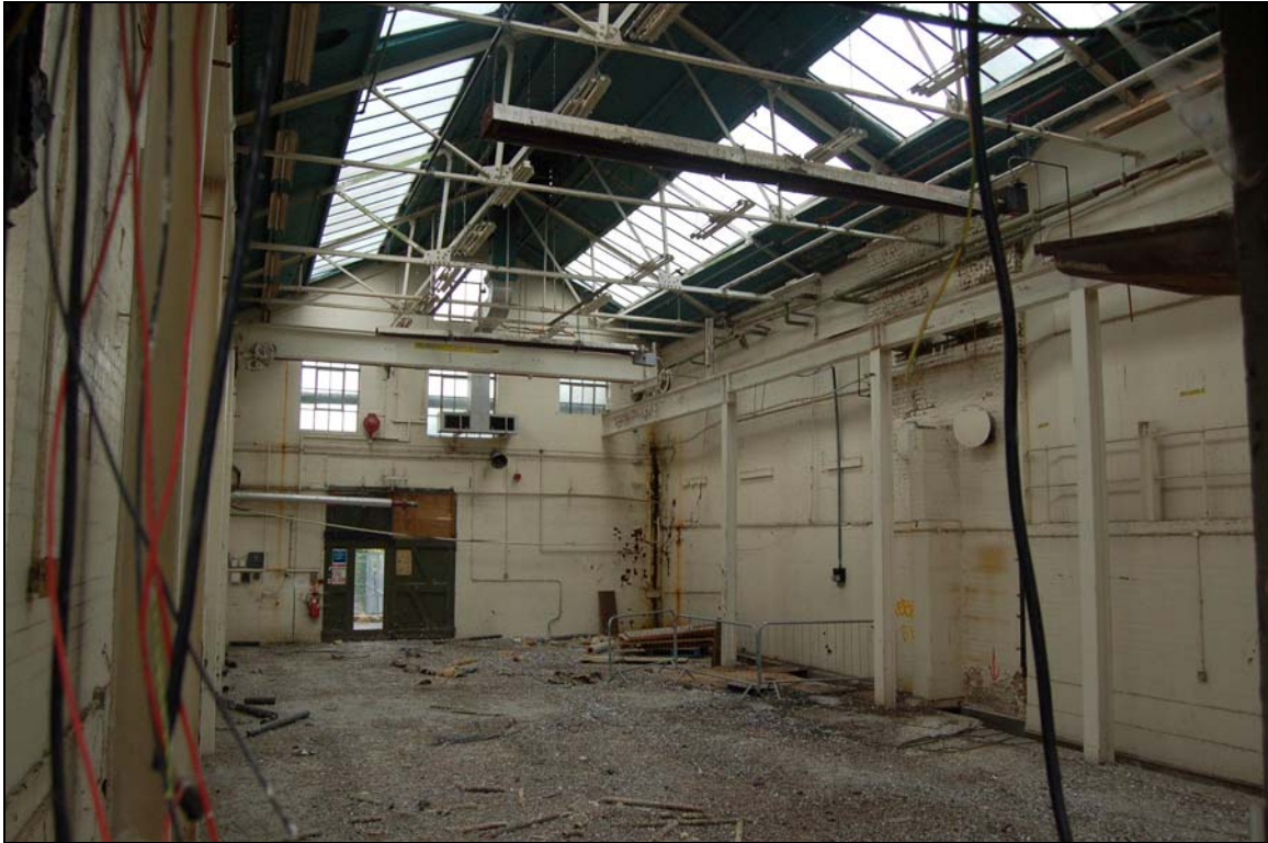
Plate 131 Generator room viewed to west
