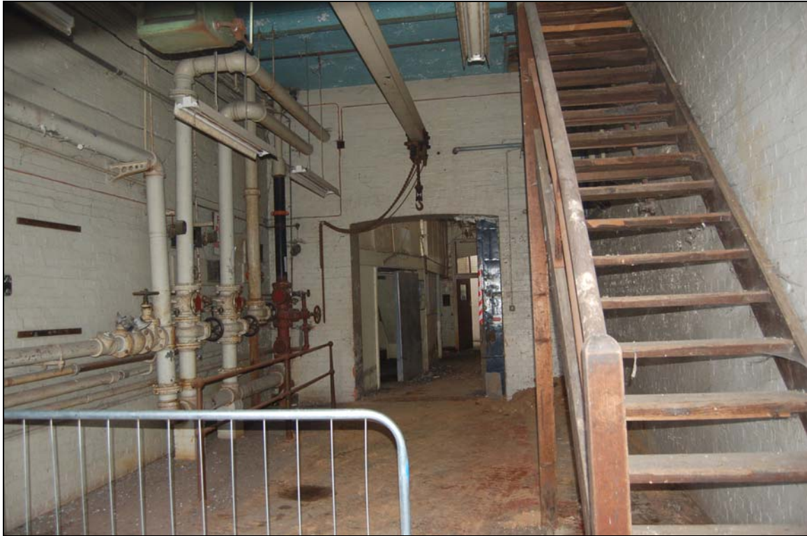
Plate 53 Interior of water tower (ground floor) looking into factory
