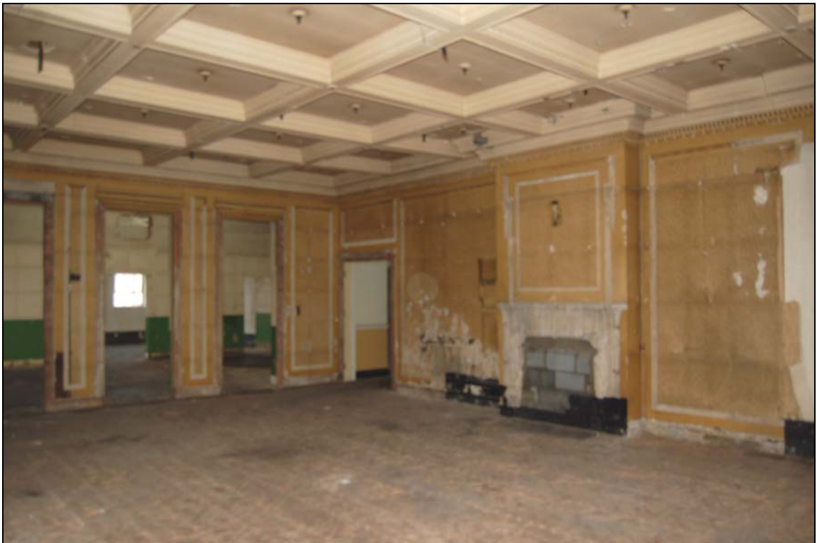
Plate 26 Dining room 10 after stripping-out
