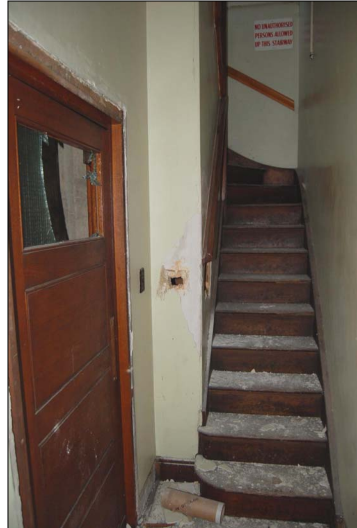
Plate 76 Stairs to second floor above manager's office 2
