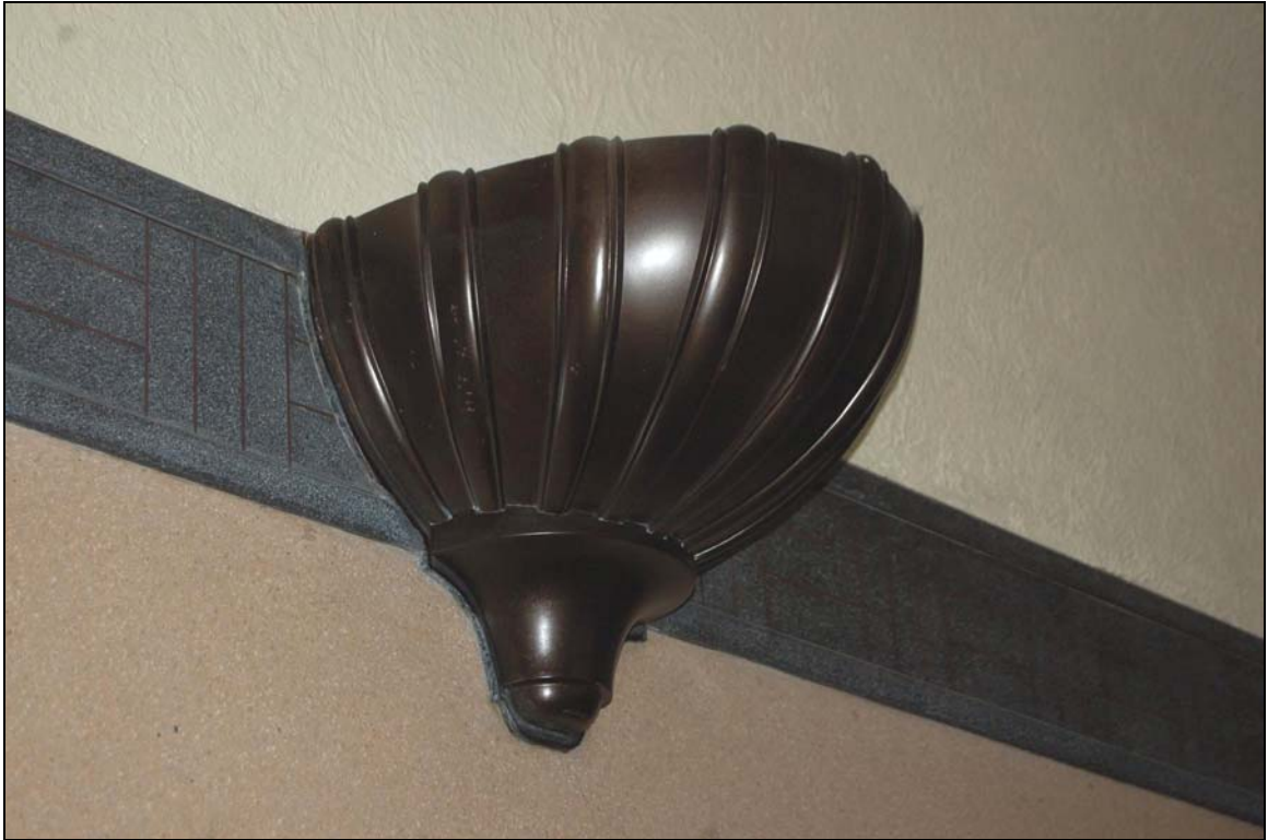
Plate 89 Steel up-light above lift
