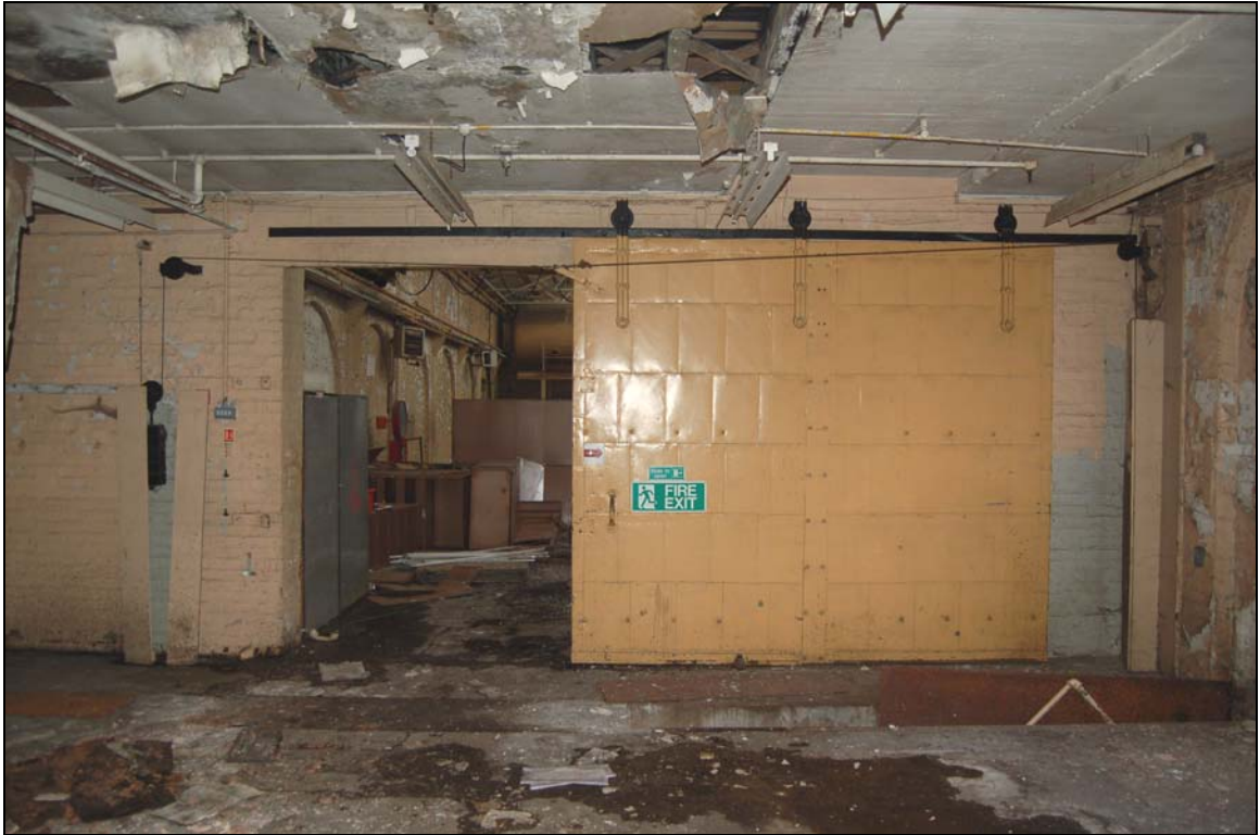
Plate 49 Typical factory sliding door
