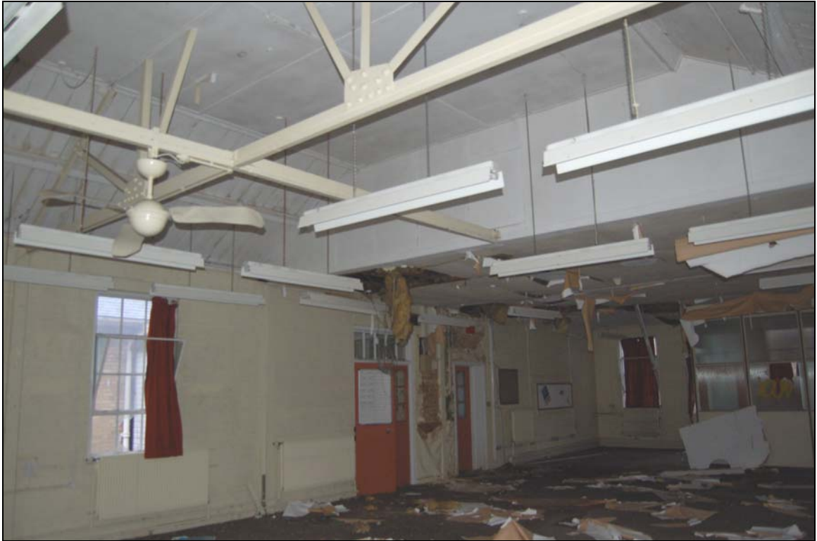
Plate 39 Room 13 in 1929 extension
