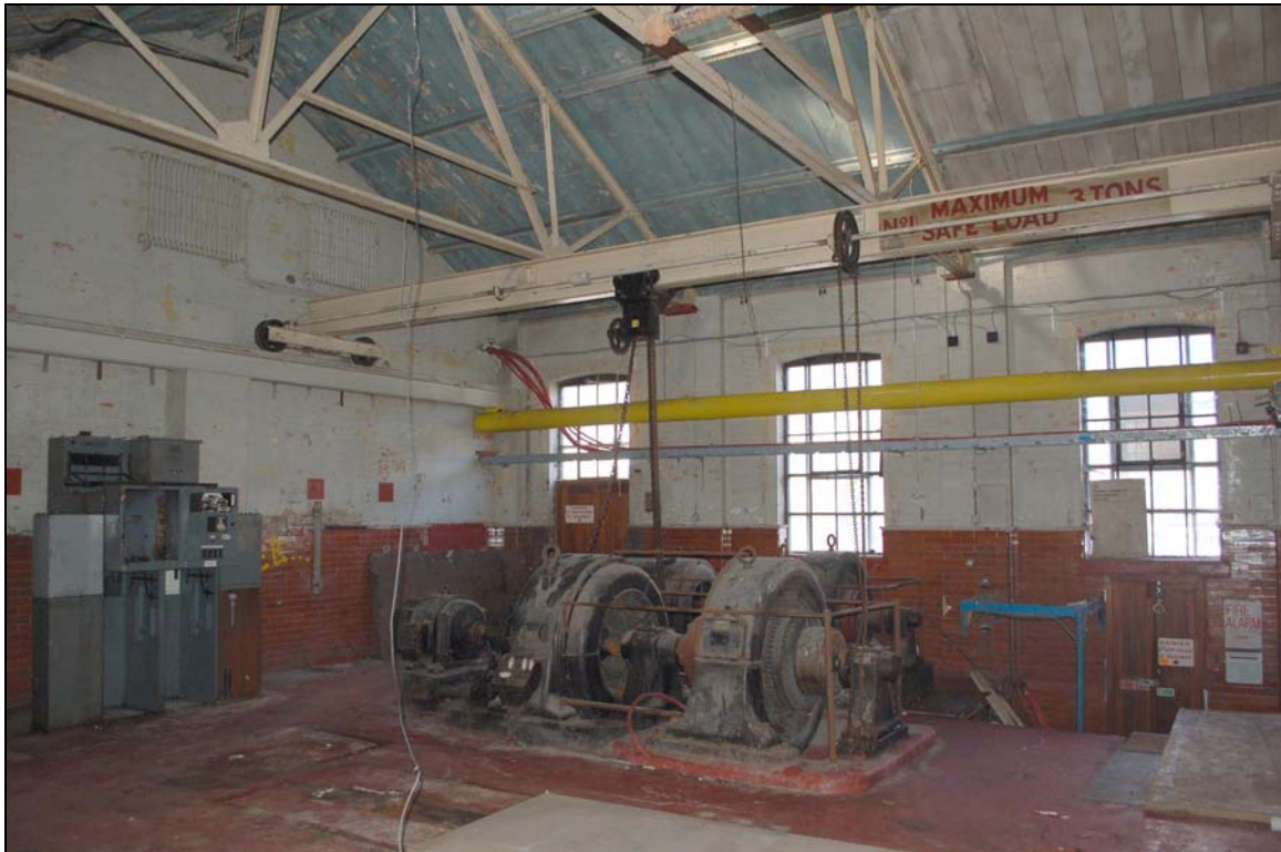
Plate 129 Turbine room viewed to north-west
