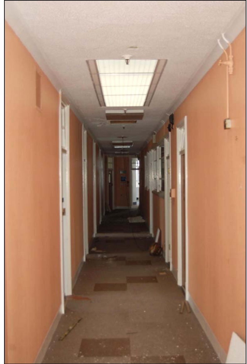
Plate 96 Corridor 2 (fourth floor)
