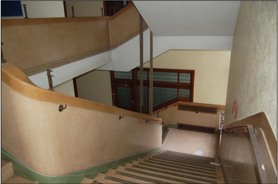
Plate 91 Art Deco stair and metal vents on half-landing
