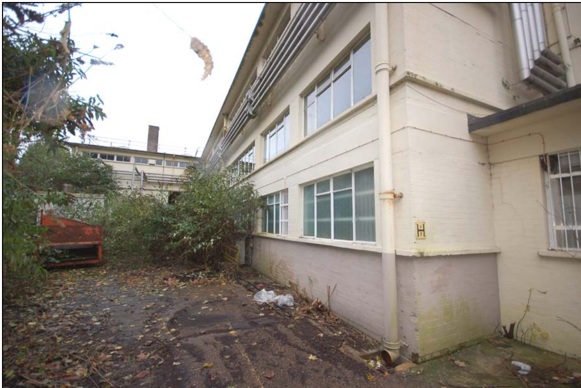
Plate 112 Rear of Building 720 viewed to north-west
