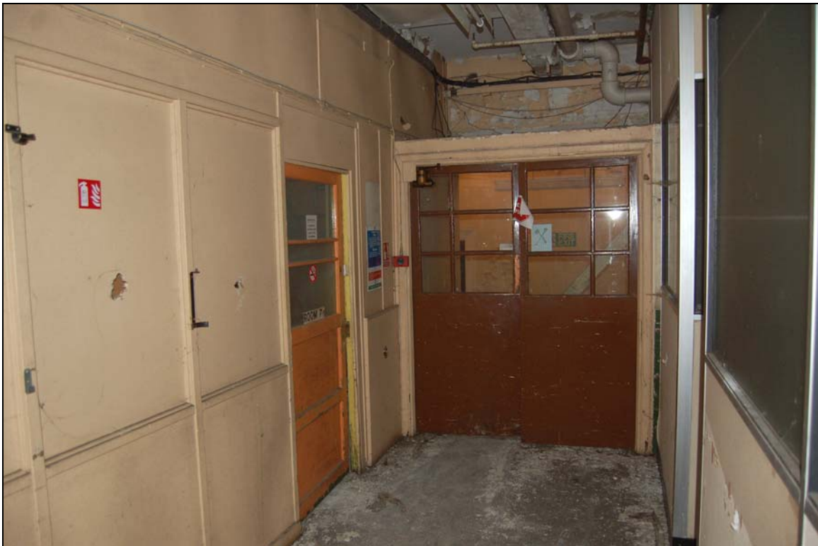
Plate 16 Inserted corridor between offices and 1912 factory
