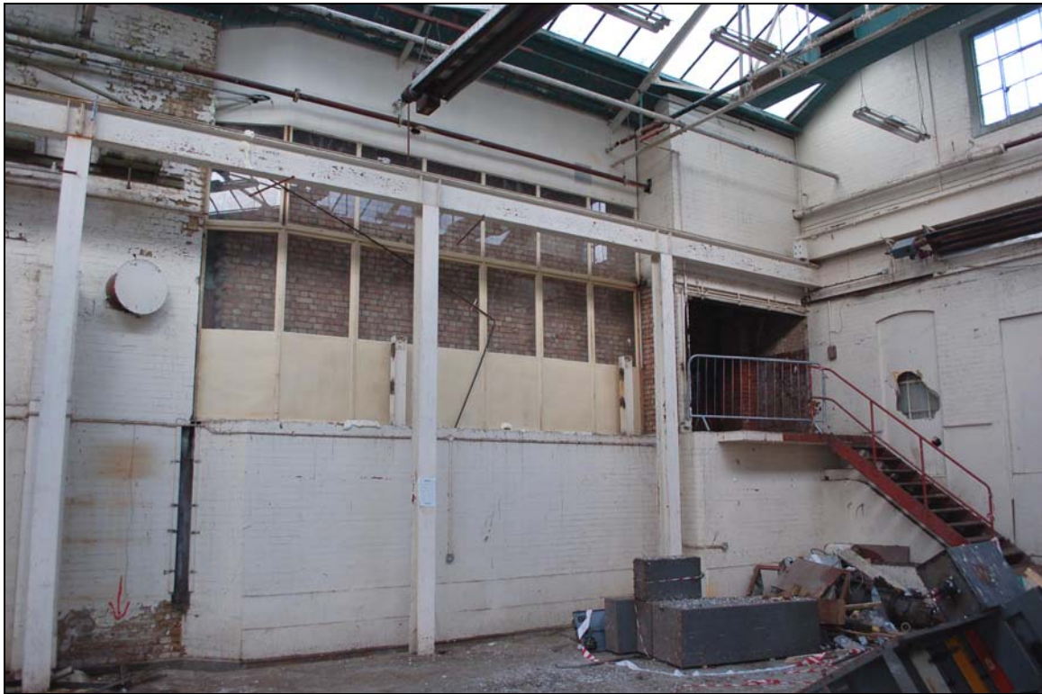
Plate 133 Former turbine room viewing bay
