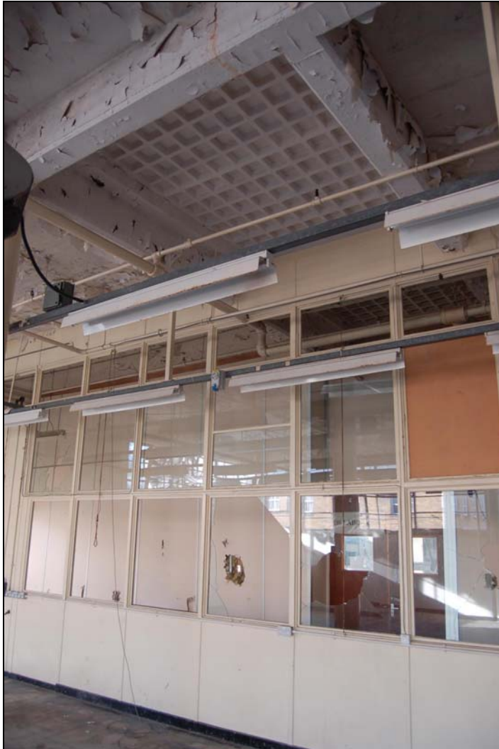
Plate 69 hard-boarded partition to room 4
