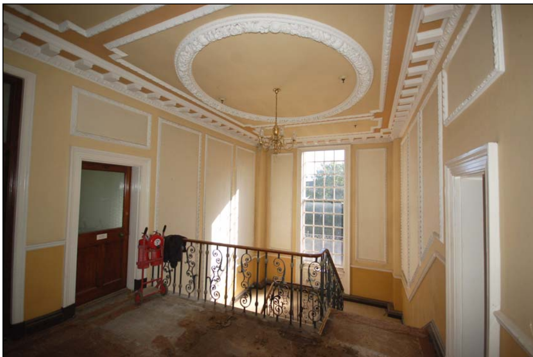
Plate 20 First floor landing viewed to east
