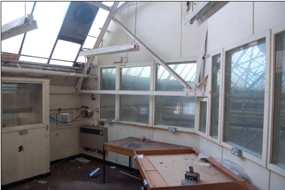
Plate 60 First floor office 21, with view over factory floor
