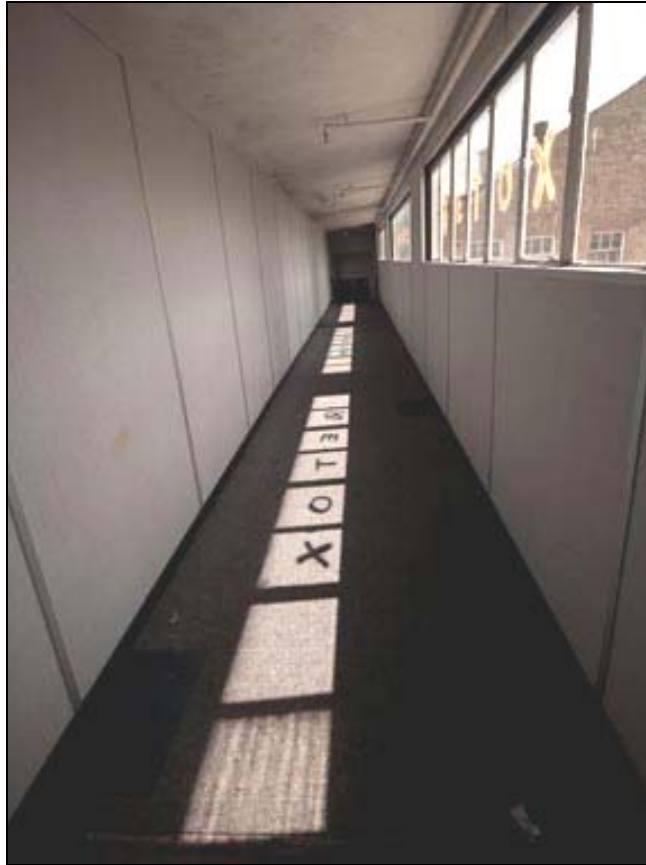
Plate 71 Corridor between 1912 offices and 1937 factory
