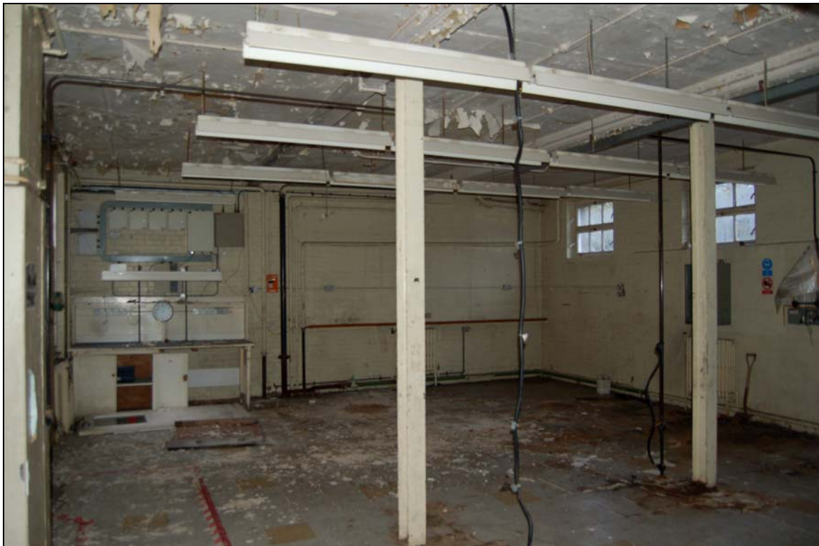
Plate 36 Interior of room 5, former mess room
