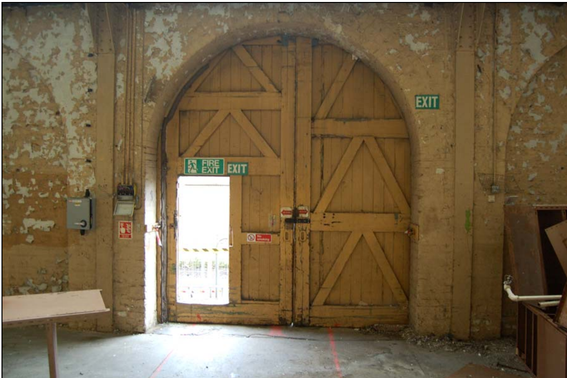
Plate 52 Typical factory loading door from railway siding
