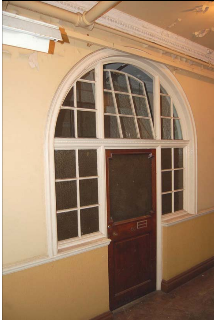
Plate 9 Typical office doorway
