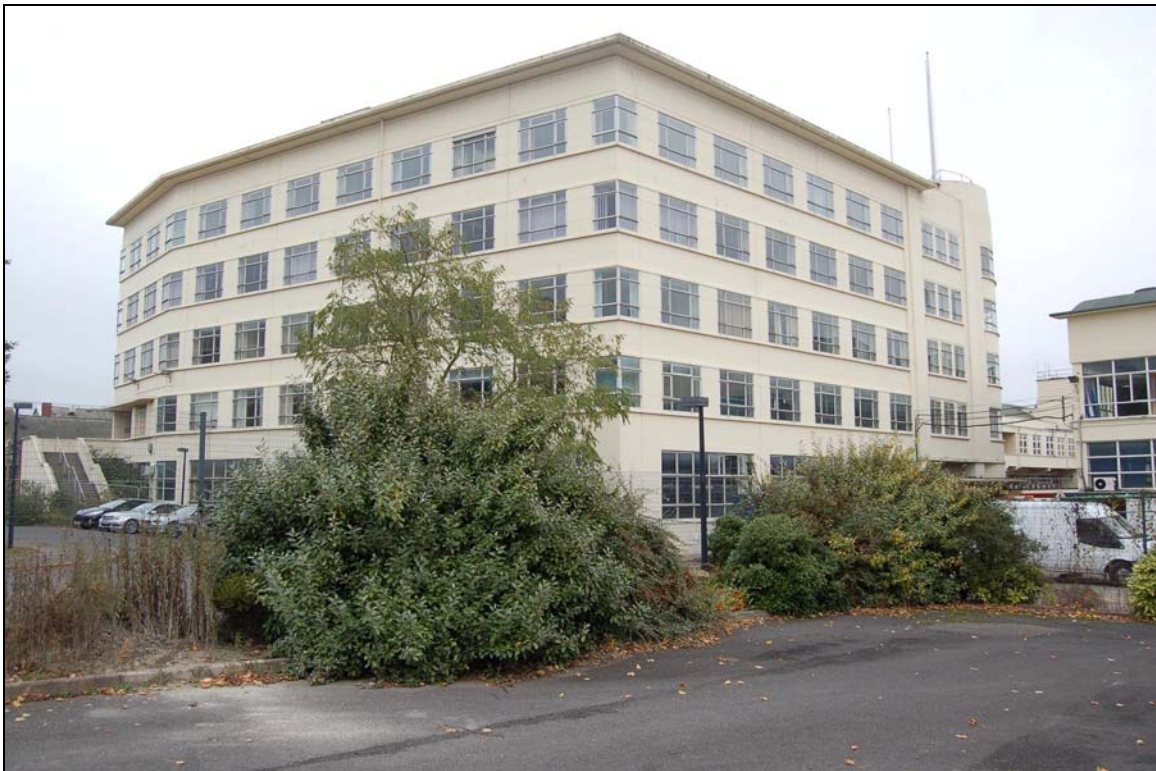
Plate 82 Marconi House viewed to north-east
