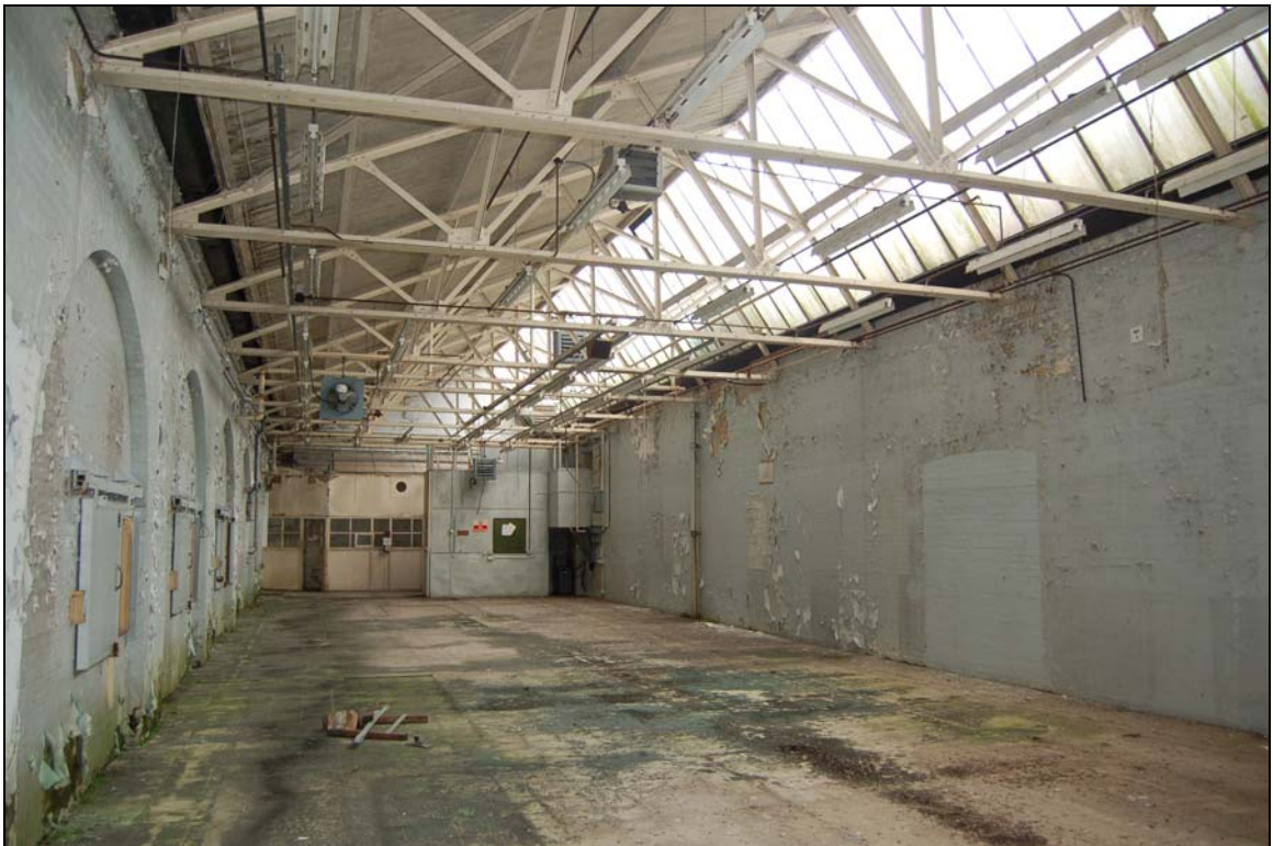
Plate 50 Room 4 (former 1912 finished stores) viewed to west
