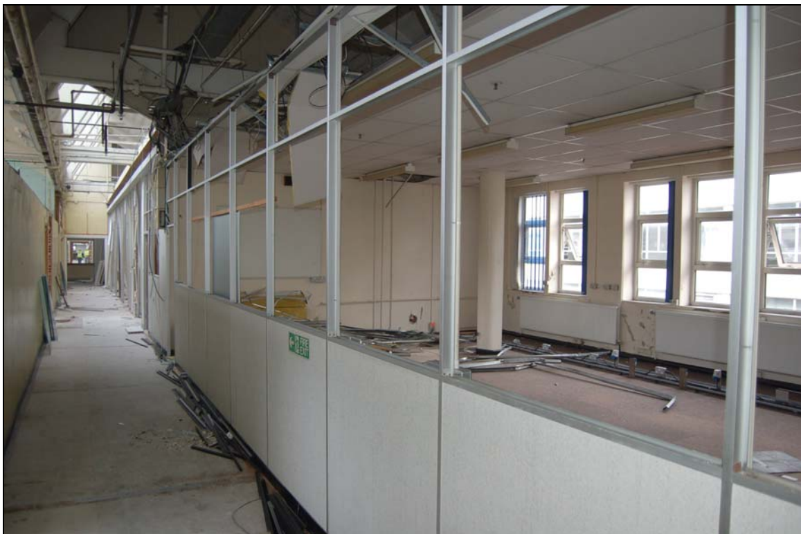
Plate 72 View along corridor 1 on first floor (from west)
