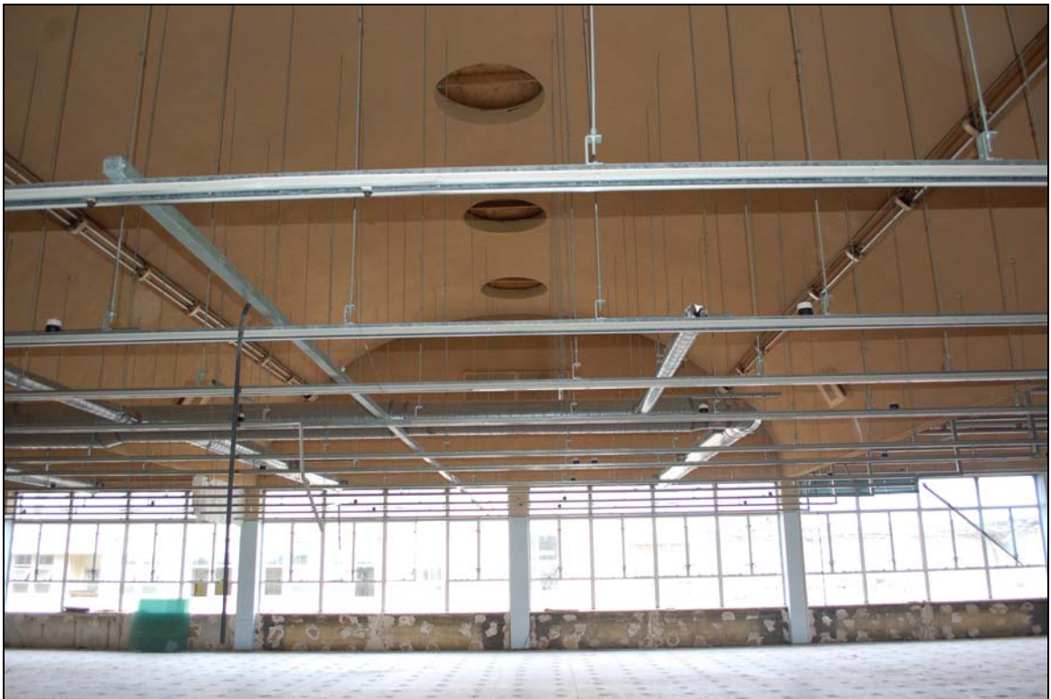
Plate 120 Exposed barrel-vaulted ceiling
