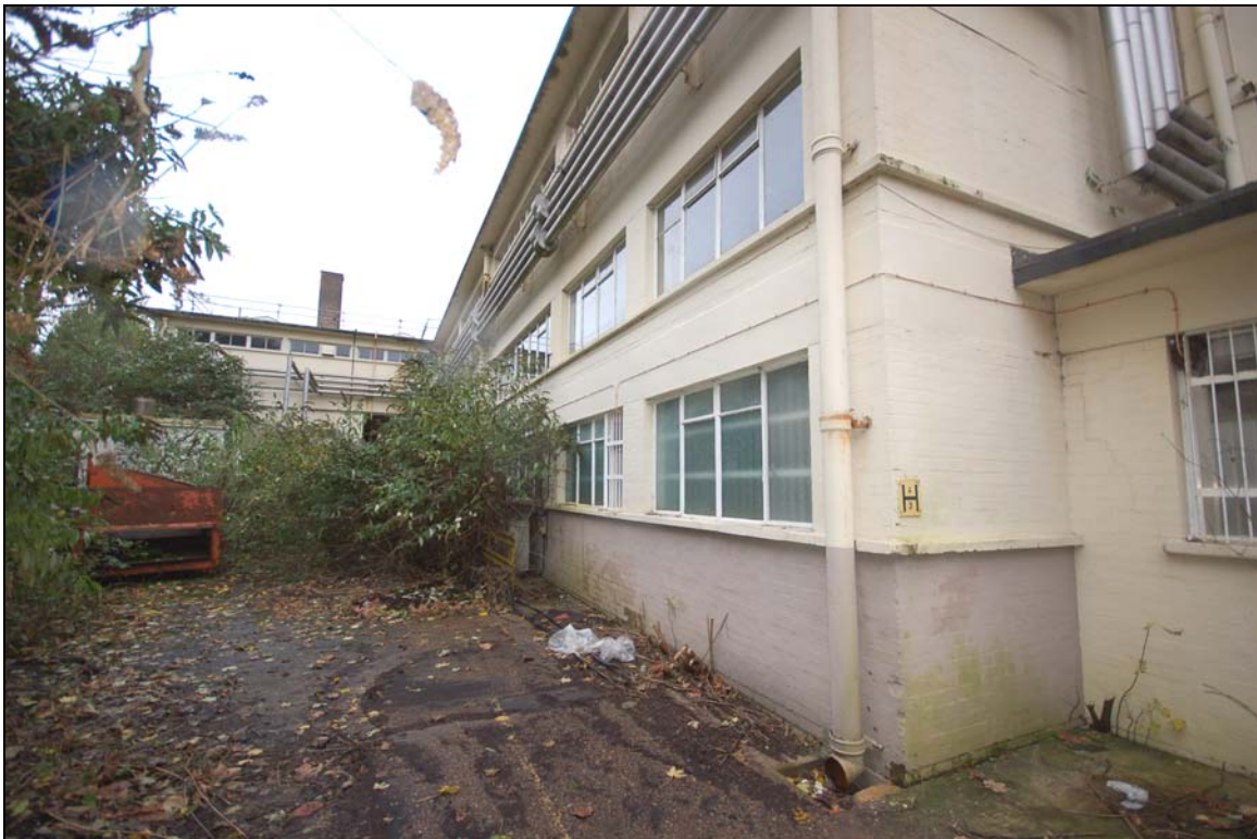
Plate 112 Rear of Building 720 viewed to north-west
