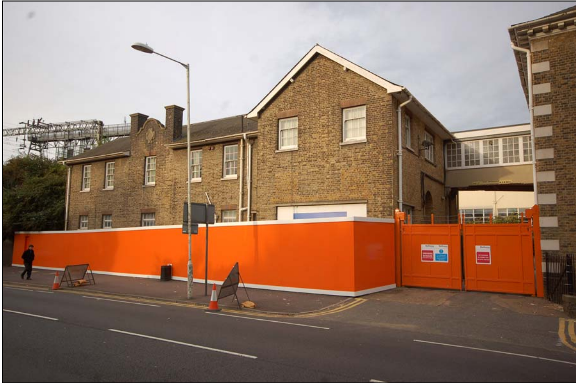
Plate 29 Gatekeeper's house and mess rooms viewed to west
