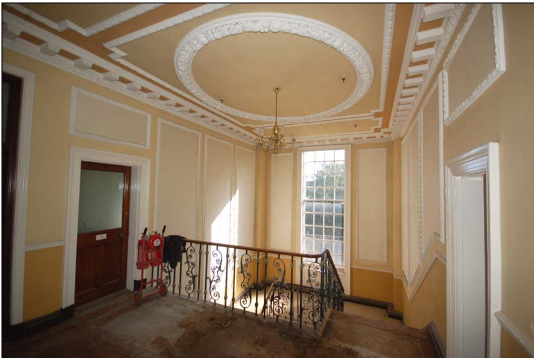
Plate 20 First floor landing viewed to east
