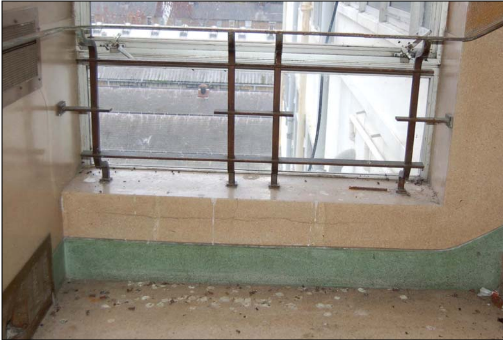
Plate 93 Remains of Geometric style window railing
