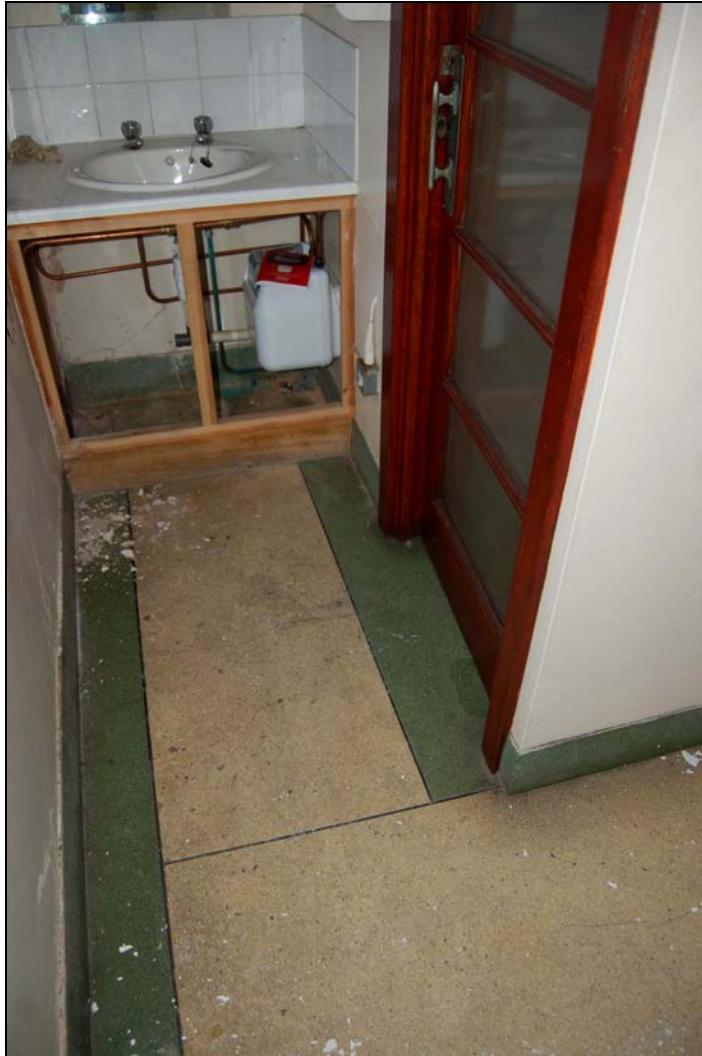
Plate 75 Lavatory beside first floor stair landing
