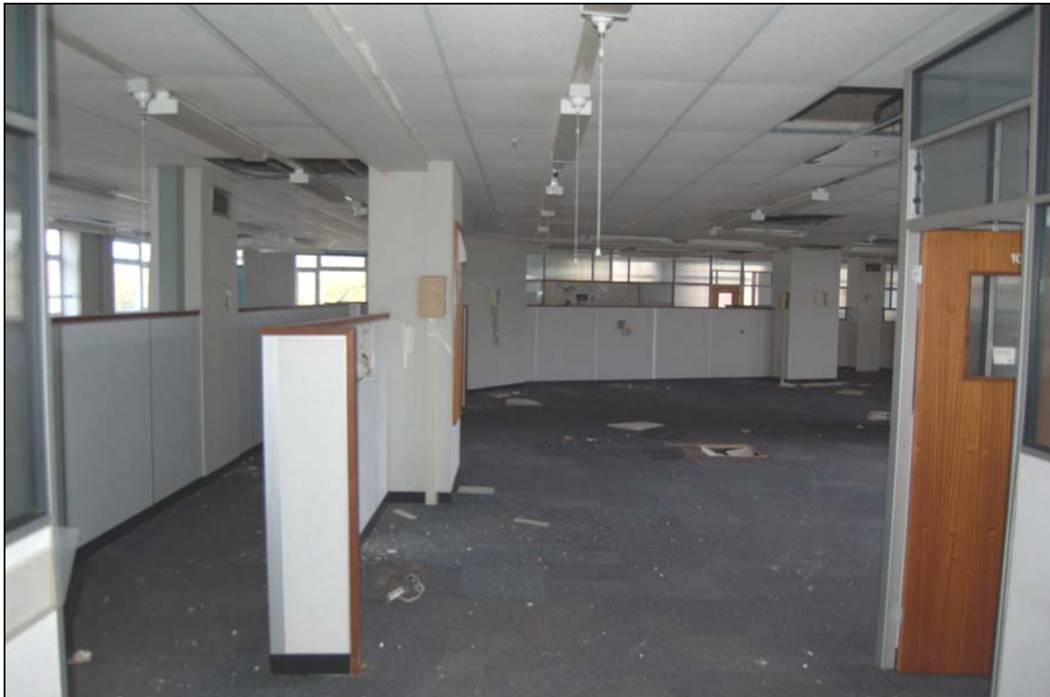
Plate 103 First floor modern office space (rooms 3 & 8)
