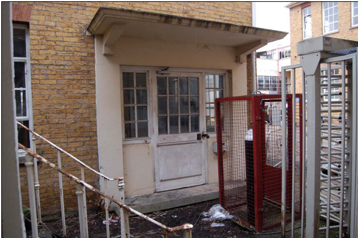
Plate 34 Entrance into 1929 extension beside modern turnstile
