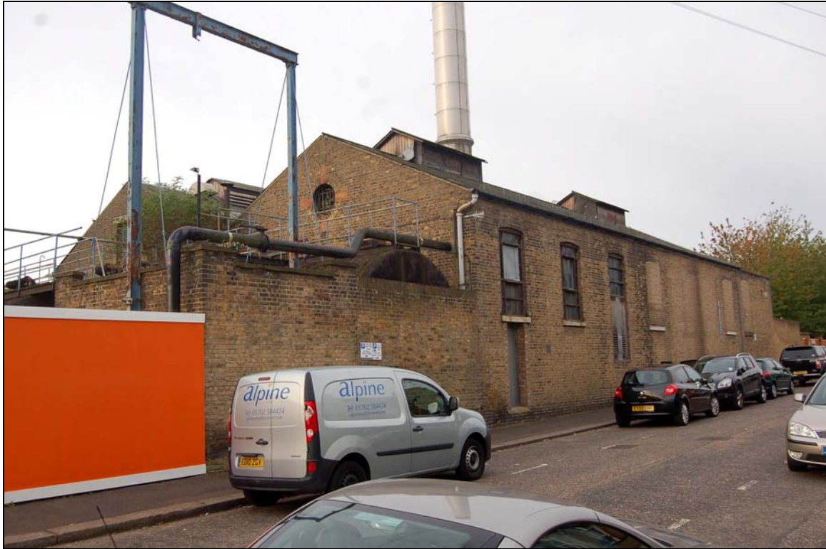
Plate 125 Power house viewed to south-west
