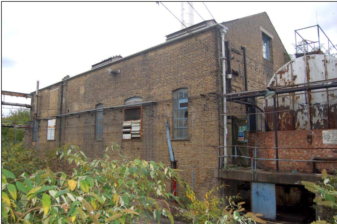
Plate 126 Power house viewed to north-west
