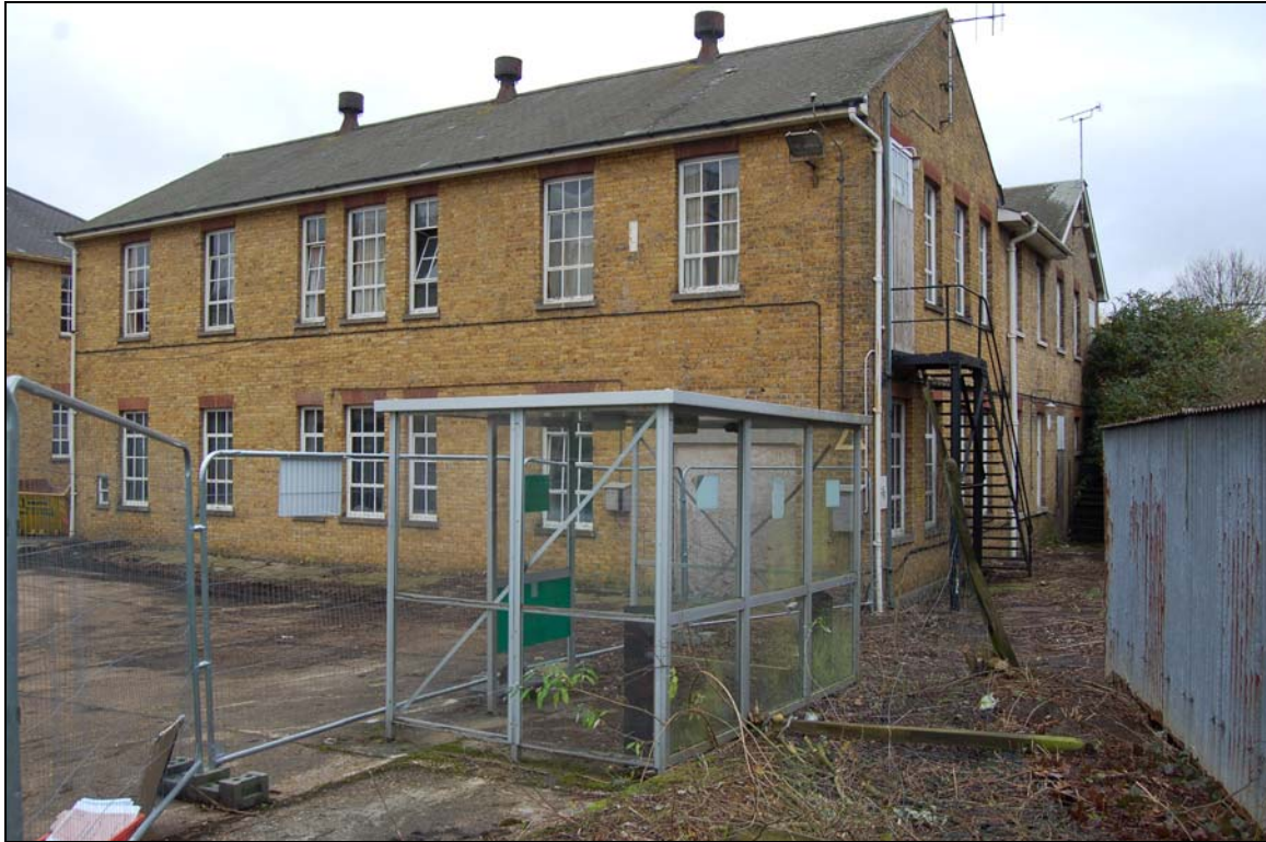
Plate 33 Mess rooms viewed to north-east
