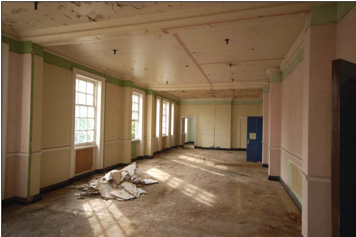
Plate 22 Room 4 after stripping-out, viewed to south
