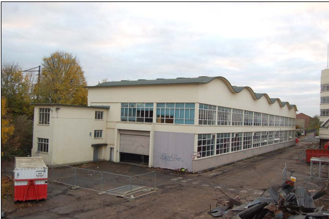
Plate 110 Building 720 viewed to south-west
