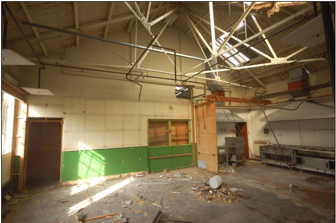
Plate 28 Room 11 (former 1929 drawing office)
