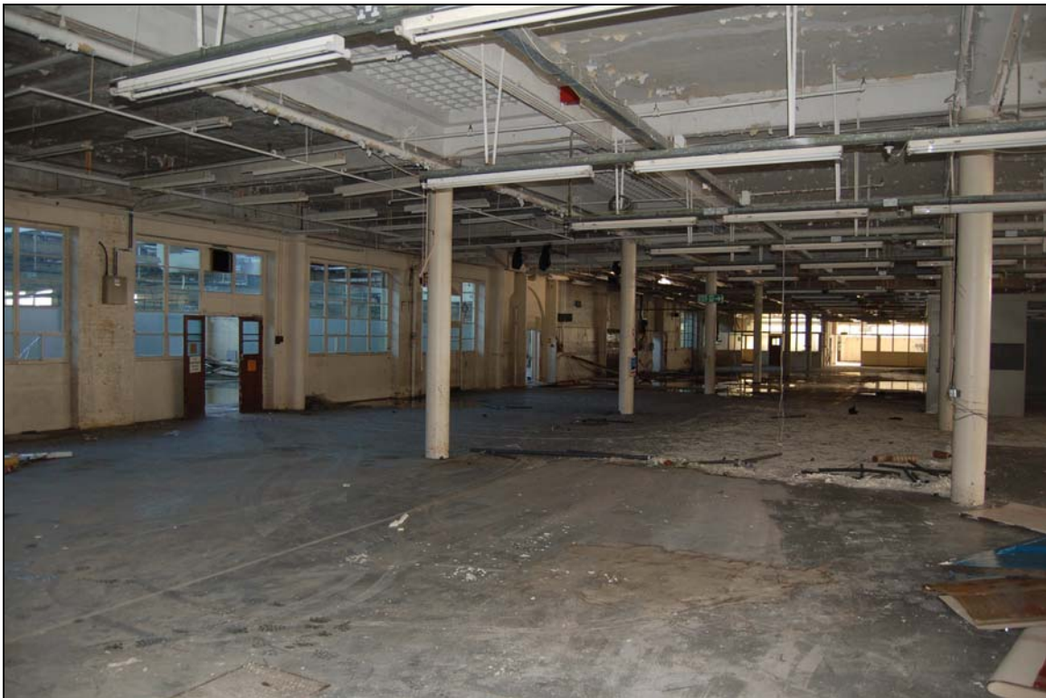
Plate 68 Factory interior viewed to north-east (outer wall of 1912 factory)
