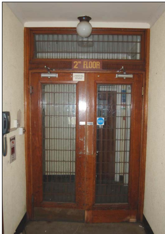
Plate 94 typical corridor swing doors
