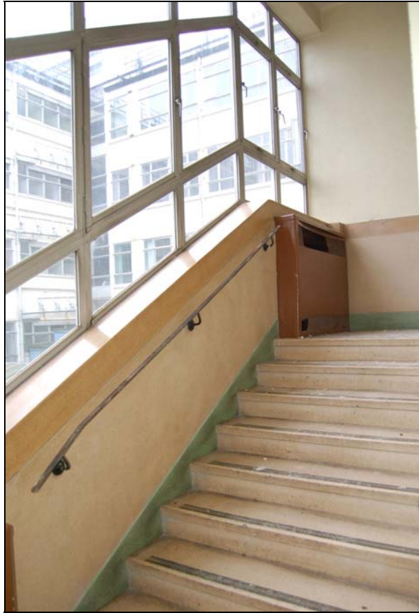
Plate 109 West wing stair
