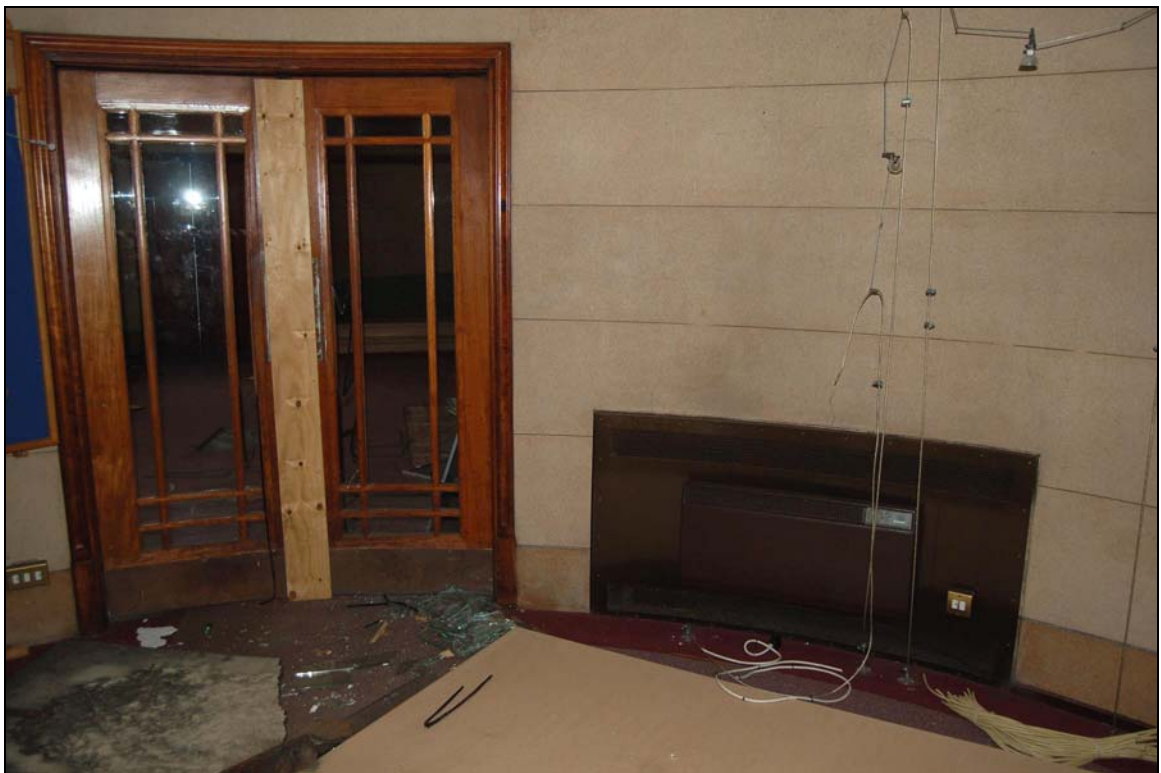
Plate 86 Doors between lobby 1 and foyer 2
