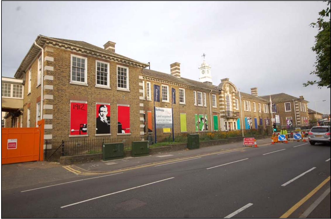
Plate 1 1912 Offices viewed to north-west
