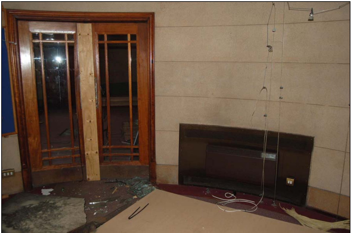
Plate 86 Doors between lobby 1 and foyer 2
