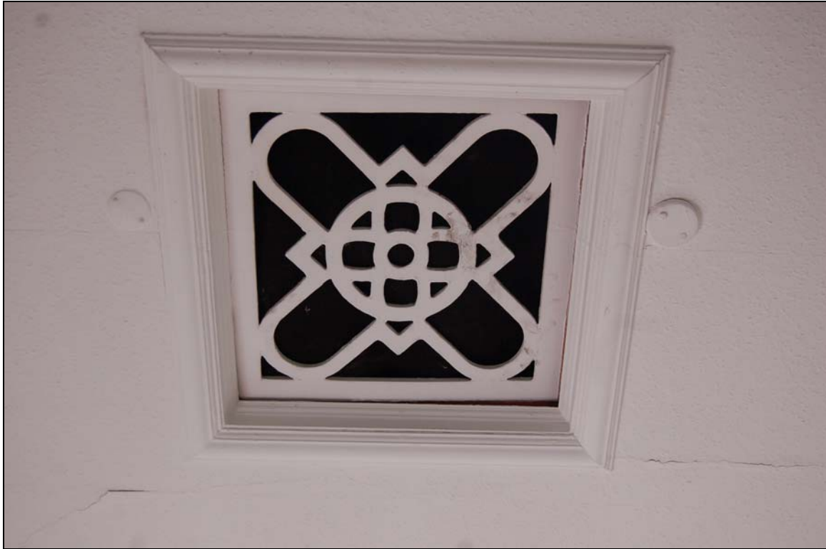
Plate 21 Ventilation grill observed in room 3 on first floor of 1912 offices
