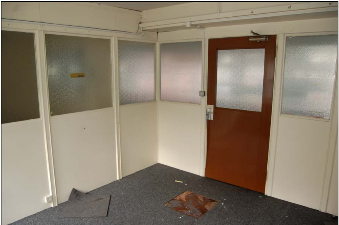
Plate 118 Typical office interior
