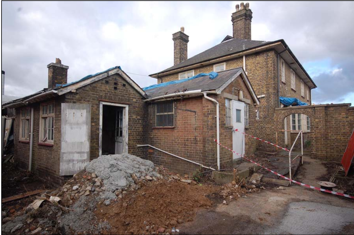
Plate 143 Weigh house and oil store viewed to north-west
