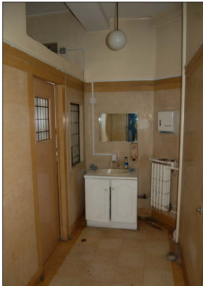
Plate 100 Washroom adjacent to room 4 on second floor
