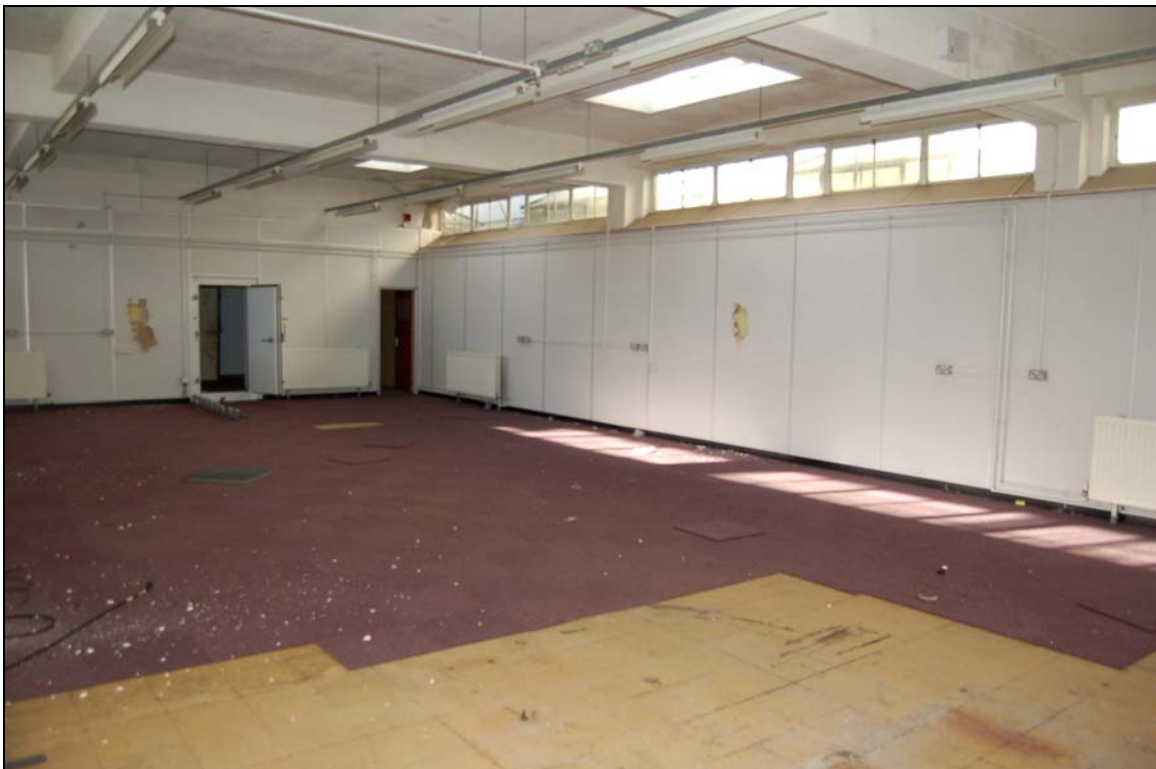
Plate 124 Kitchen 3 viewed to north-west
