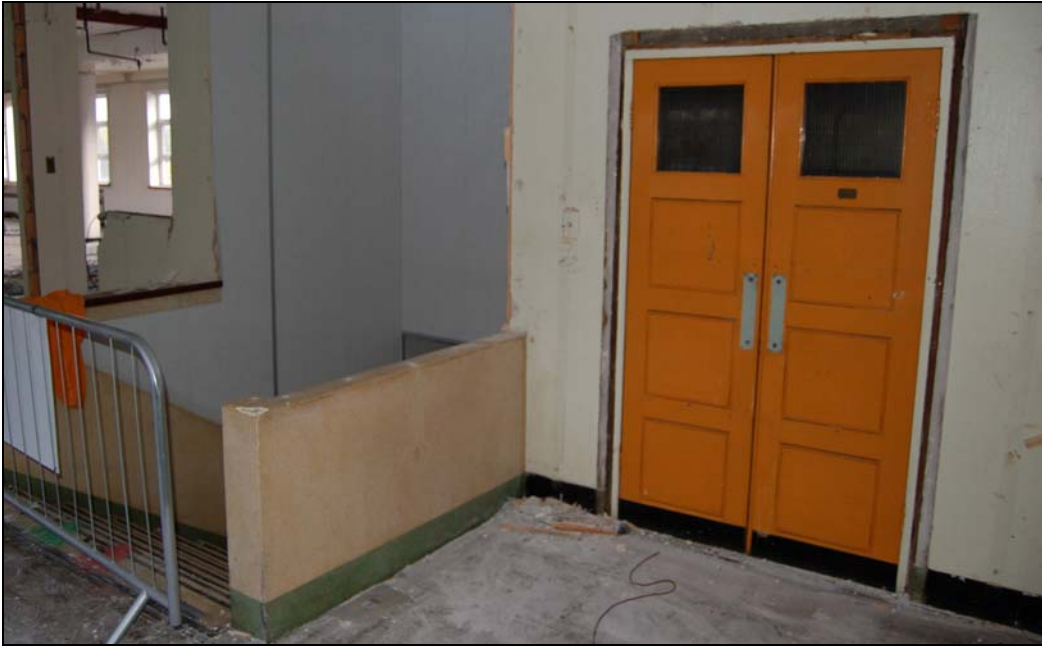
Plate 73 Typical corridor doorway
