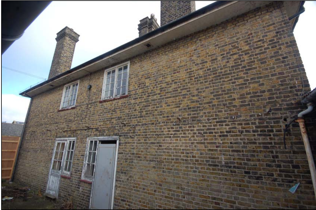
Plate 137 Rear elevation (west)
