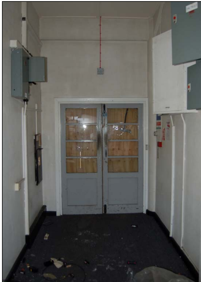
Plate 74 Typical fire escape doorway
