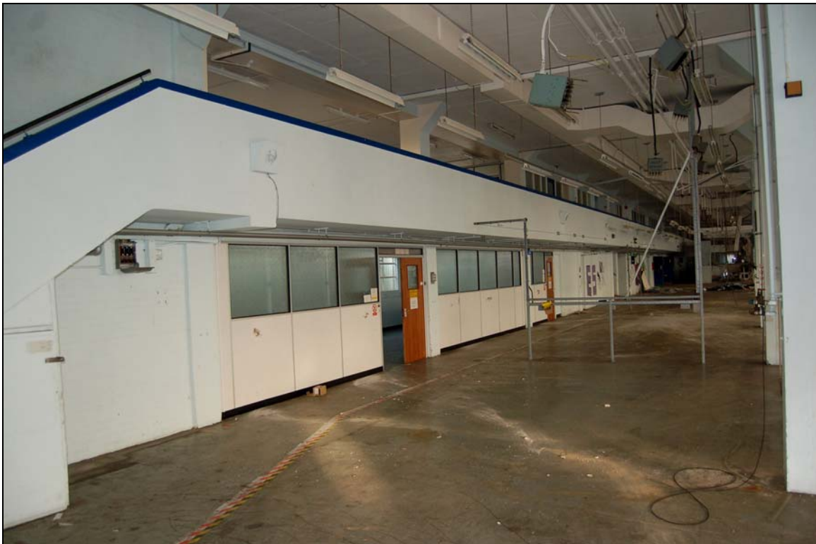
Plate 114 Balcony and mezzanine floor over factory
