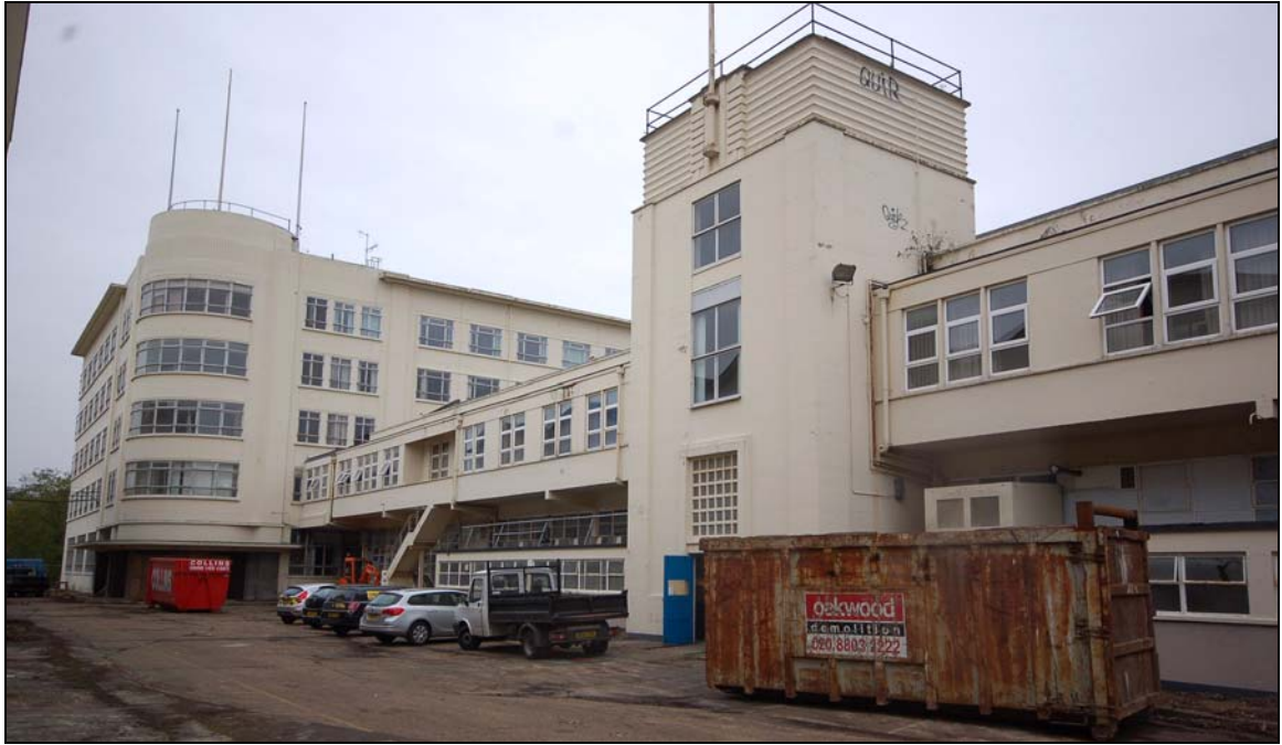
Plate 61 West end of 1937 factory, with Marconi House to left
