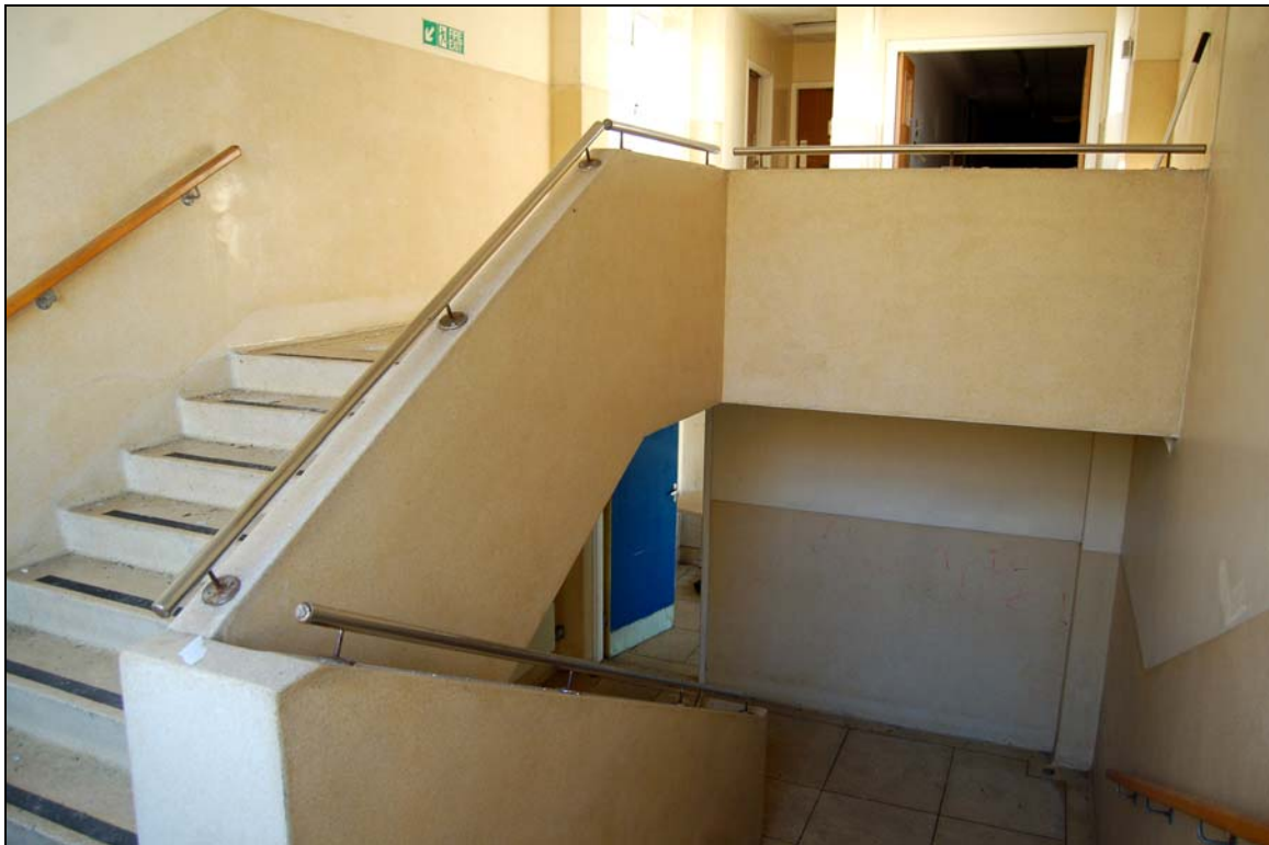
Plate 116 Stairs in Building 720
