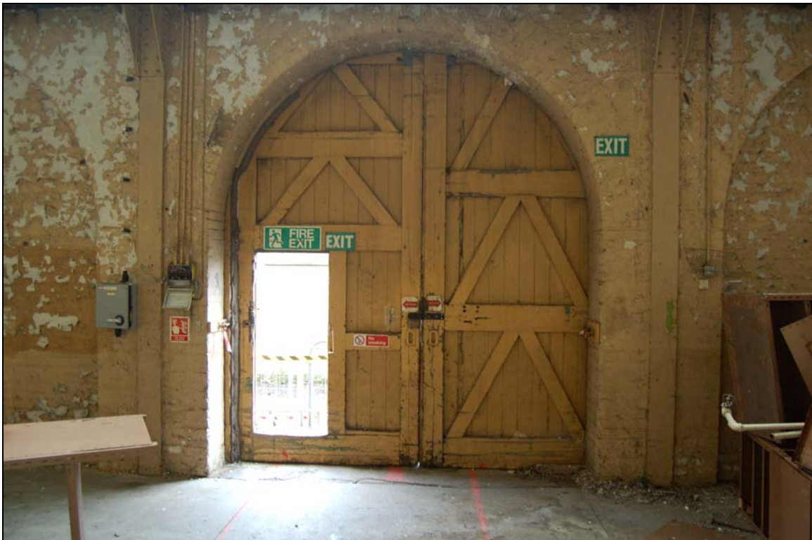
Plate 52 Typical factory loading door from railway siding
