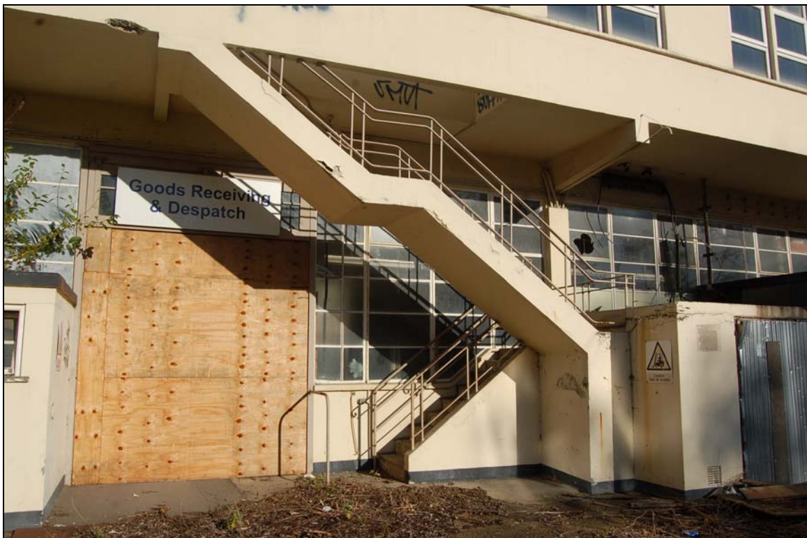
Plate 64 Fire escape stair
