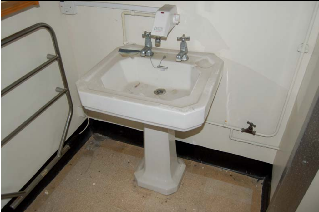
Plate 105 Sink adjacent to room 14
