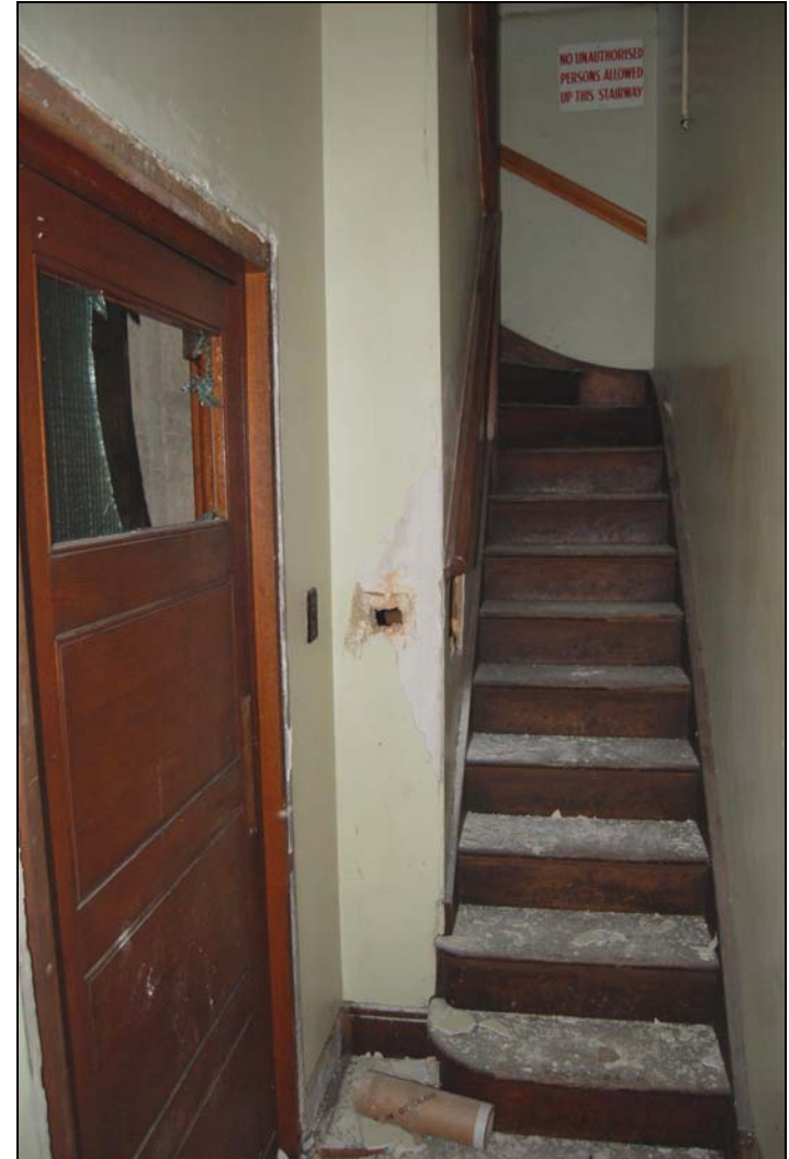
Plate 76 Stairs to second floor above manager's office 2
