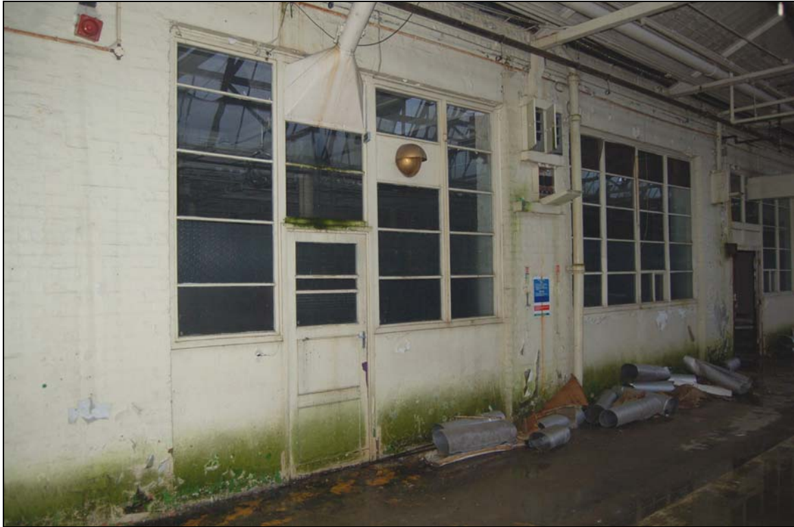
Plate 47 1930s partitioning on south wall of 1912 factory
