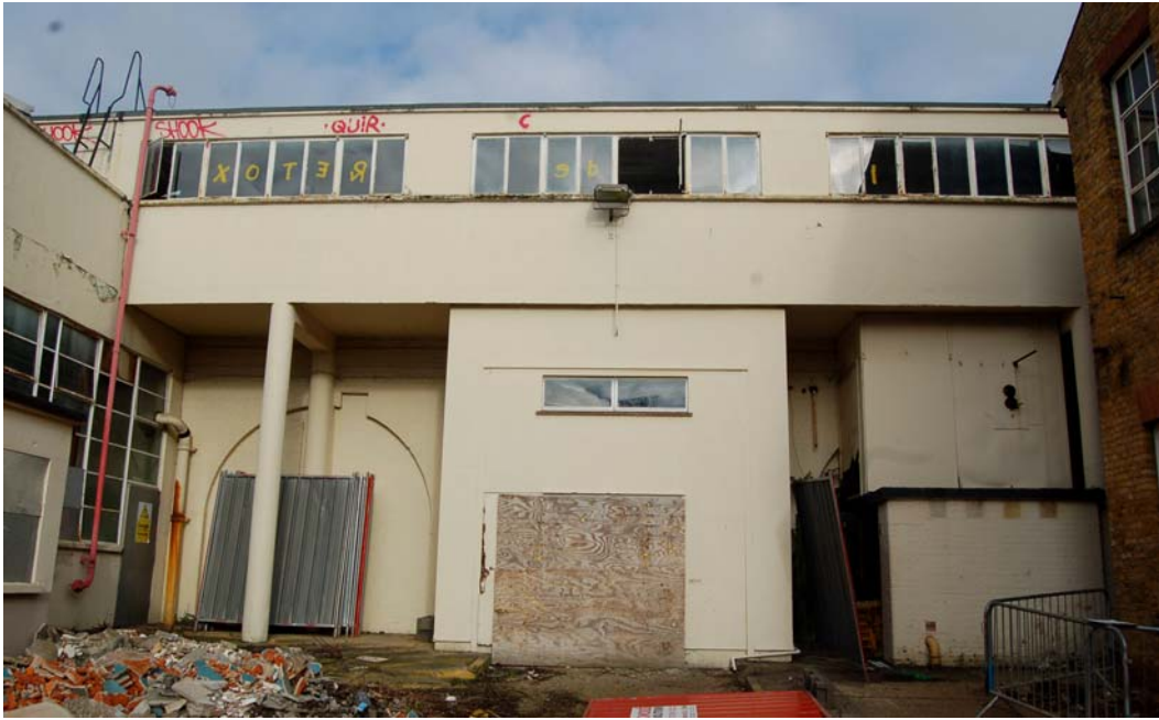
Plate 43 Exposed arch on south elevation of 1912 factory
