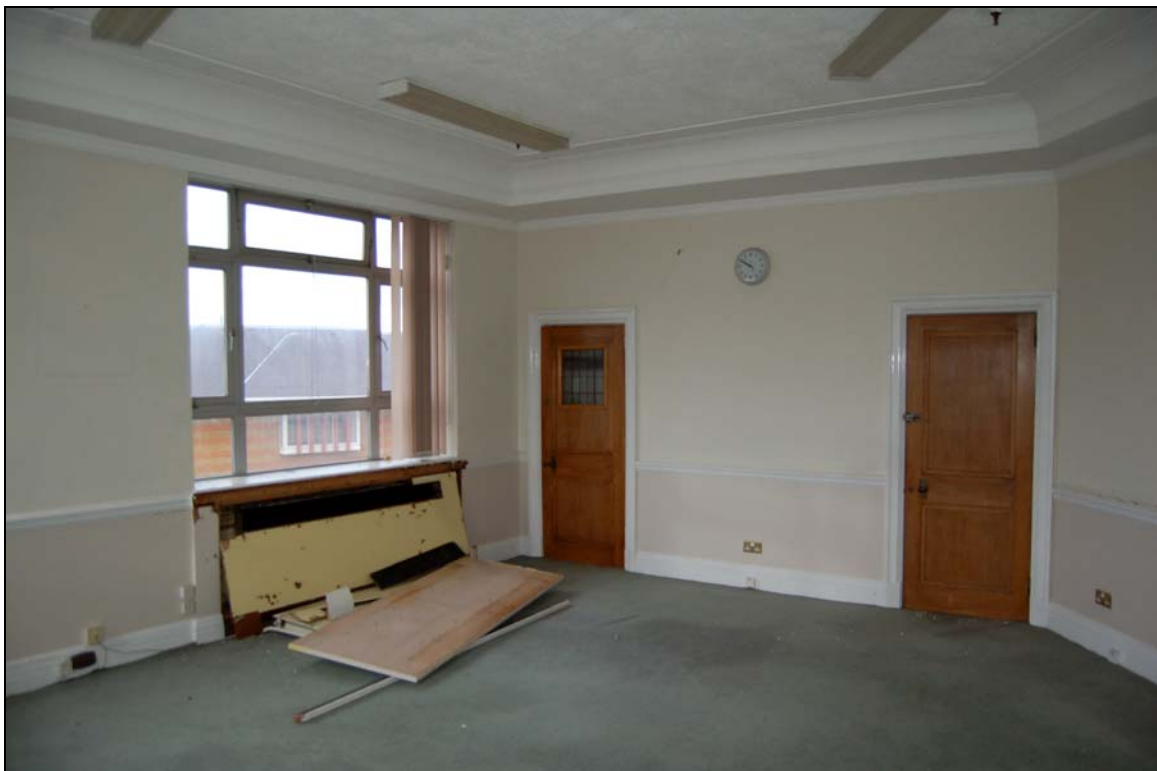
Plate 104 Room 14 on first floor, viewed to north-west
