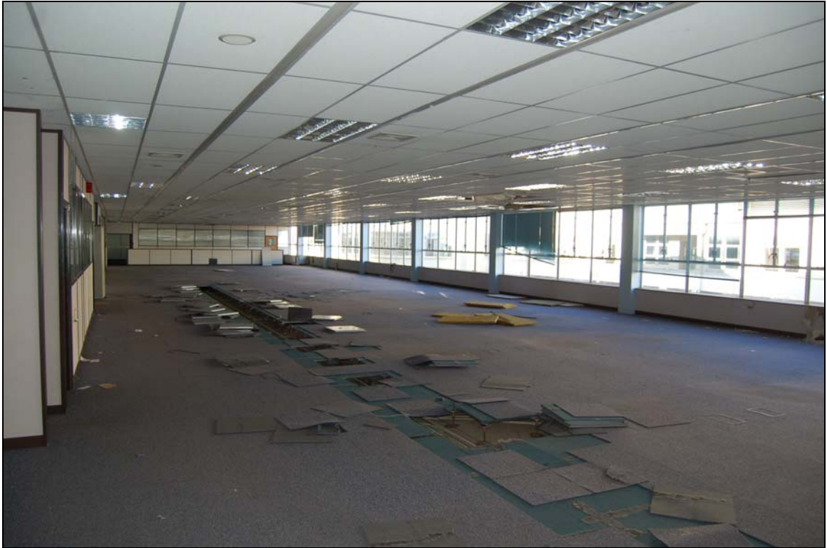
Plate 119 First floor viewed to west
