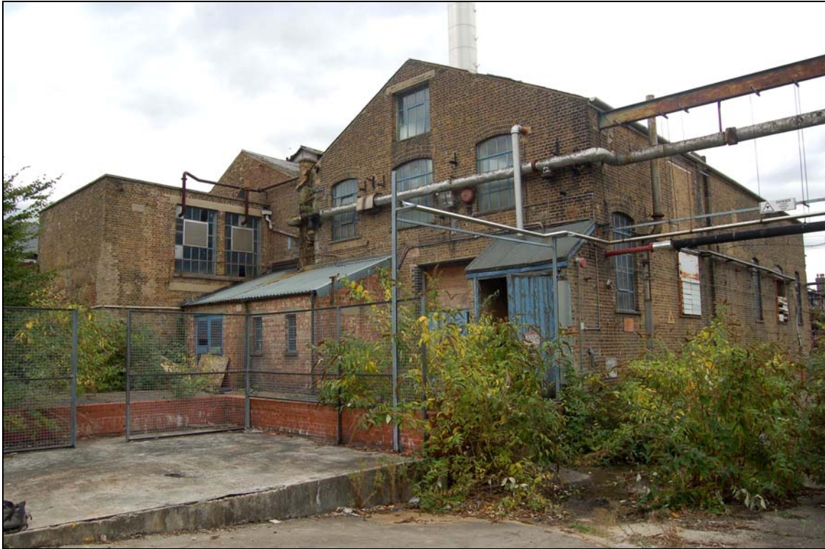
Plate 127 Power house viewed to north-east
