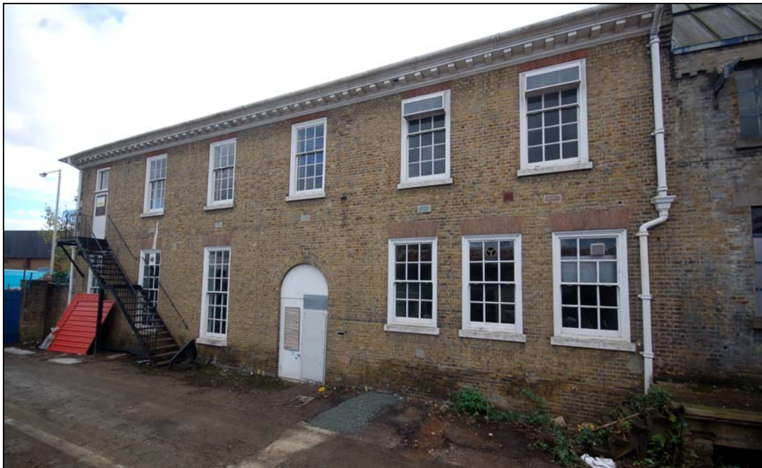
Plate 4 North elevation of 1912 offices
