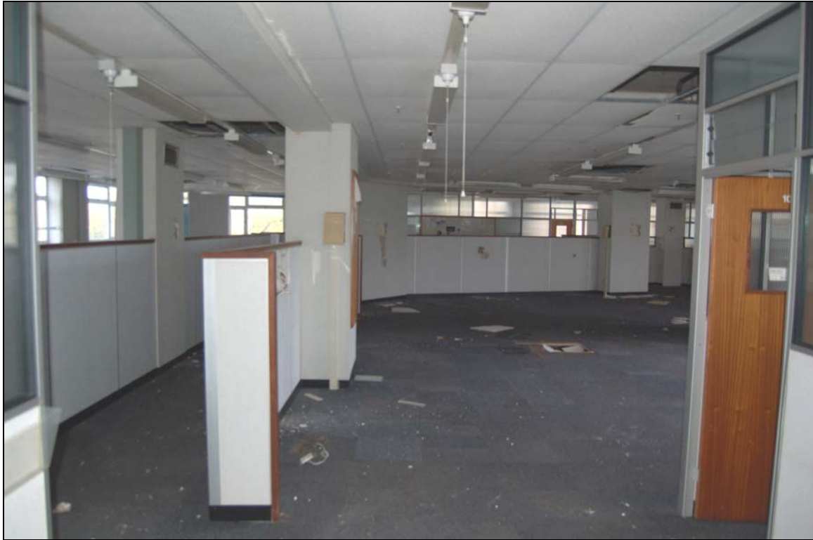
Plate 103 First floor modern office space (rooms 3 & 8)
