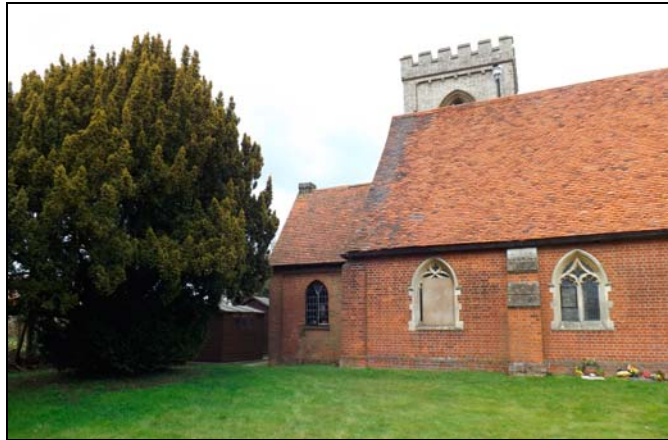
Plate 1: Vestry location at the west end of the nave, looking north.
