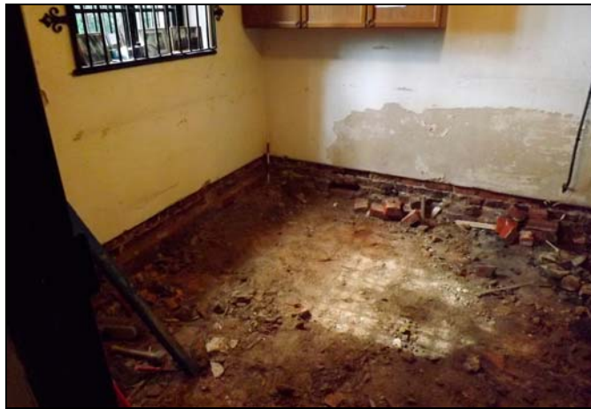
Plate 2: Vestry interior after the removal of existing timber flooring, looking west.
