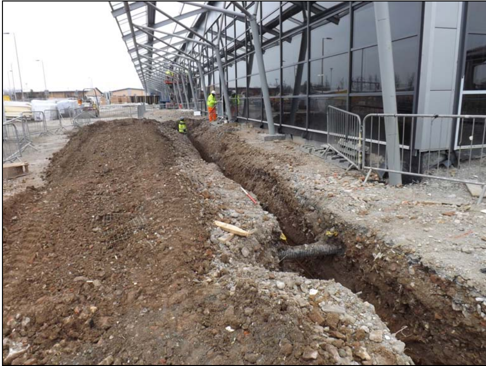
Plate 3: Sewer trench east of terminal extension, looking south (1m scale)
