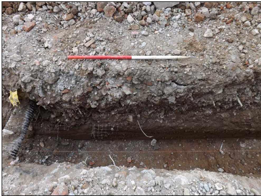
Plate 4: West facing section of sewer trench, looking east (1m scale)
