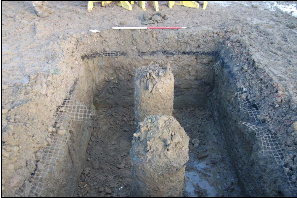
Plate 1: Excavation around pile cap 74, looking north (1m scale)
