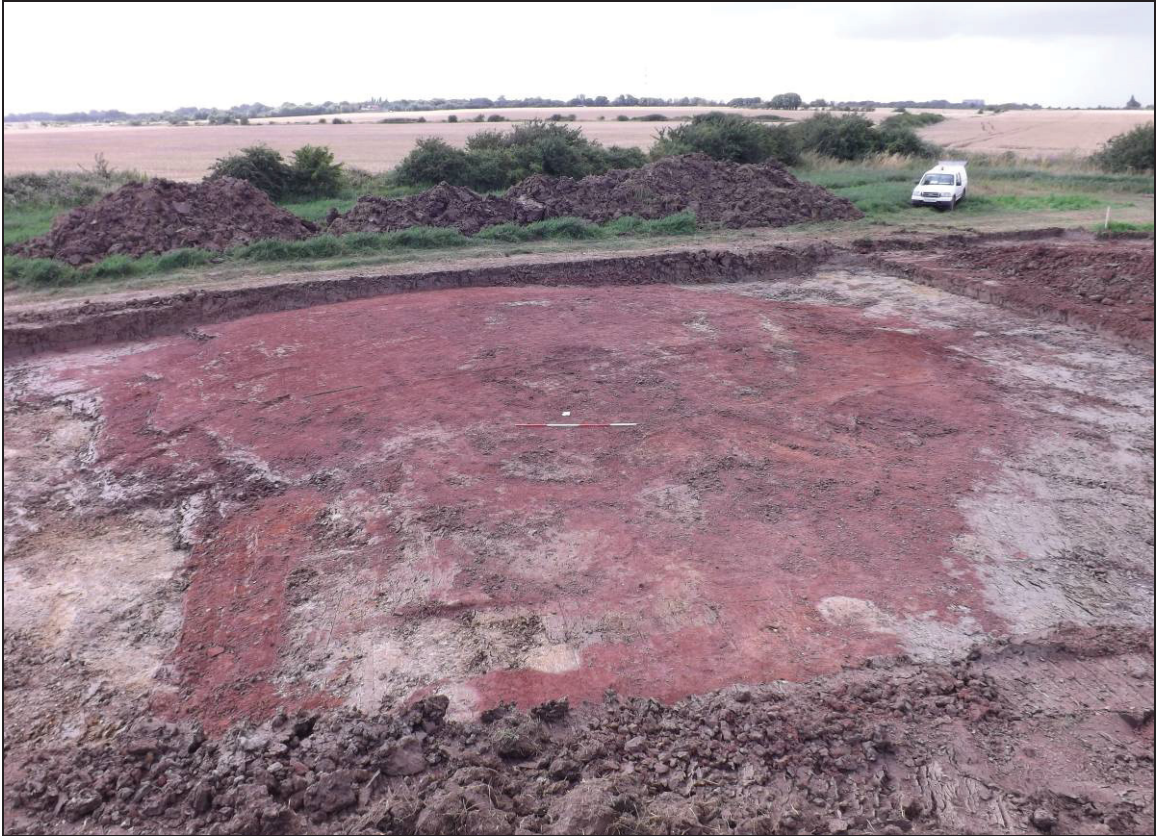
Plate 1. Turbine 106 site - general view prior to excavation, looking NW (2m scale)
