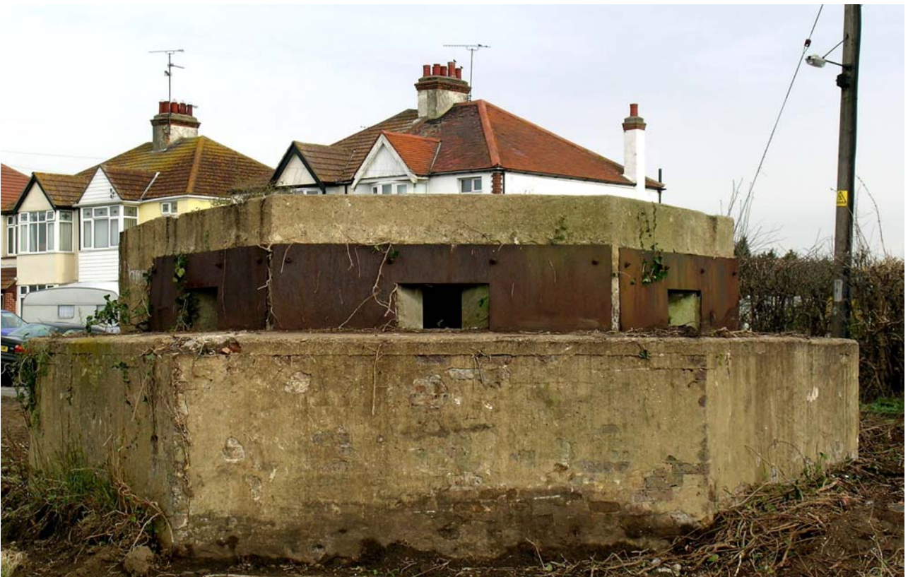
Plate 2. South-east facing side of pillbox (section 1)
