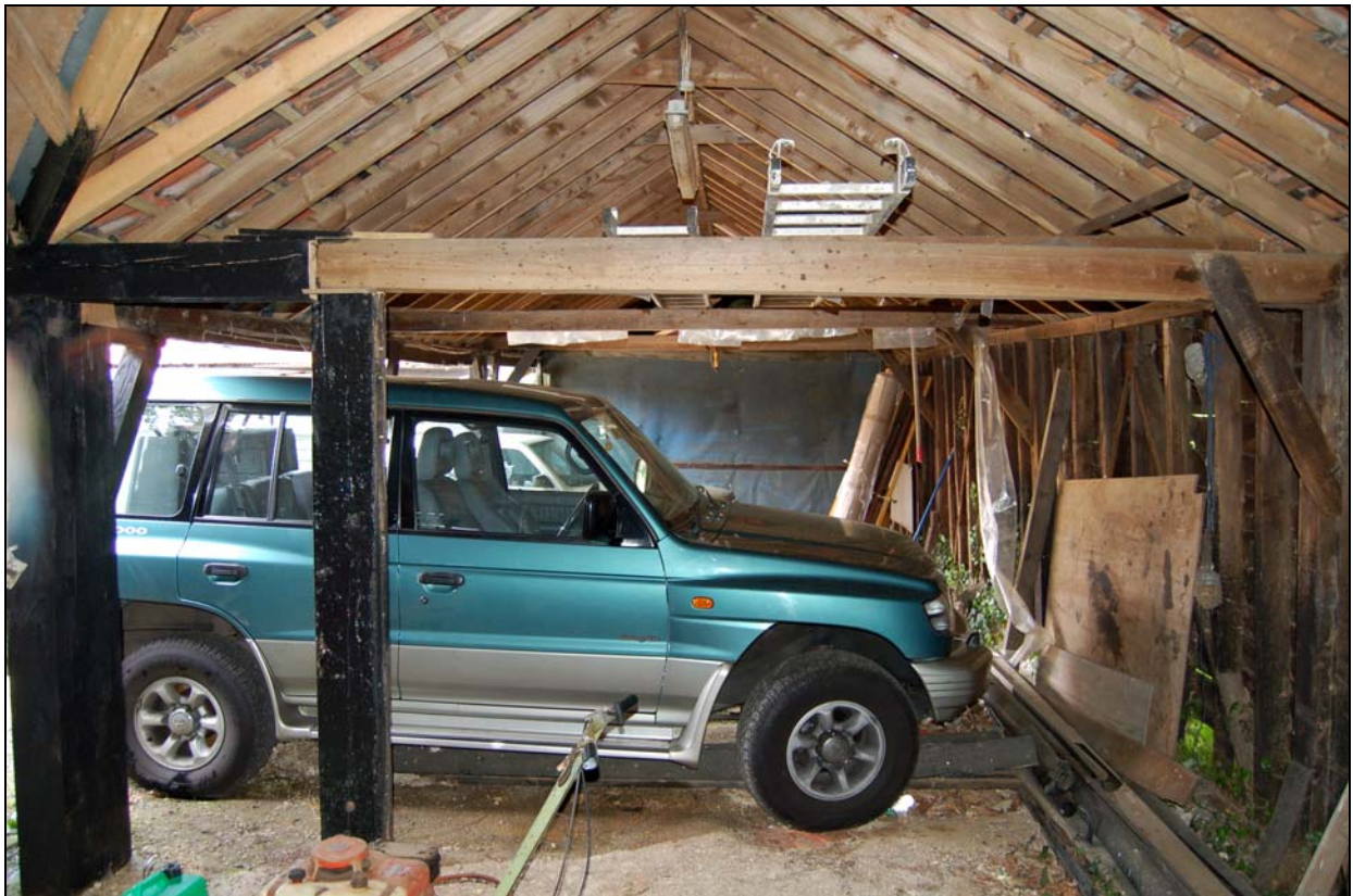
Plate 20 Interior of Shelter Shed 5 viewed from south-west
