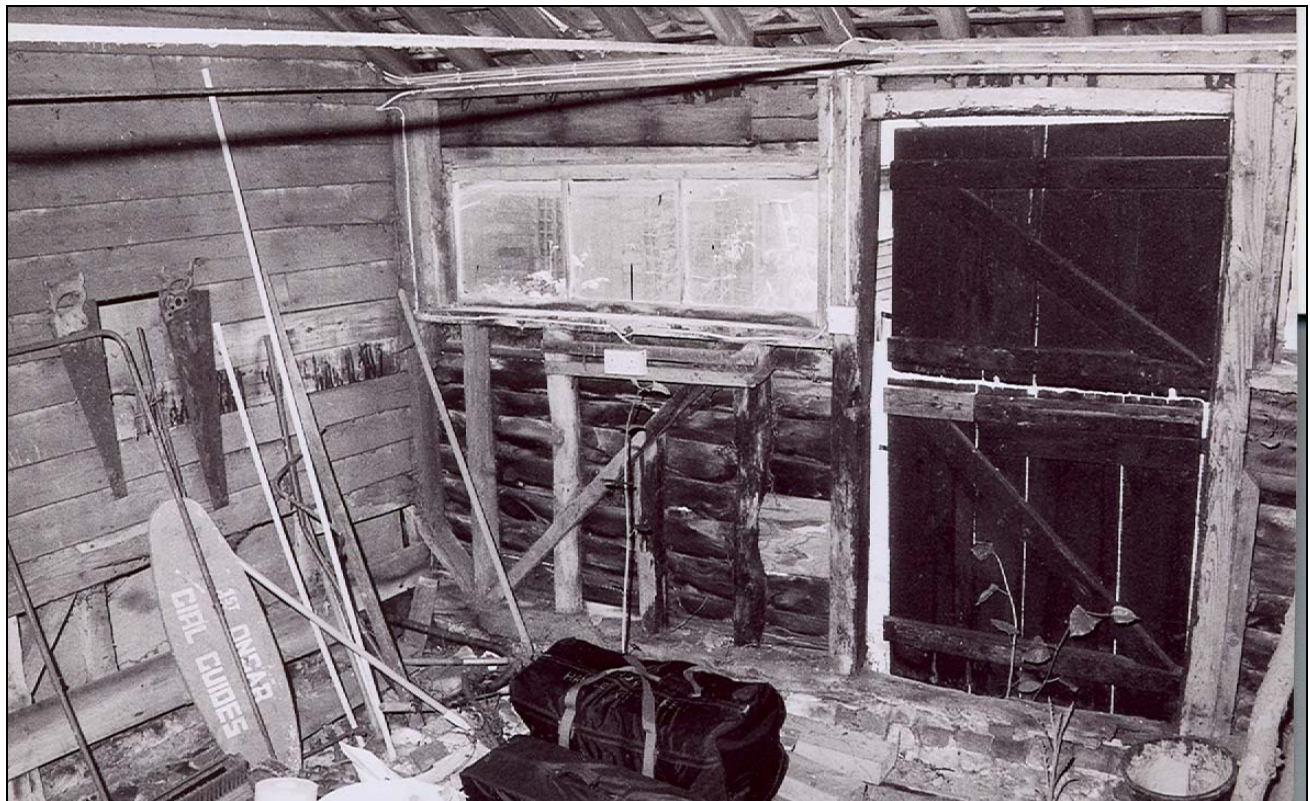
Plate 12 Partial 18th-century walling in first bay of Cowhouse 2
