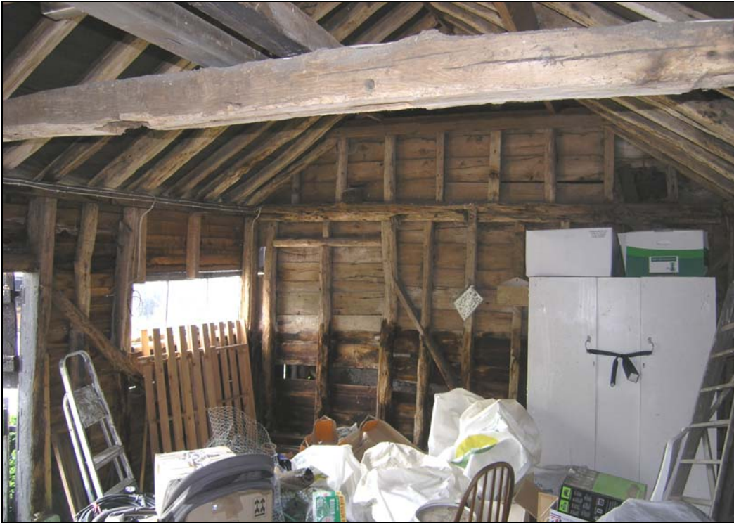
Plate 6 Interior of Shed 1, viewed from north showing blocked doorway
