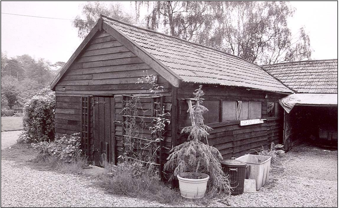
Plate 21 Former Shelter Shed 6, viewed from west
