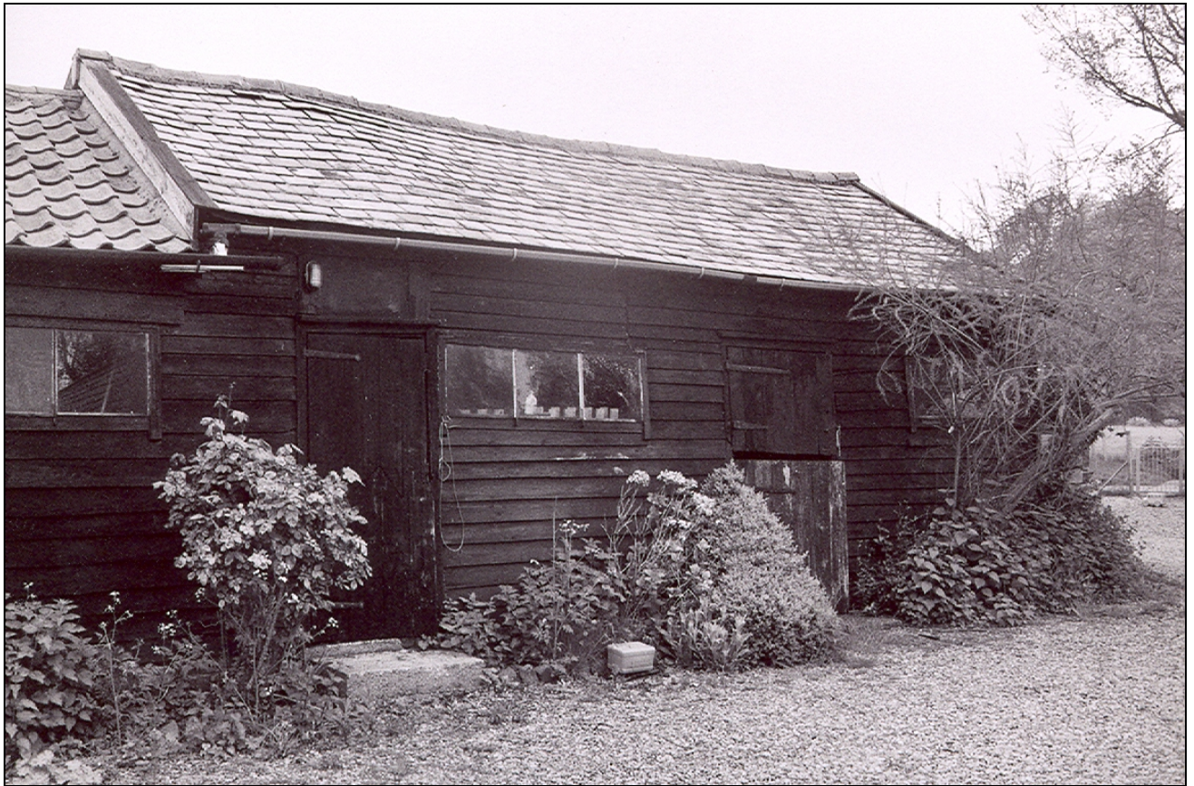
Plate 4 Former Shelter Shed 1 viewed from south
