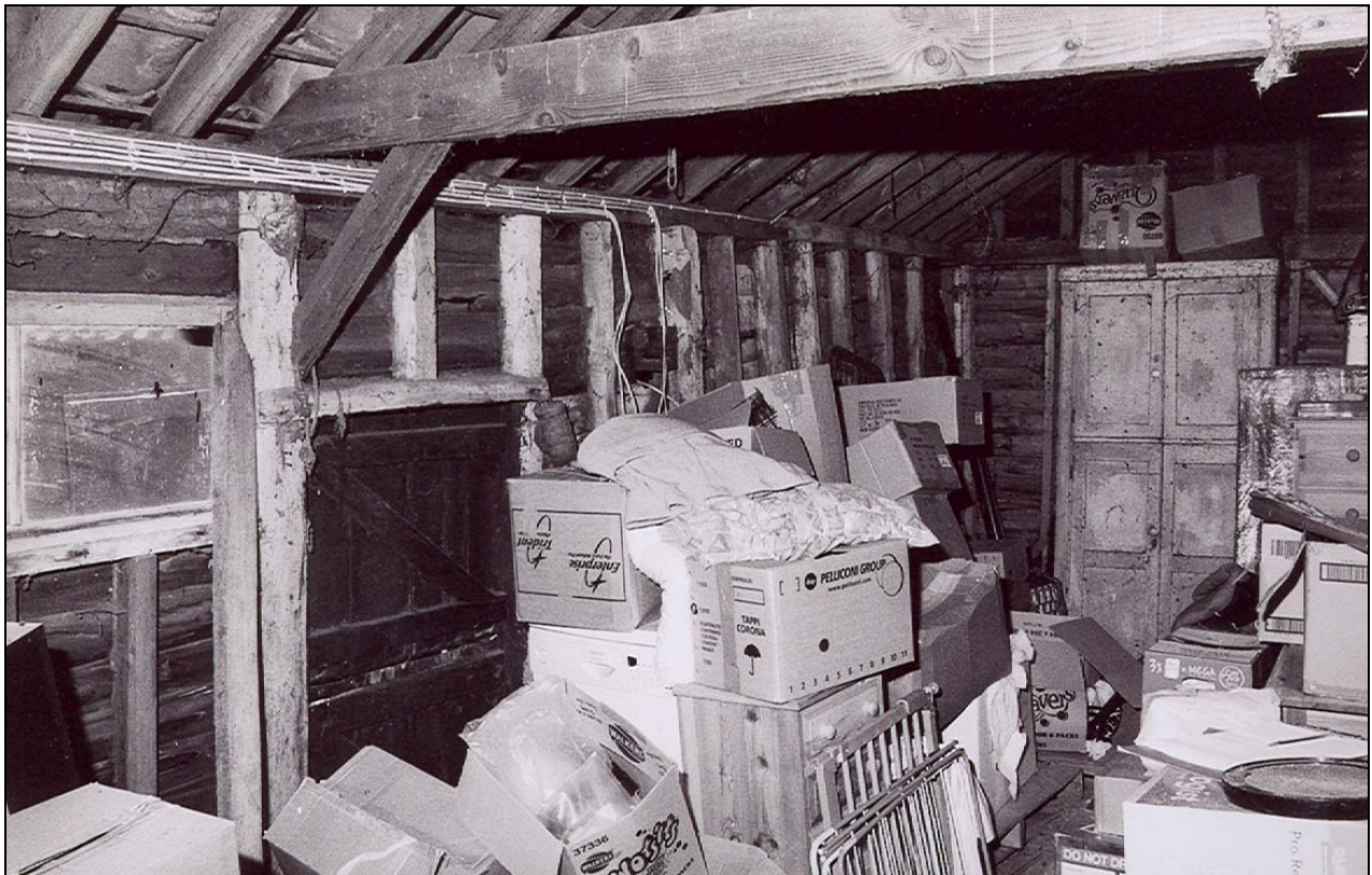
Plate 14 Original wall framing around doorway into third bay of Cowhouse 2
