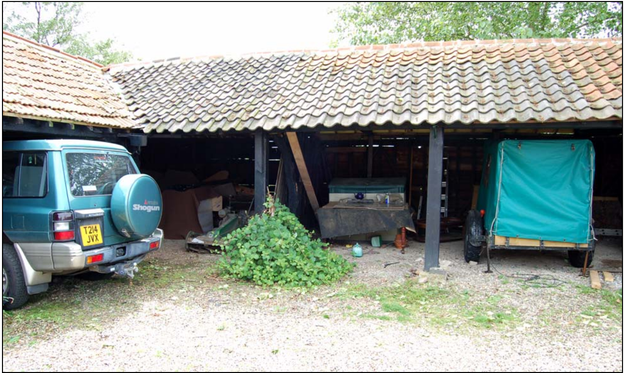
Plate 17 Close-up photograph of Shelter Shed 4
