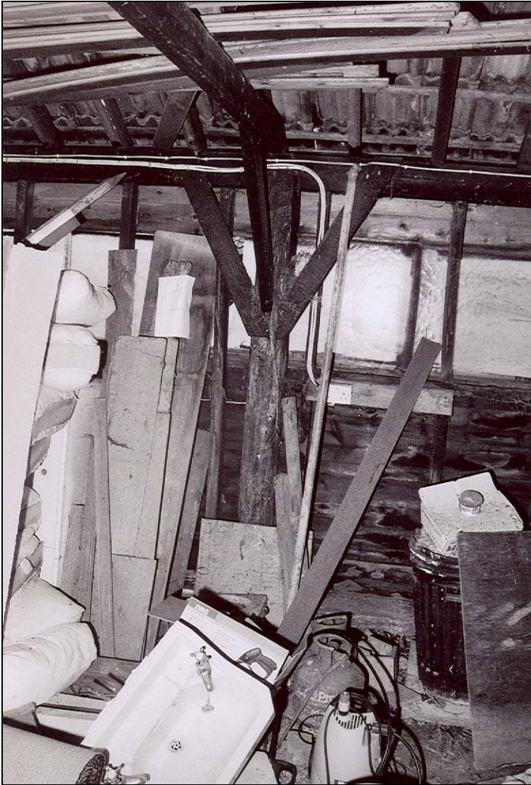
Plate 23 Braced bay post inside Shelter Shed 6
