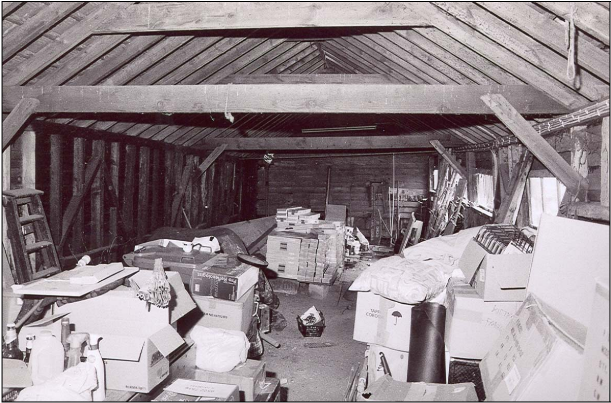
Plate 13 Interior of Cowhouse 2 viewed from south-west
