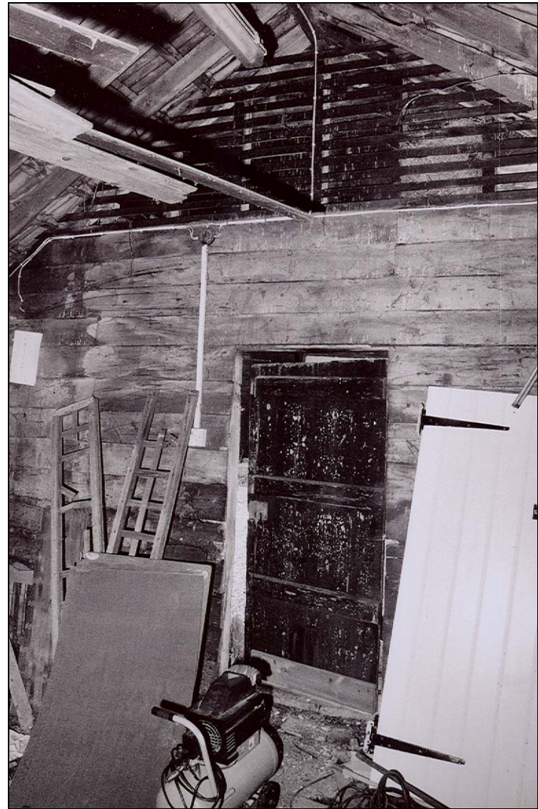
Plate 24 Ventilated gable inside north-west gable of Shelter Shed 6
