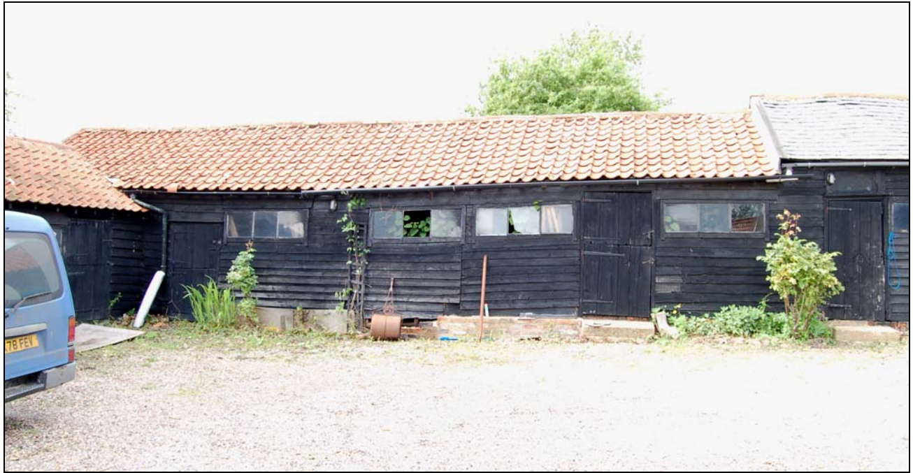
Plate 11 Front elevation of Cowhouse 2, showing wall scar between bays 1 and 2
