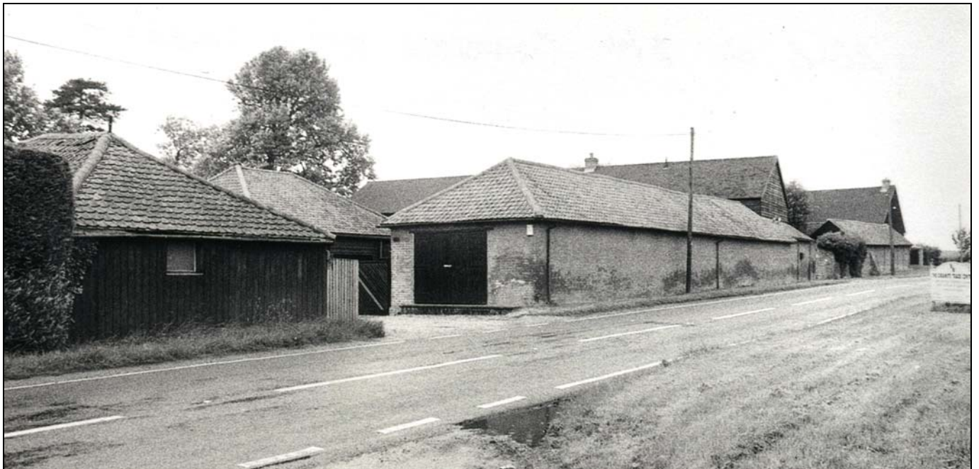
Plate 6 Longbarns farm viewed to north-west from main road
