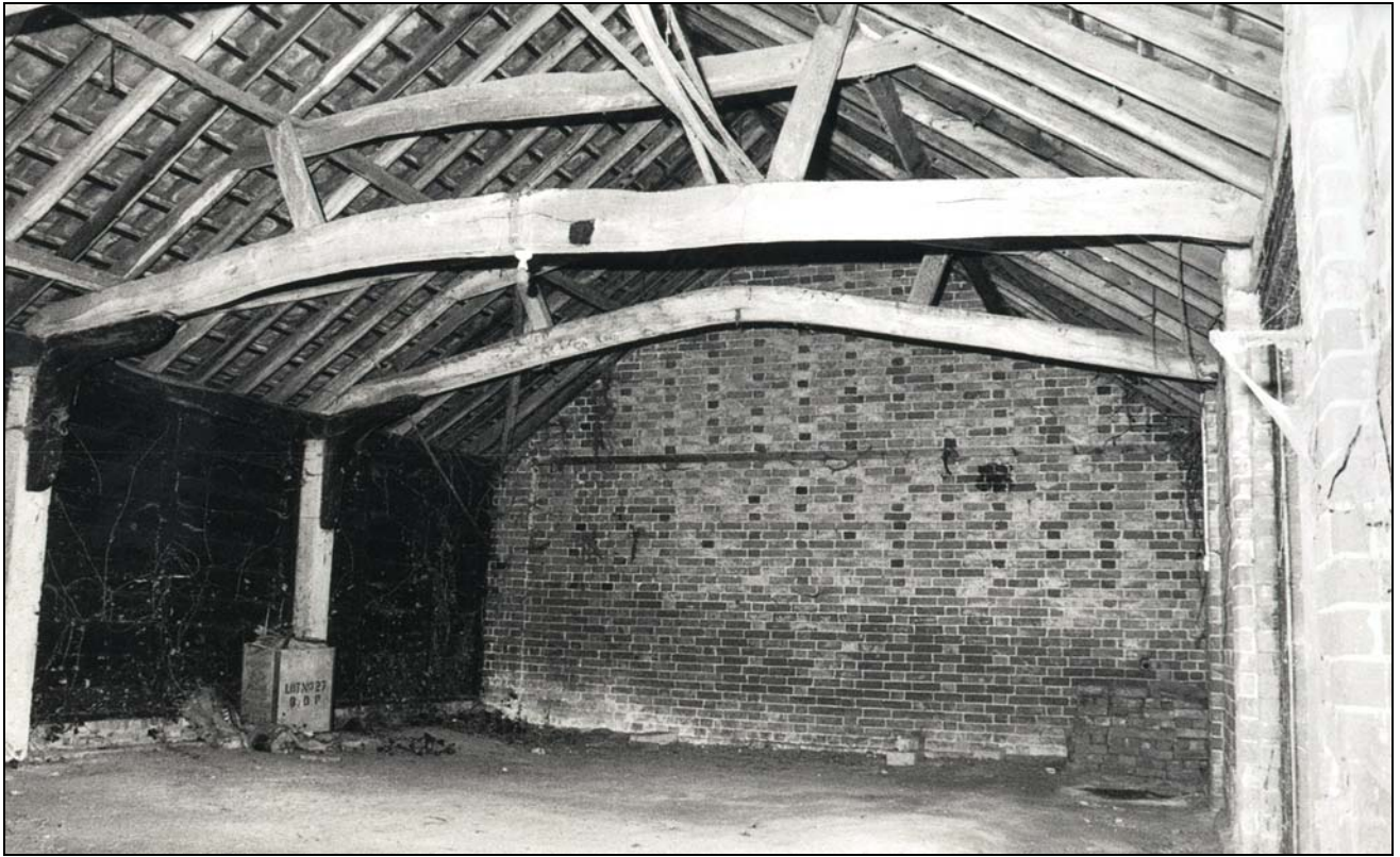
Plate 11 East wall of cart shed
