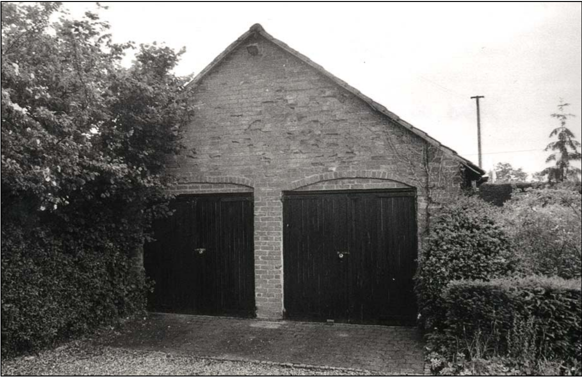
Plate 3 Inserted garage doors on west elevation
