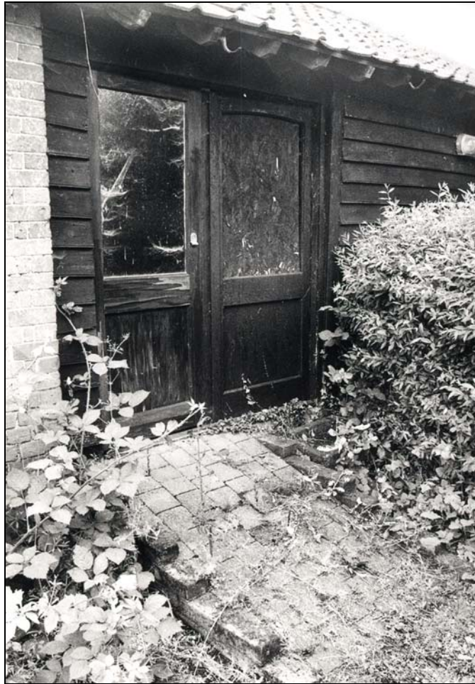
Plate 5 South elevation of stable
