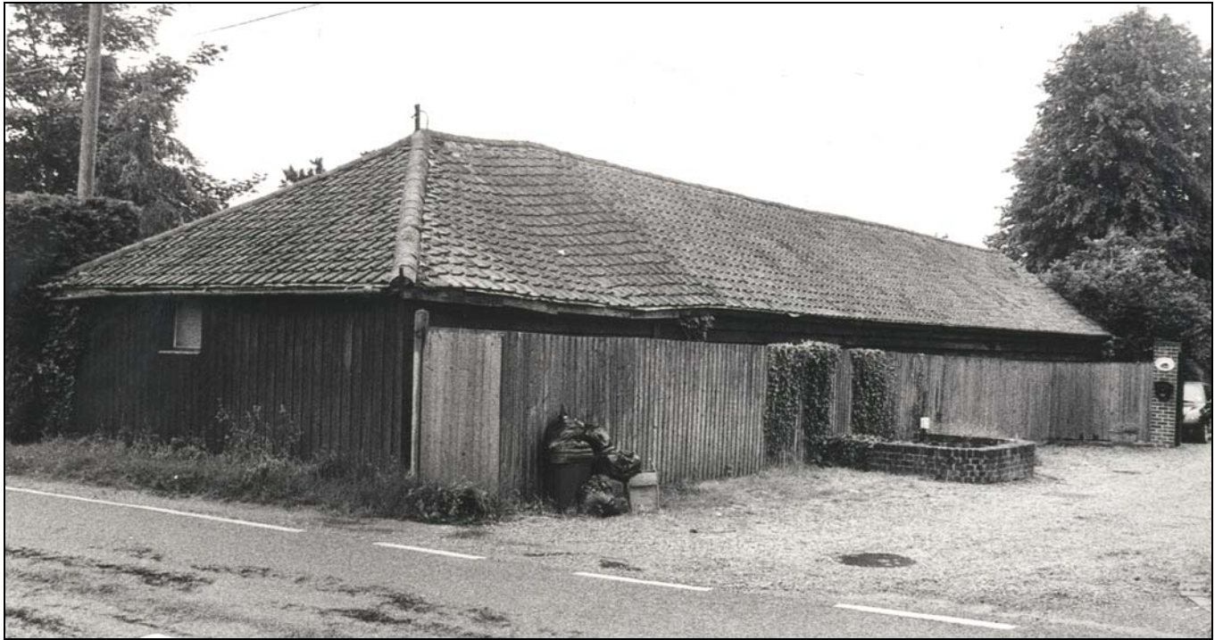
Plate 7 Cart shed viewed to south-west
