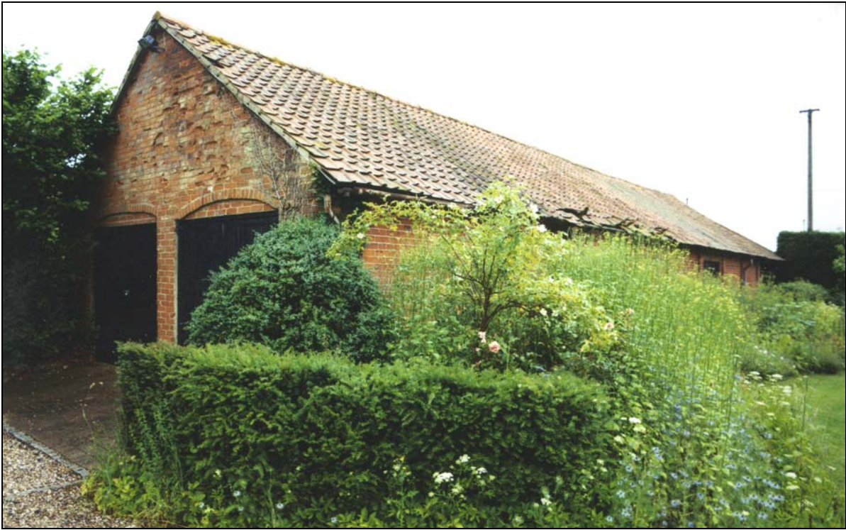
Plate 1 Cart shed viewed toward north-east
