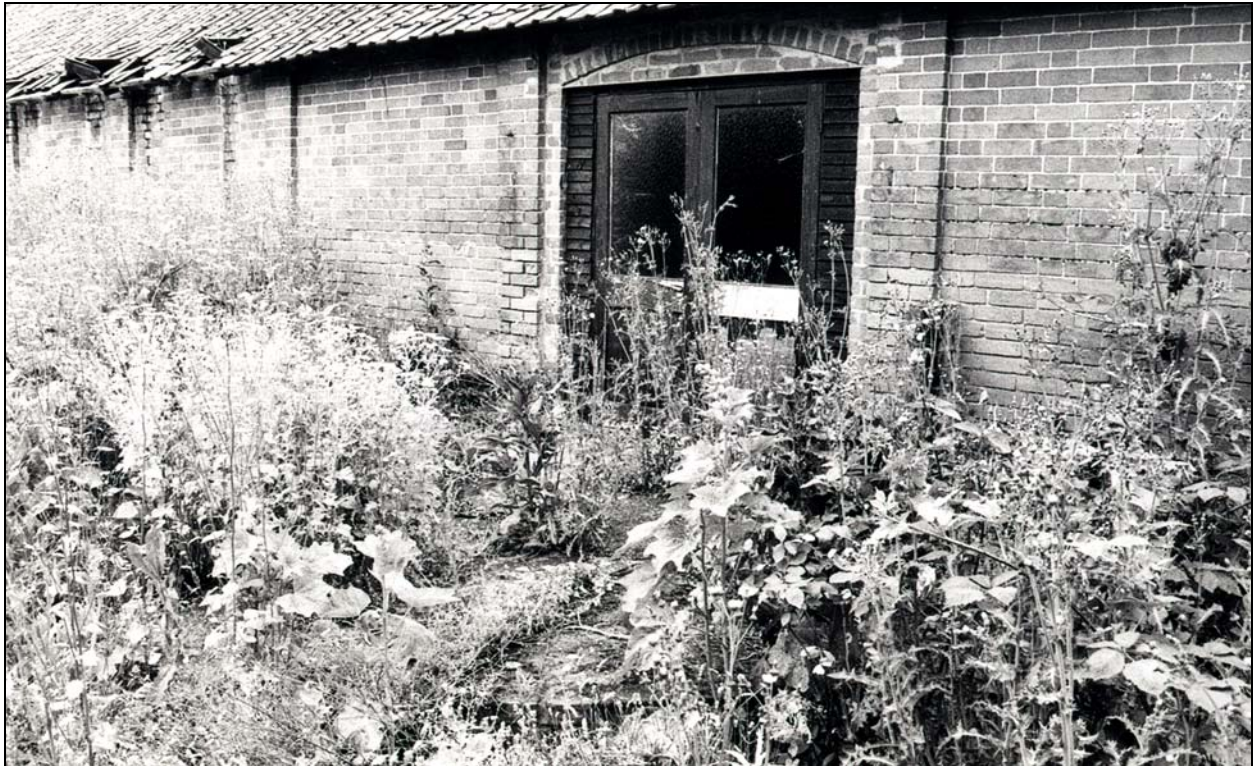
Plate 4 Modern entrance into cart shed, possibly a later insertion
