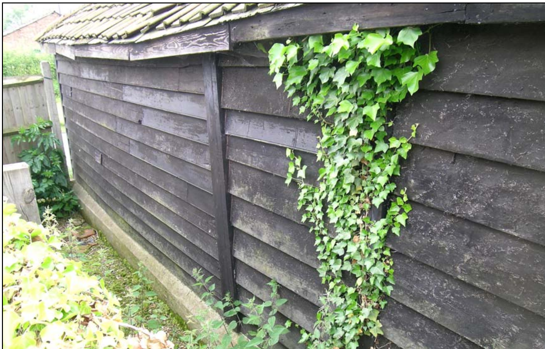
Plate 8 Later plain clap board infill of cart shed (right) compared with beaded covering to stable (left)
