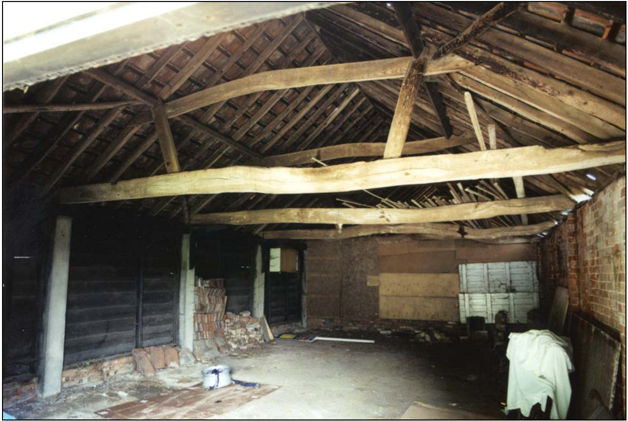
Plate 9 Interior of cart shed viewed to east and modern partition
