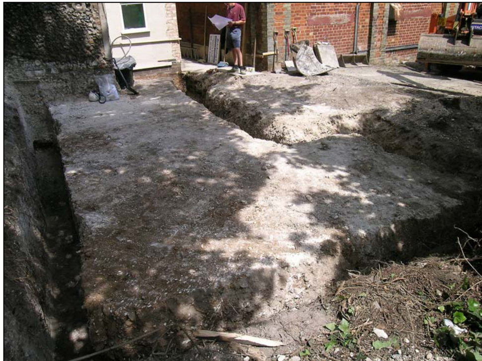
Plate 2. Site reduced and foundation trenches cut; looking northeast
