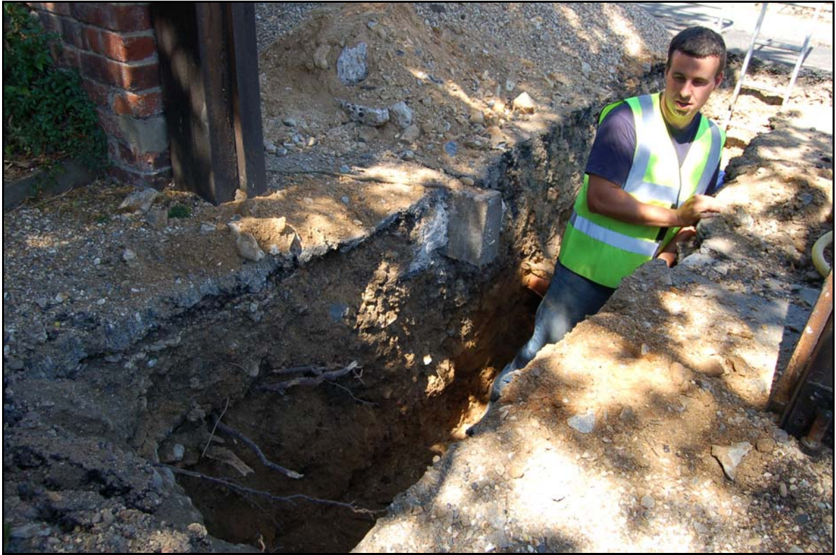
Plate 1. Sewer trench at point of postulated Roman enclosure wall foundation
