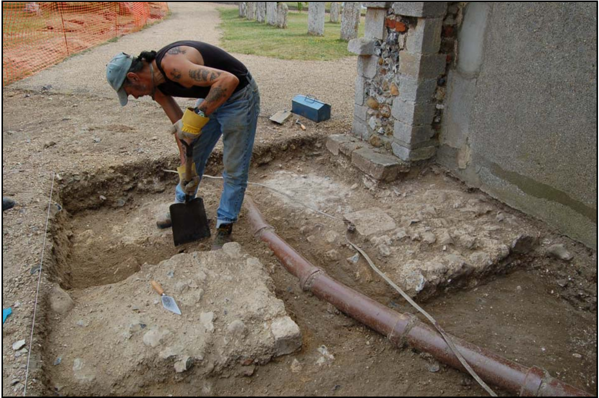
Plate 3. Footprint of proposed toilet facilities, wall 14, looking north
