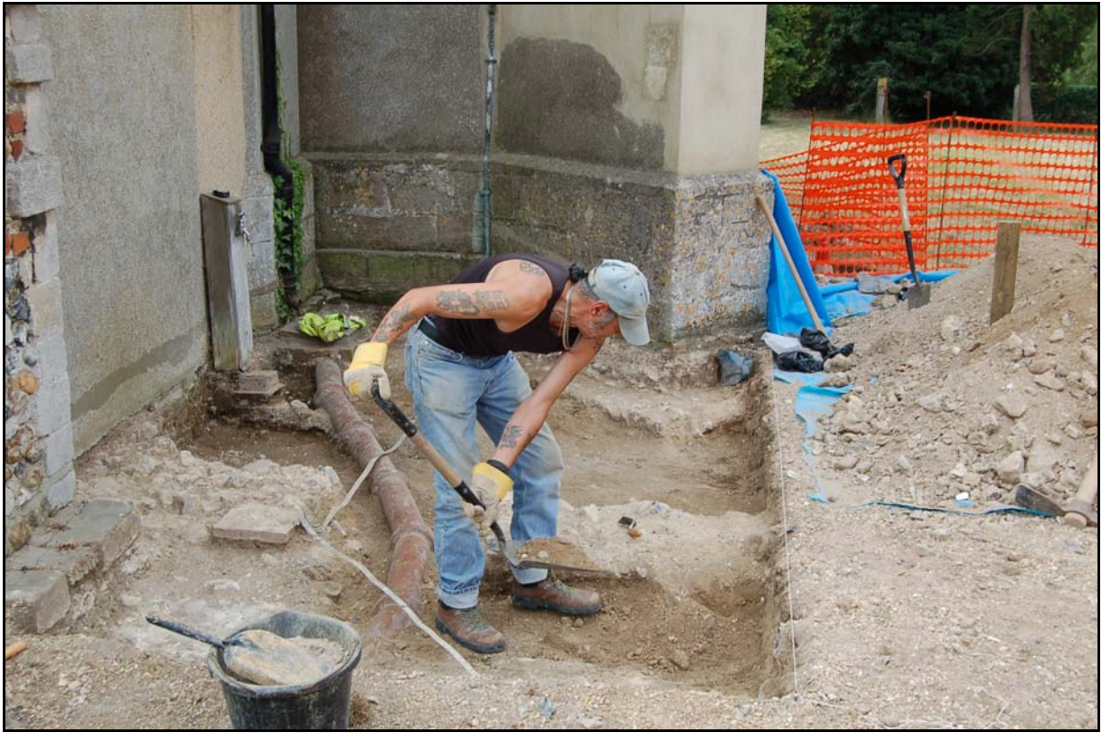
Plate 2. Footprint of proposed toilet facilities, looking south towards church tower
