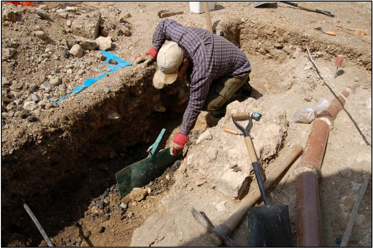
Plate 4. Copper-alloy plate, earthing point for lightning conductor
