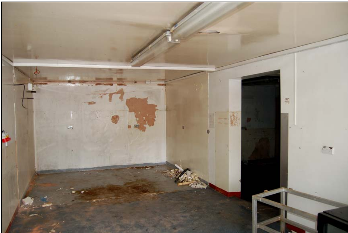
Plate 8 Stripped-out shop interior
