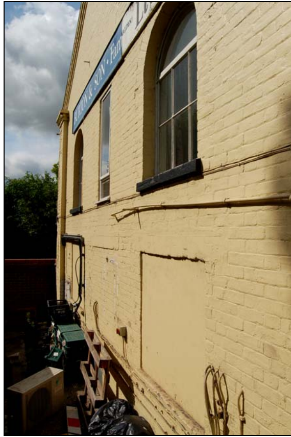
Plate 5 Blocked central doorway and modern windows on east elevation
