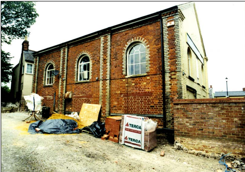
Plate 6 Exposed brickwork on south elevation of chapel
