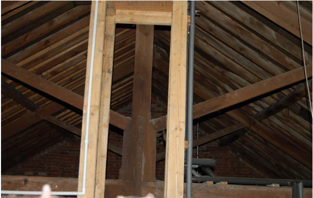
Plate 13 King post strut roof truss
