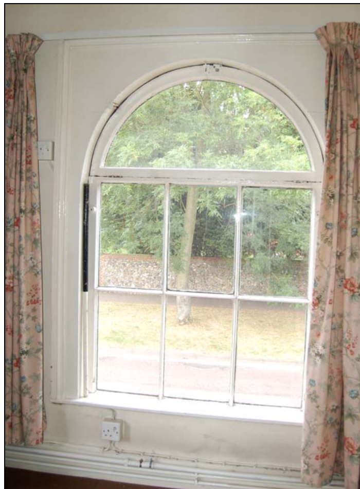
Plate 10 Top-opening window on east elevation
