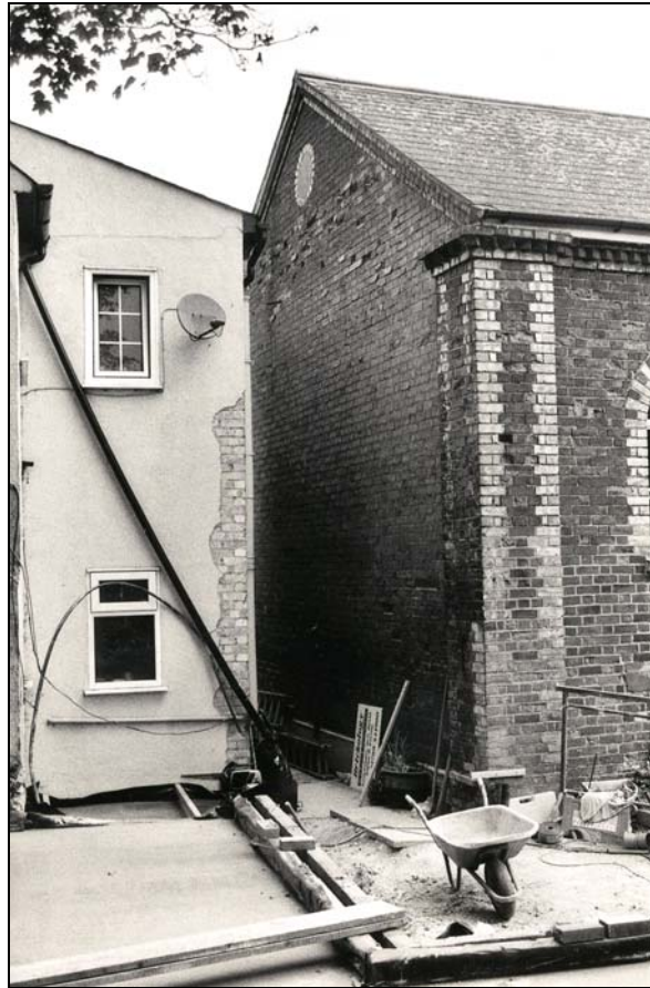
Plate 7 Blocked gable light on west elevation during building works
