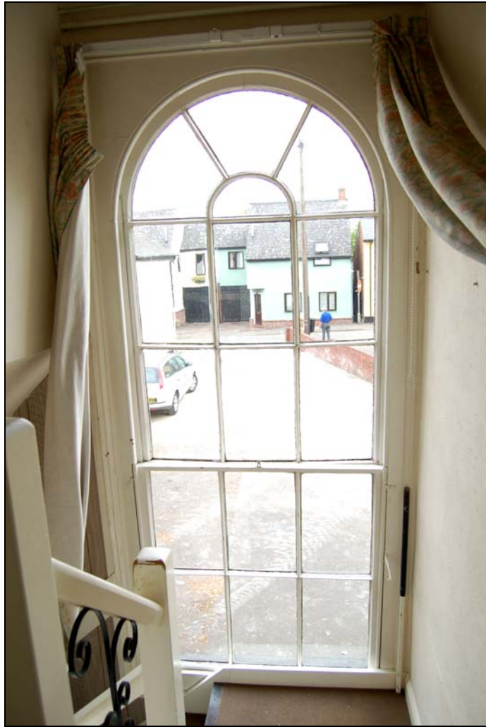
Plate 11 Stair window on north elevation
