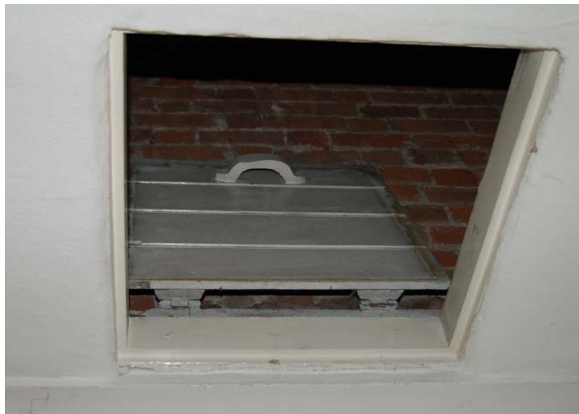
Plate 12 Loft hatch in bathroom
