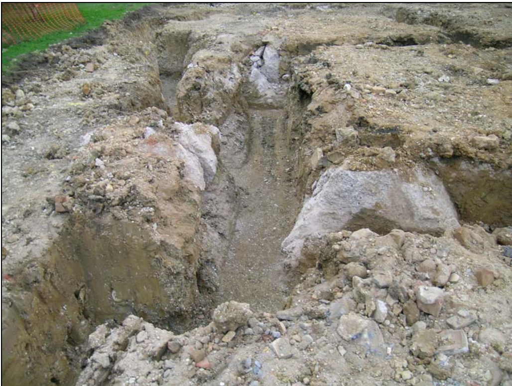
Plate 2. Detail of modern disturbance in house foundation trenches
