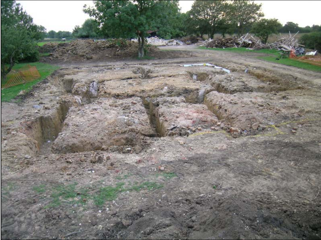
Plate 1. House foundation trenches, looking west
