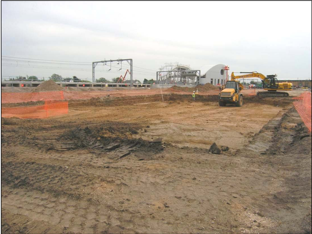
General view of attenuation tank excavation. Looking south-east
