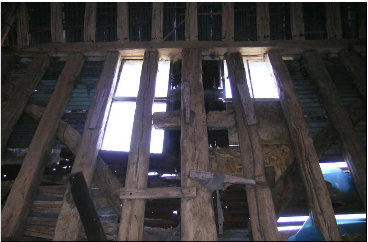
Plate 14 Empty mortices for window mullions on north-east gable
