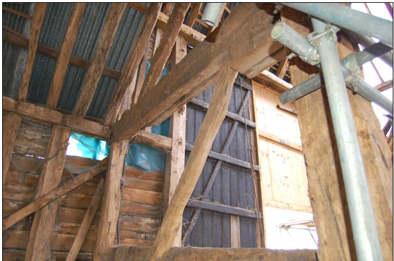
Plate 12 Wattle grooves to north-west aisle of partition with primary-braced framing in background
