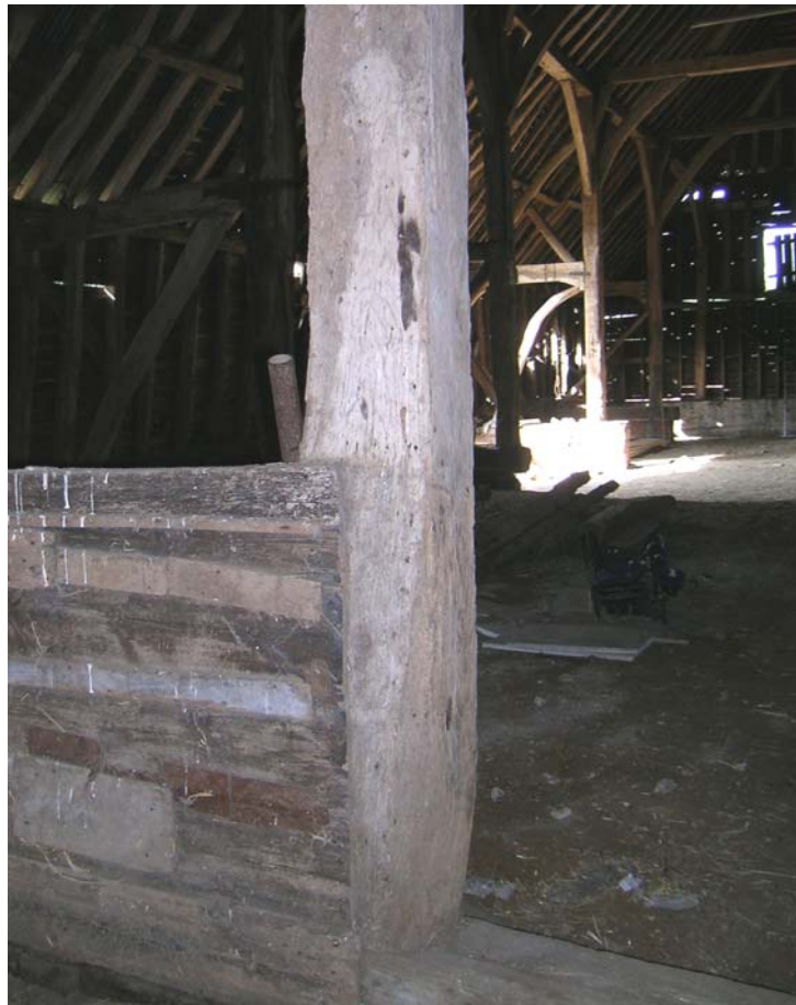
Plate 24 Rushlight burn mark on partition post
