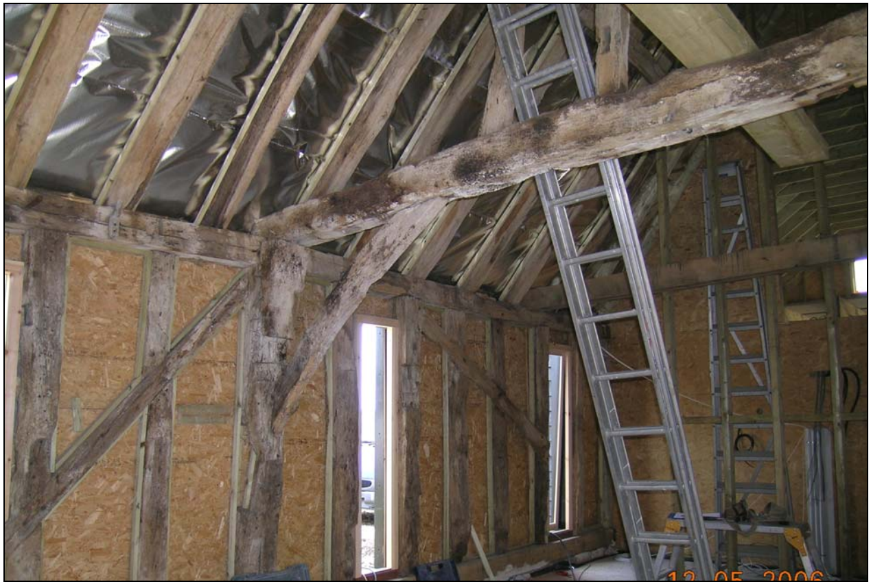
Plate 28 Comparison of internal and primary braced bays in byre
