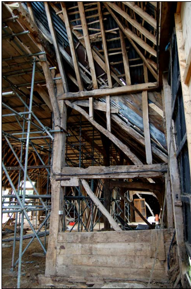
Plate 19 Typical porch construction
