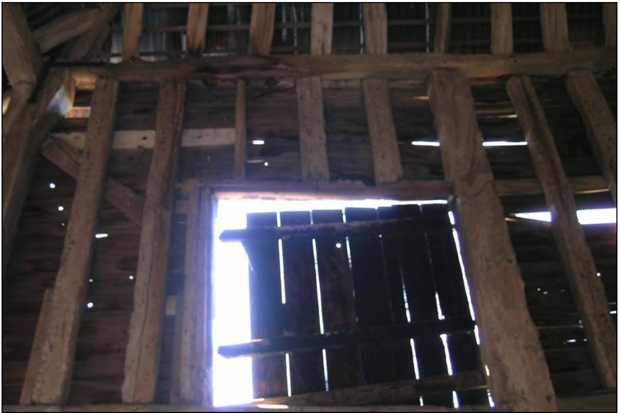
Plate 15 Pitching door inserted into mullioned window in south-west gable
