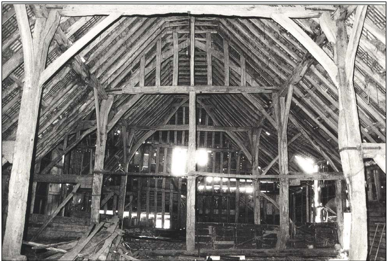
Plate 11 Remains of partition framing viewed to north-east
