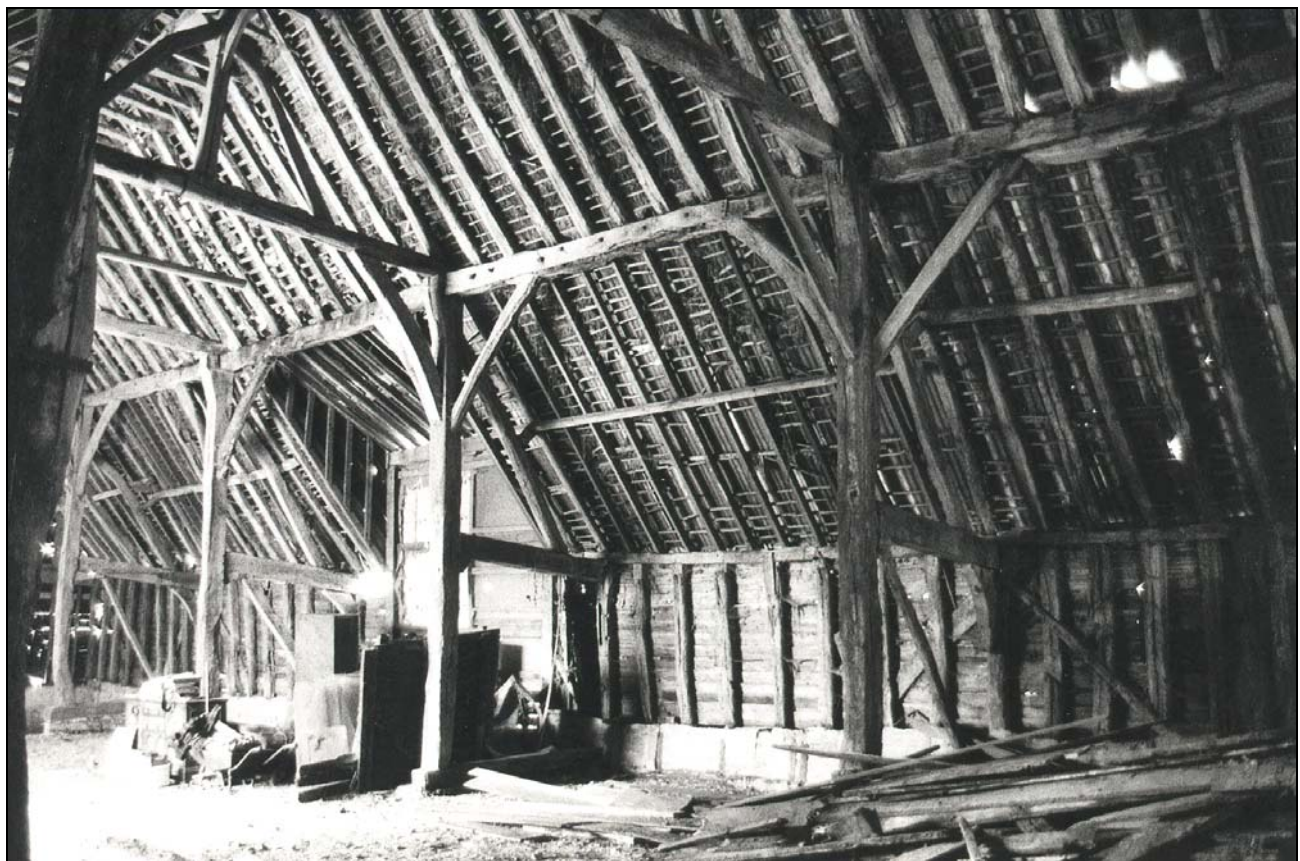
Plate 10 Comparison of external and primary braced framing on south-west wall to bays 3 and 4
