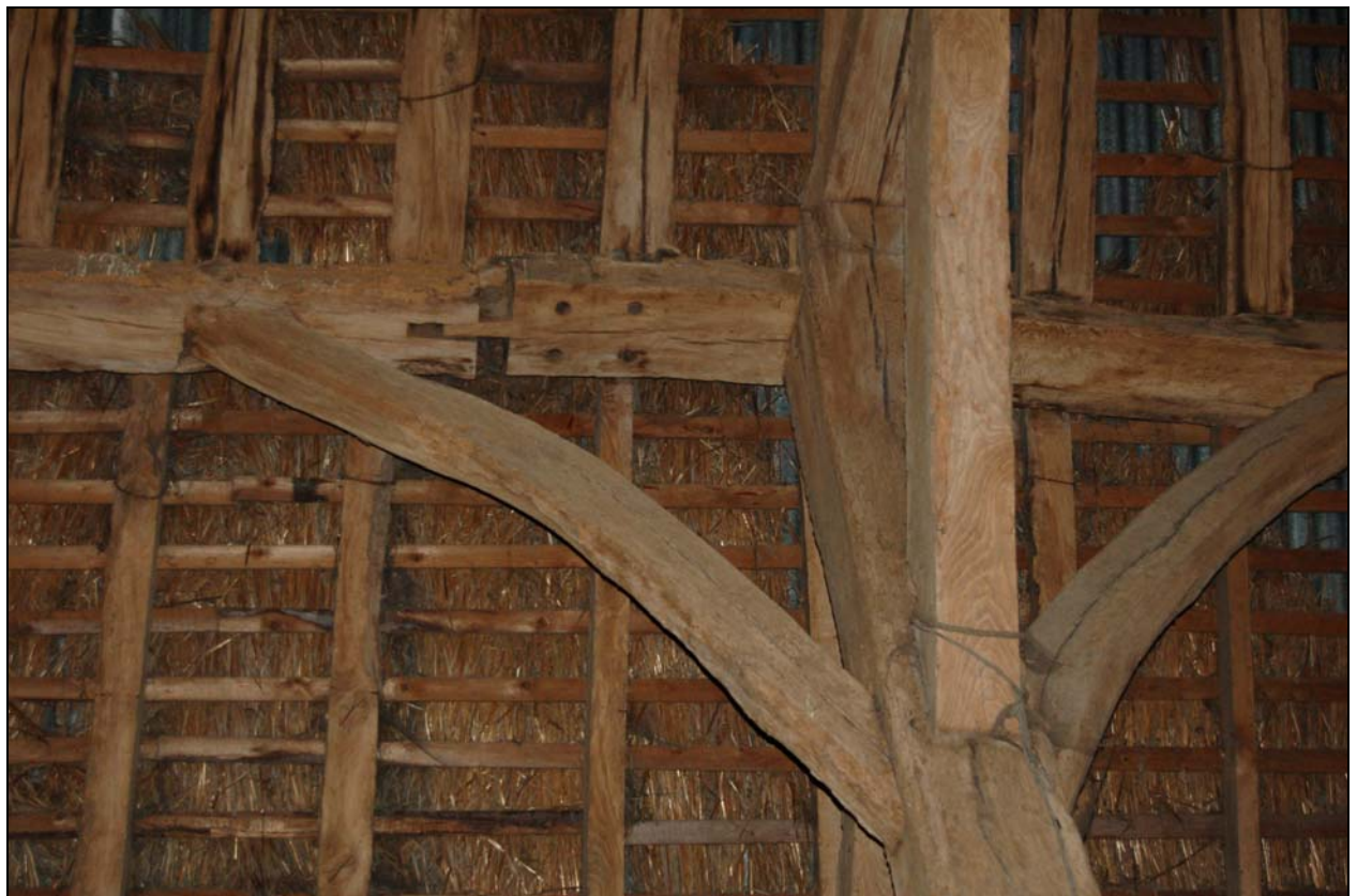
Plate 18 Typical side-halved and bridled joint in barn
