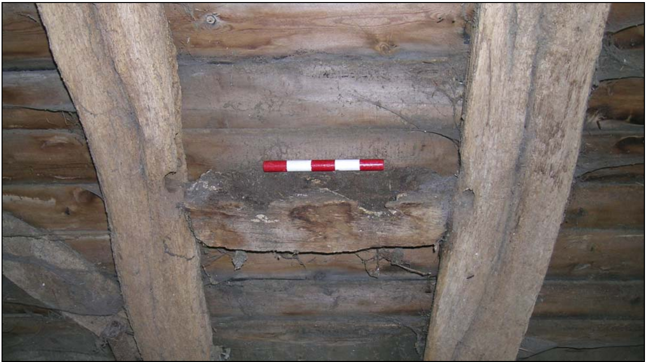
Plate 17 Remaining sill to medieval side window containing rotted diamond mullion recesses
