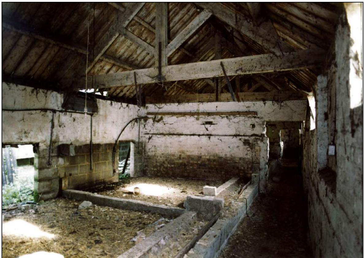
Plate 20 Converted interior of shelter shed
