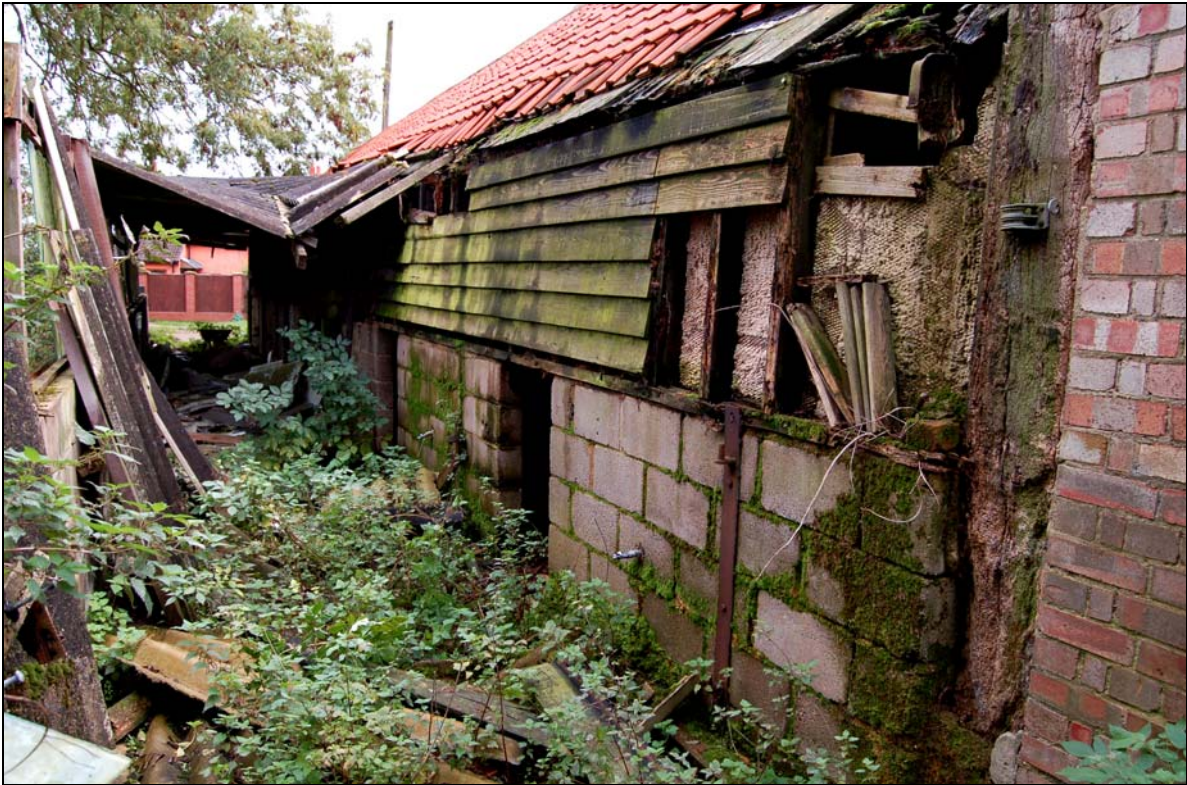
Plate 19 Exposed timber framing to shelter shed viewed from west
