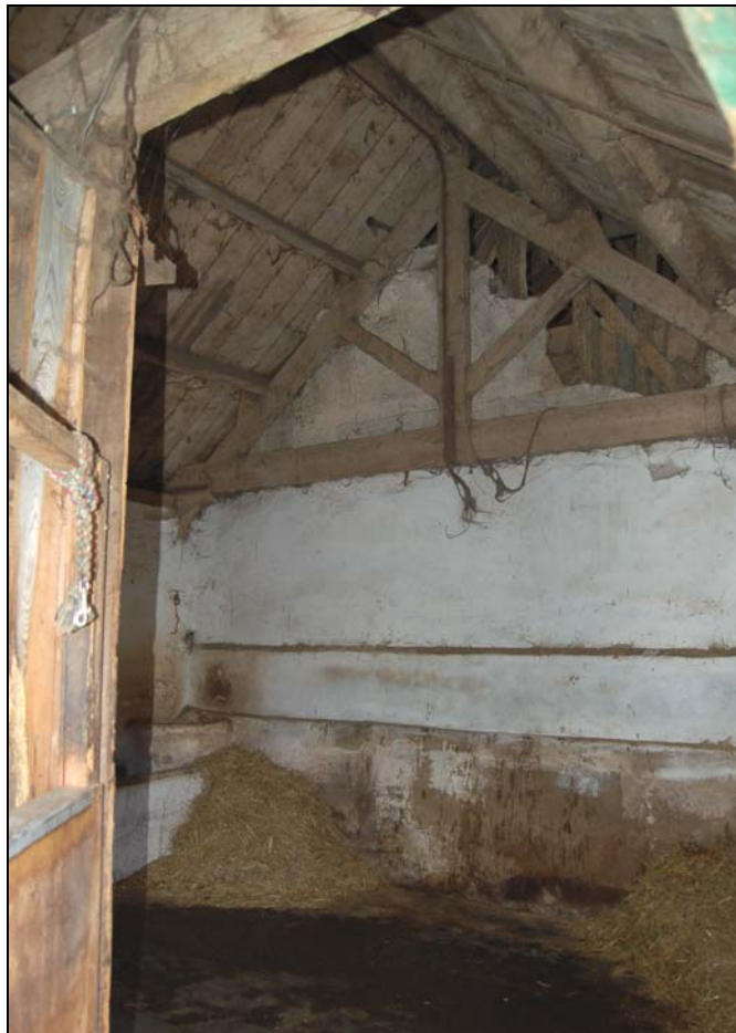
Plate 22 Interior of stable viewed from north-east
