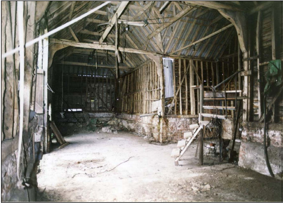
Plate 7 Interior of barn viewed from north-west
