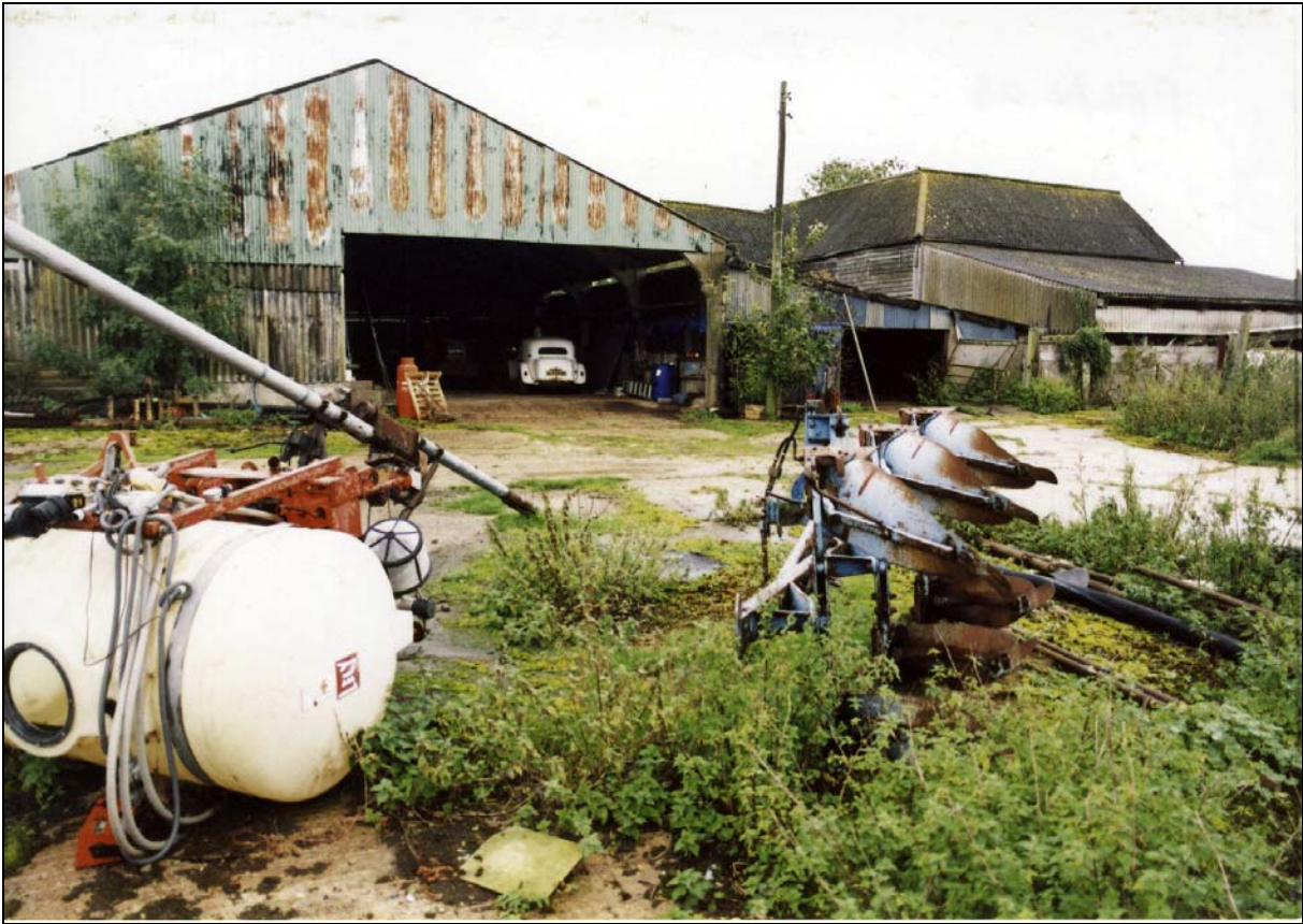
Plate 23 Modern pre-fabricated sheds viewed from south-east with barn to right
