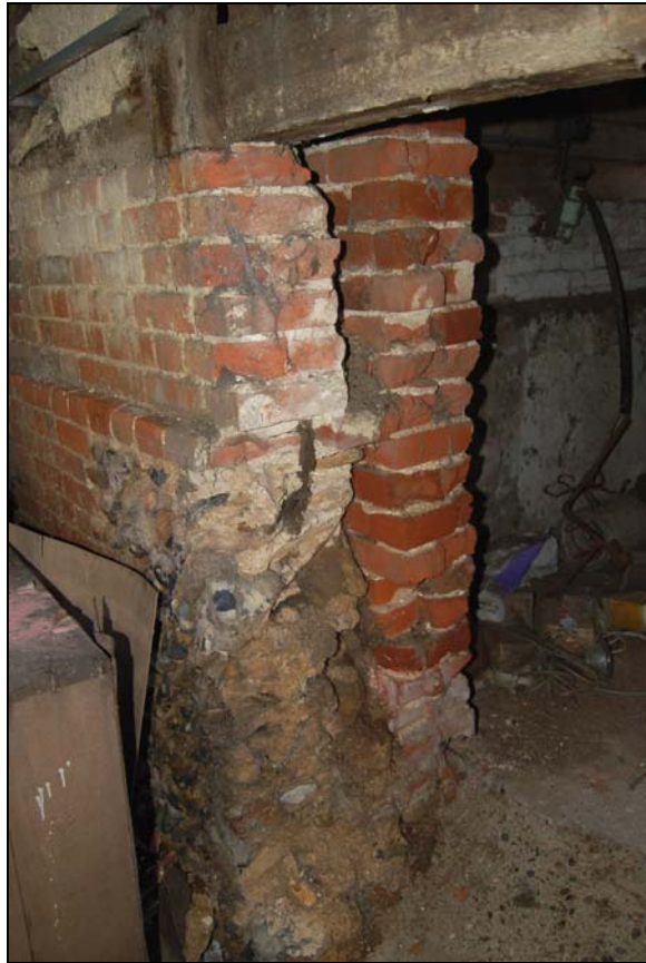
Plate 11 Detail of brickwork skin supporting first floor in granary
