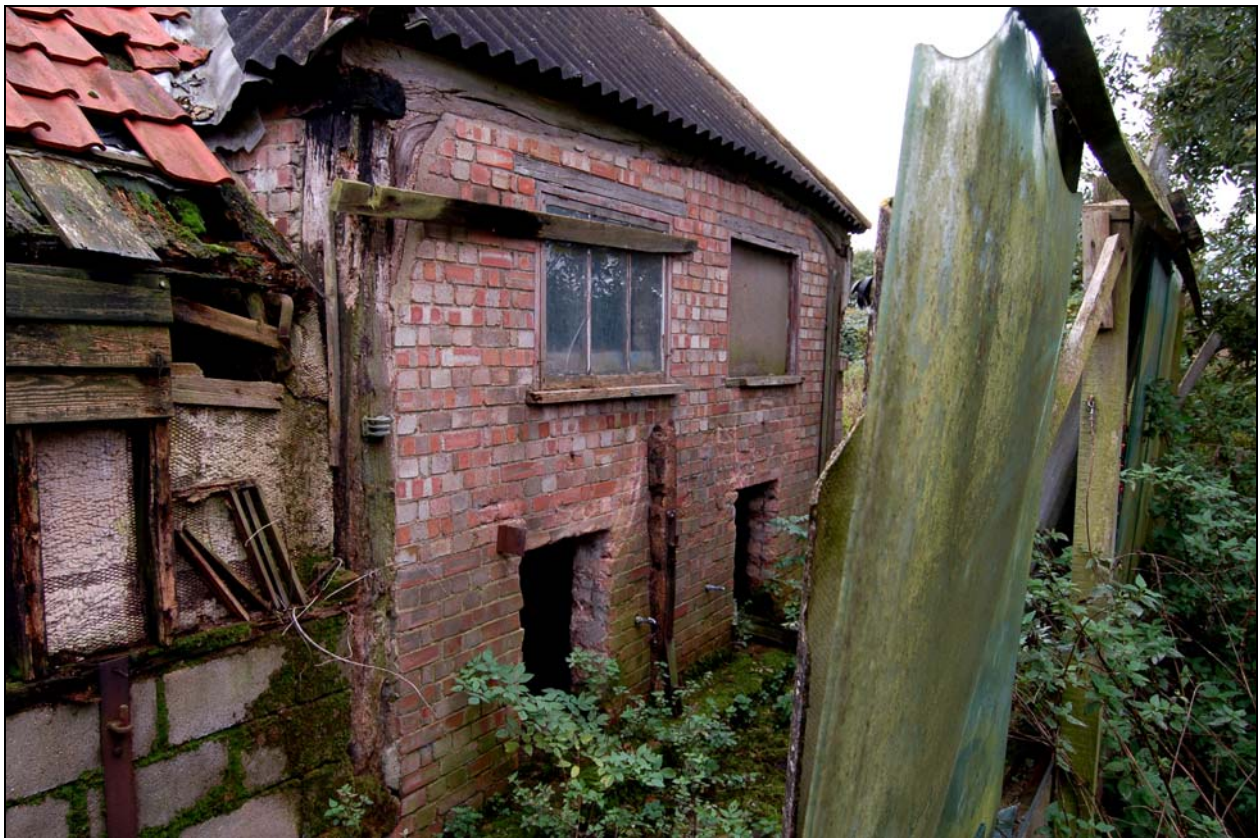
Plate 14 Brick infill to gable end of loose box viewed from north-east
