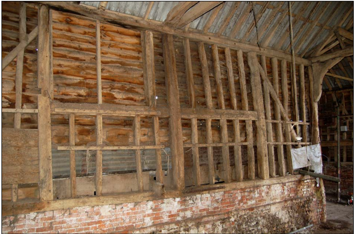
Plate 8 Reused main framing on south-west side of barn
