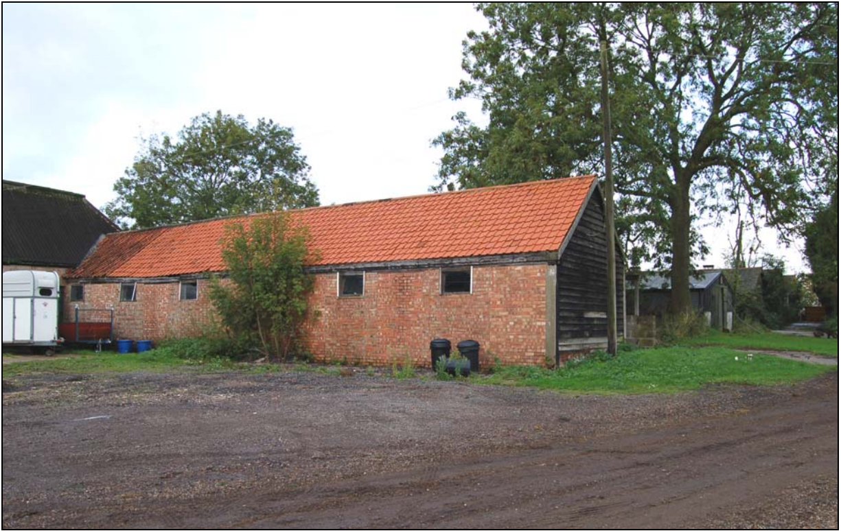
Plate 17 Shelter shed viewed from south-east
