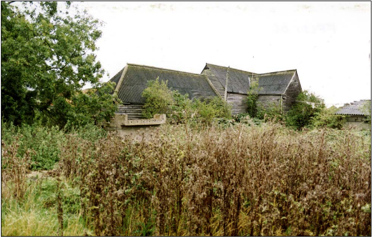
Plate 3 Farm group viewed from west
