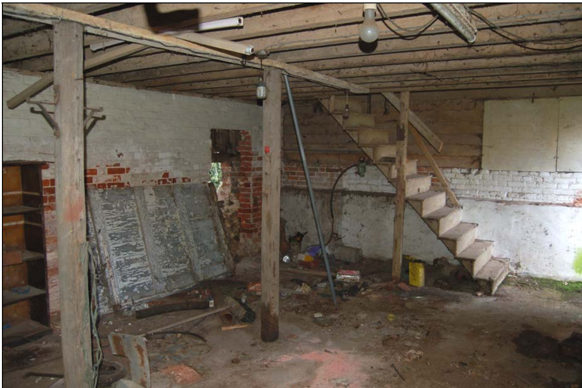
Plate 10 Ground floor of granary viewed from north
