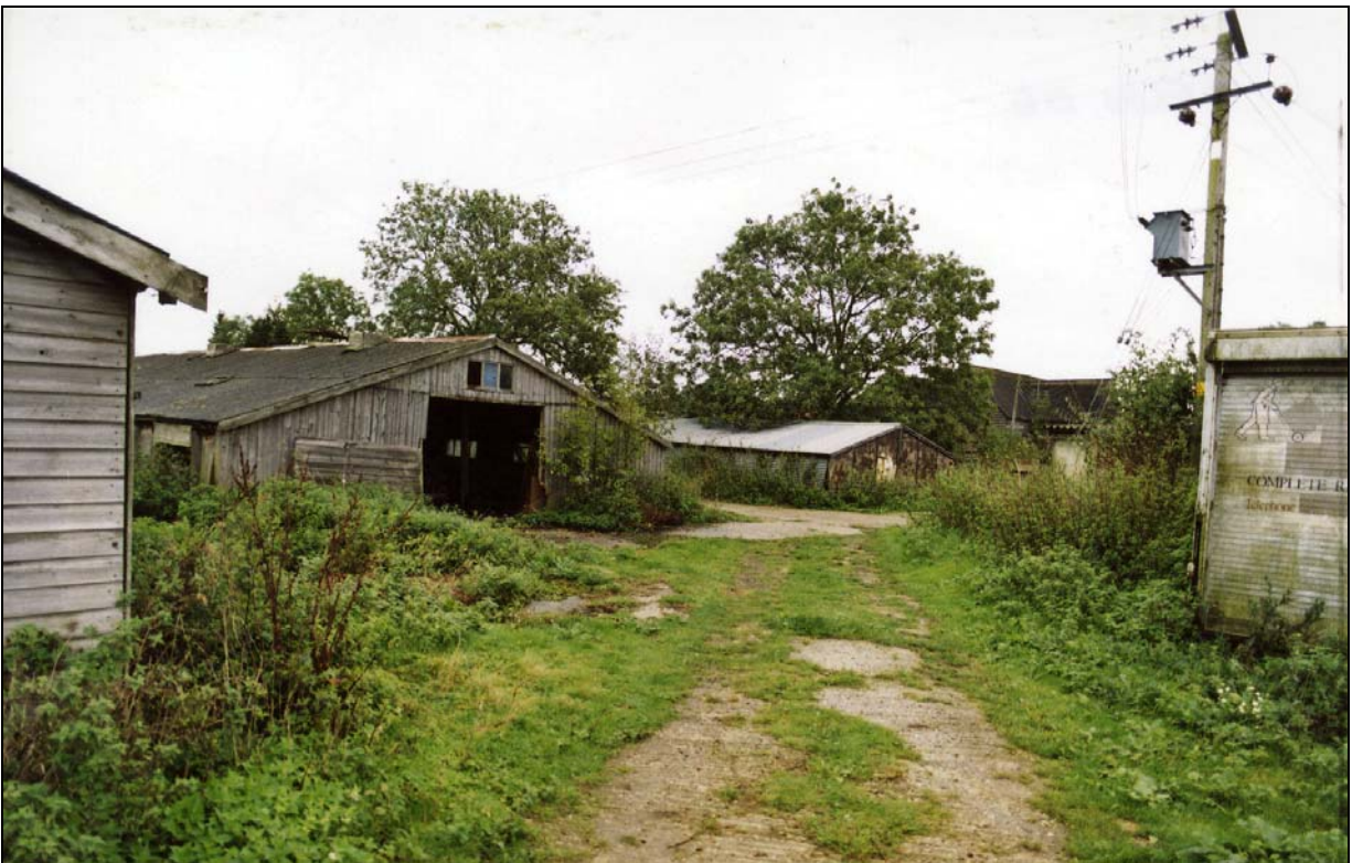
Plate 24 Battery sheds viewed from north-west, with barn centre right
