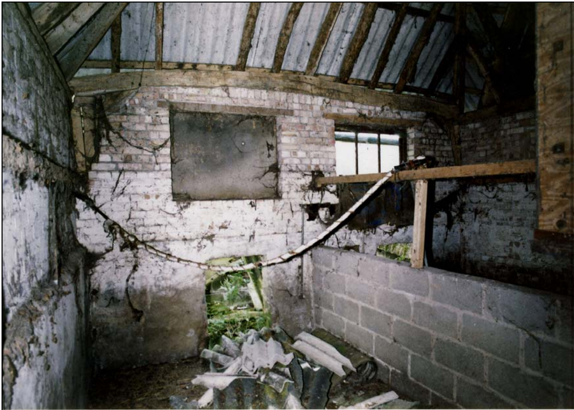
Plate 16 Interior of loose box converted to pig stalls
