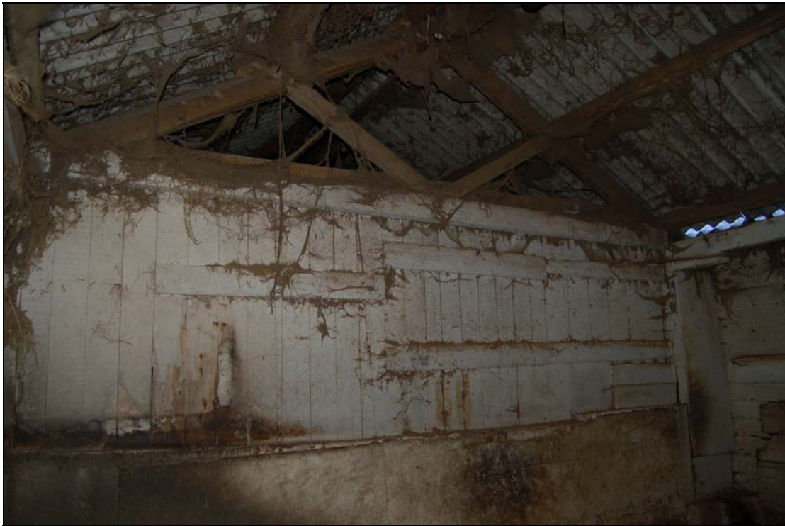
Plate 26 Reused partition inside Stables 6
