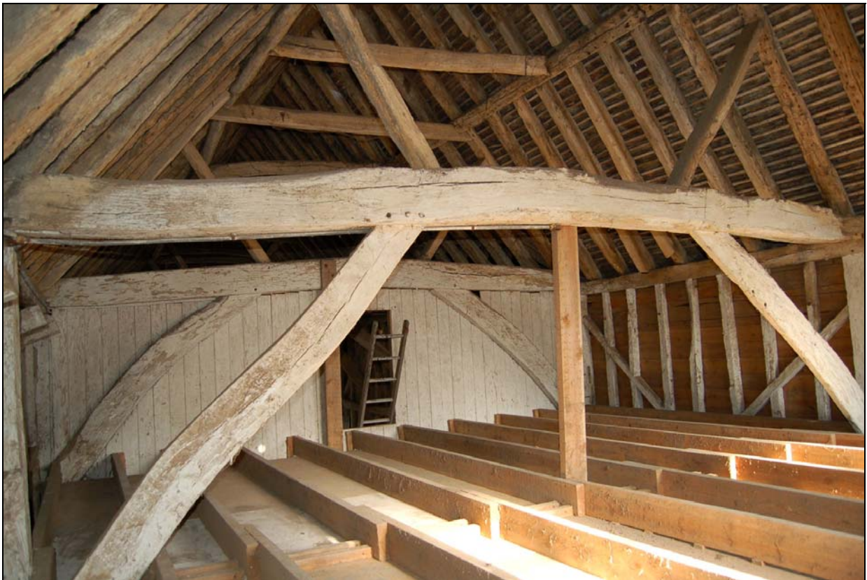
Plate 16 Roof-space above Dairy viewed from south
