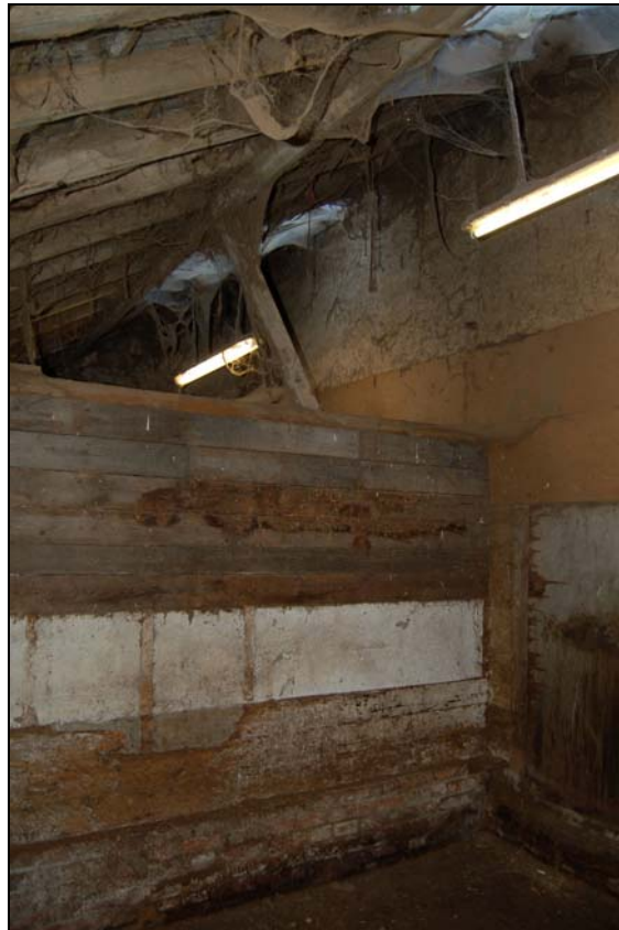
Plate 22 Interior of Stables 3 showing external daub render to Barn
