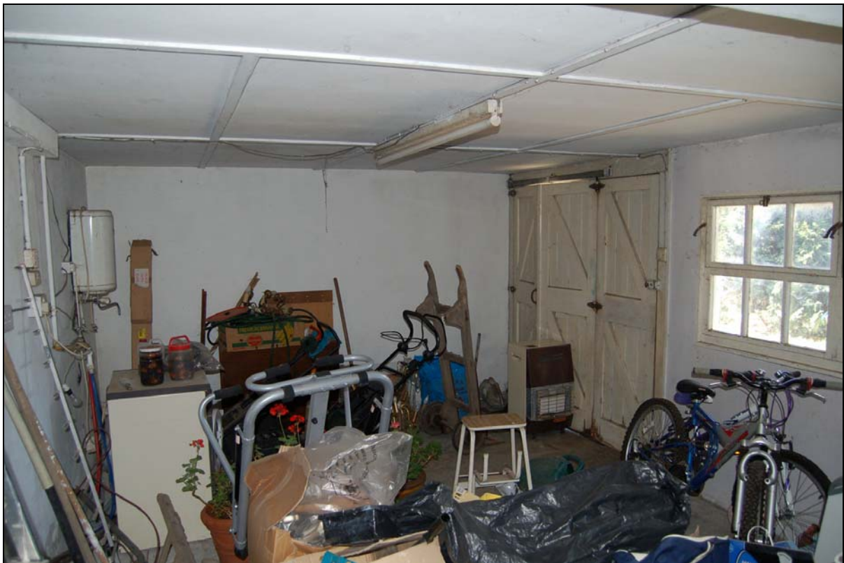
Plate 18 Interior of Stable 2a viewed toward cow doors
