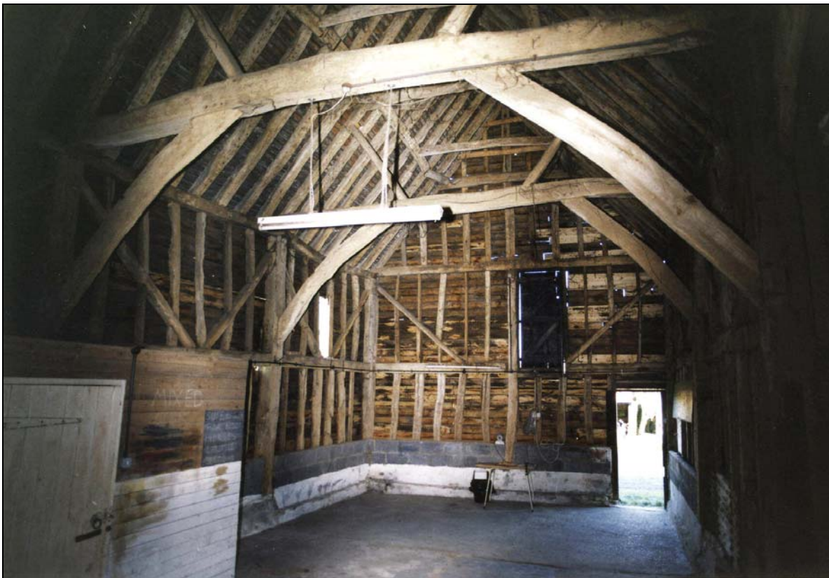
Plate 8 Interior of Barn viewed from south-east
