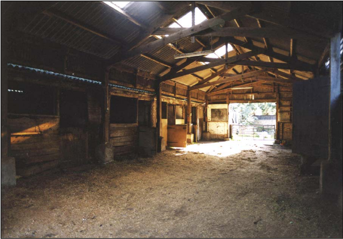
Plate 25 Interior of Covered Yard viewed toward south-east (Stables 6)
