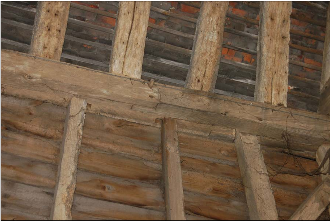
Plate 10 Typical edge-halved and bladed scarf joint in wall plate
