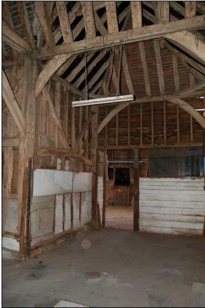
Plate 13 Barn porch viewed from south-west to Covered Yard
