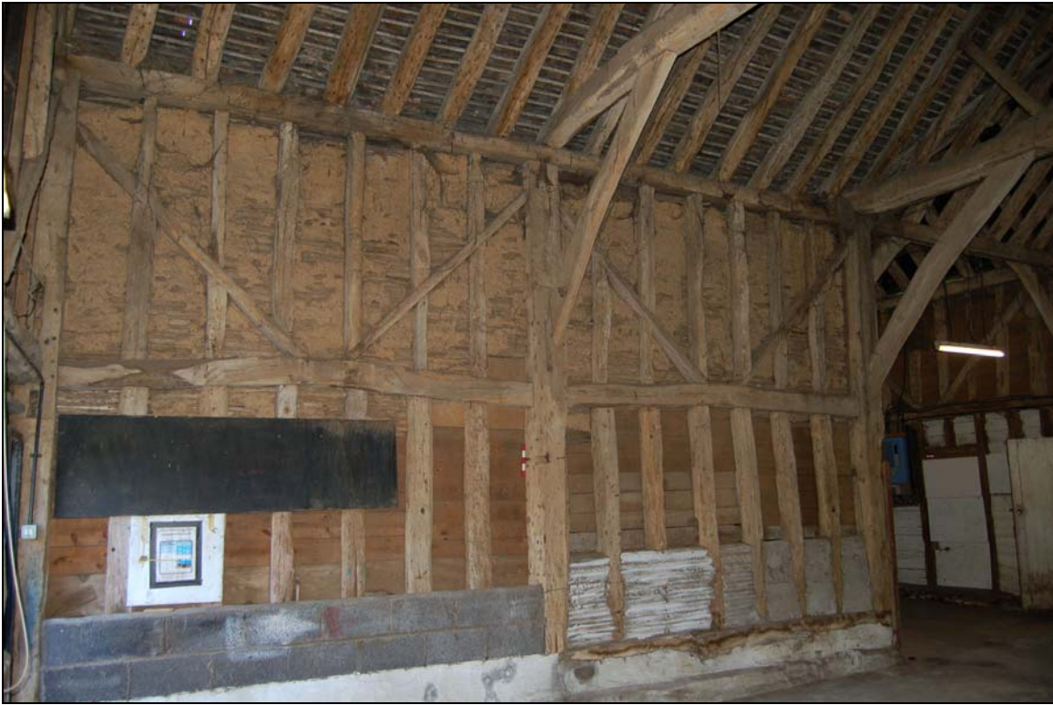
Plate 9 Variations in wall framing between upper and lower registers in bays 1 & 2 east
