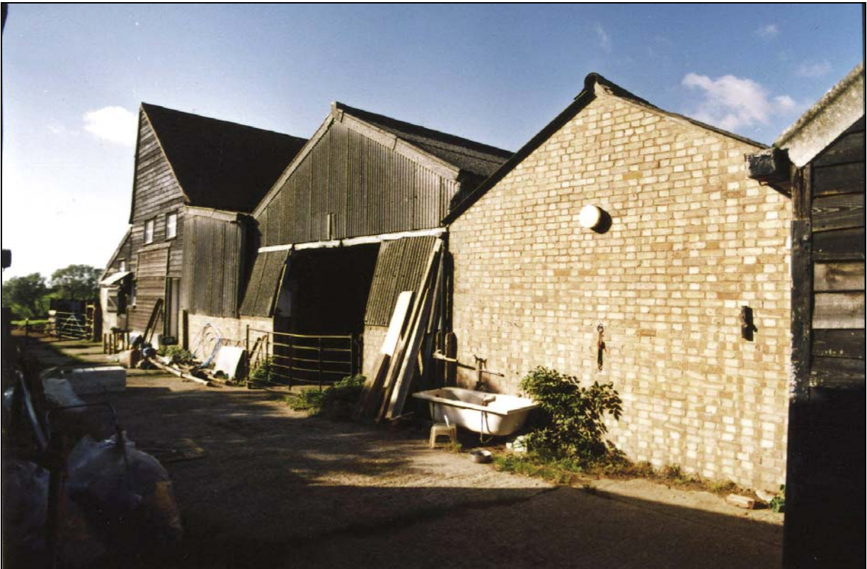
Plate 2 Barn and Covered Yard viewed from south-east
