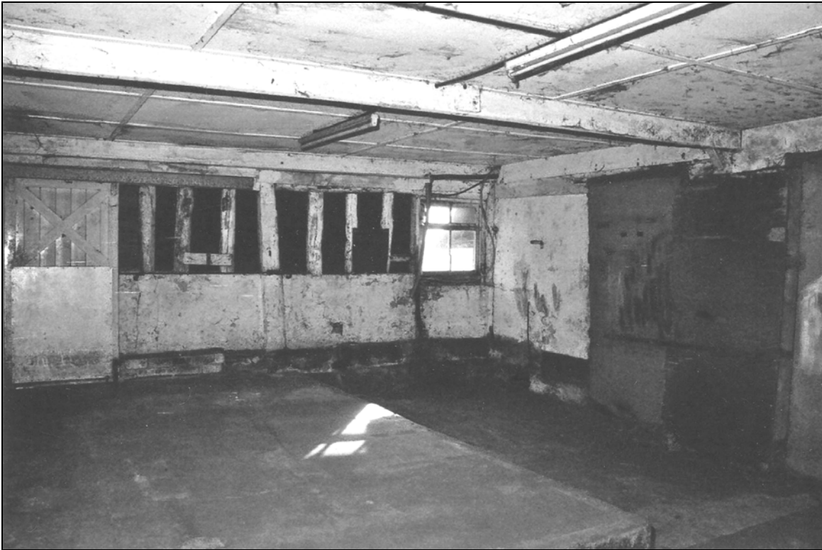
Plate 15 Interior of Dairy viewed from north-east
