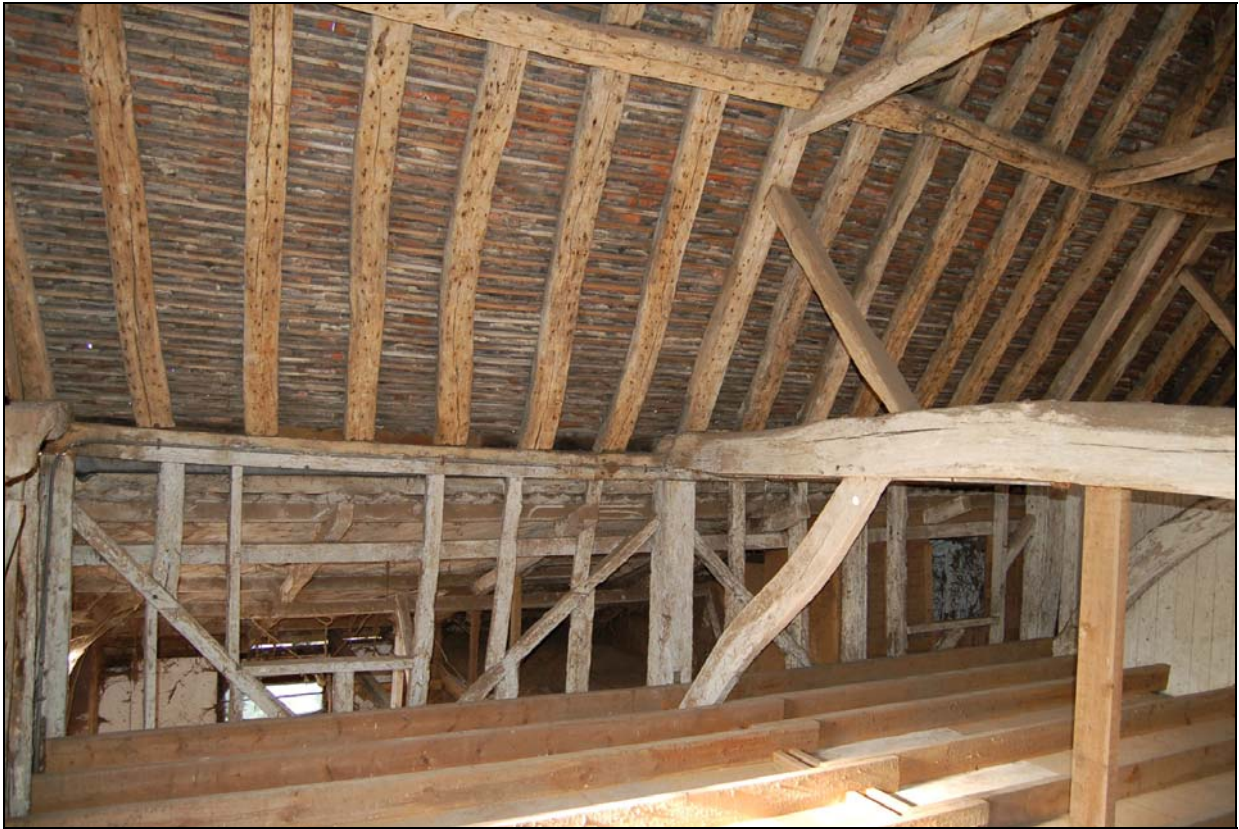
Plate 17 Openings on bays 4 & 5 south-west wall of Barn
