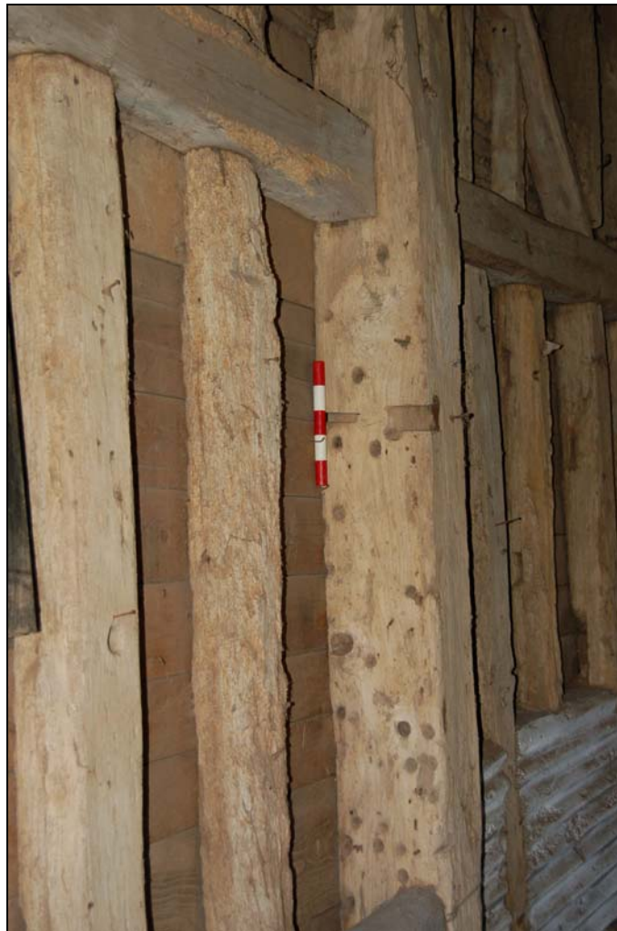
Plate 12 Possible reused ship's timber
