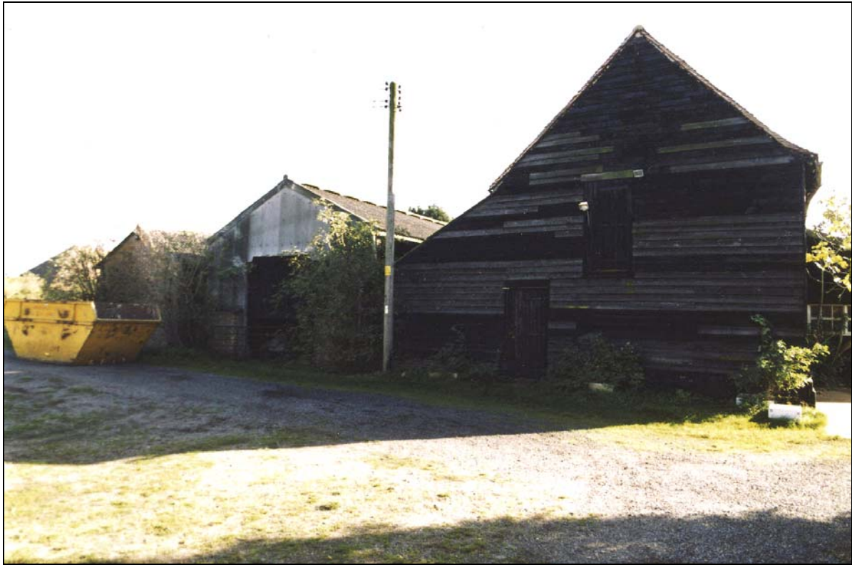
Plate 3 Barn and Covered Yard viewed from north-west
