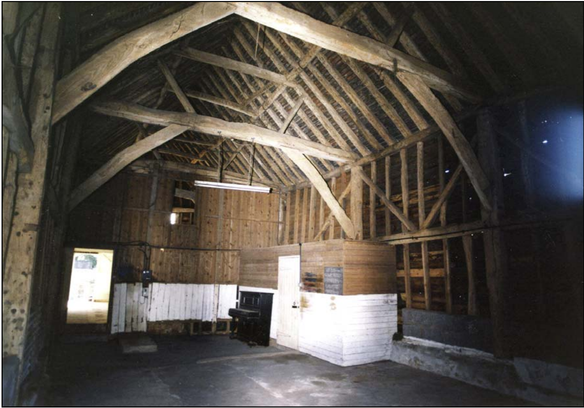
Plate 7 Interior of Barn viewed from north
