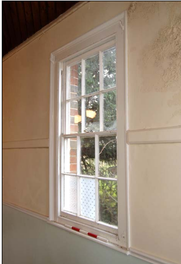
Plate 11 Window detail inside main hall
