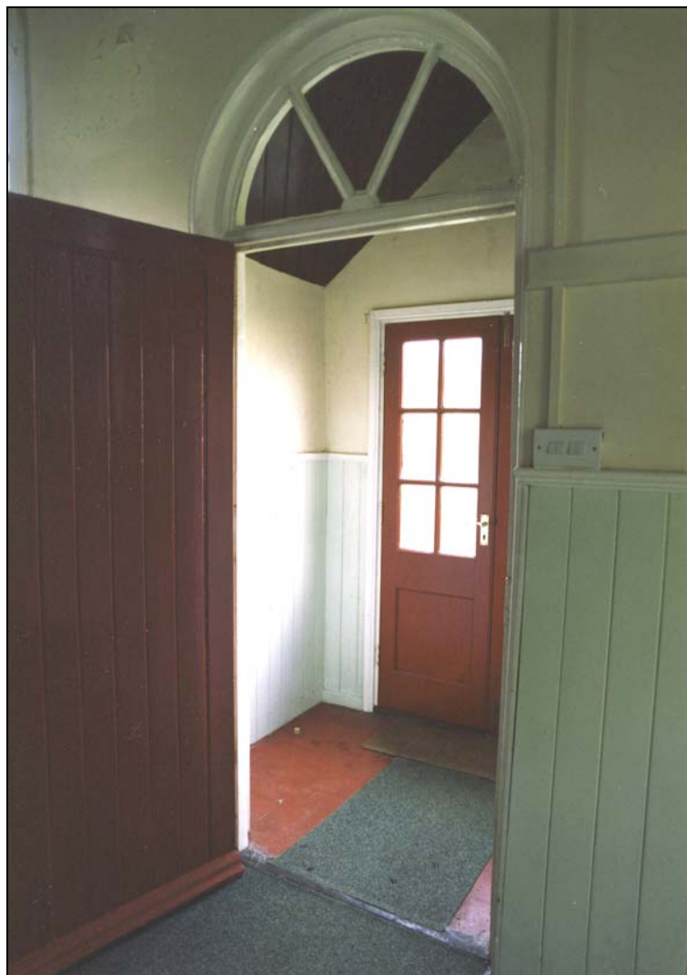
Plate 6 Interior of porch viewed from main hall
