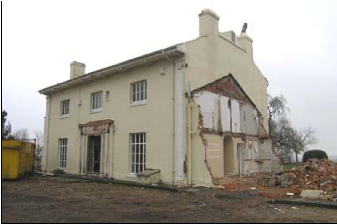
Plate 1 Main (north) elevation and demolished west wing
