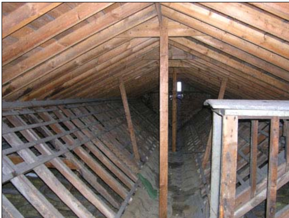
Plate 14 View inside roofspace toward west
