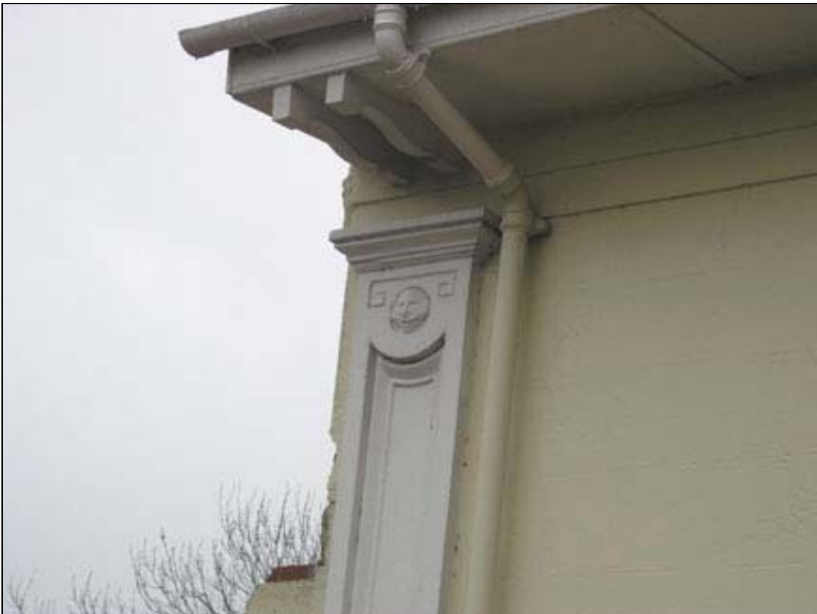
Plate 4 Pilaster carving on main elevation
