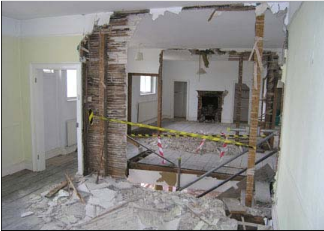
Plate 11 View from bedroom 7 to bedroom 9
