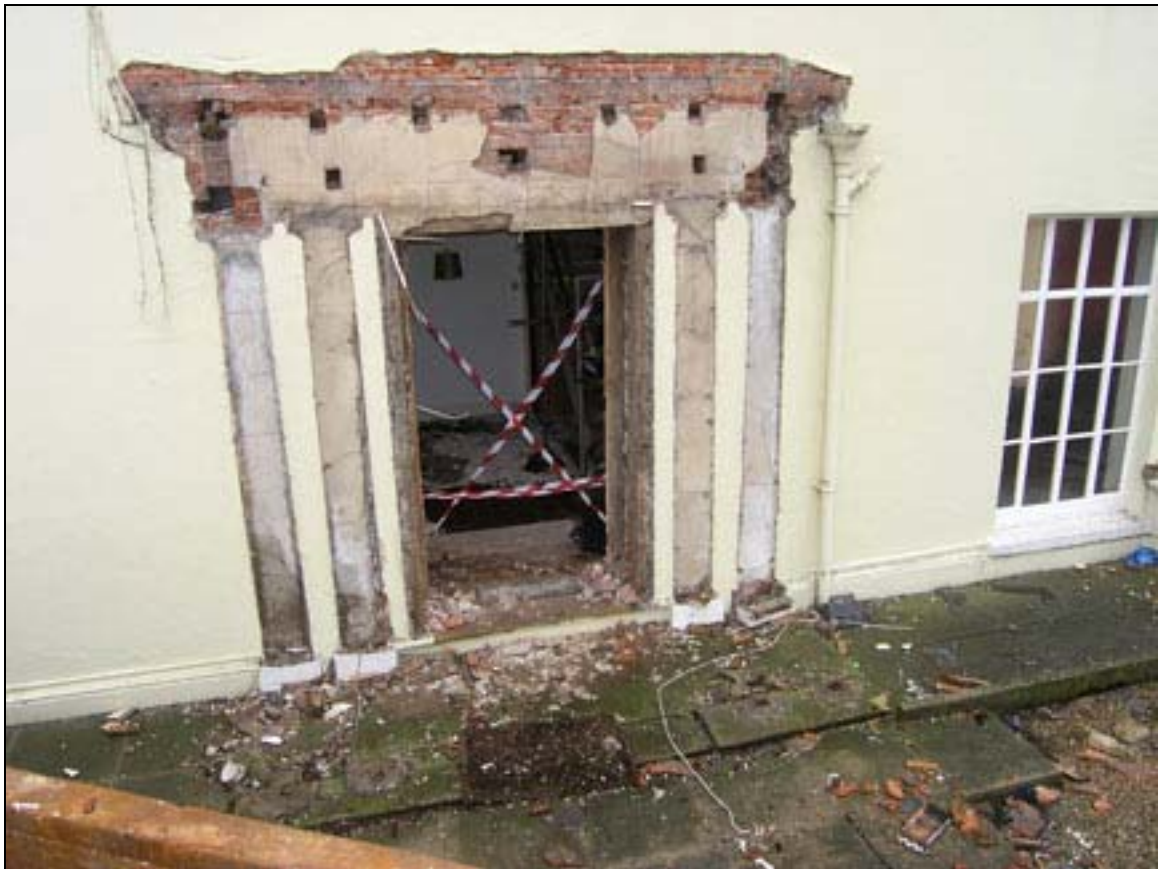
Plate 2 Scar of removed portico on main elevation
