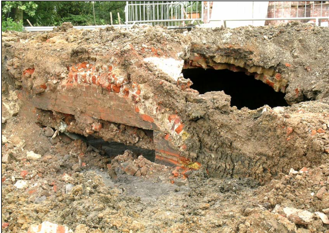
Plate 15 Underground brick chamber with roof intact
