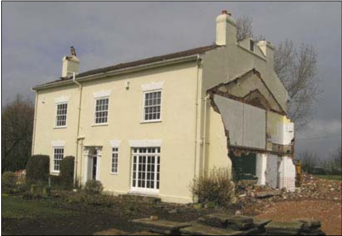
Plate 5 South elevation and demolished east wing
