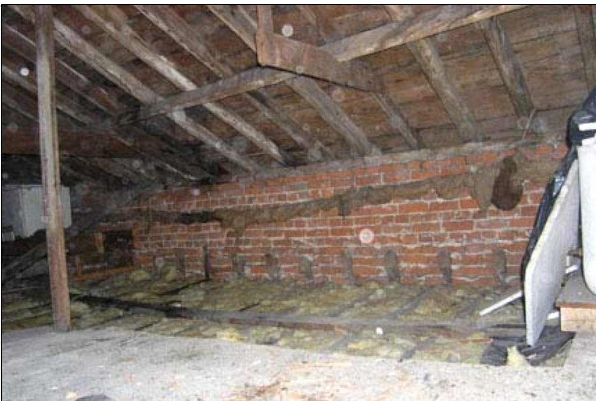
Plate 13 Parapet seen inside roofspace, with sawn-through original rafters
