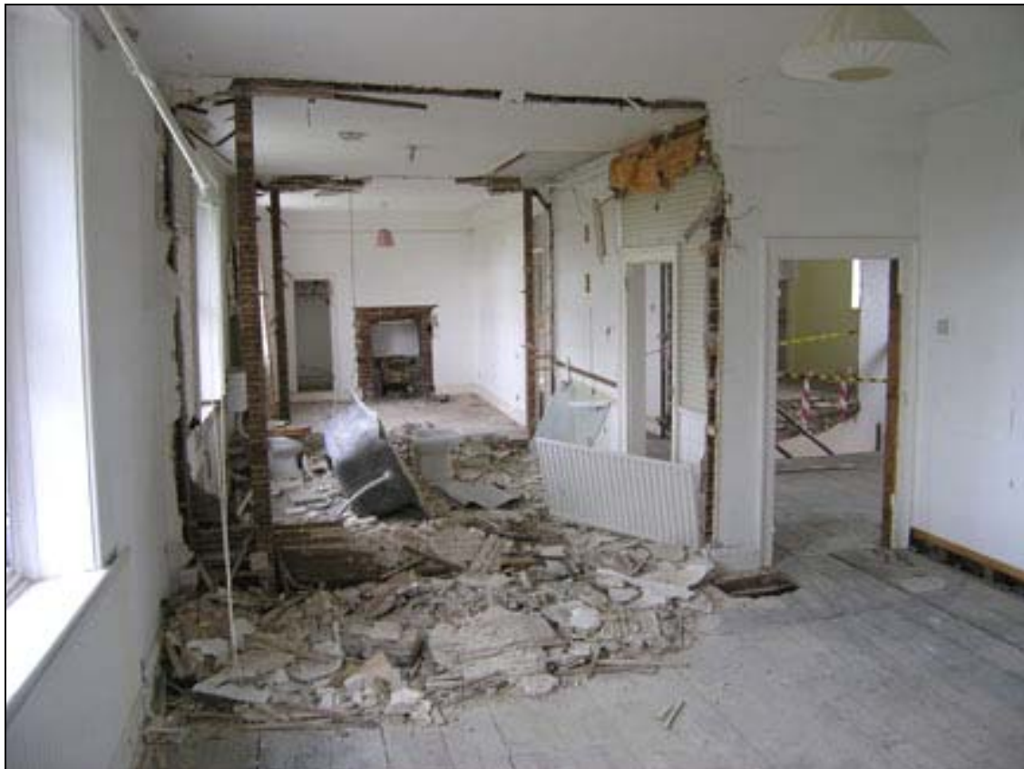
Plate 10 View from bedroom 10 to bedroom 12
