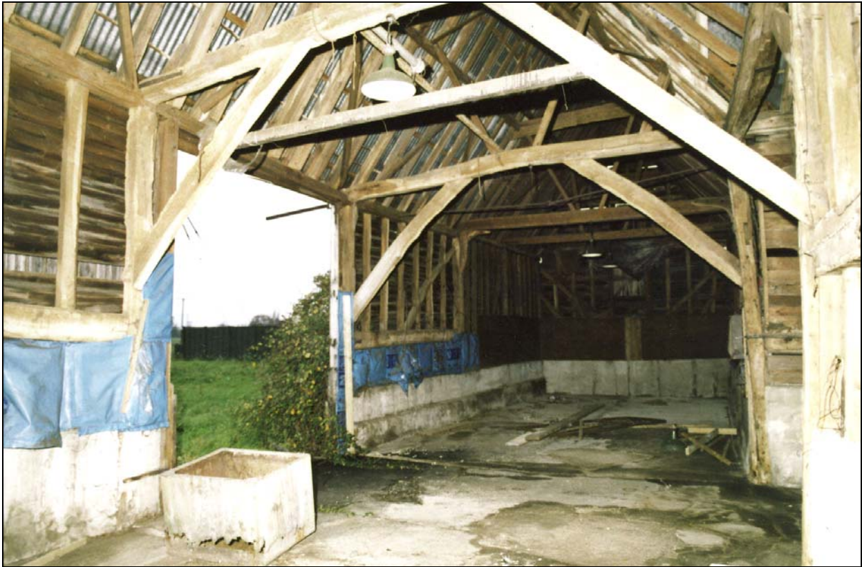
Plate 7 Barn interior viewed to rebuilt north end
