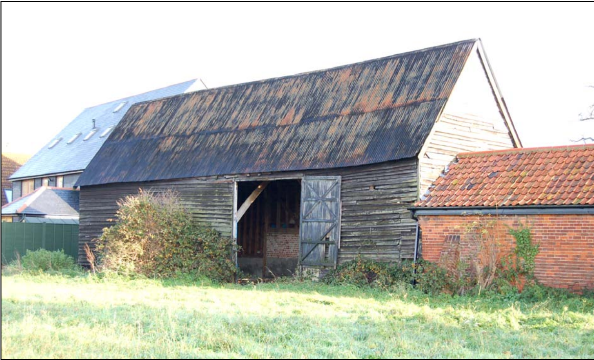
Plate 5 West elevation of barn
