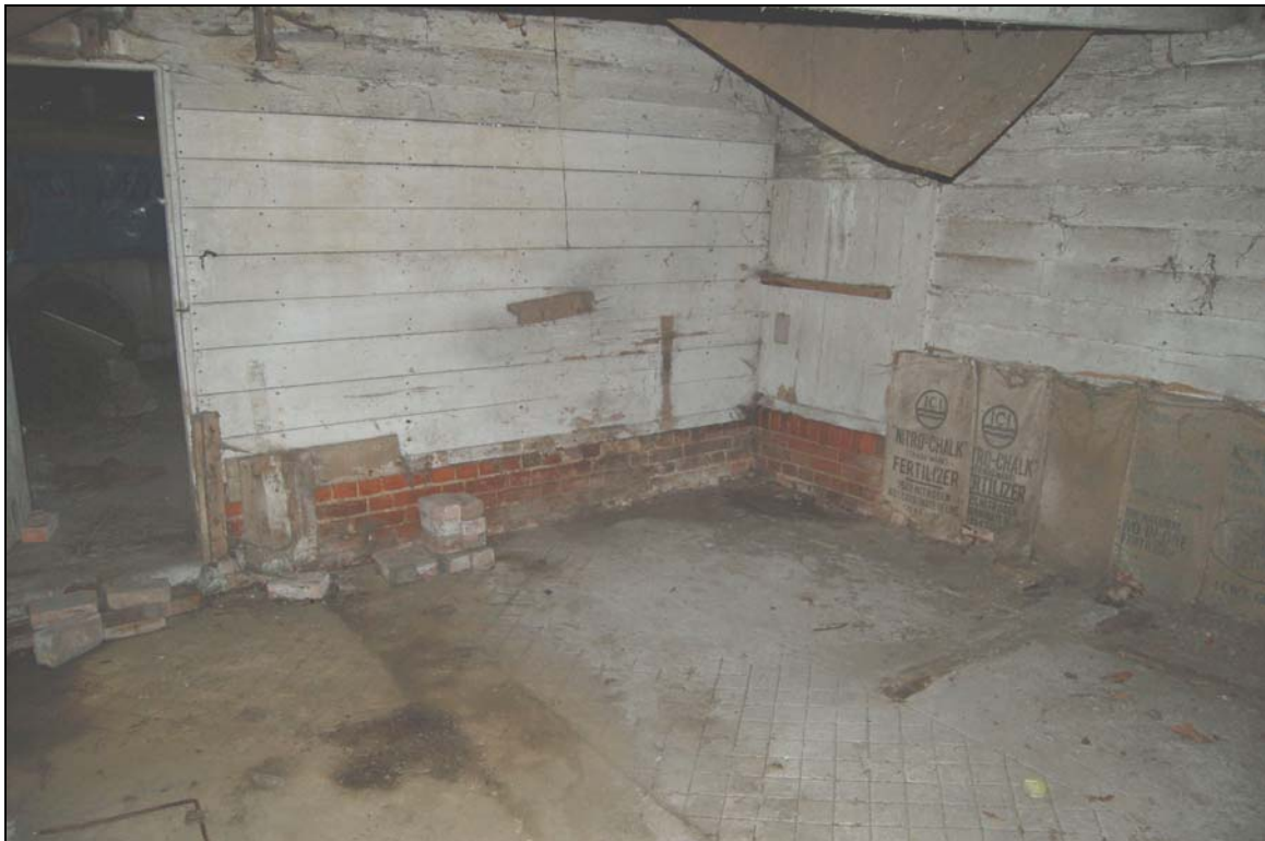
Plate 10 Interior of loose box 2
