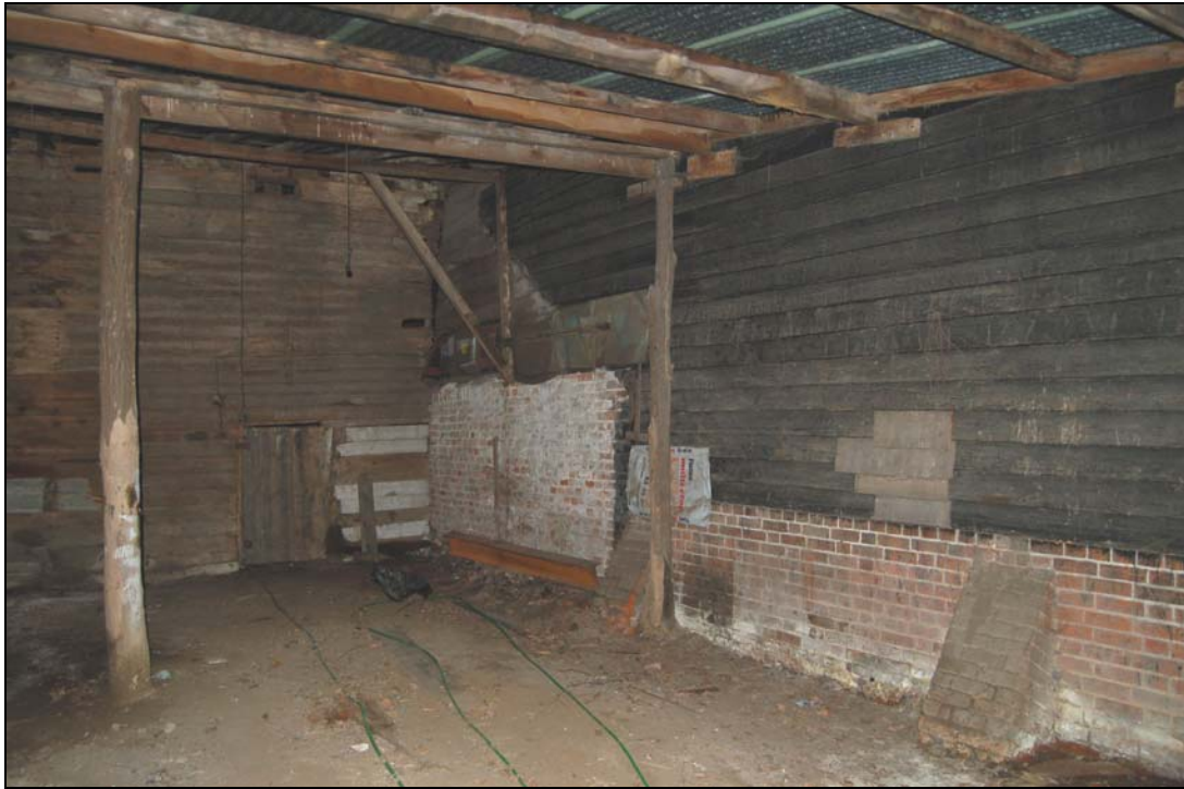
Plate 3 Barn extension and evidence for former cowhouse viewed inside pole barn
