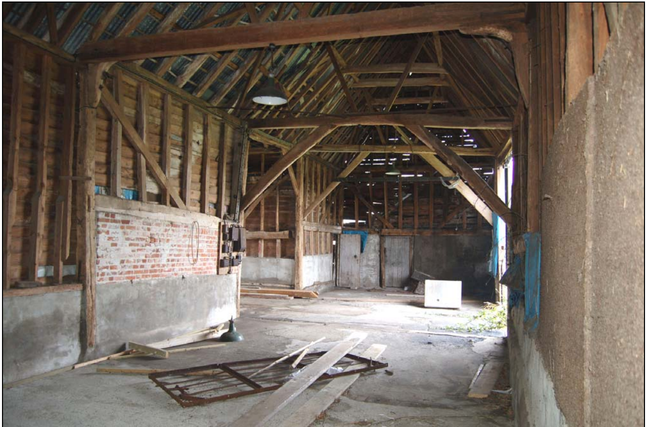
Plate 6 Barn interior viewed to south end
