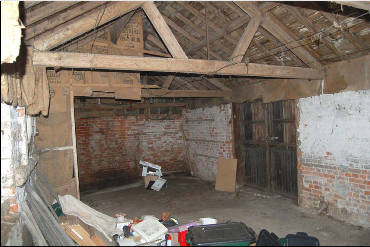
Plate 19 Interior of cowhouse 5 showing exposed brick floor by cow doors
