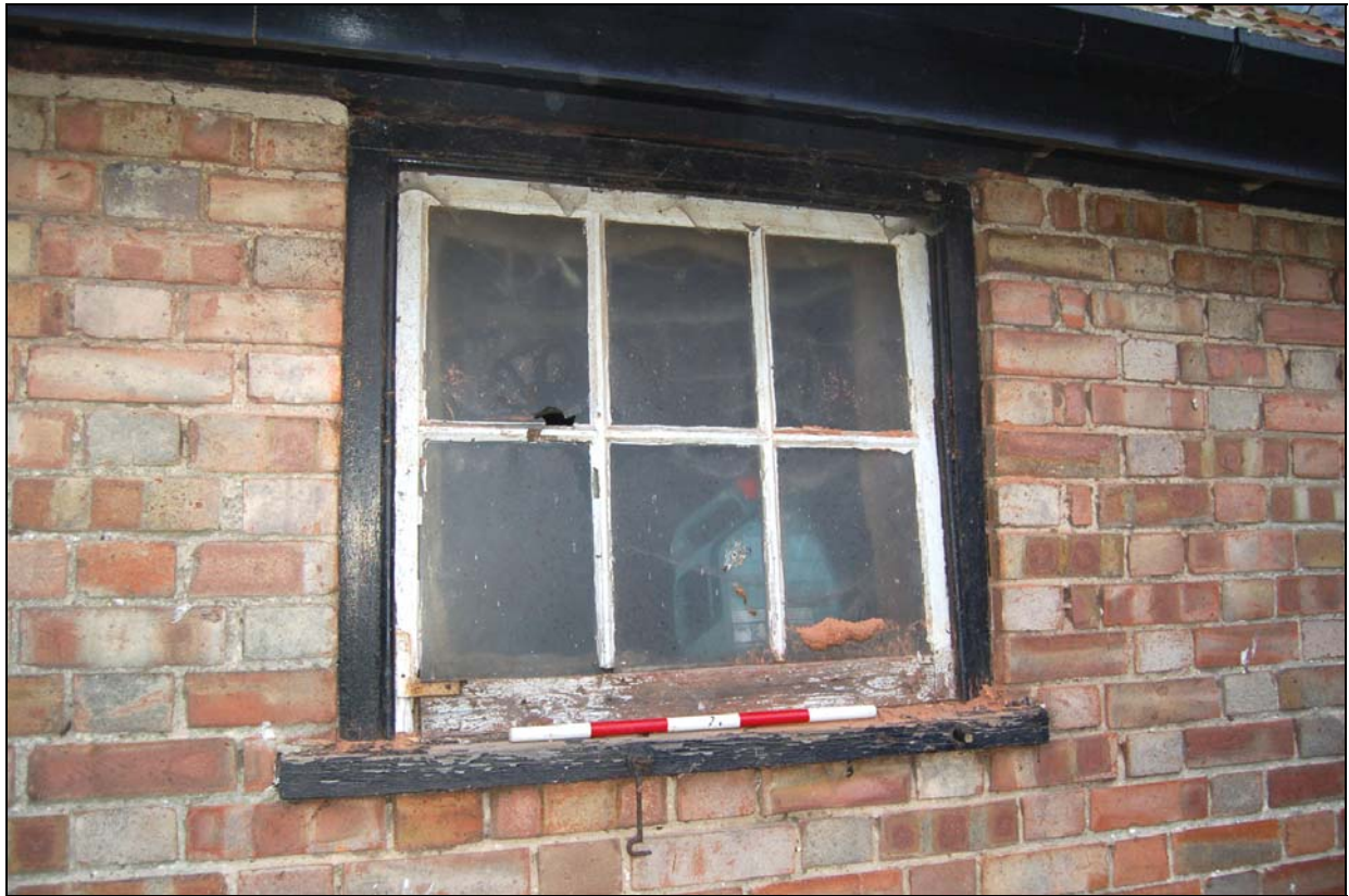
Plate 22 Typical cowhouse 6 window set within later brickwork
