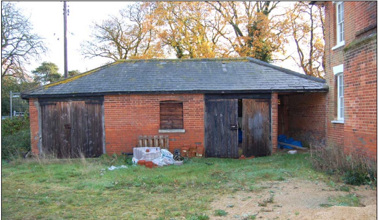
Plate 26 West elevation of wagon house/stables
