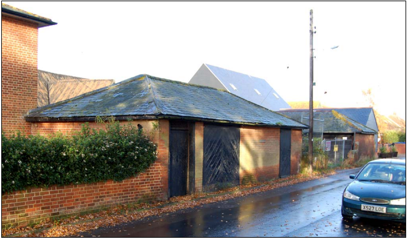
Plate 27 Wagon house/stables viewed from road
