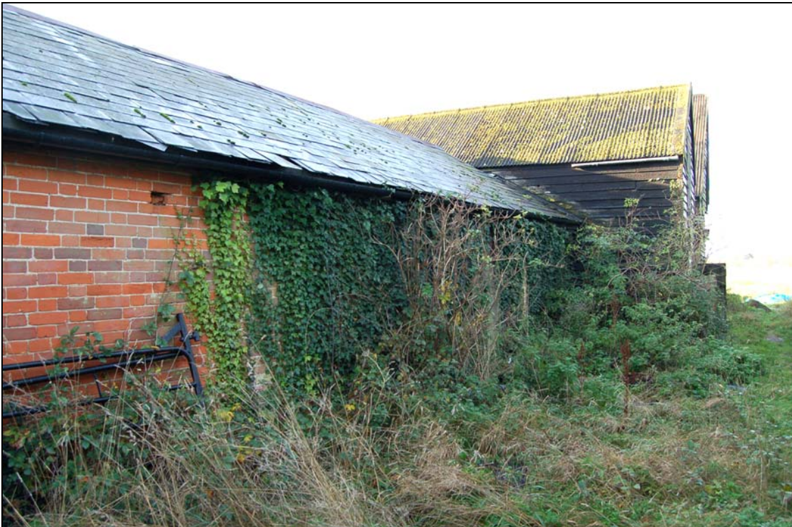
Plate 18 Rear of cowhouse 5 and overgrown cow doors
