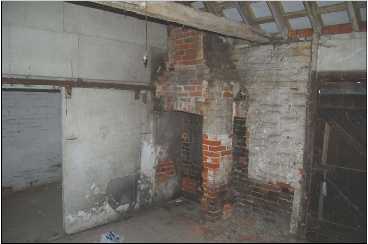
Plate 25 Interior of probable washhouse at southern end of cowhouse 6
