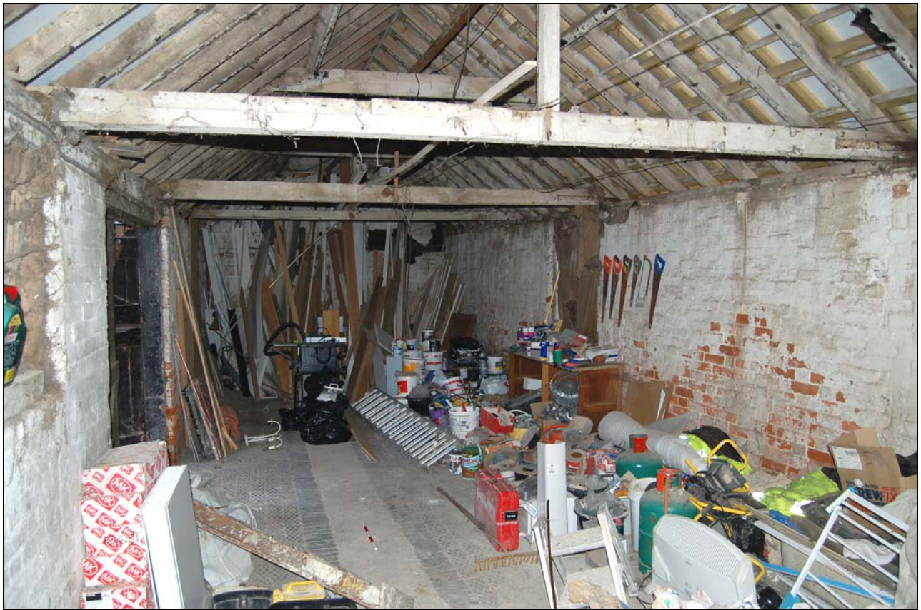
Plate 24 Interior of cowhouse 6 viewed to south
