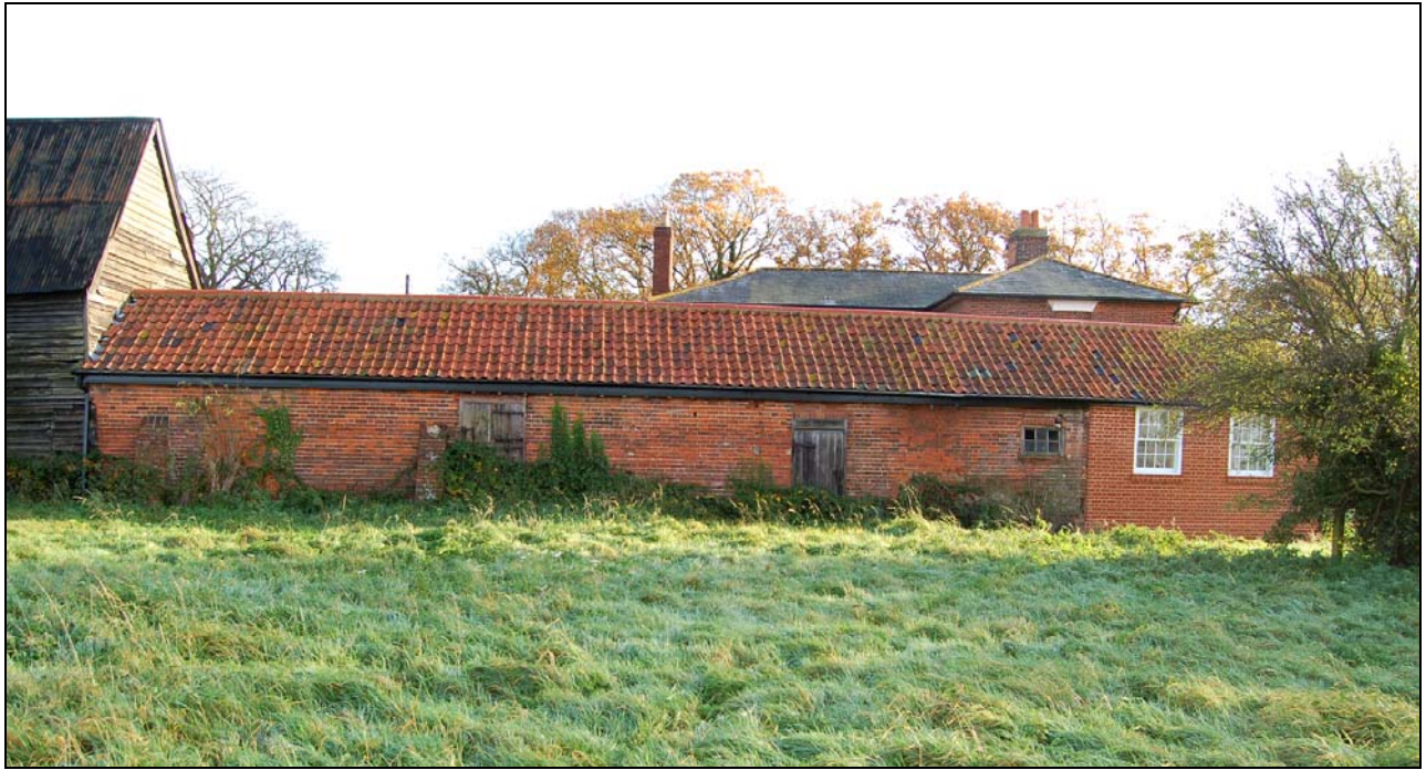
Plate 23 Rear (west) elevation of cowhouse 6
