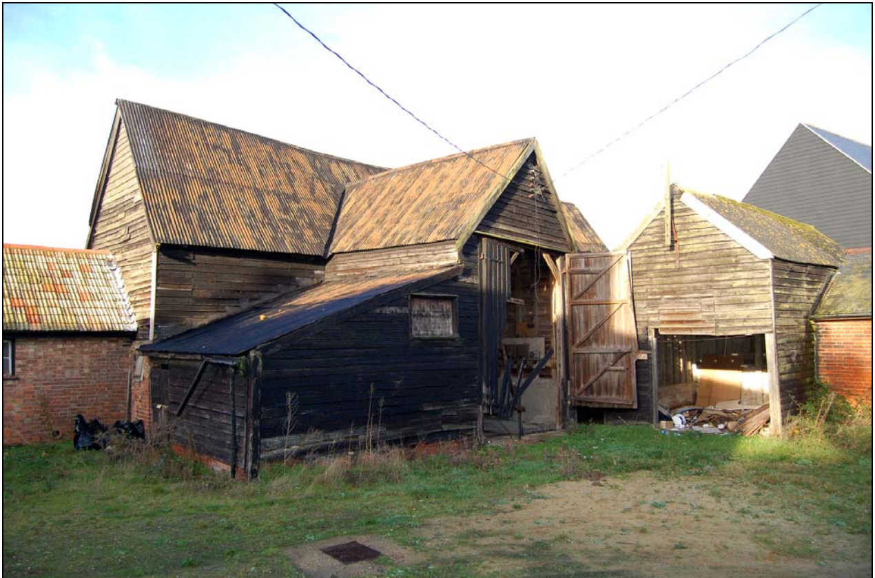
Plate 2 Barn viewed from yard
