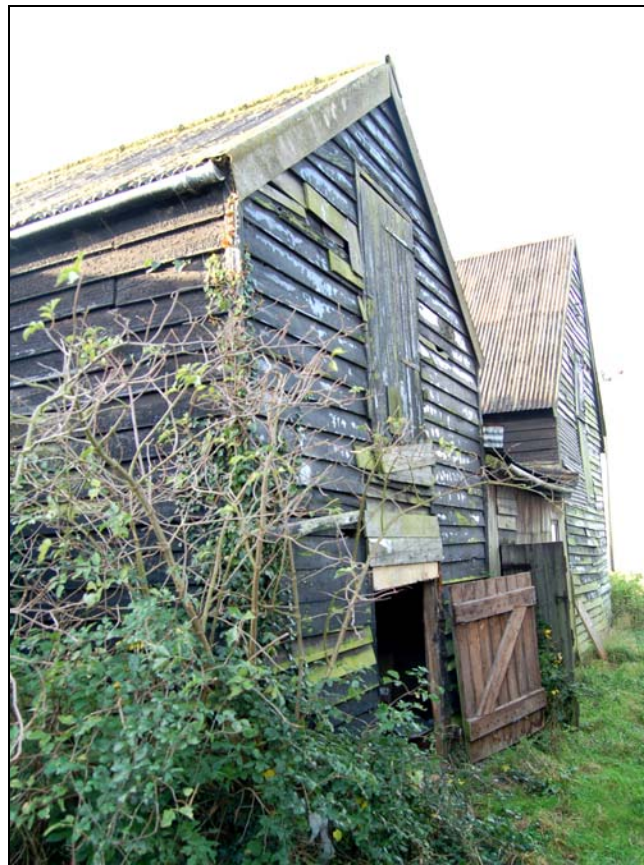
Plate 12 North front of granary with first floor taking-in door
